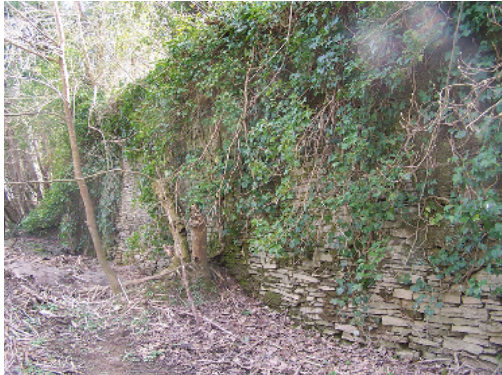
Figure 3: Retaining Wall (1) which defines the eastern boundary of the works (RCAHMMW: 2006_113_001)
