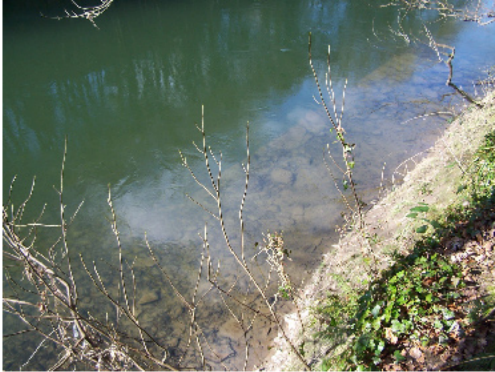
Figure 10: Section of apron quay below the water line (RCAHMW: 2006_111_003)
