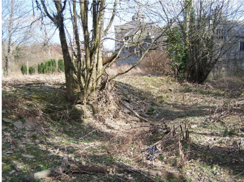
Figure 6: Remains of retaining wall 2 (RCAHMW: 2006_108_001)
