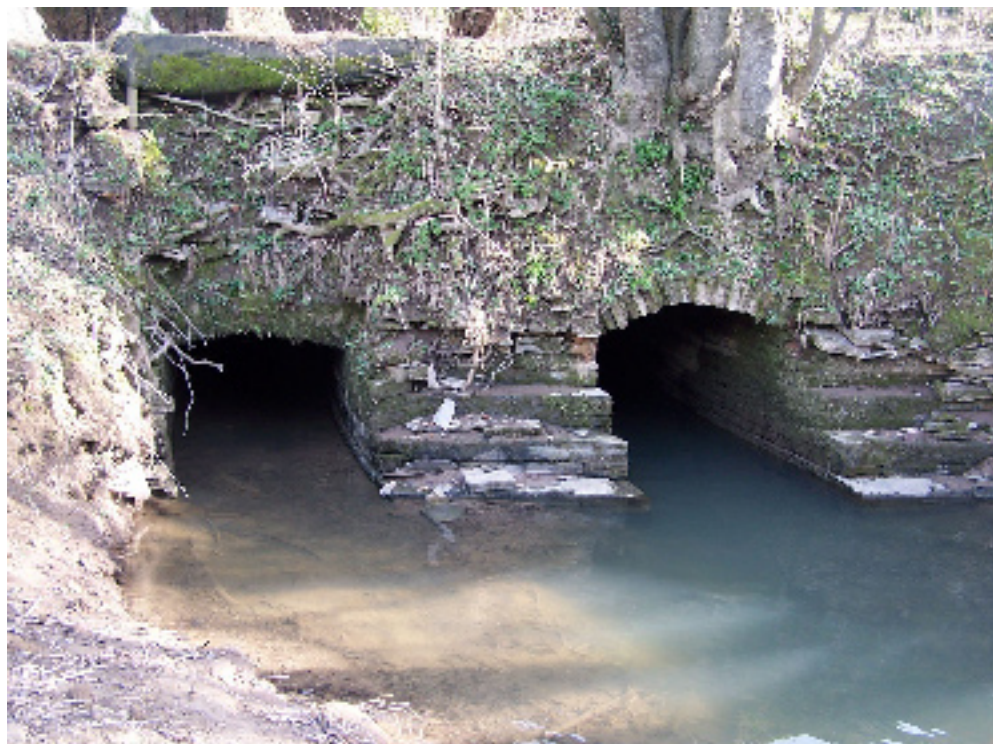
Figure 7: Outtake of the culvert (RCAHMW: 2006_109_002)
