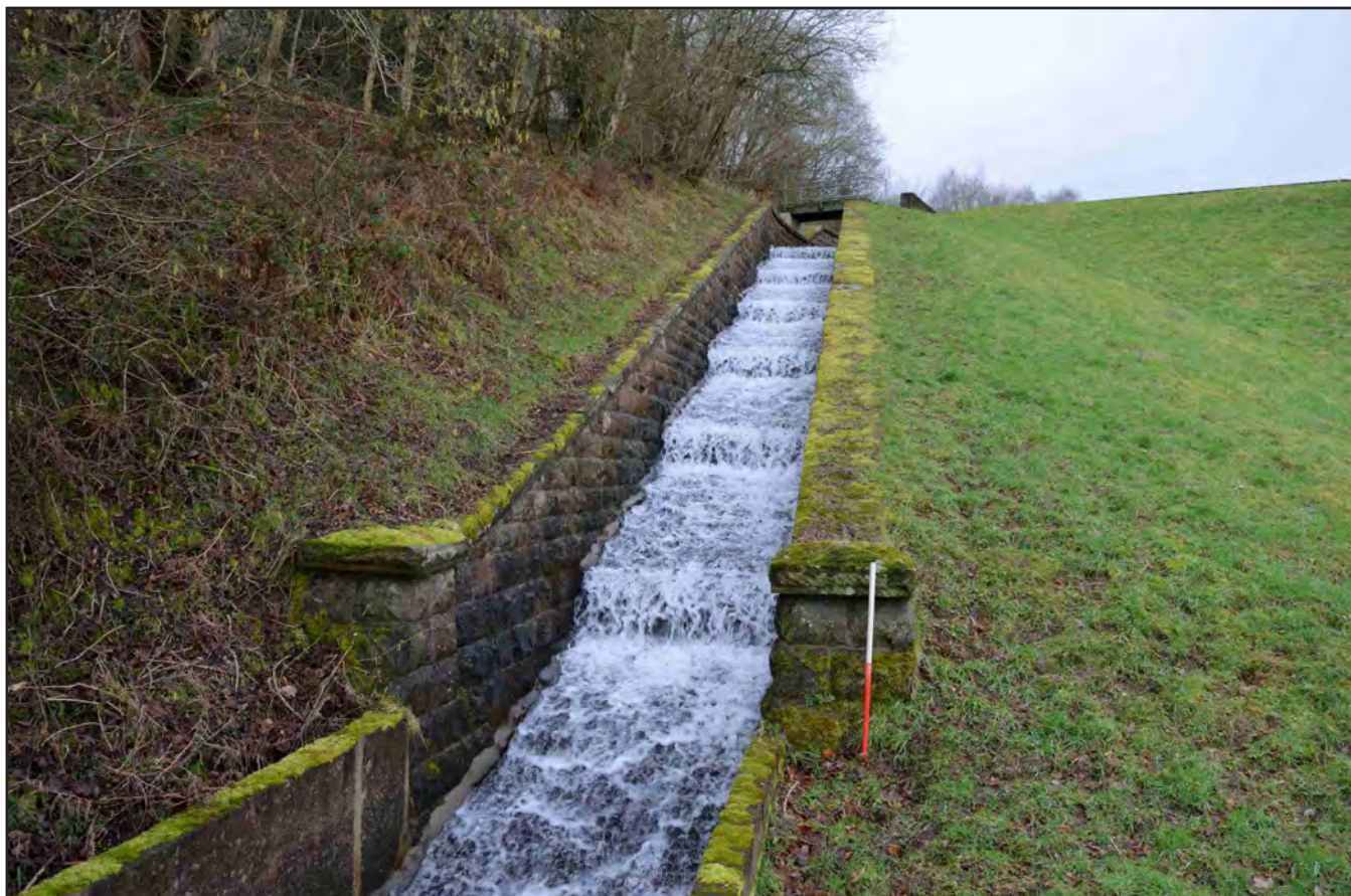
Plate 09: Concrete reinforcement at base of spillway; scale 1x1m (archive reference: G2596_018)
