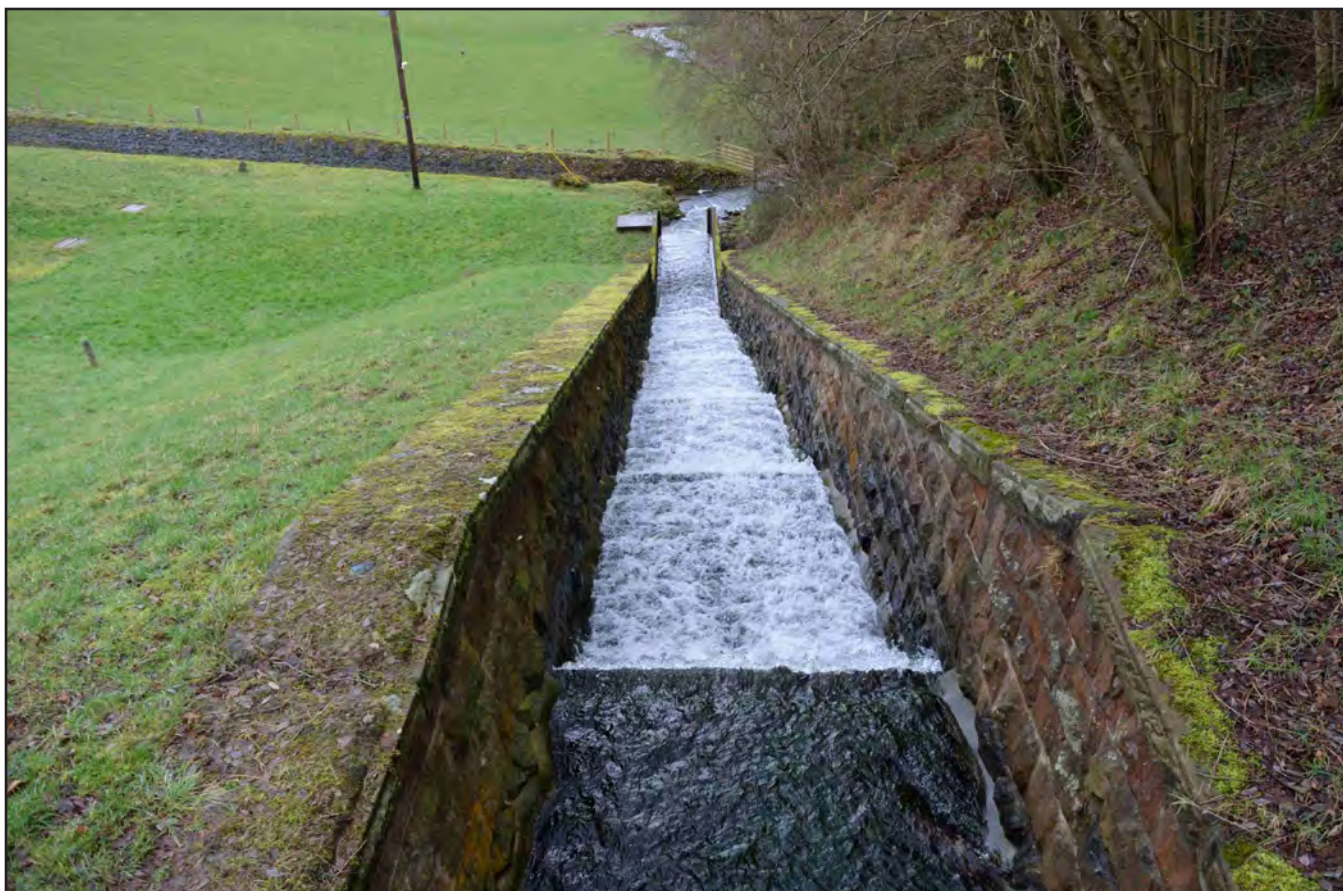
Plate 08: Original stepped spillway leading to Aber Eilun; no scale (archive reference: G2596_016)
