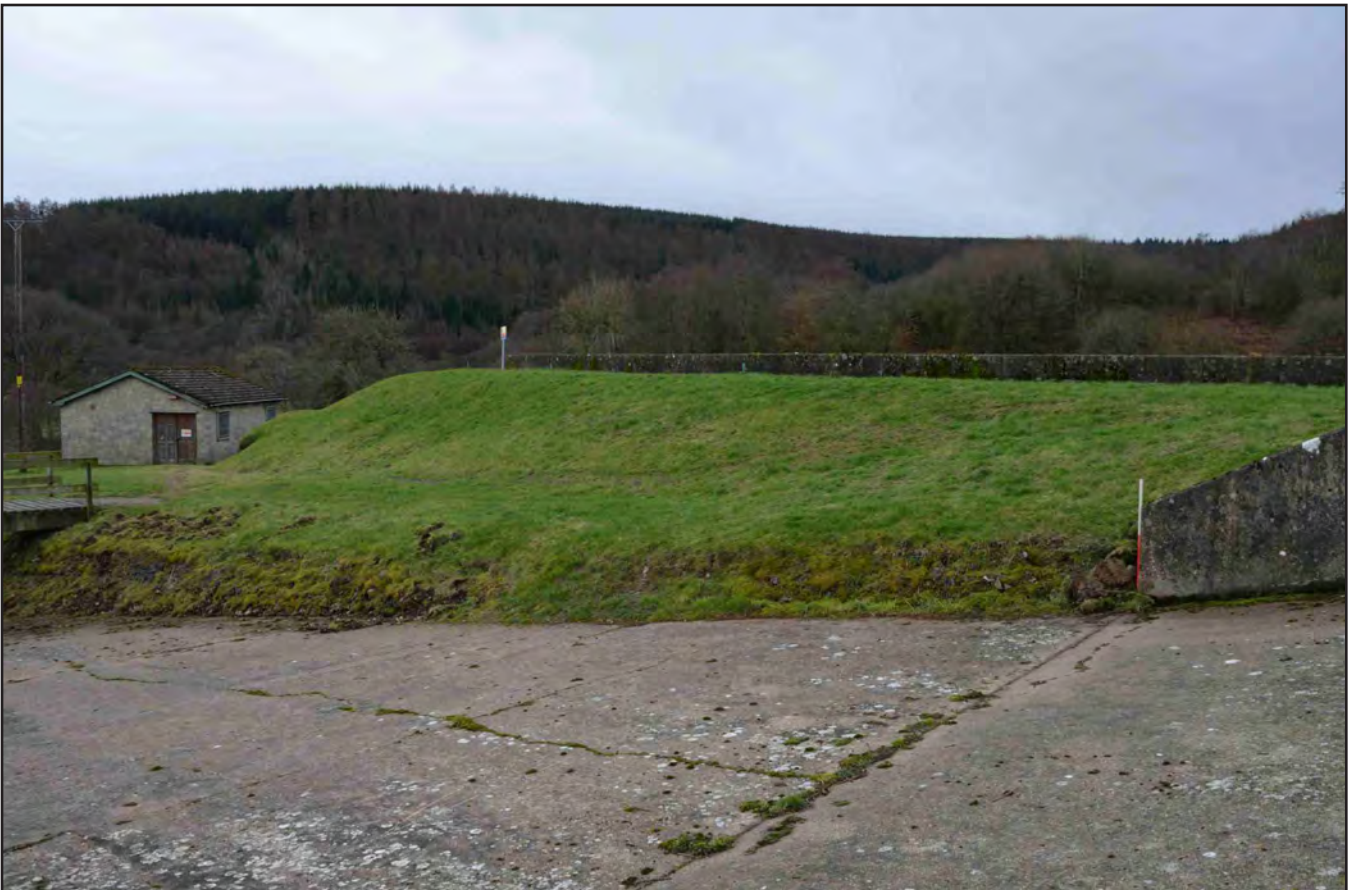
Plate 04: Earthfill embankment, North western end; scale 1x1m (archive reference: G2596_007)
