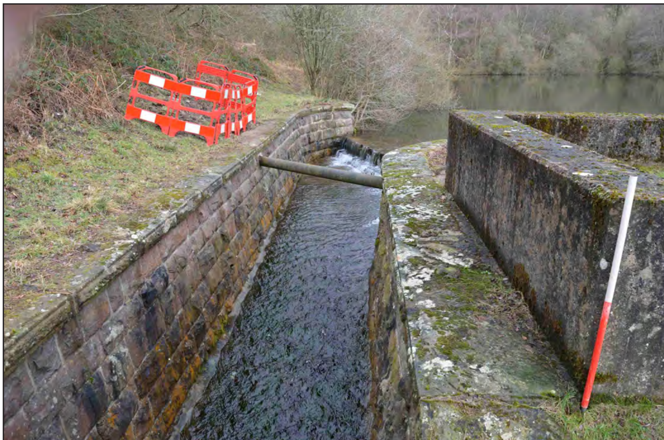
Plate 07: Original Victorian retaining walls and spillway access; scale 1x1m G2596_015)
