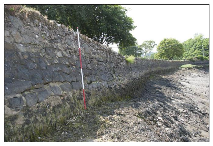
Plate 20: Collapsing section of wall, viewed from the NE (scale: 1x2m, archive image ref G2527\_017).
