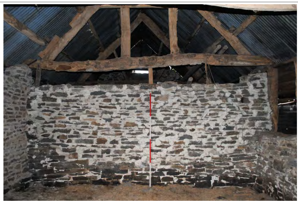
Plate 164. The northern elevation of Bay C, showing a full-height masonry wall with cill and struts supporting Truss B.
