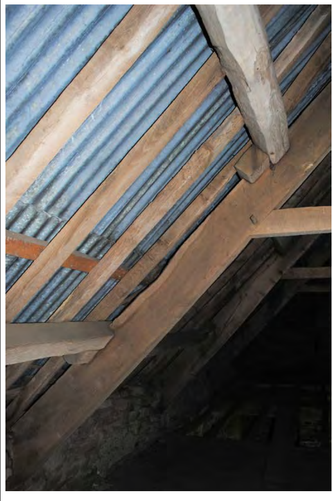
Plate 113. Northern side of Truss C. Looking east.
