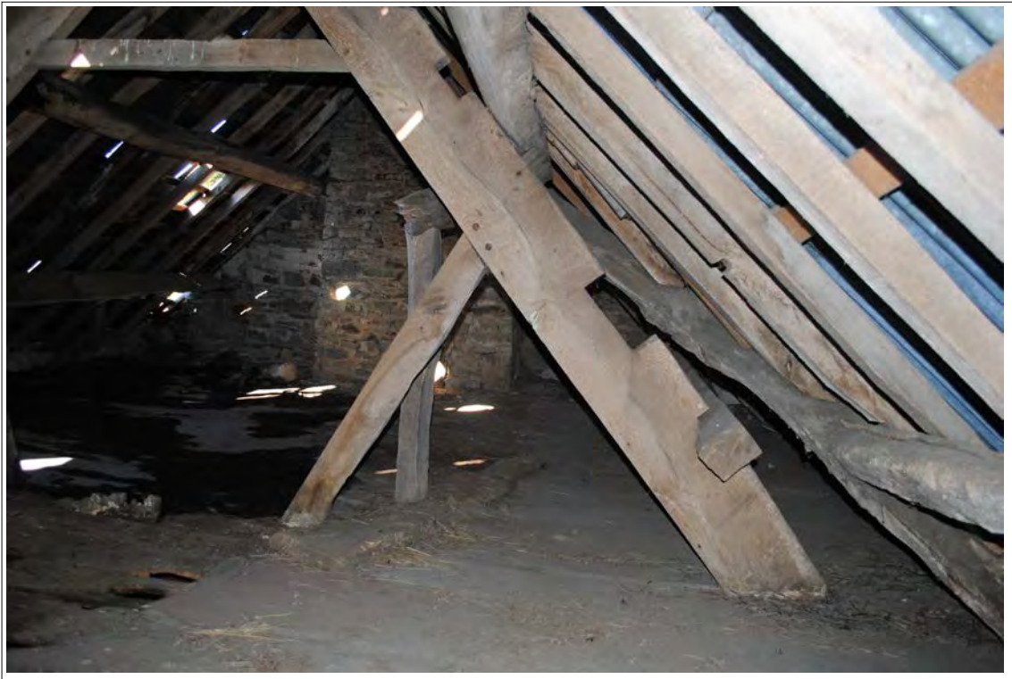
Plate 103. Northern side of Truss A. Looking west.
