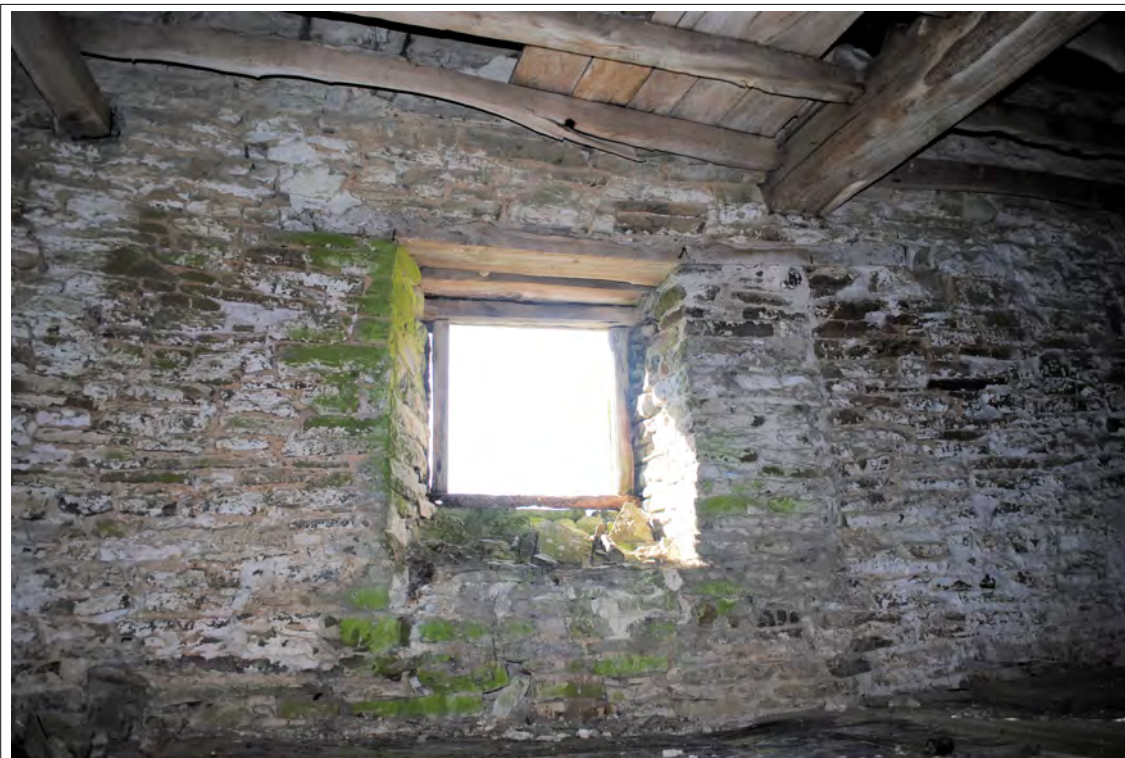
Plate 88. The eastern window on the southern wall of Room 3 (front of farmhouse) positioned to the left (east) of a straight joint in the stonework.
