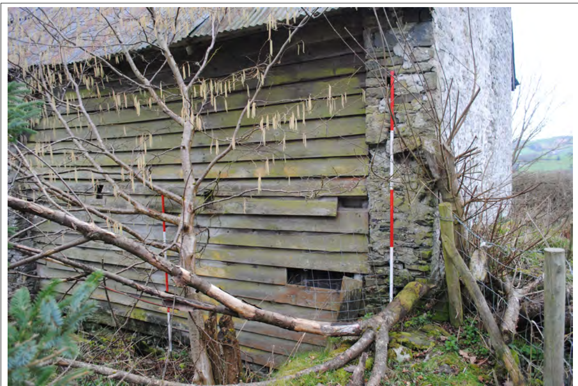
Plate 49. End-on view of the western gable wall. Looking east-southeast.
