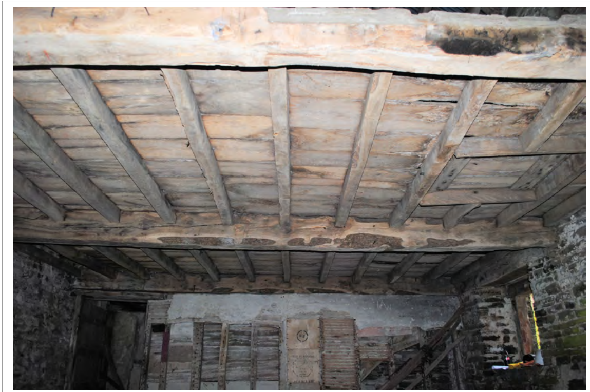
Plate 70. General view of the ceiling in Room 1. Looking west.
