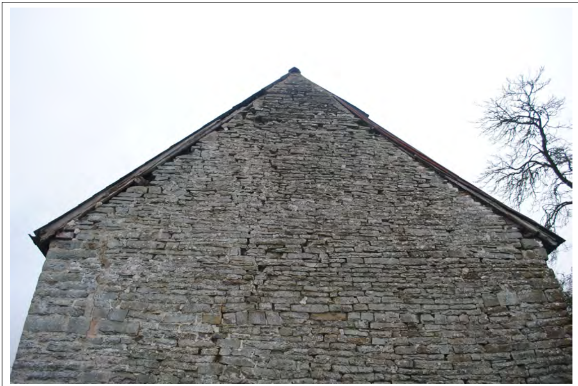
Plate 36. The upper eastern gable of the farmhouse. Looking west.
