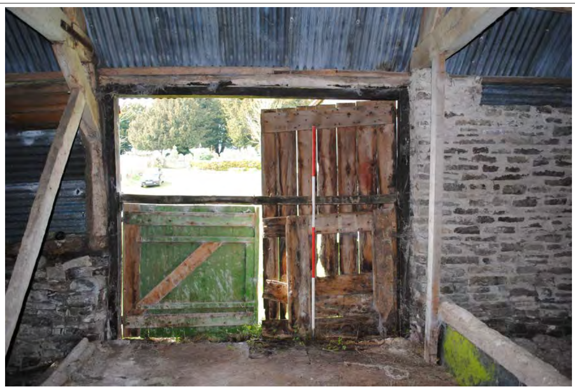
Plate 170. The western entrance to Bay D, showing low double doors and a stone threshing floor.
