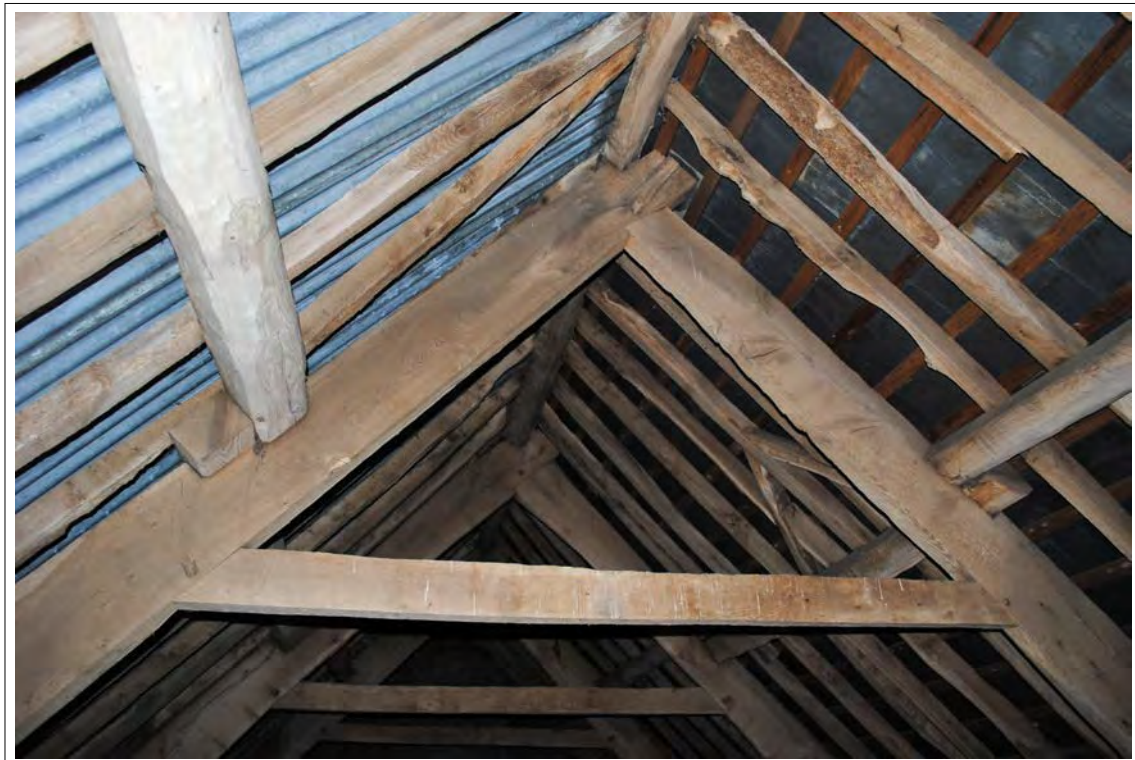
Plate 114. Upper section of Truss C. Looking east.
