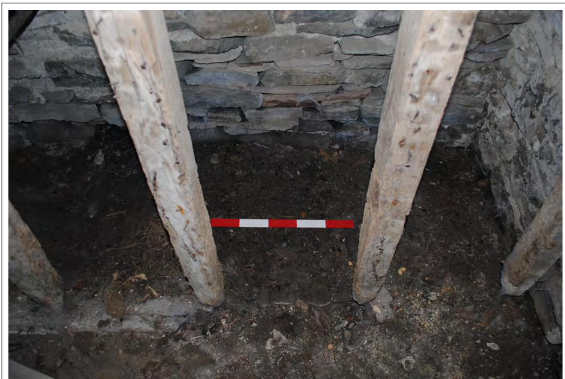
Plate 65. Floor of stone cobbles under the staircase, viewed from Room 1.
