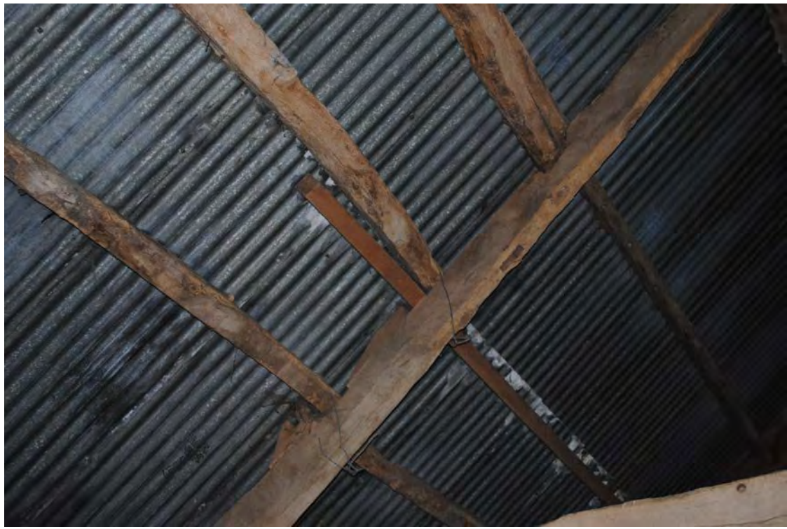
Plate 203. Eastern side of Truss D. Looking south.
