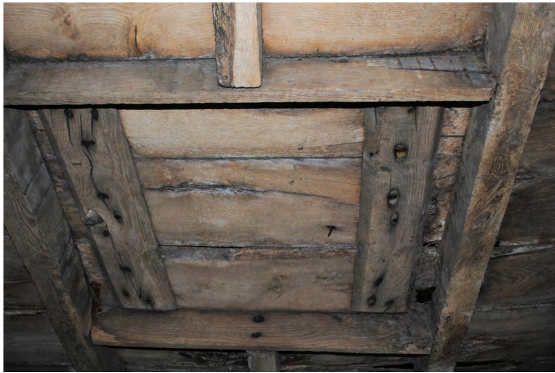
Plate 71. Detail of a hatch in the ceiling located near the northern wall of Room 1.
