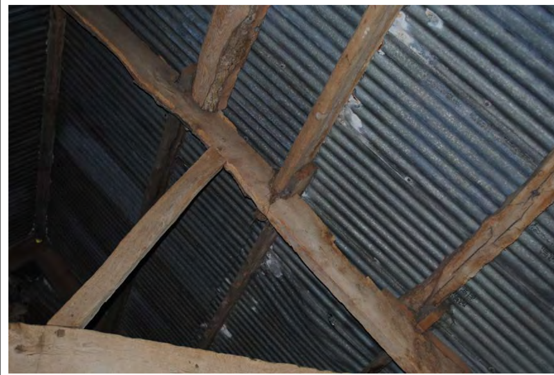
Plate 204. Western side of Truss D. Looking southwest.
