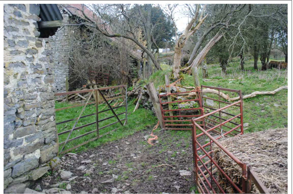
Plate 22. View of stone walling adjacent to the farmhouse. Looking west.
