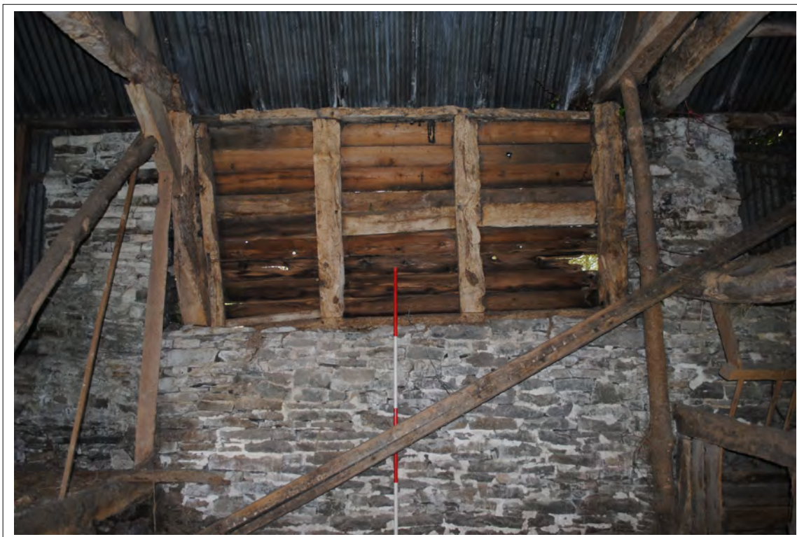
Plate 176. Detail of the timber-framing along the eastern elevation of Bay E.
