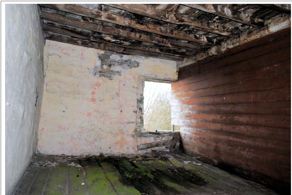
Plate 94. In Room 4a, the timber partition divides the central window on the southern wall (front of the farmhouse). Looking south-southwest.
