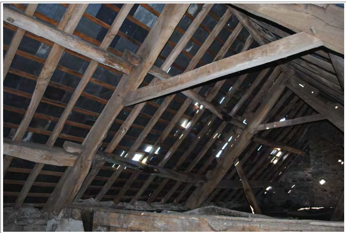
Plate 106. Southern side of Truss B. Looking southwest.
