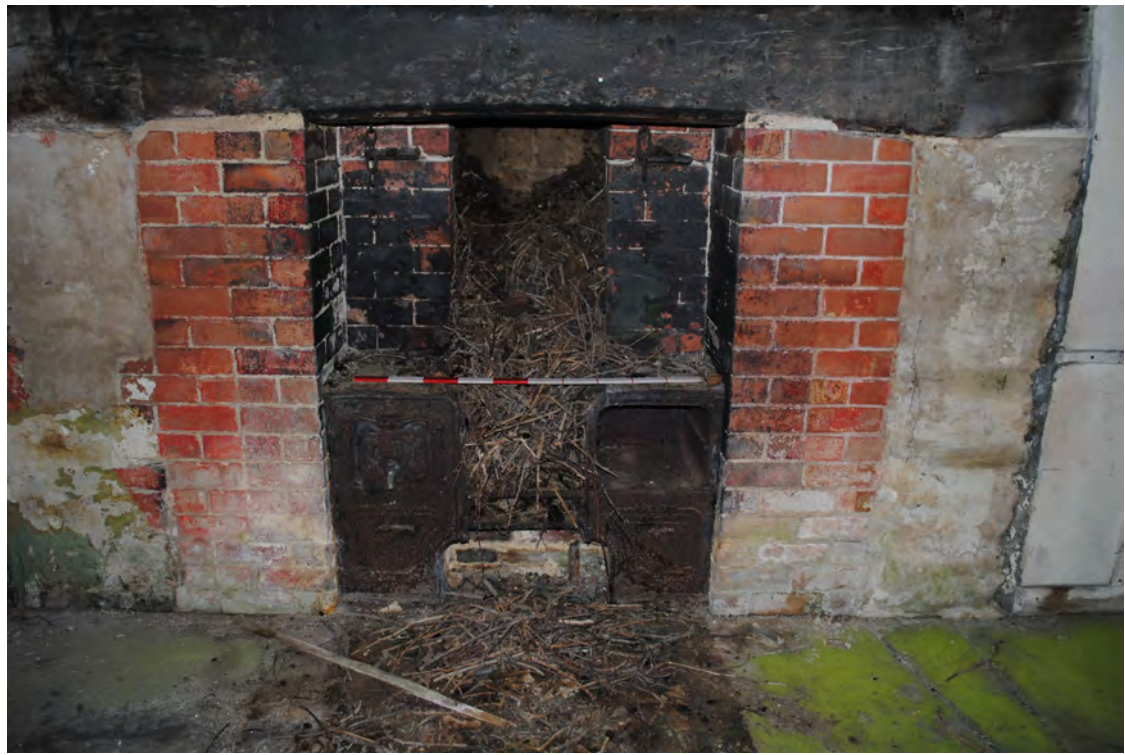
Plate 73. Detail of later range inserted into original fireplace on the western wall.
