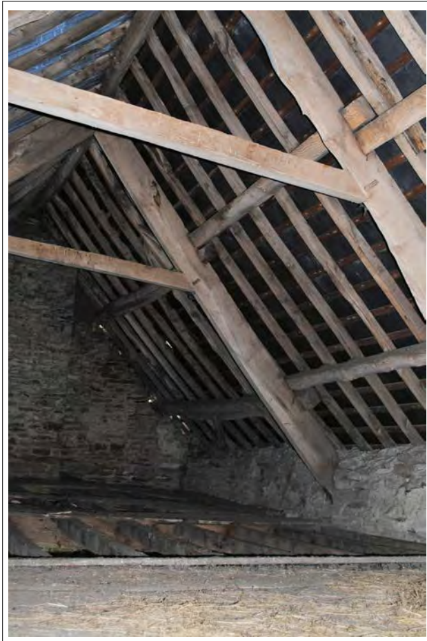
Plate 122. Southern side of Truss E (background). Looking east-southeast.
