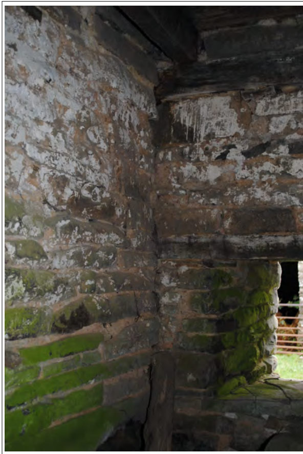
Plate 55. View of chimney built against the eastern wall of Room 1.
