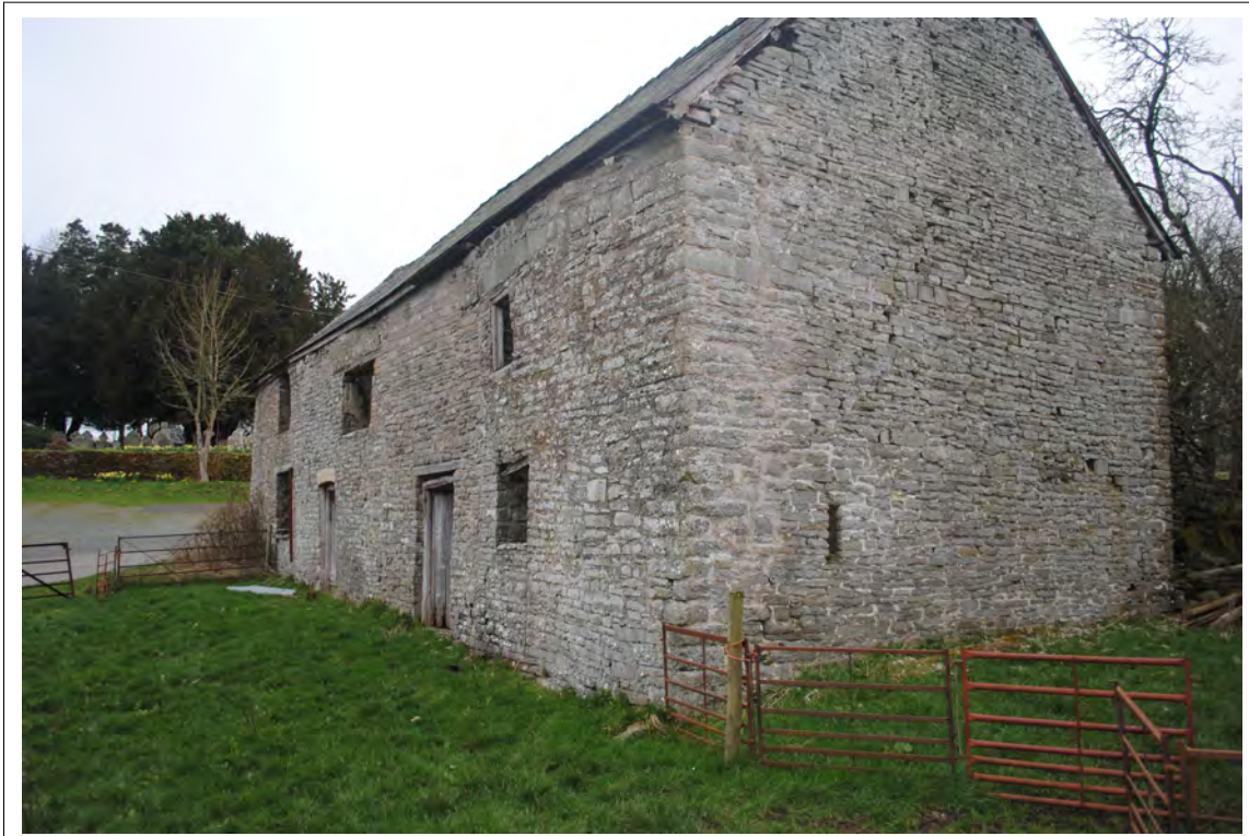
Plate 33. Oblique view of the eastern and southern elevations of the farmhouse. Looking northwest.
