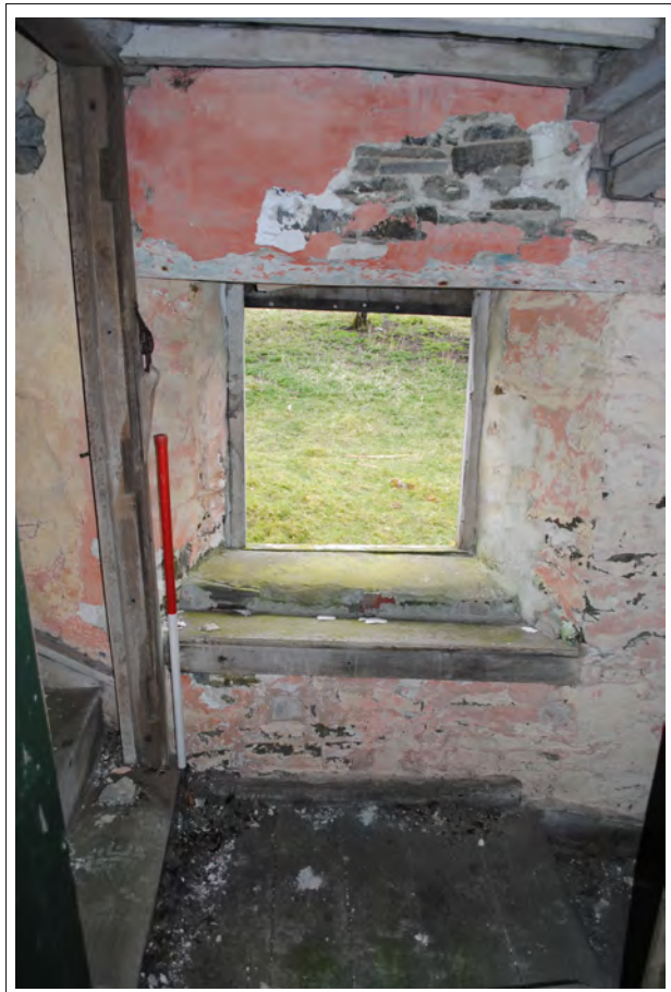
Plate 84. Window on the northern wall of the first floor landing.
