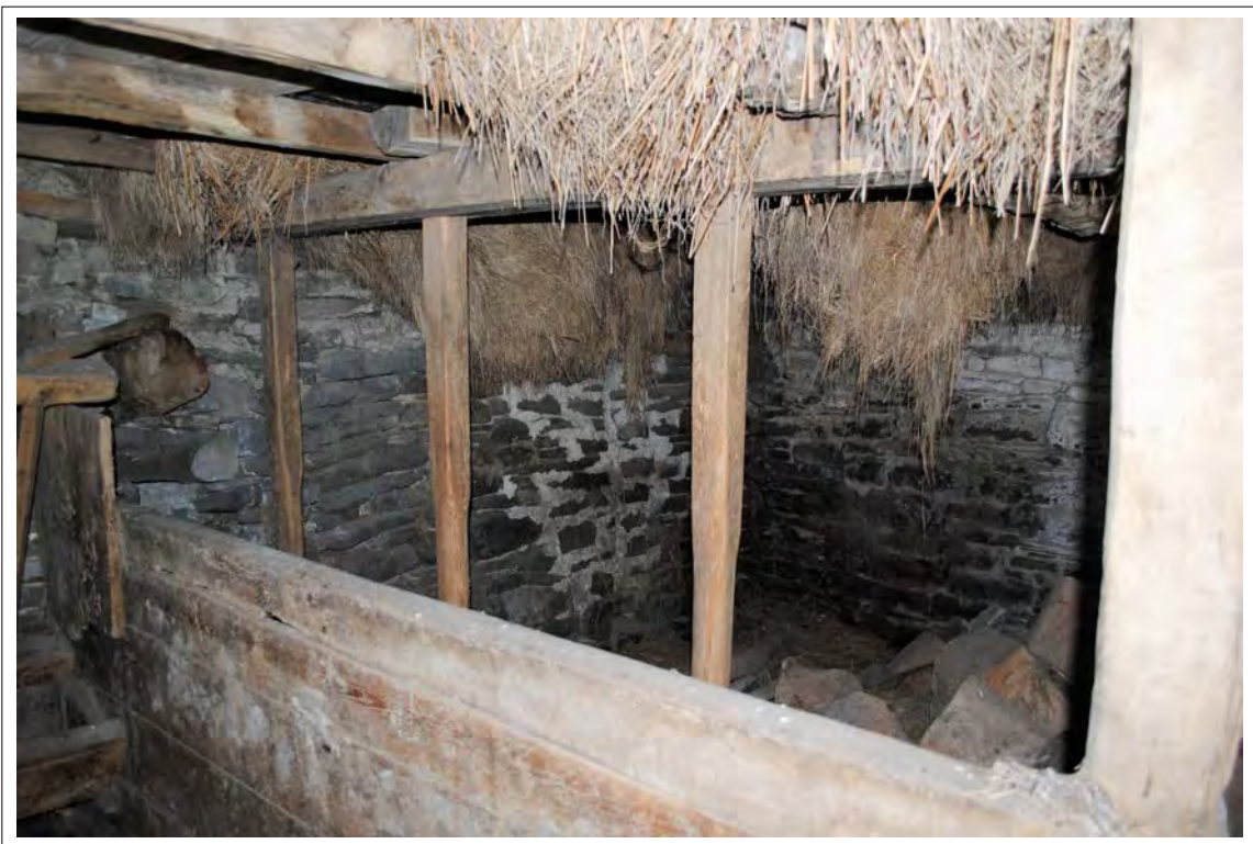
Plate 179. Oblique view of posts within Bay F for a probable cowhouse. Note the straight joint in the eastern masonry wall (Bay G). Looking south-southeast.
