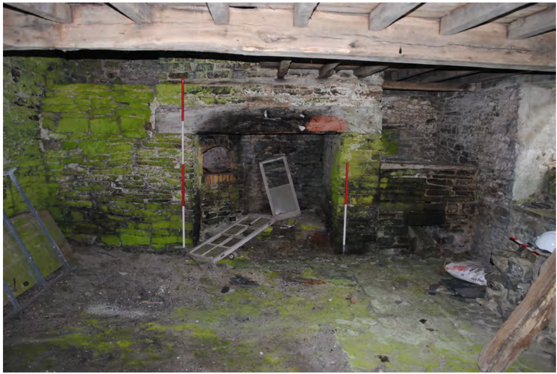
Plate 51. Fireplace on the eastern wall in Room 1 of the farmhouse.
