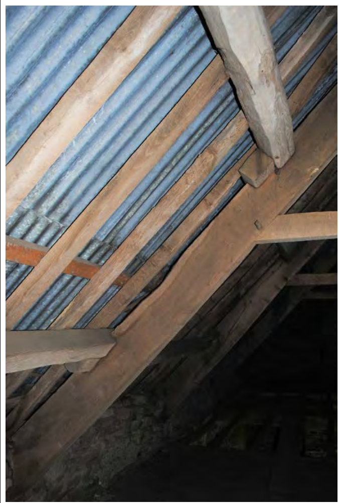
Plate 113. Northern side of Truss C. Looking east.
