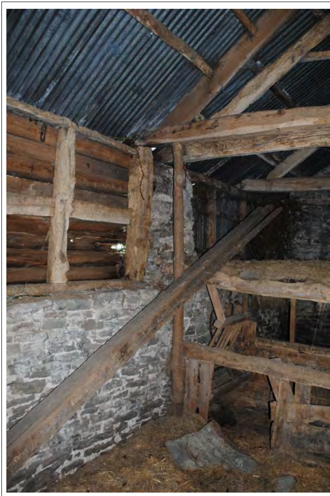
Plate 206. Eastern end of tie-beams for Trusses E1 & E2. Looking south-southeast.
