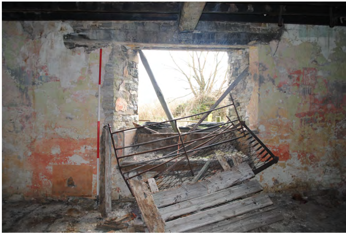
Plate 77. Window on the southern wall of Room 2.
