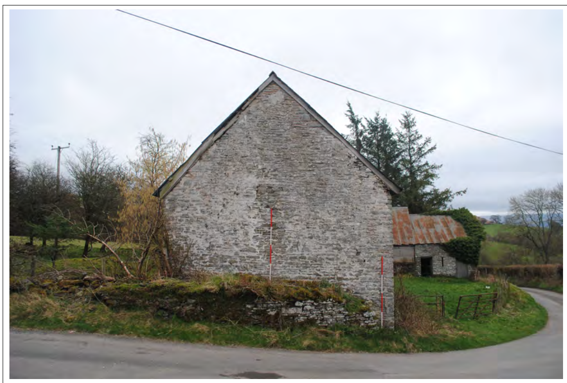
Plate 50. Overall view of the western gable. Looking east.
