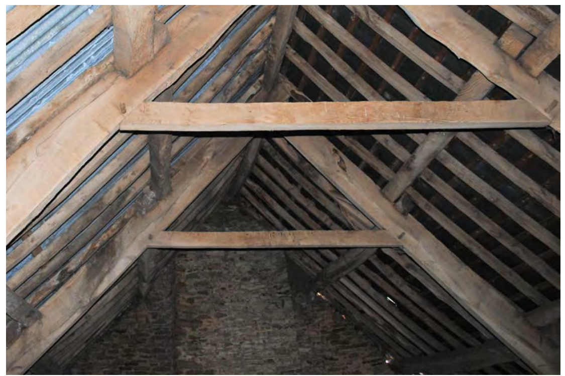
Plate 120. Upper section of Truss E (background). Looking east.
