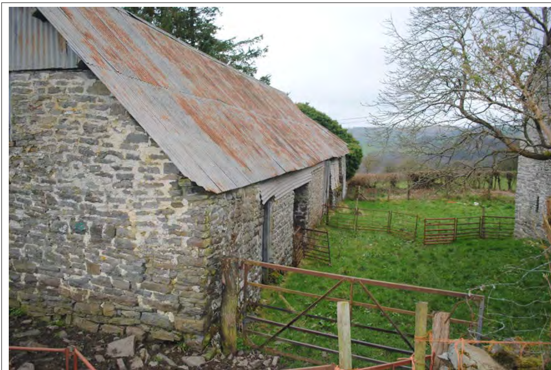
Plate 144. View of the northwest corner of the barn range. Looking south.
