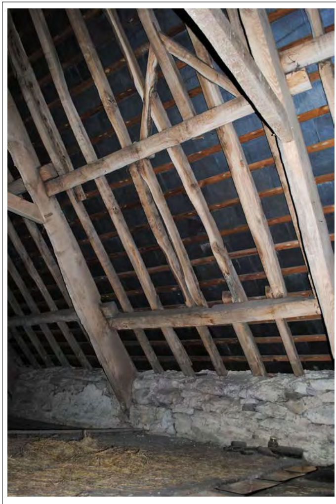
Plate 118. Southern side of Truss D (and Bay D). Looking southeast.
