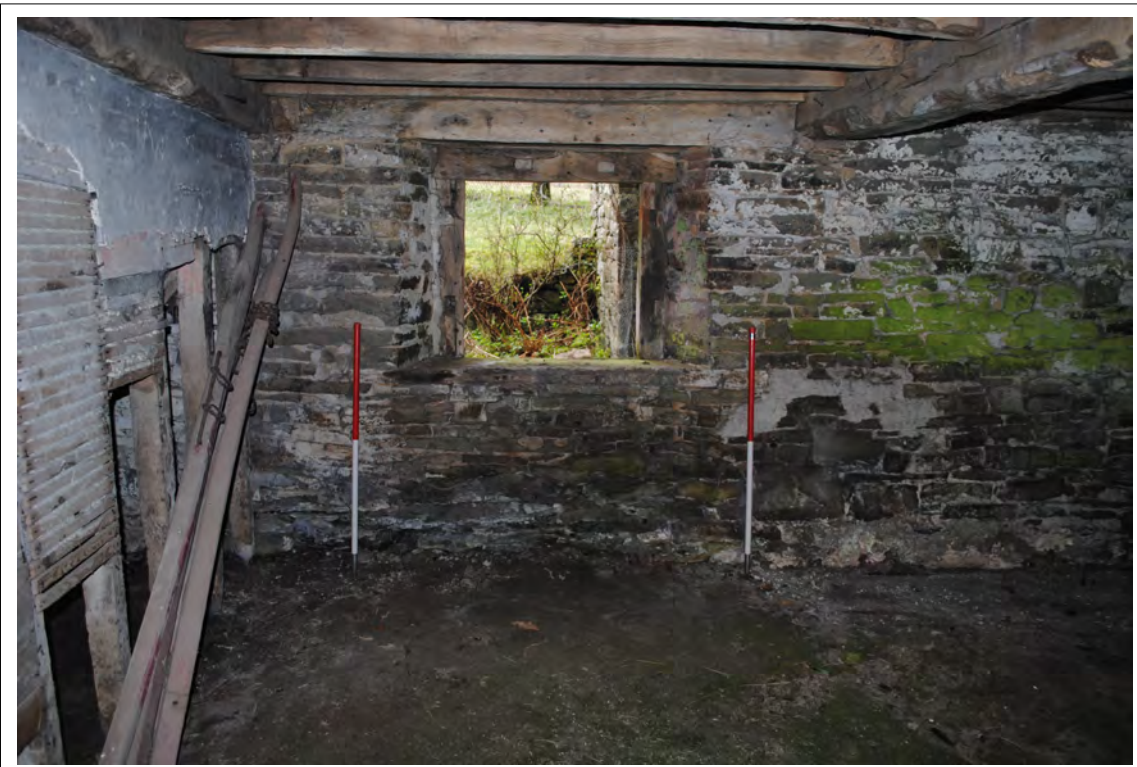
Plate 62. Window on the northern wall of Room 1.
