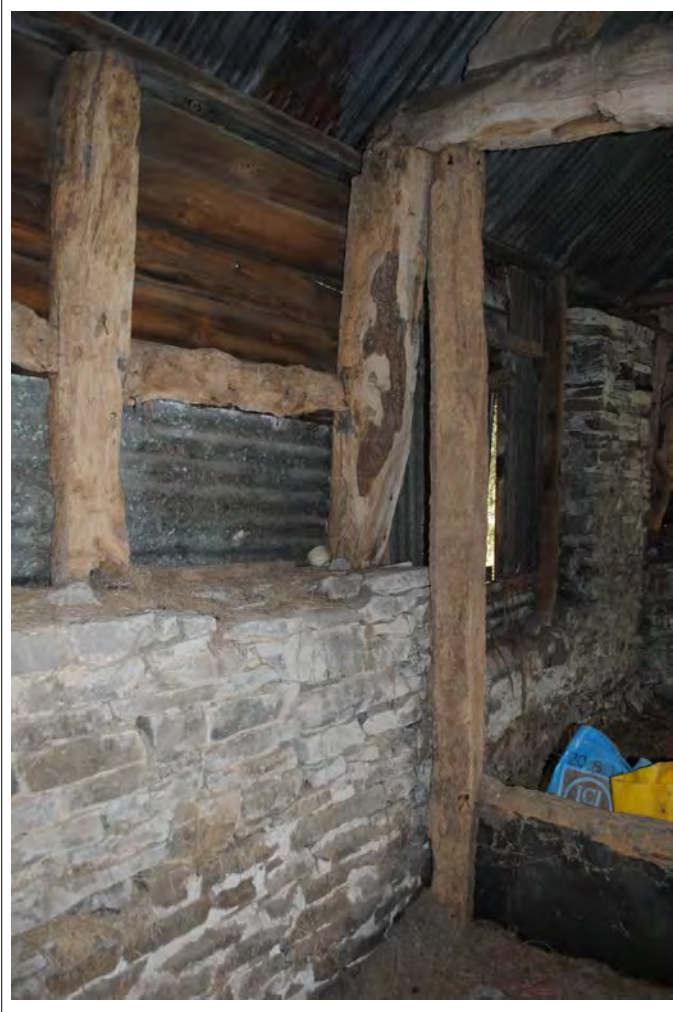
Plate 197. The eastern end of Truss C tie-beam. Looking south-southeast.
