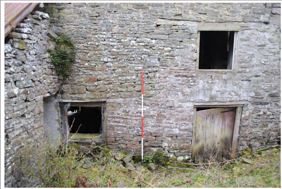
Plate 46. The back door with window above (right) and single lower window (left) forming part of the western and eastern internal divisions of the farmhouse, respectively. Looking south.
