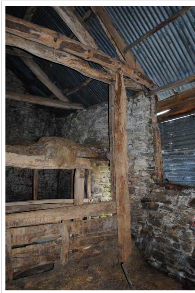
Plate 209. Western end of tie-beams for Trusses E1 & E2. Looking southwest.
