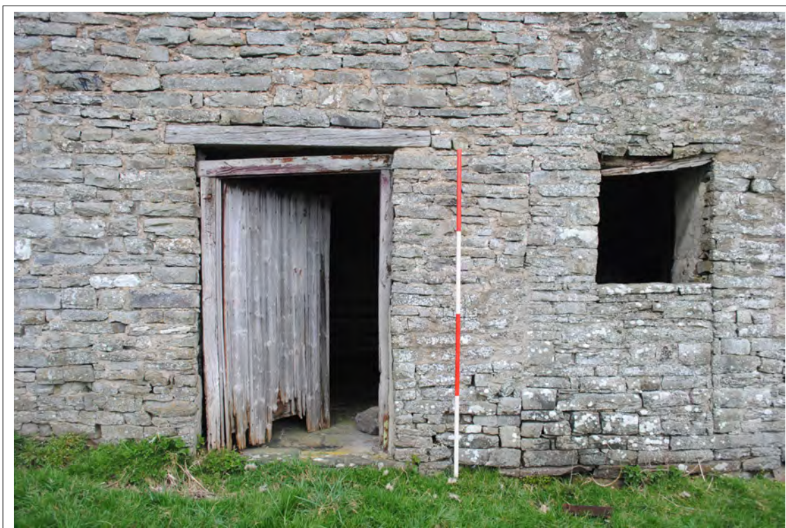
Plate 32. The front entrance to the eastern part of the farmhouse, with blocked doorway to the right (southern elevation). Looking north.
