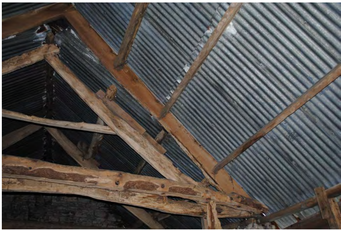
Plate 208. Western side of Trusses E1 & E2. Looking southwest.
