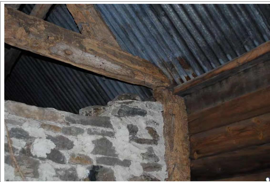
Plate 195. Eastern end of Truss B tie-beam. Looking northeast.
