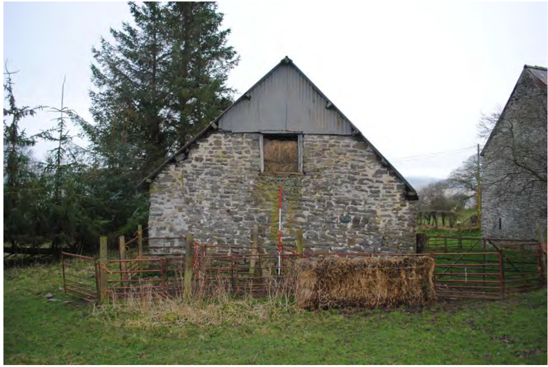
Plate 145. General view of the northern gable. Looking south-southwest.
