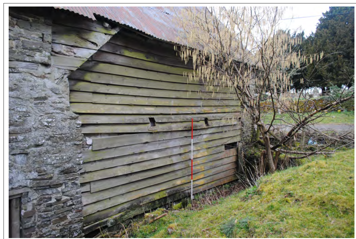
Plate 48. View of weatherboarded section of external wall, over timber frame, along the northern elevation of the farmhouse. Looking west-southwest.
