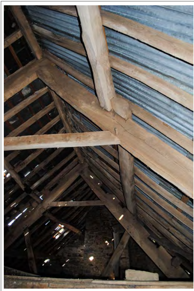
Plate 108. Northern side of Truss B. Looking west.
