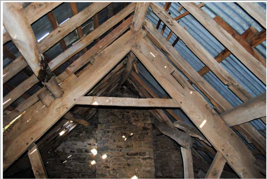
Plate 102. Upper section of Truss A. Looking west.
