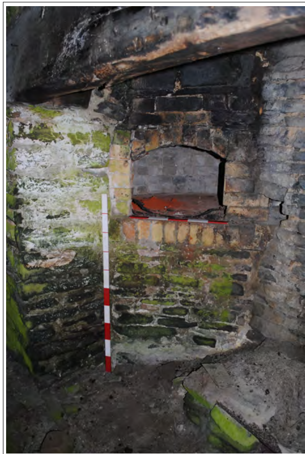
Plate 56. General view of oven inserted into the main fireplace (Room 1).
