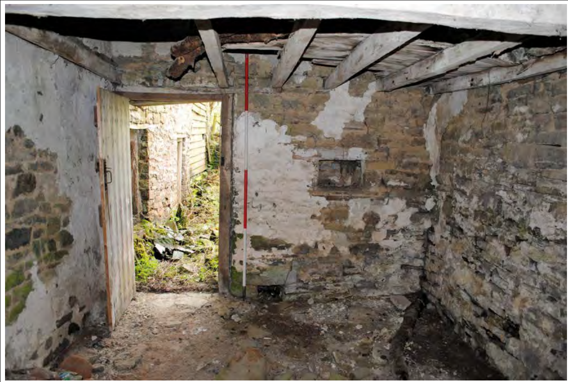
Plate 127. The western wall of the lean-to, with doorway (left) and small recess (right). The stonework has patches of lime plaster.
