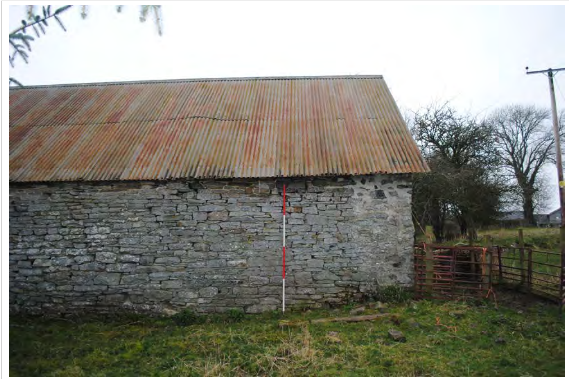
Plate 149. Detail of the eastern elevation, Bays A & B. Looking west-northwest.
