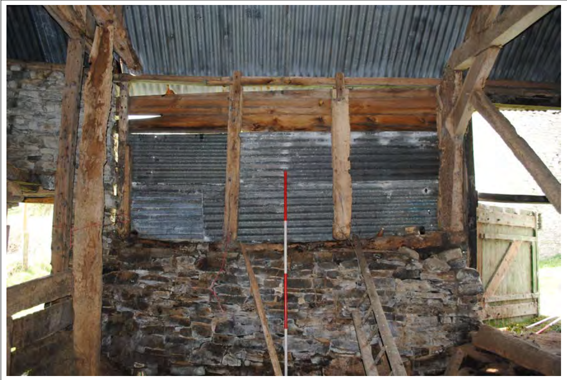
Plate 173. Detail of the timber-framing along the western elevation of Bay E.
