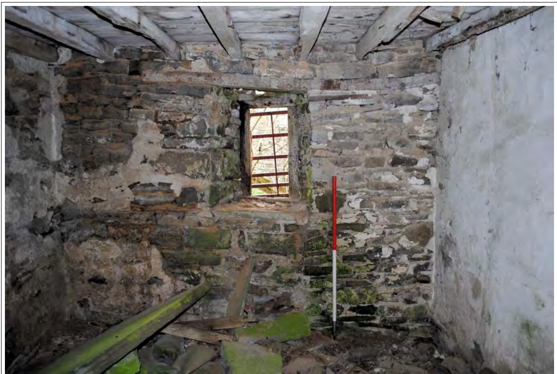
Plate 124. Small lower window in the eastern wall of the lean-to. The stone wall has patches of lime plaster.
