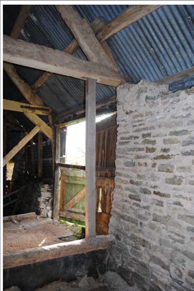
Plate 200. The western end of Truss C tie-beam. Looking southwest.
