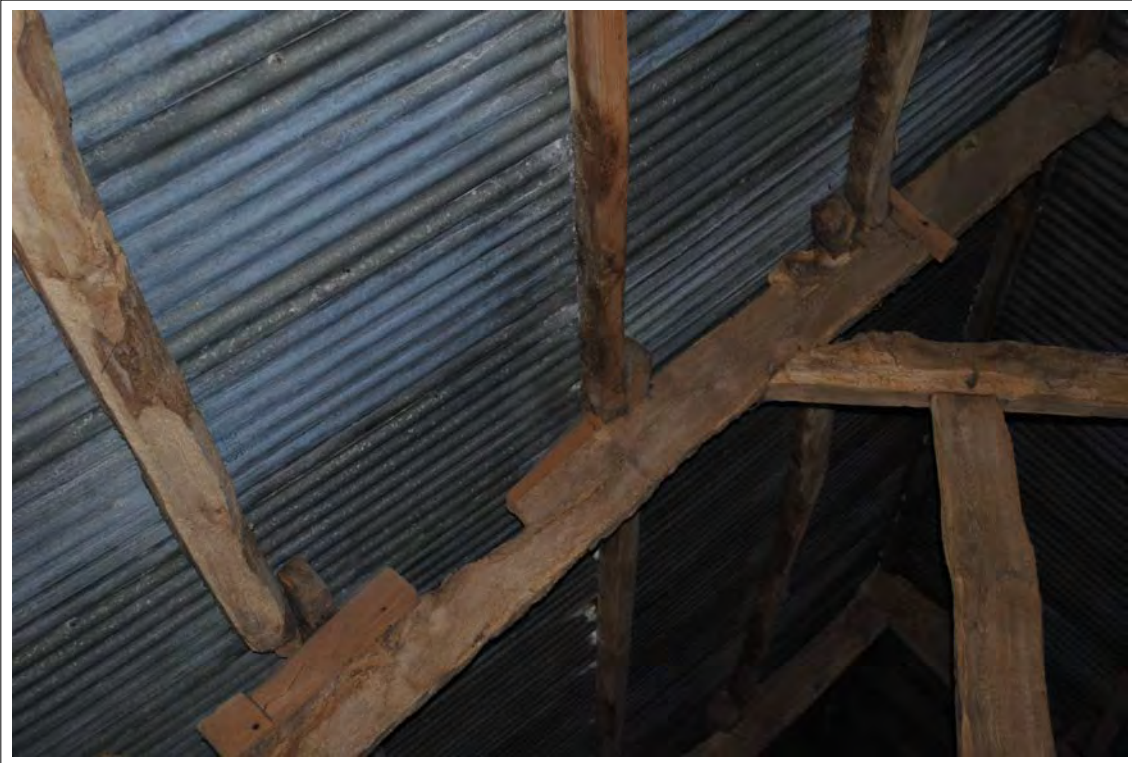
Plate 193. Western side of Truss B. Looking north-northeast.
