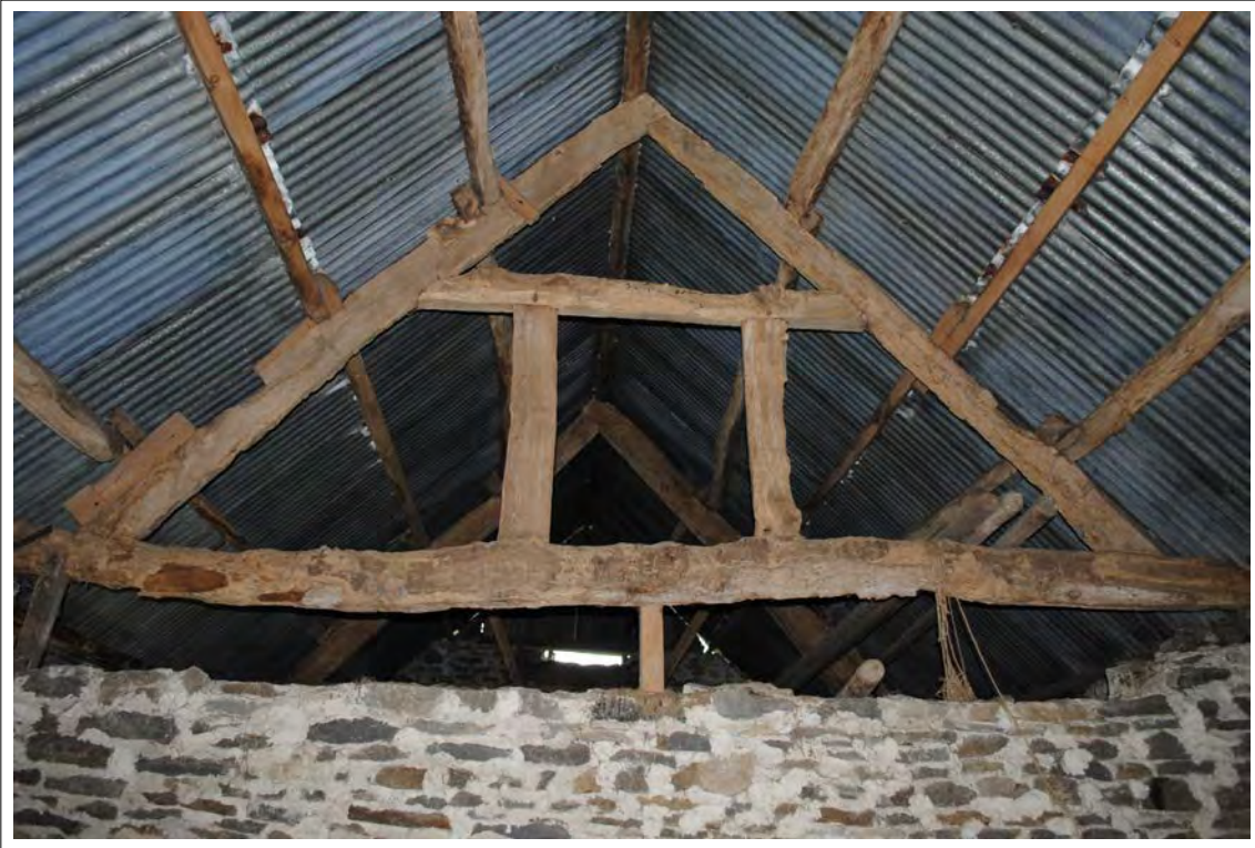
Plate 191. General view of Truss B. Looking north-northeast.
