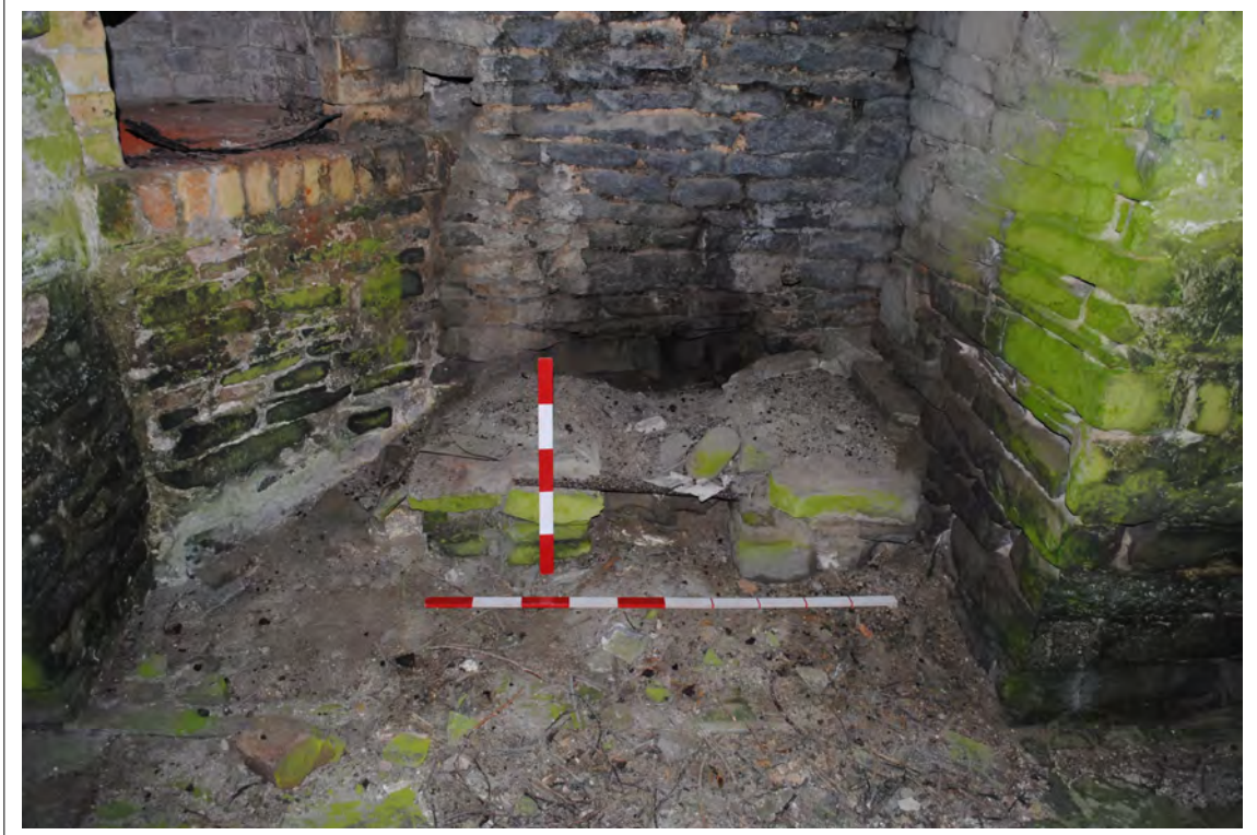
Plate 57. Later fireplace adjacent to oven in Room 1.
