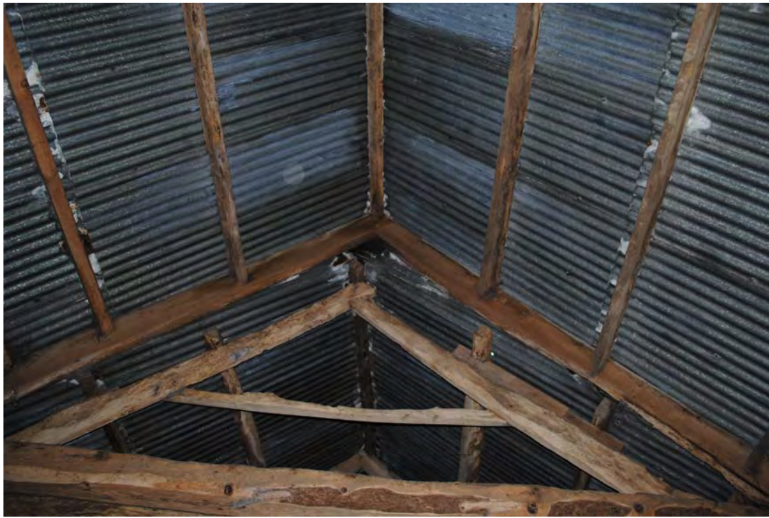
Plate 205. General view of Trusses E1 & E2. Looking south-southwest.
