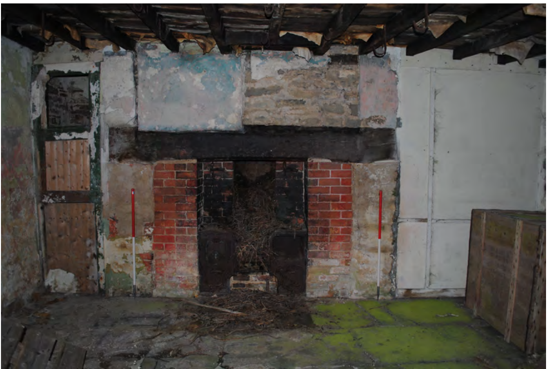
Plate 72. Fireplace on the western wall in Room 2 of the farmhouse.
