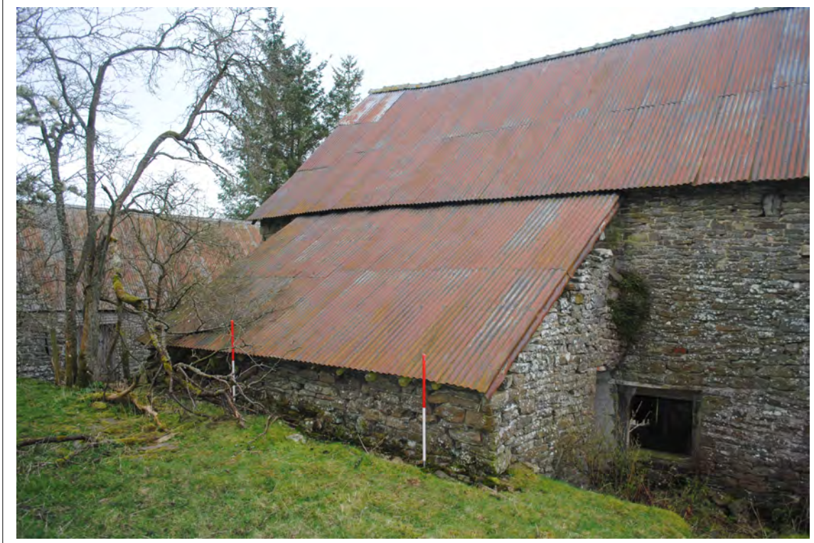
Plate 41. Oblique view of the lean-to at the back of the farmhouse, showing the corrugated steel roof on the northern side of the building. Looking southeast.
