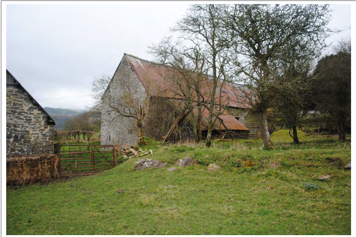
Plate 21. The rear of the farmhouse in relation to the barns. Looking south-southwest.
