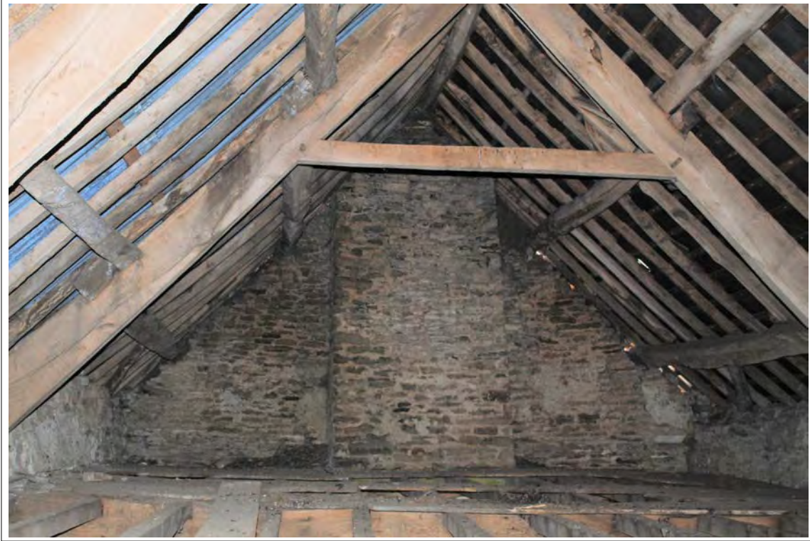
Plate 121. Internal face of the east gable wall. Looking east.
