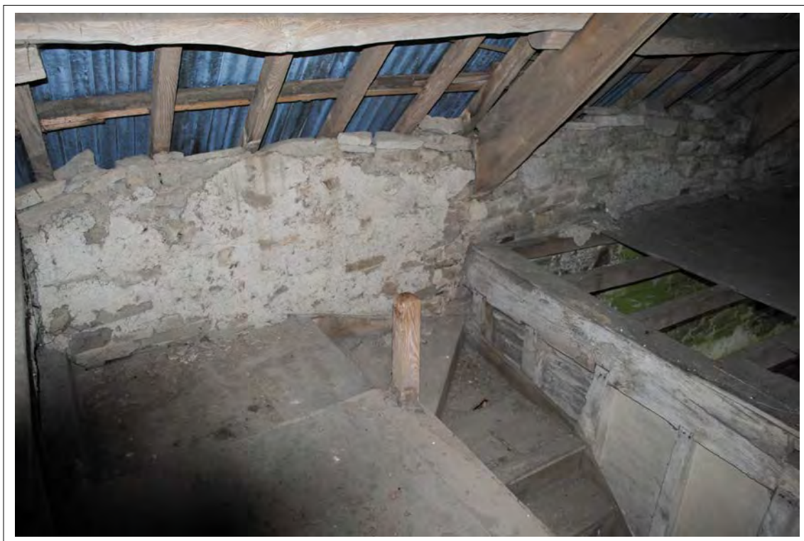
Plate 112. Northern side of Truss C. Looking northeast.
