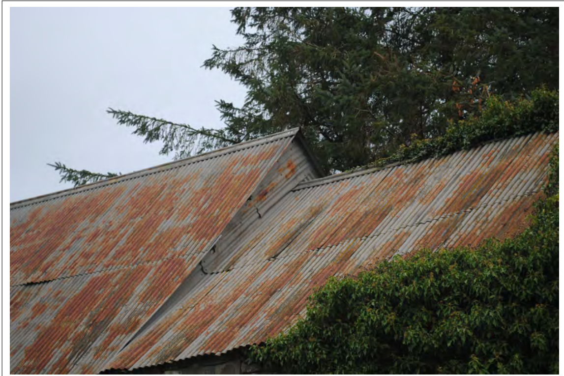
Plate 136. Detail of the corrugated steel roof, with a change in height between the main barn (left) and cowhouse or looseboxes (right). Looking east-northeast.
