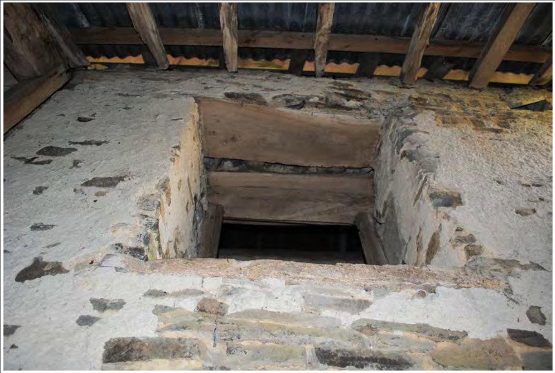
Plate 129. Window in the southern wall, originally an external back window of the farmhouse. Looking south.
