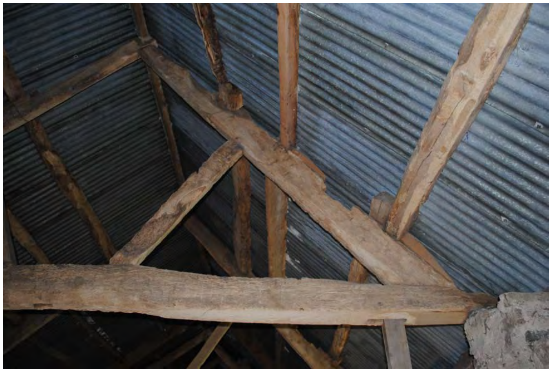
Plate 199. Western side of Truss C. Looking south-southwest.
