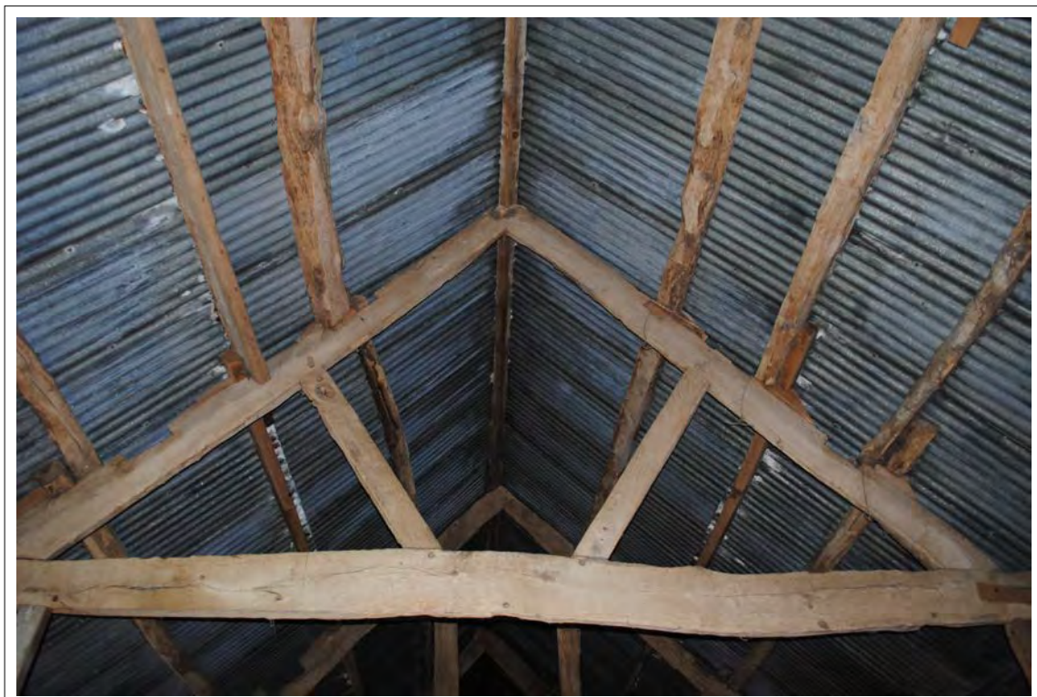
Plate 196. General view of Truss C. Looking south-southwest.
