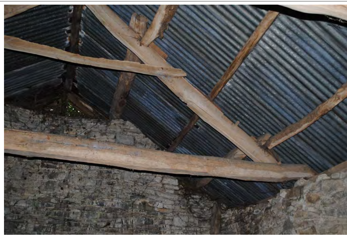
Plate 212. Western side of Truss F. Looking southwest.
