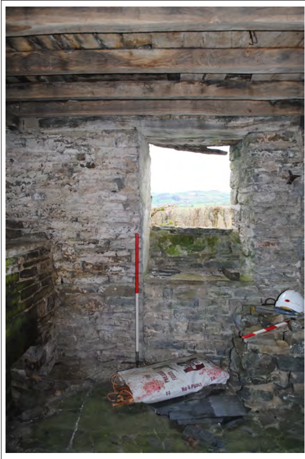
Plate 69. Part blocked doorway, now window, on the southern wall of Room 1.
