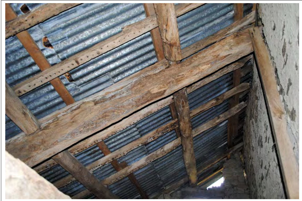
Plate 132. General view of the roof timbers of the lean-to. Looking east.
