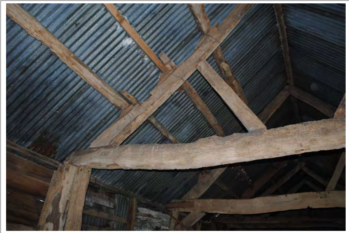
Plate 198. Eastern side of Truss C. Looking south.
