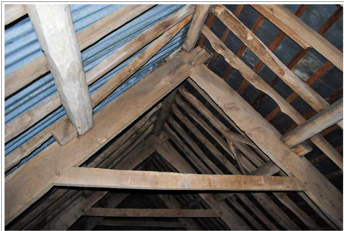
Plate 114. Upper section of Truss C. Looking east.
