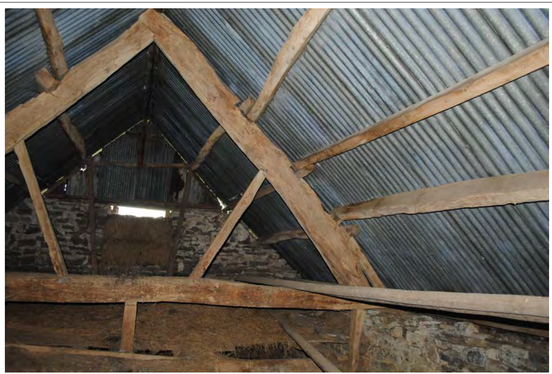
Plate 190. Eastern side of Truss A. Looking northeast.
