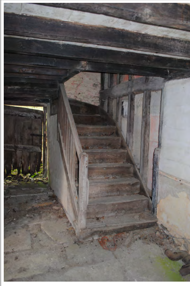
Plate 79. General view of the farmhouse hallway, showing the staircase built against an internal timber wall. Looking north-northeast.
