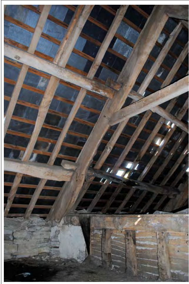
Plate 105. Southern side of Truss B. Looking southwest.
