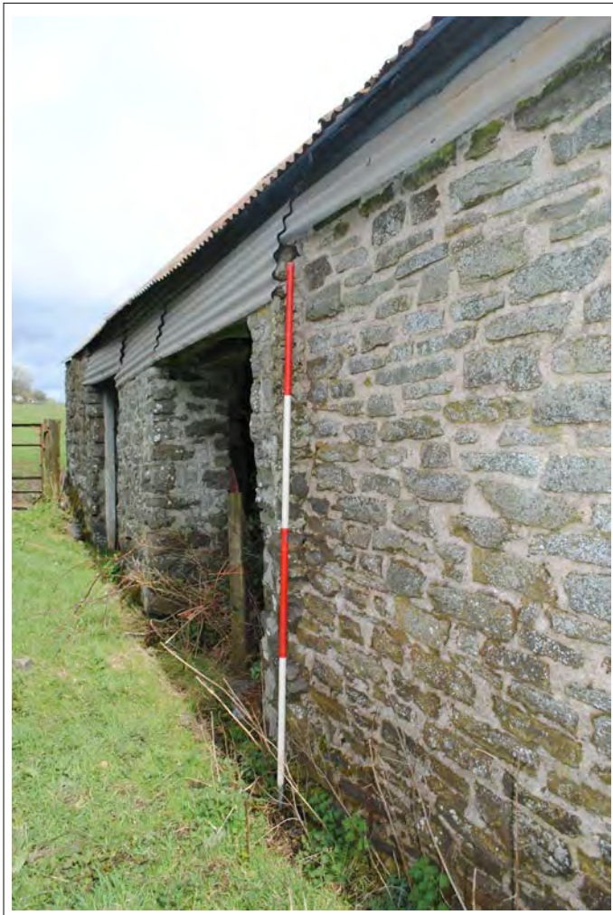
Plate 142. Detail of the separate phases of stonework between the barn (Bay C) and the cartlodge (Bay B) on the western elevation. Looking north-northeast.
