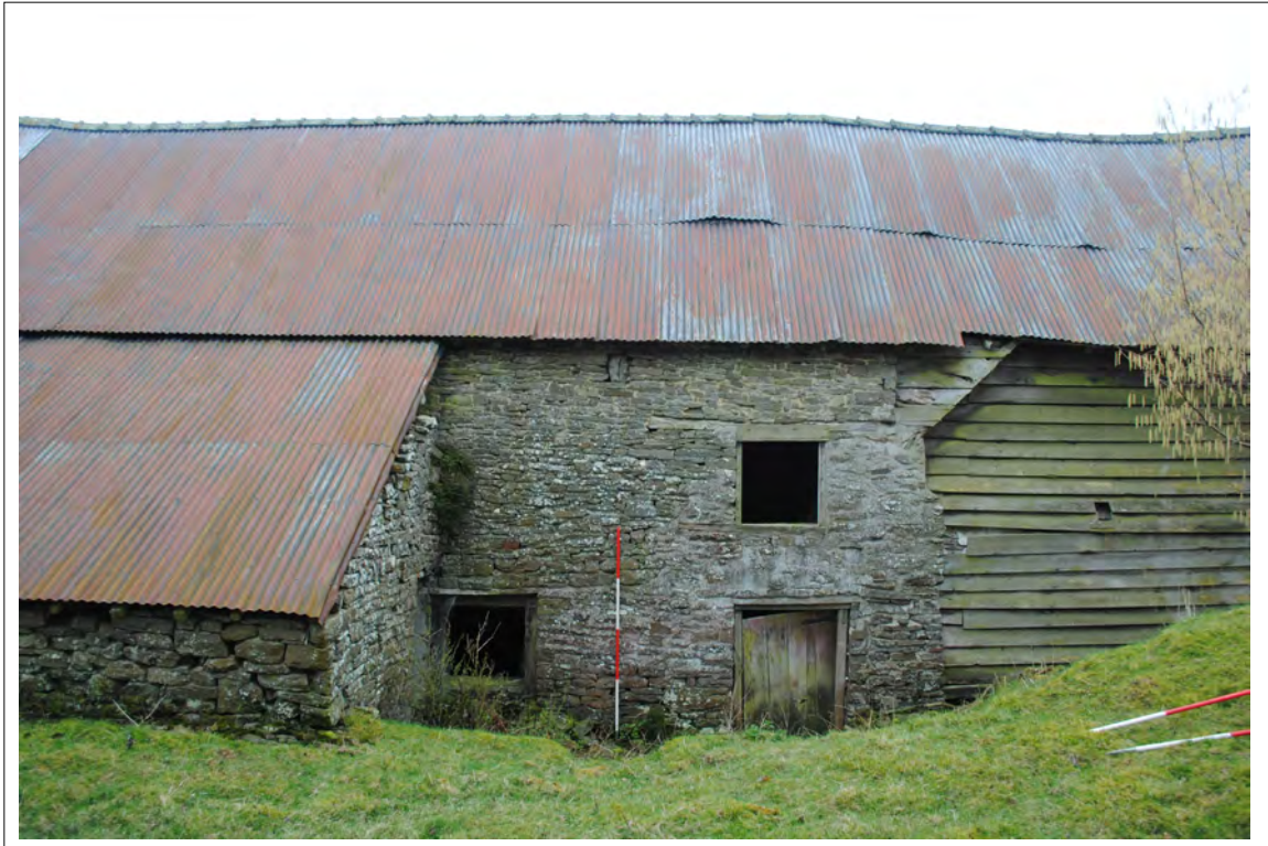
Plate 45. General view of the northern elevation. Looking south.
