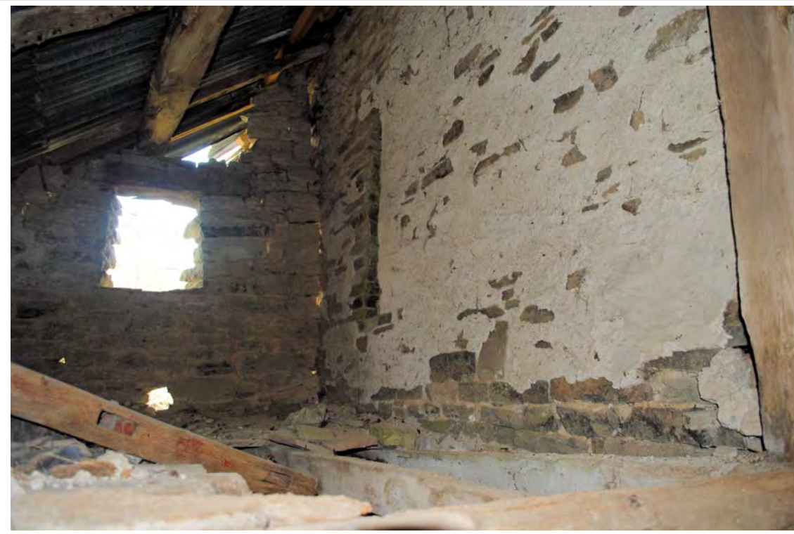
Plate 128. Oblique view of the ventilation in the southern wall, with patches of lime plaster evident. The eastern wall has a small window below collapsed stonework. Looking east-southeast.
