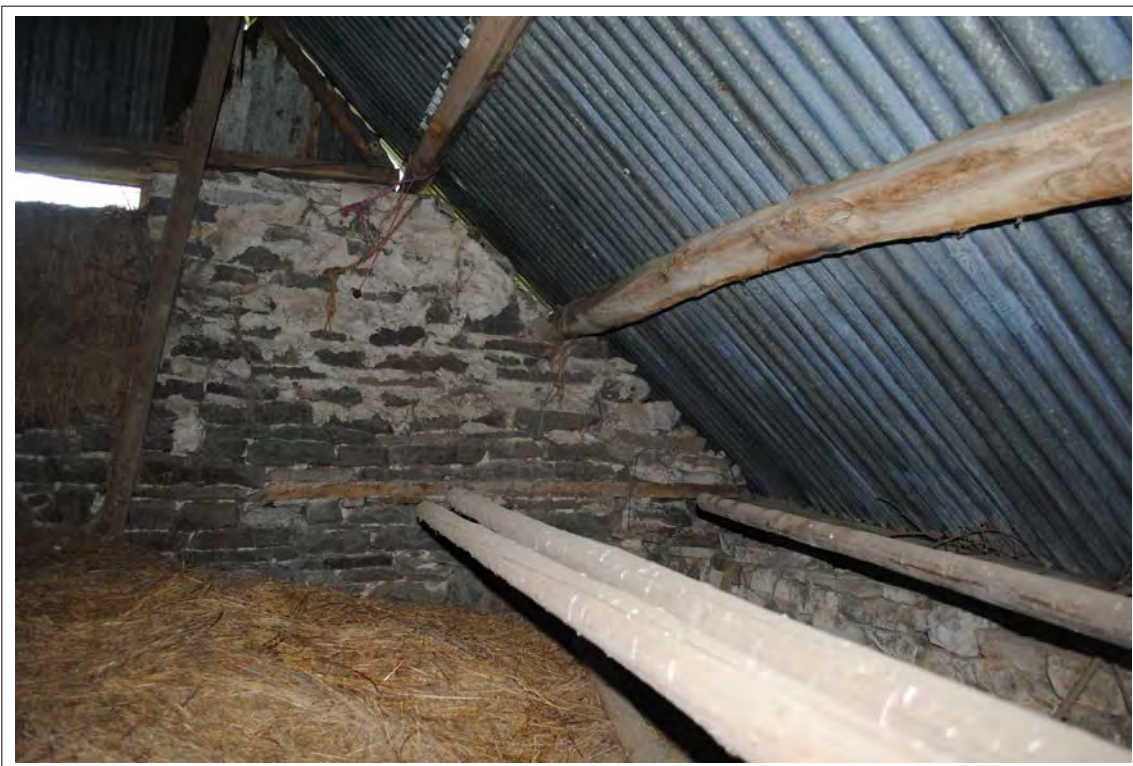
Plate 187. Eastern side of the upper north gable. Looking northeast.
