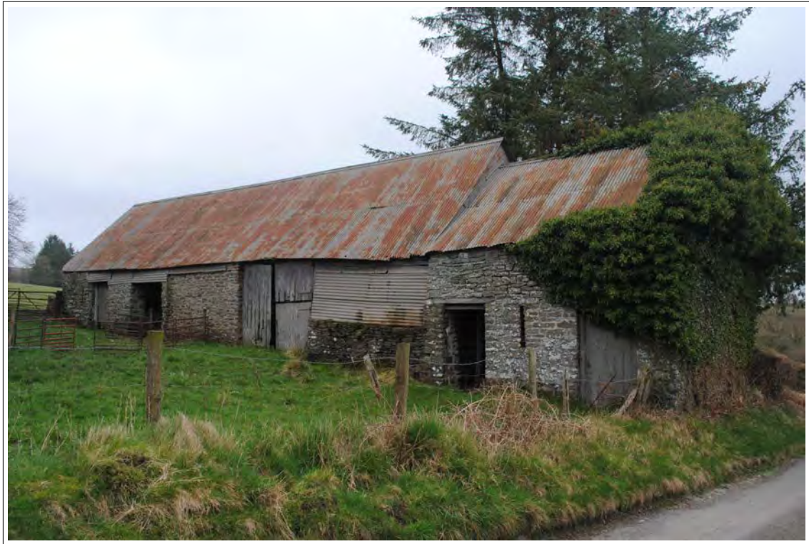
Plate 133. General view of the barns at Church House Farm. Looking east-northeast.
