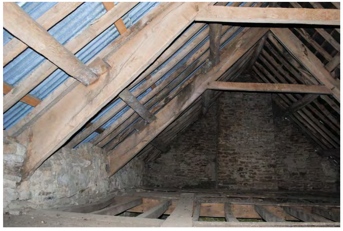
Plate 119. Northern side of Truss E (background). Looking east.
