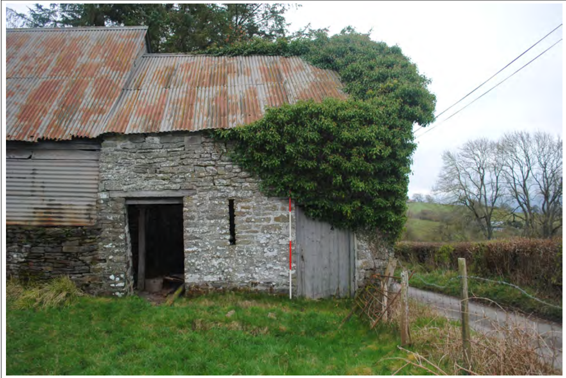
Plate 135. View of two entrances and a ventilation slit on the western elevation for a probable cowhouse or looseboxes (Bays F & G). Looking east-southeast.
