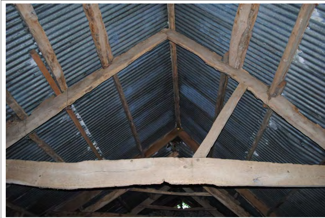
Plate 202. General view of Truss D. Looking south-southwest.
