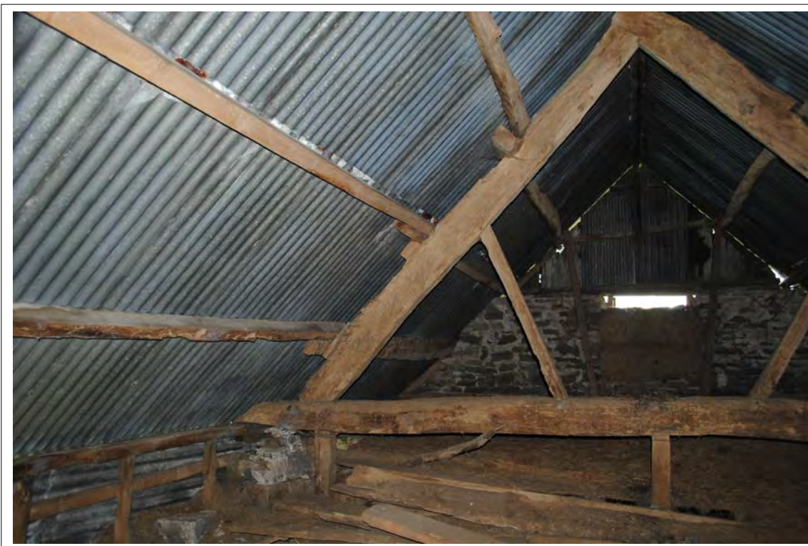
Plate 189. Western side of Truss A. Looking north.
