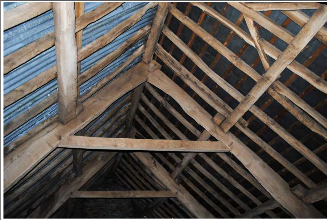
Plate 117. Upper section of Truss D. Looking east.
