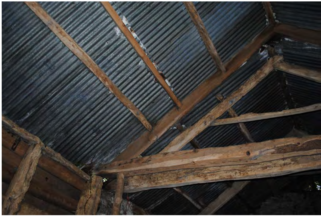
Plate 207. Eastern side of Trusses E1 & E2. Looking south.
