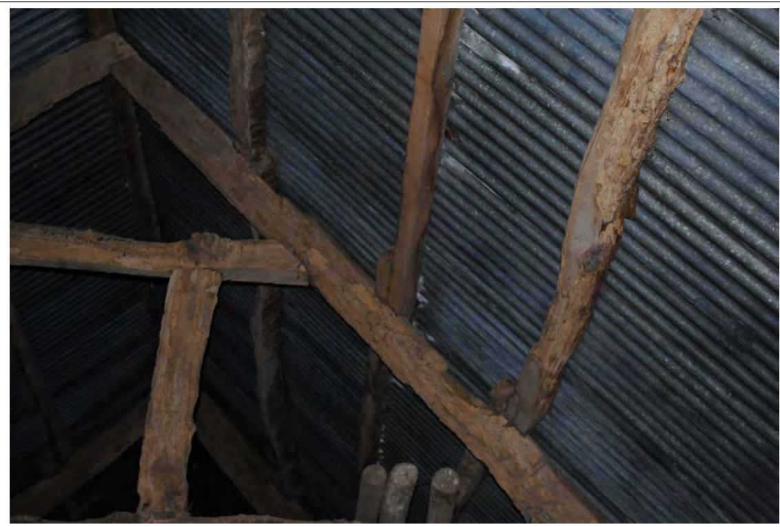
Plate 194. Eastern side of Truss B. Looking north-northeast.
