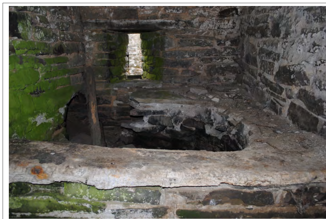
Plate 54. View of ventilation slit and flue for the 'copper' on the eastern wall of Room 1.
