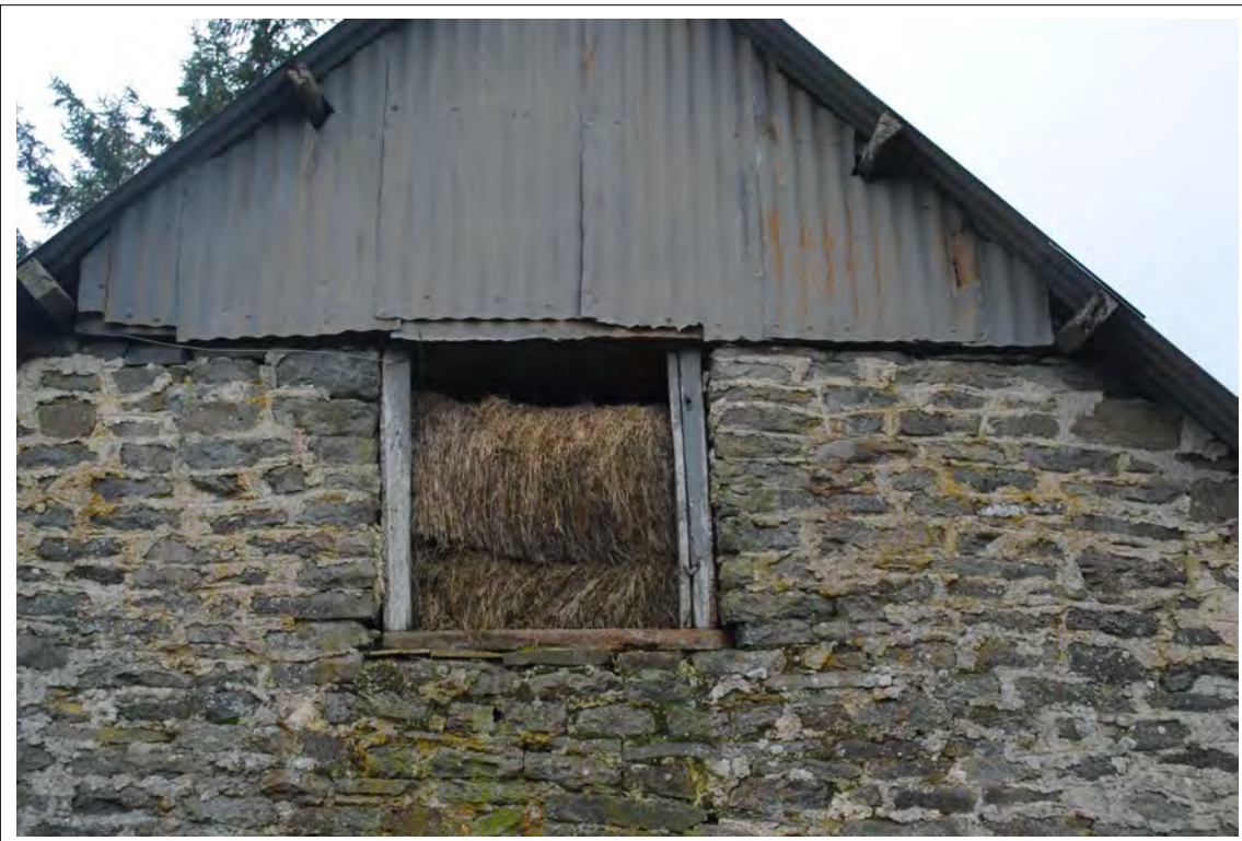
Plate 146. Detail of the pitch-hole on the northern gable. Looking south-southwest.
