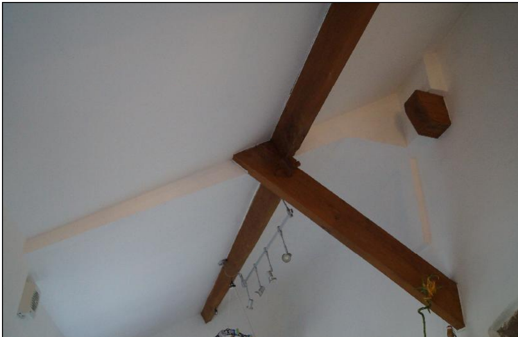
Plate 24: LPT2018_028, An internal view of the ceiling inside the kitchen extension showing the change in rafter height. The lower ceiling reflects the height of the late 19 th century extension to the building, the higher ceiling is modern. Looking south.
