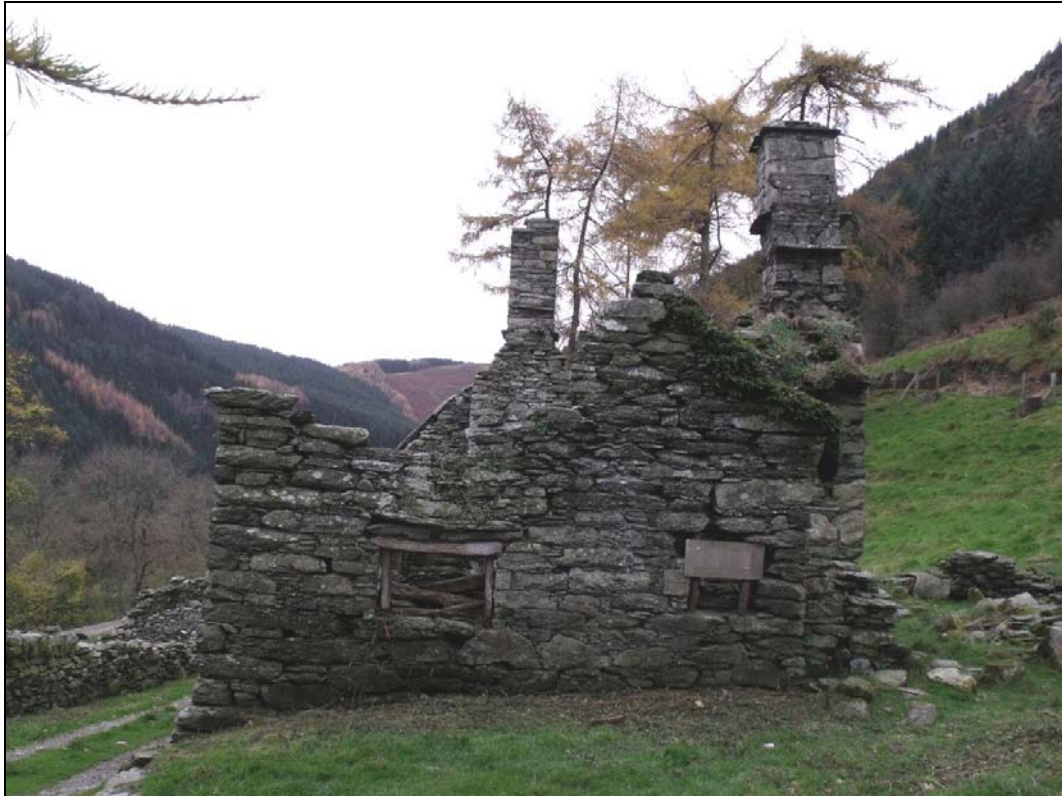
Fig. 8 The partially collapsed eastern gable wall. Photo CPAT 3729-0001
