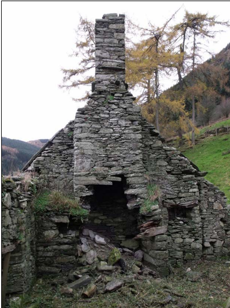
Fig. 6 The collapsed fireplace in the western gable. Photo CPAT 3729-0013
