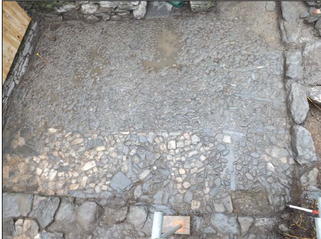
Fig. 9 The cobbled floor in the parlour. Photo CPAT 3800-0059
