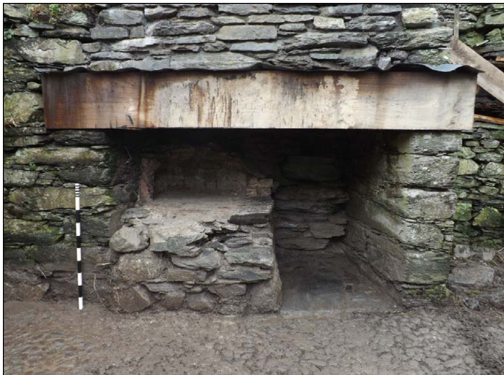
Fig. 10 The repaired fireplace in the parlour with the inserted bread oven on the left. Photo CPAT 3800-0011
