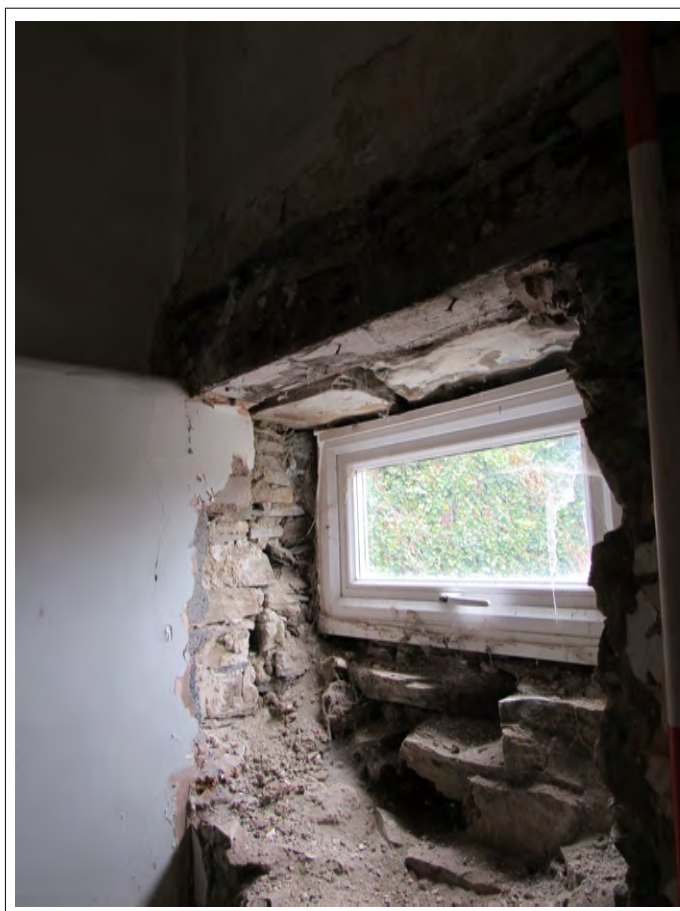
Plate 70. Stairs PVC window. View SE.
