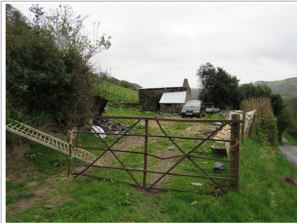
Plate 37. Building remains down the track to the SE. View SE.
