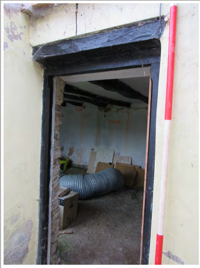
Plate 67. Lounge entrance from porch. View NE. 2m scale
