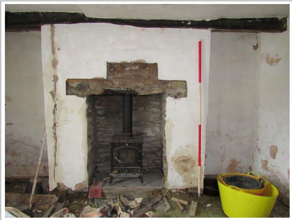
Plate 61. Lounge fireplace. View NW. 2m scale
