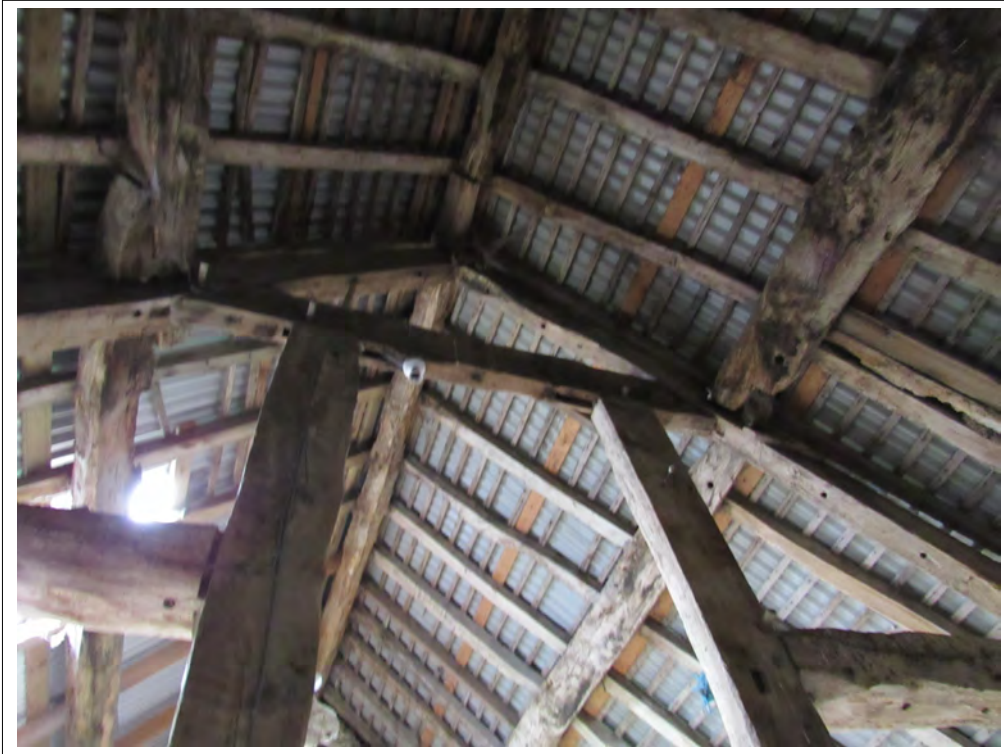
Plate 119. Barn interior, truss frame detail from passage. View SW
