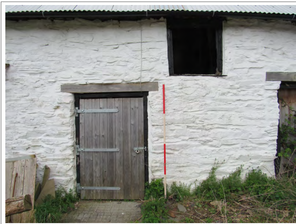
Plate 12. Barn south-east elevation with door. View NW. 2m scale
