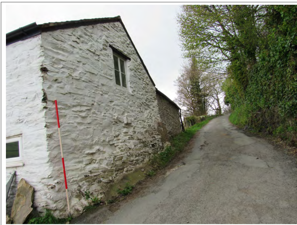
Plate 16. House north-east elevation. View NW. 2m scale
