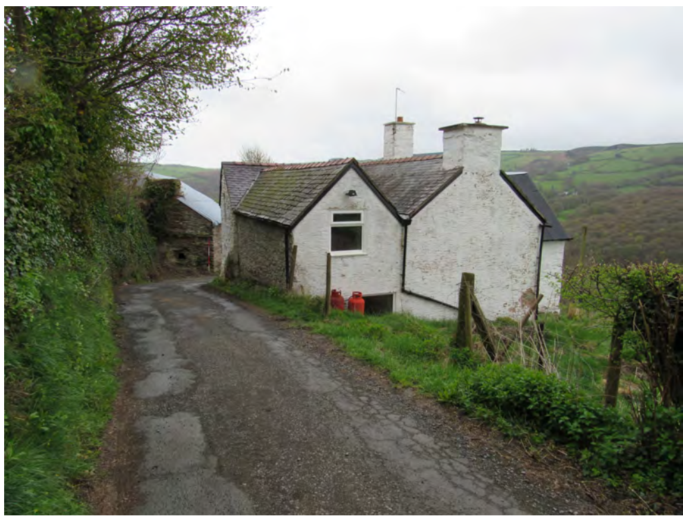
Plate 41. Building remains opposite to the NE. View SE. 2m scale
