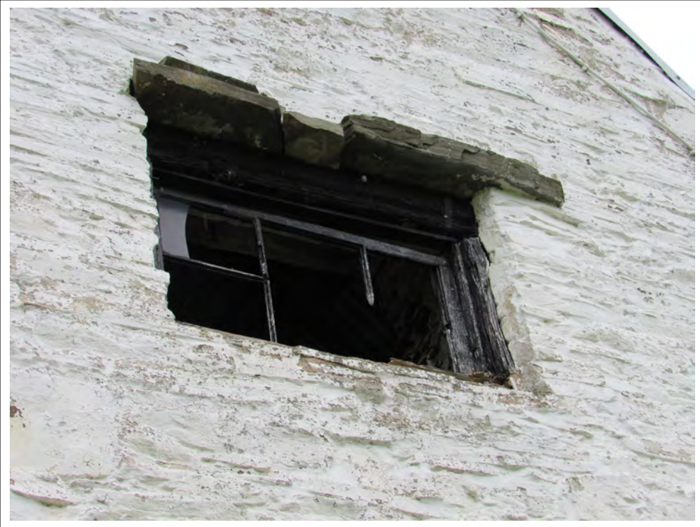
Plate 33. Barn south-west elevation first floor window. View NE.
