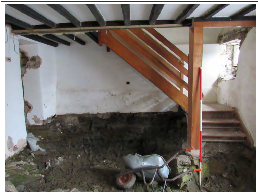
Plate 49. Dining room. View NE. 2m scale
