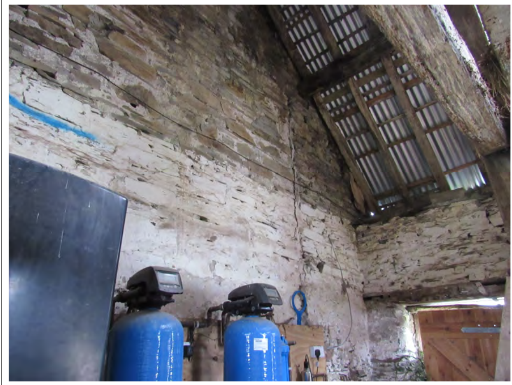
Plate 111. Barn interior, barn passage. View SE. 2m scale
