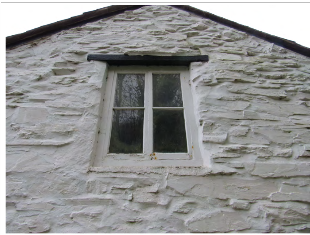
Plate 18. House north-east elevation first floor window. View SW.
