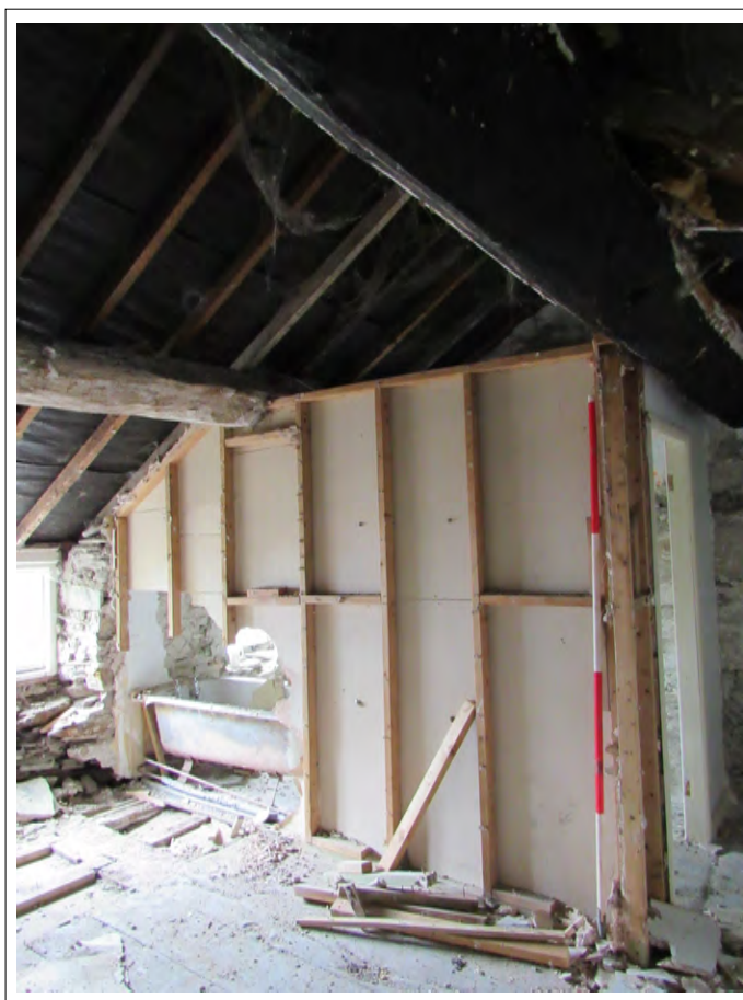
Plate 74. Bedroom 1. View SW. 2m scale
