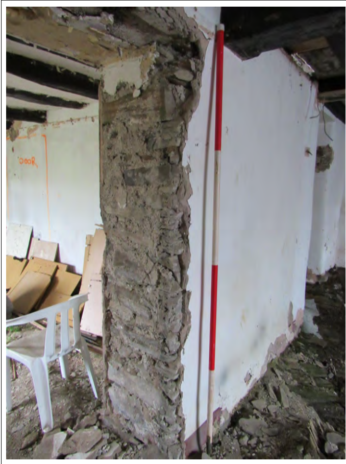
Plate 51. Dining room NW wall, doorway to lounge. View N. 2m scale
