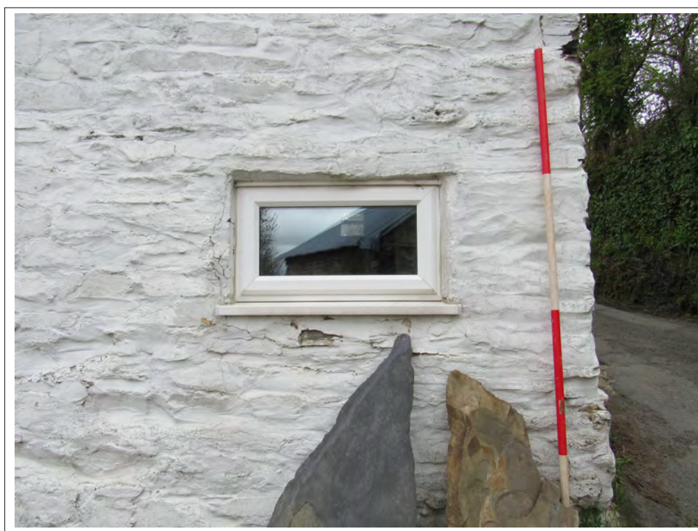
Plate 8. House south-east elevation with stairs PVC window. View NW. 2m scale
