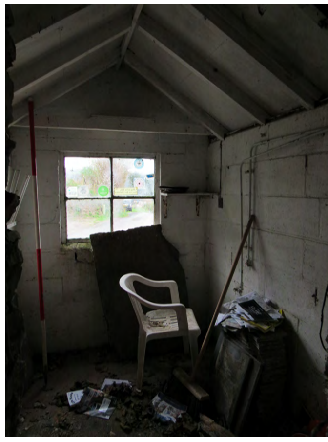
Plate 57. Porch on dining room. View SE. 2m scale
