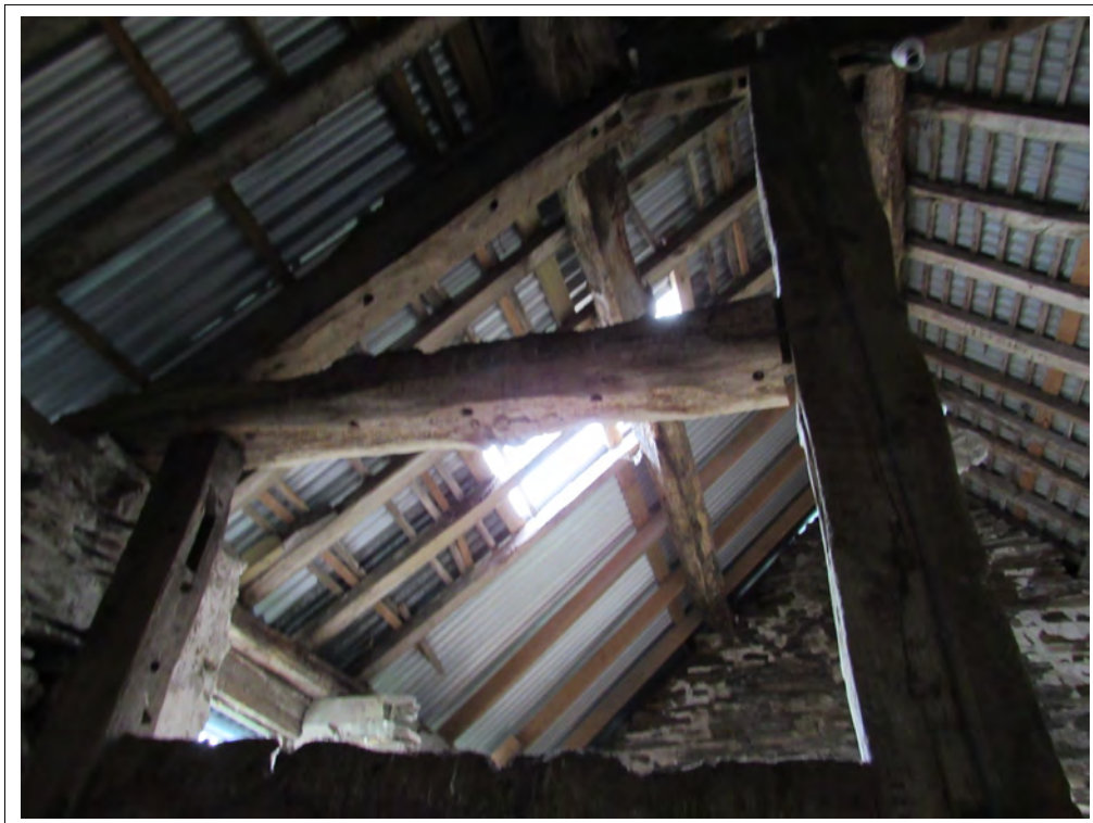
Plate 118. Barn interior, truss frame detail from passage. View SW.
