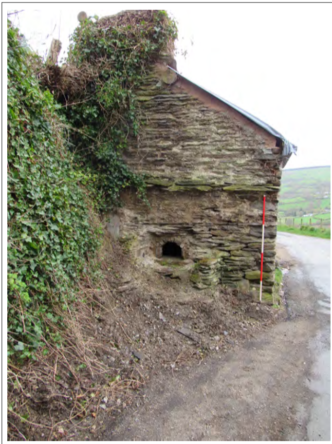
Plate 43. Building remains opposite to the NE. View SE. 2m scale
