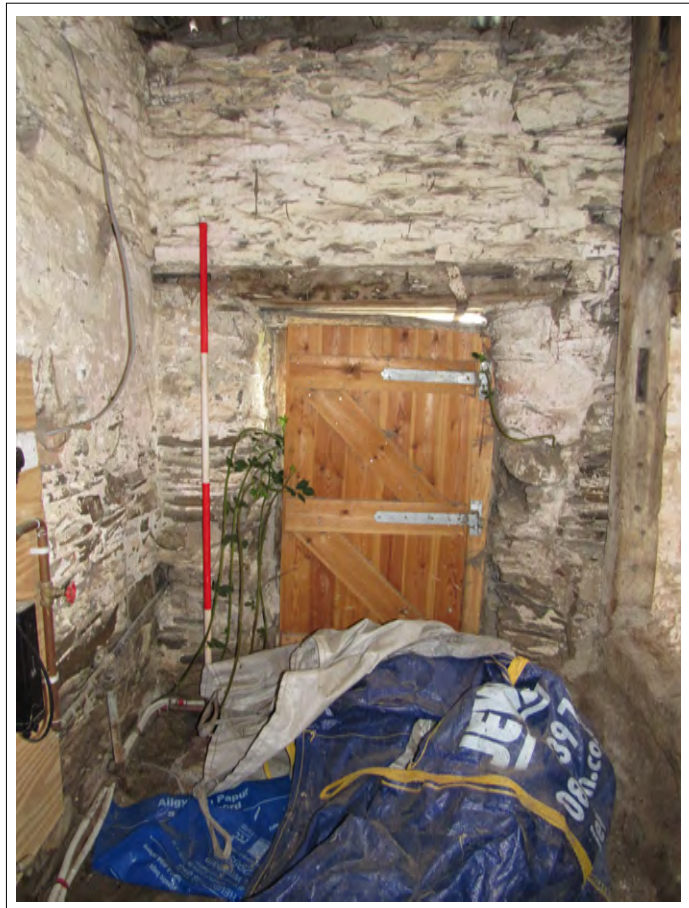
Plate 110. Barn interior doorway of passage. View SE. 2m scale
