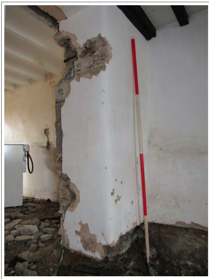
Plate 53. Dining room NW wall, doorway to kitchen. View N. 2m scale
