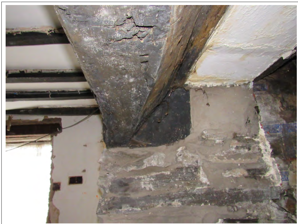
Plate 54. Dining room fireplace mantel. View SE.
