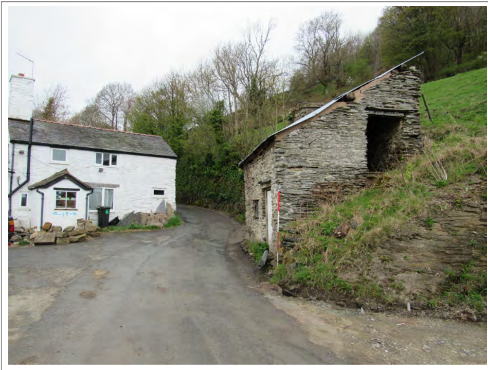
Plate 40. Building remains opposite to the NE. View NW. 2m scale
