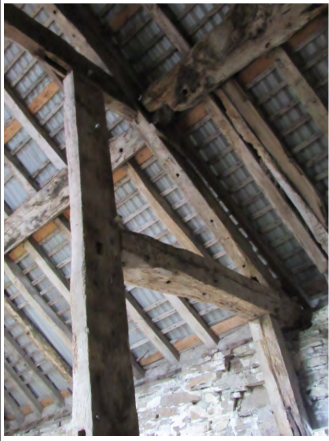
Plate 117. Barn interior, truss frame detail from passage. View W.
