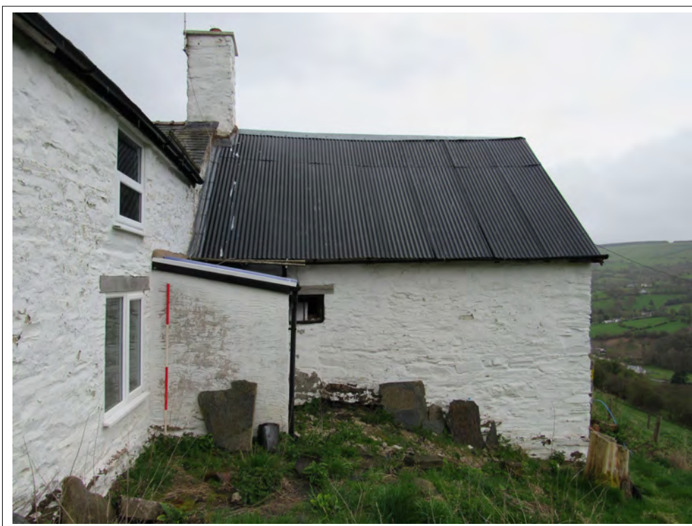
Plate 24. Barn north-west elevation. View SE. 2m scale
