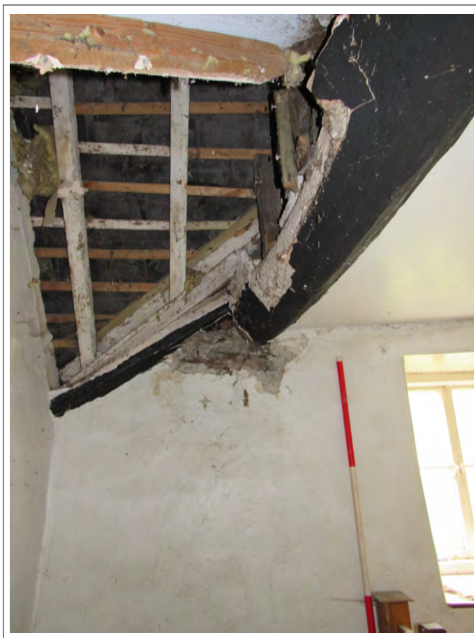
Plate 73. Stairs first floor. View NE. 2m scale
