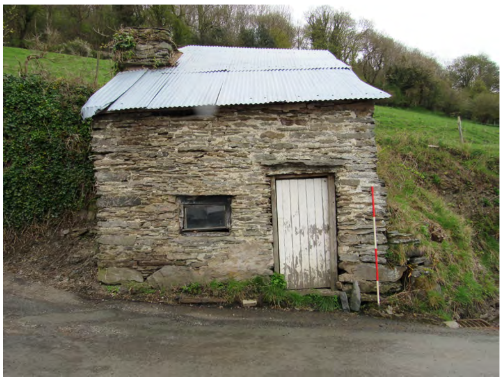
Plate 39. Building remains opposite to the NE. View NE. 2m scale
