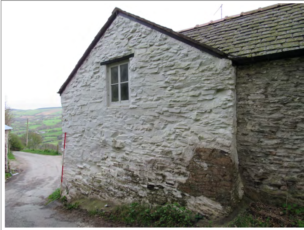
Plate 17. House north-east elevation. View SW. 2m scale
