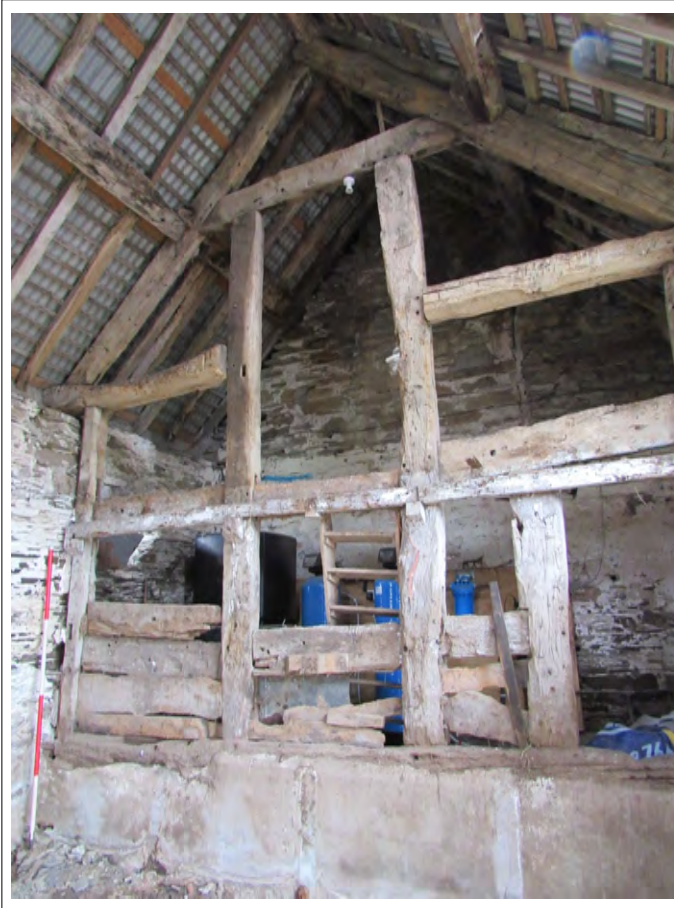
Plate 101. Barn interior with truss. View NE. 2m scale
