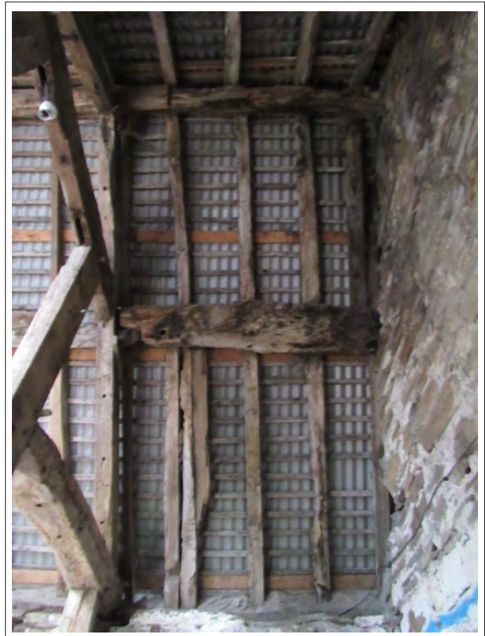
Plate 116. Barn interior, roof above barn passage. View NW. 2m scale
