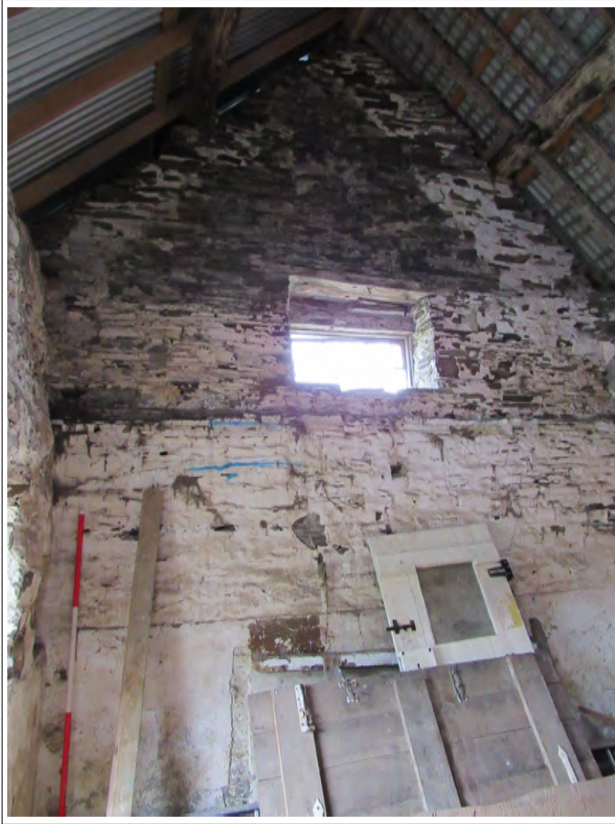
Plate 105. Barn interior. View SE. 2m scale
