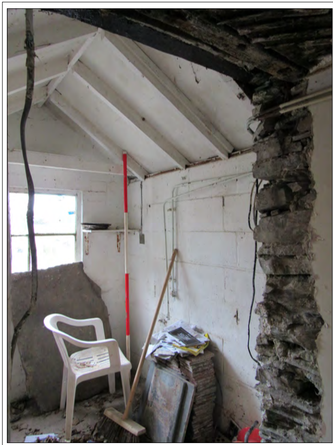
Plate 56. Dining room entrance with modern porch attached. View SE. 2m scale
