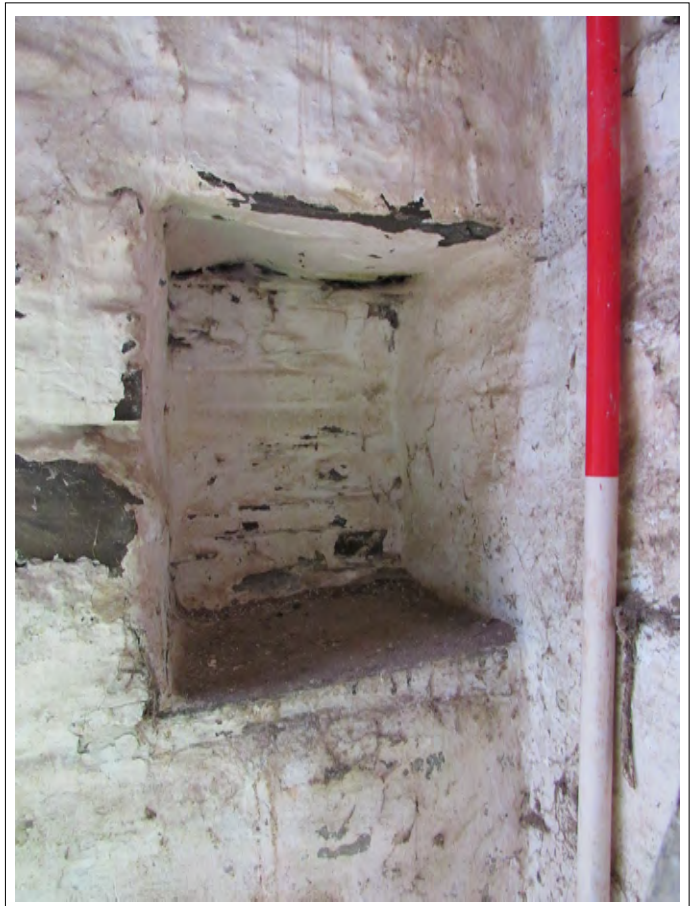
Plate 106. Barn interior blocked window on SE wall. View SE. 2m scale
