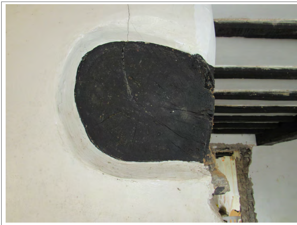
Plate 55. Dining room fireplace mantel. View NW
