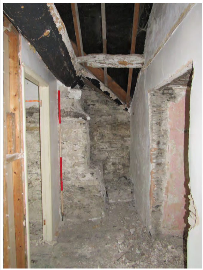
Plate 78. Landing to bathroom with chimney breast. View SW. 2m scale
