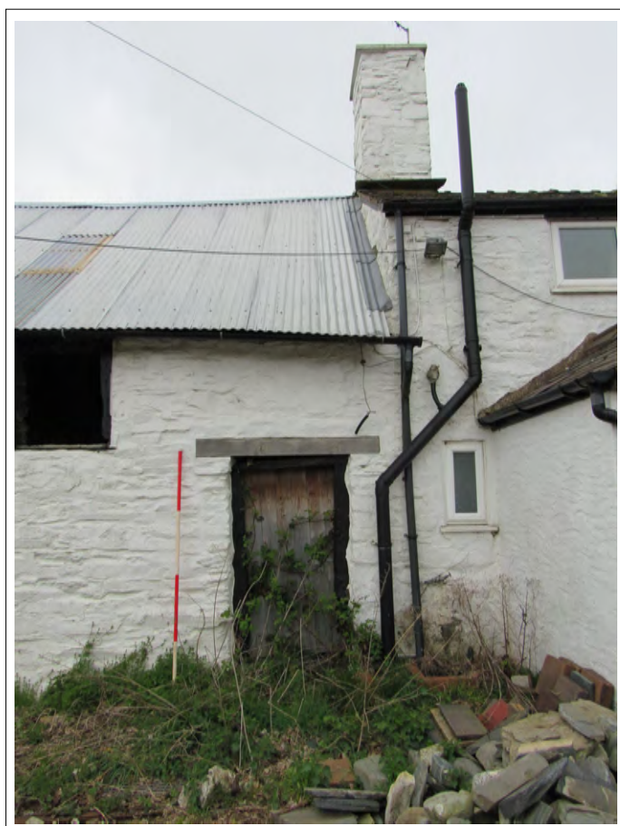
Plate 10. Barn south-east elevation with door. View NW. 2m scale
