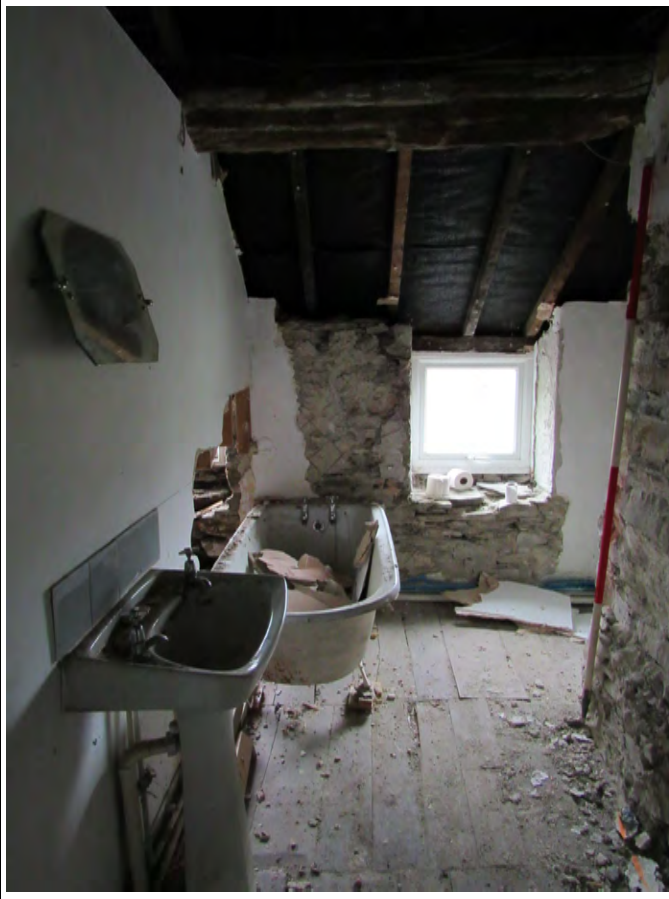
Plate 79. Bathroom. View SE. 2m scale
