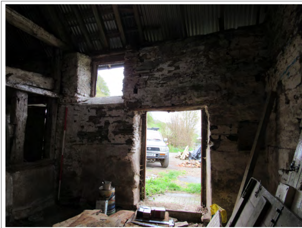
Plate 104. Barn interior. View SE. 2m scale
