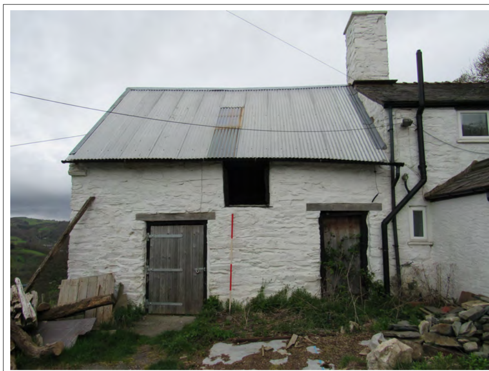
Plate 4. Barn south-east elevation. View NW. 2m scale
