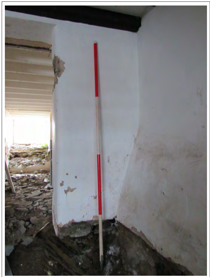
Plate 52. Dining room NW wall, doorway to kitchen. View NW. 2m scale
