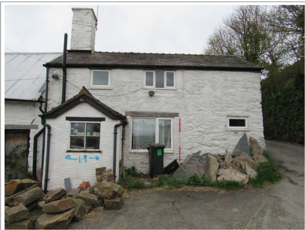
Plate 5. House south-east elevation. View NW. 2m scale
