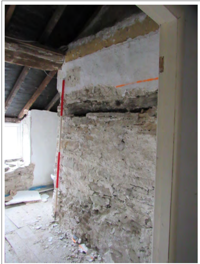
Plate 80. Bathroom with chimney breast. View S. 2m scale
