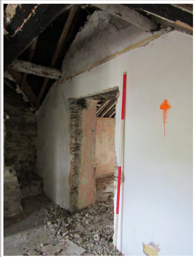
Plate 84. Bedroom 2 doorway from landing. View SW. 2m scale
