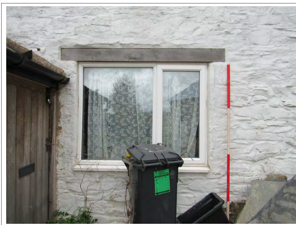
Plate 6. House south-east elevation with ground-floor PVC window. View NW. 2m scale
