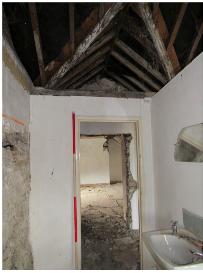
Plate 83. Bathroom with view to Bedroom 2. View NW. 2m scale
