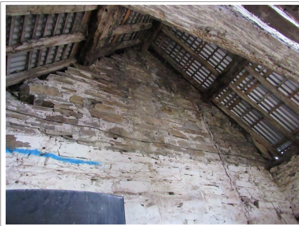
Plate 113. Barn interior, SW wall to house. View NE.
