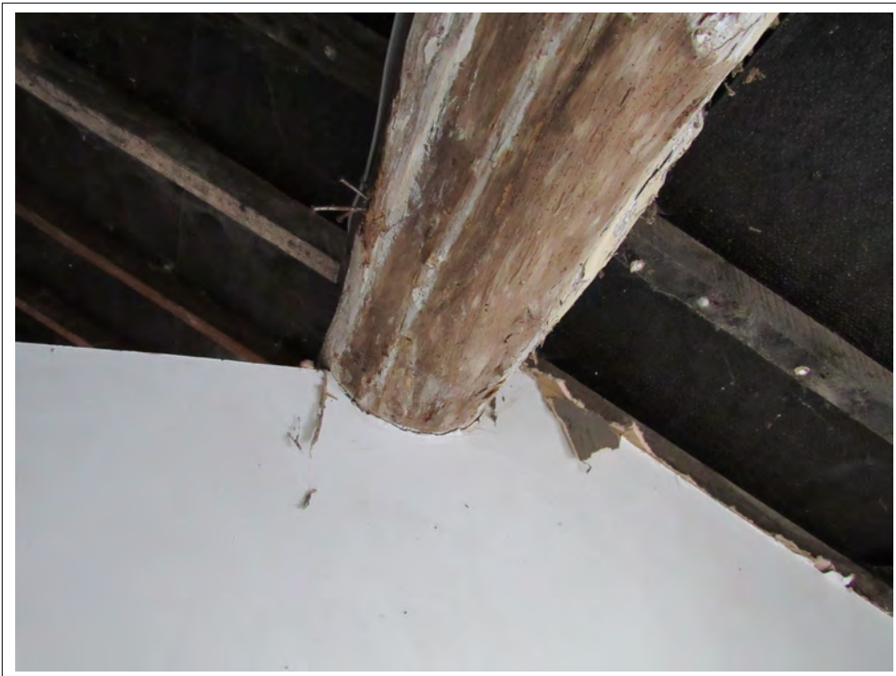
Plate 82. Bathroom with purlin visible. View NE.
