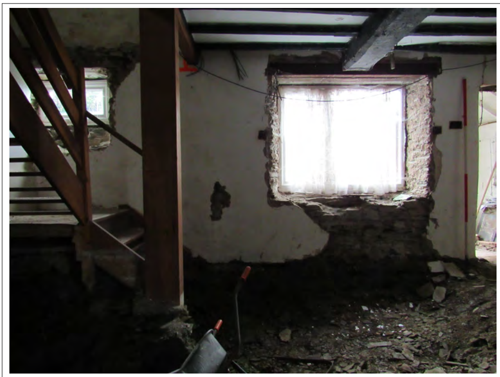
Plate 48. Dining room. View SE. 2m scale
