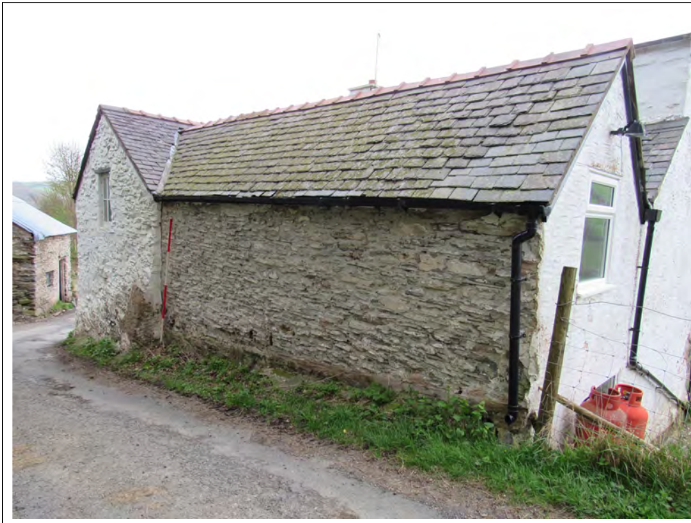
Plate 19. House north-east elevation with later extension. View S. 2m scale
