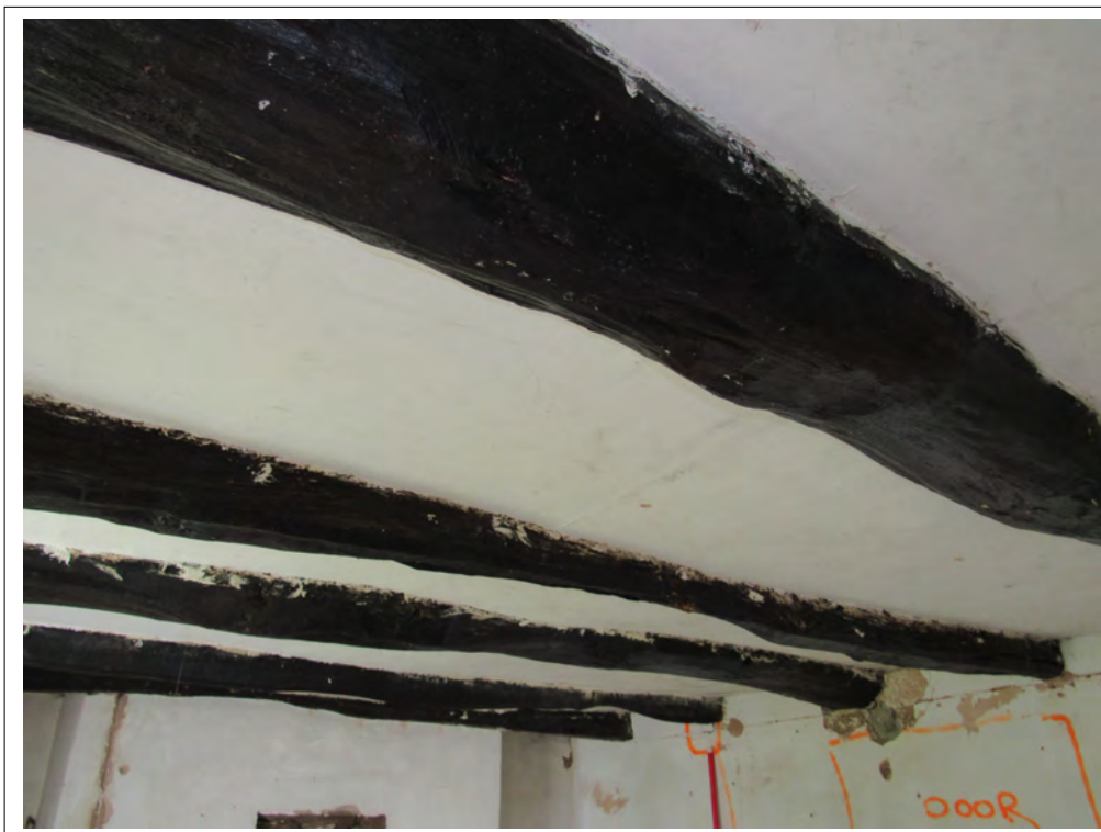
Plate 63. Lounge beams. View N. 2m scale
