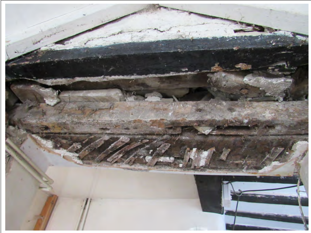
Plate 59. Dining room entrance from porch, door lintel. View NW.
