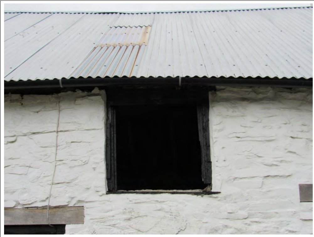
Plate 13. Barn south-east elevation window. View NW.
