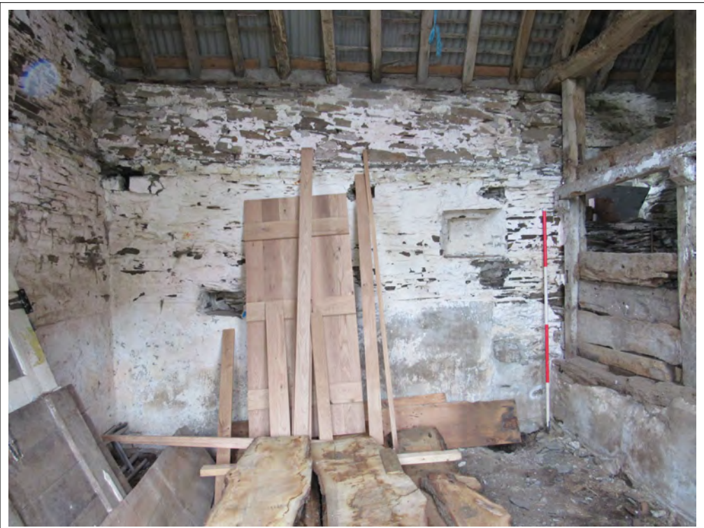
Plate 99. Barn interior. View NW. 2m scale
