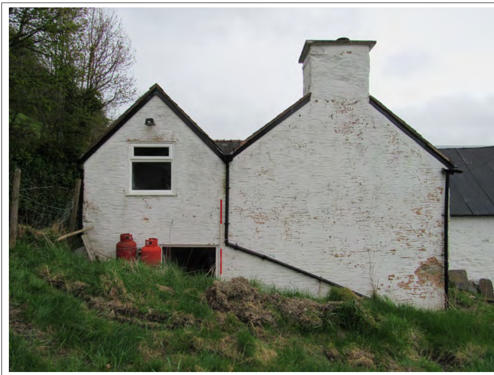
Plate 23. House north-west elevation. View SE. 2m scale
