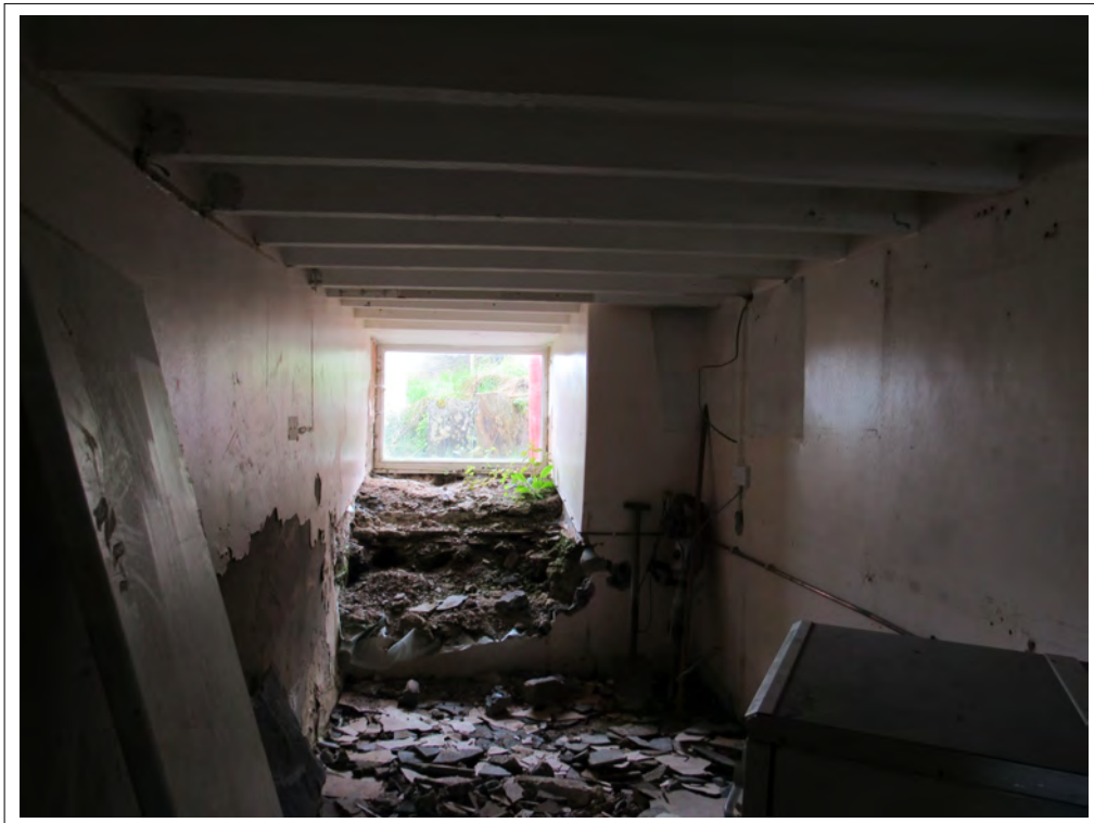
Plate 68. Kitchen extension. View NW. 2m scale
