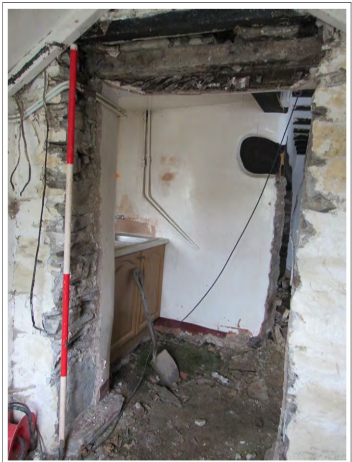
Plate 58. Entrance to dining room. View NW. 2m scale
