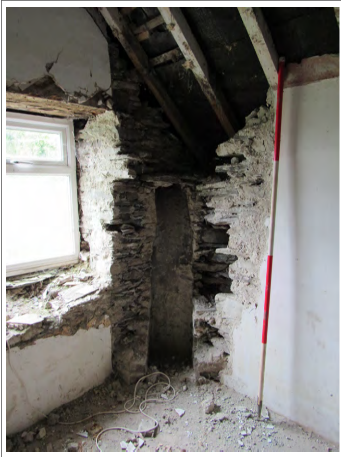
Plate 93. Bedroom 3 fireplace location. View N. 2m scale
