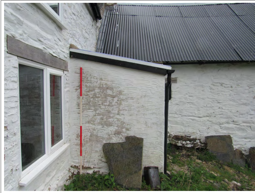
Plate 25. Barn north-west elevation with modern porch extension. View SE. 2m scale
