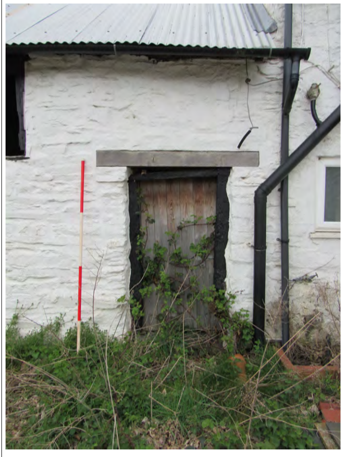
Plate 11. Barn south-east elevation with door. View NW. 2m scale
