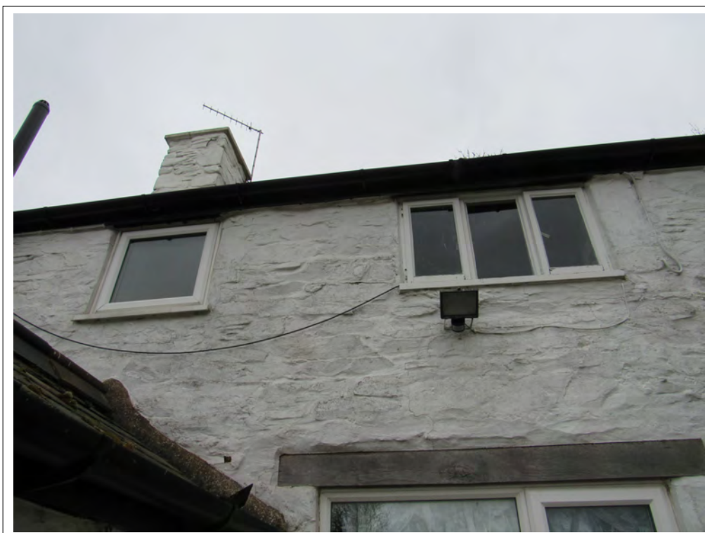
Plate 7. House south-east elevation with first floor PVC windows. View NW.
