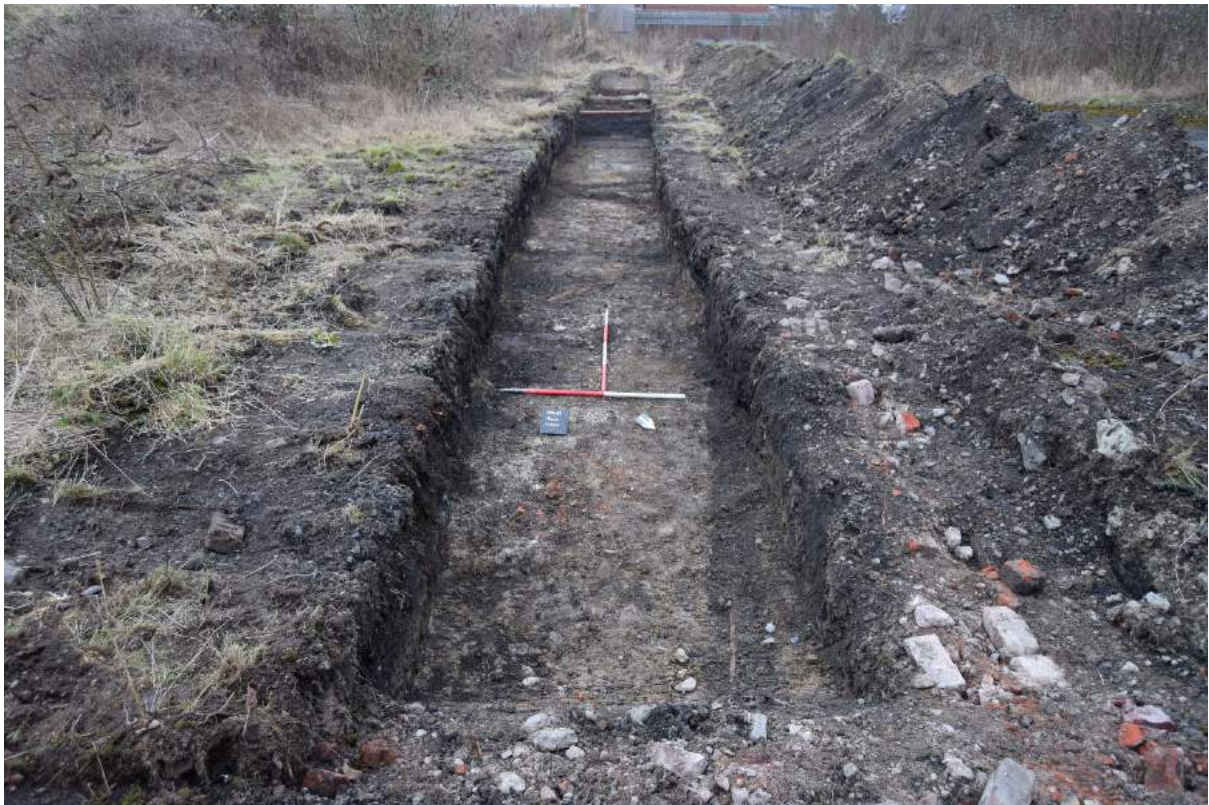
Plate 18: General view of Trench 4, with modern flats in the background; shot facing southwest.
