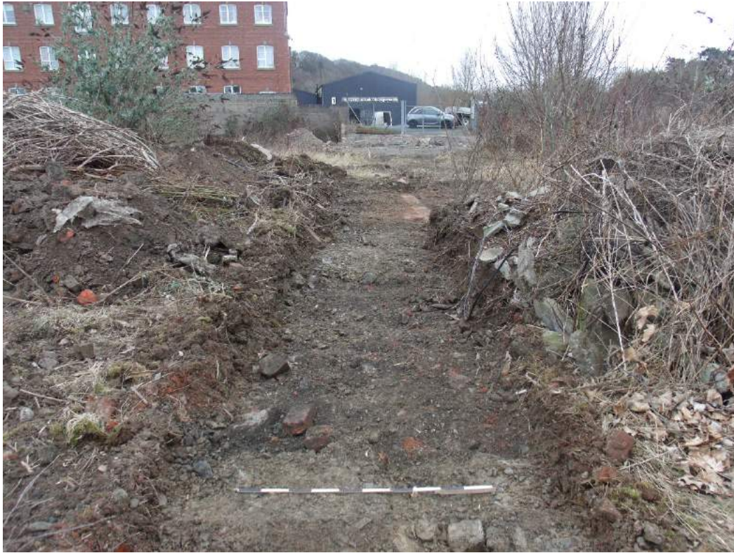
Plate 44: Re-opening of northeastern end of Trench 2: possible floor remains and brick wall at the northeast corner; shot facing northeast.
