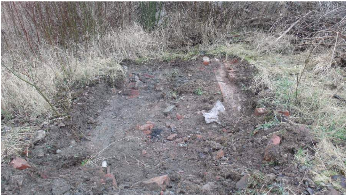
Plate 6: Opening of Trench 1 – found asbestos; shot facing southwest.
