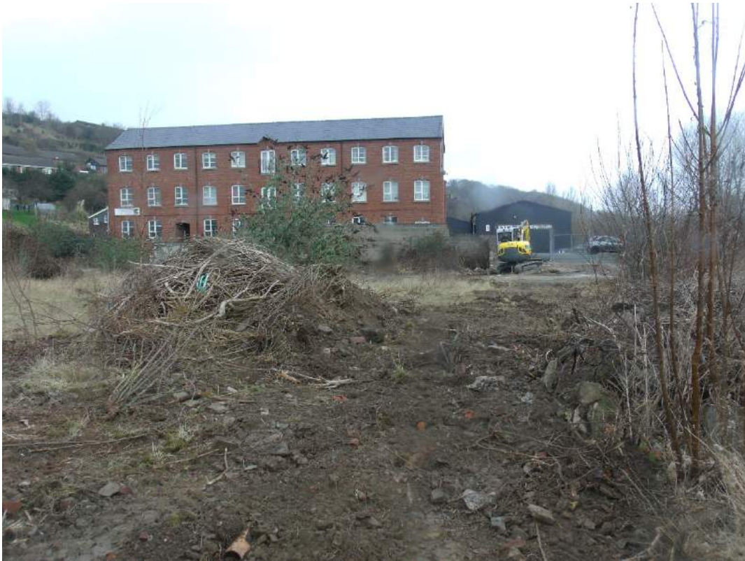
Plate 47: End of evaluation, trenches backfilled; shot facing northeast.
