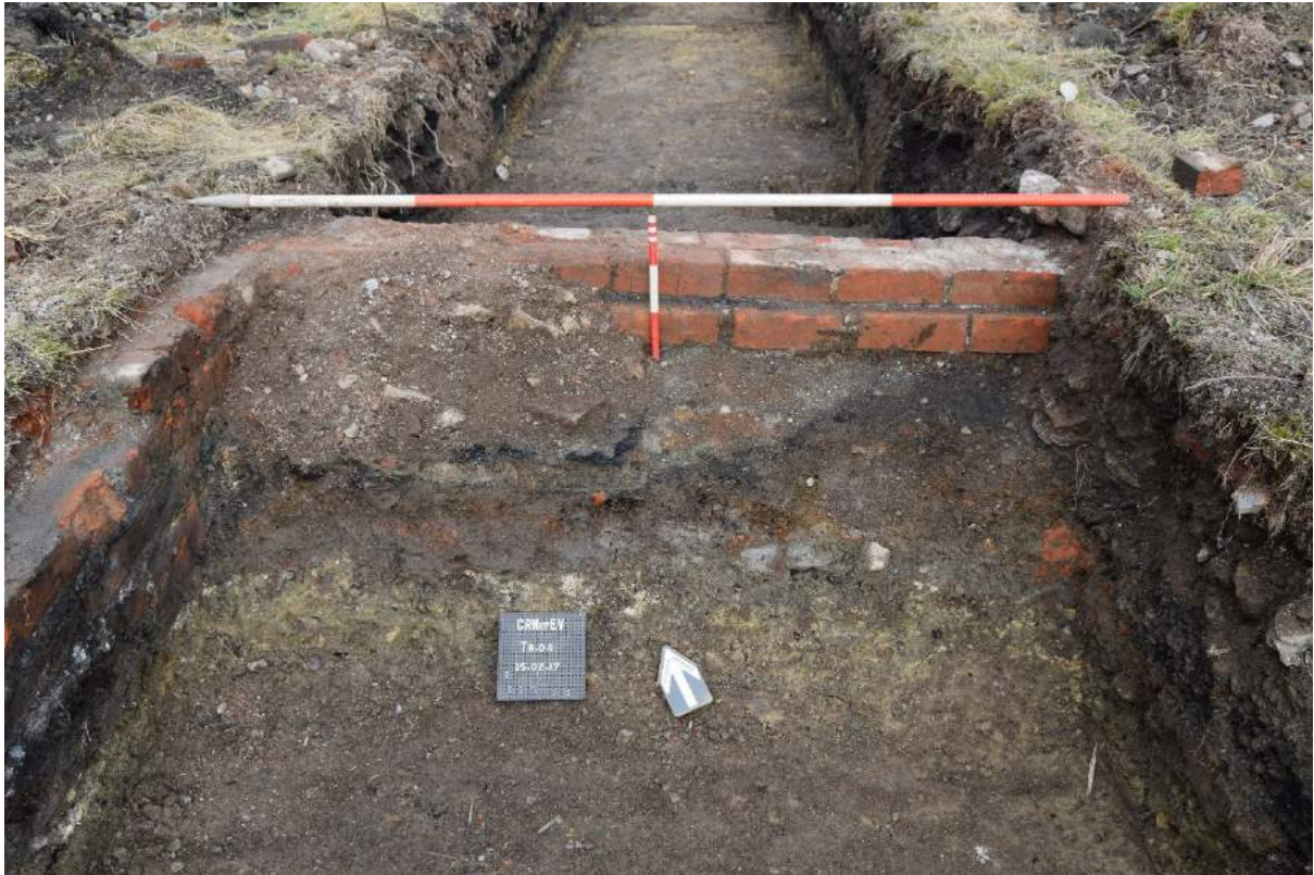
Plate 31: Detail of bricks wall in Trench 4 after excavation, with associated deposits; shot facing northeast.
