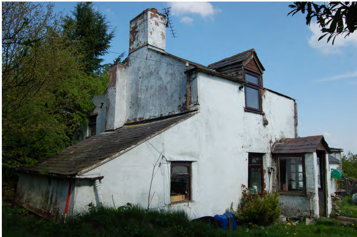
Plate 9. Western end of original house, with chimney stacks and lean-to bread-oven room. View northeast. Scale 1m
