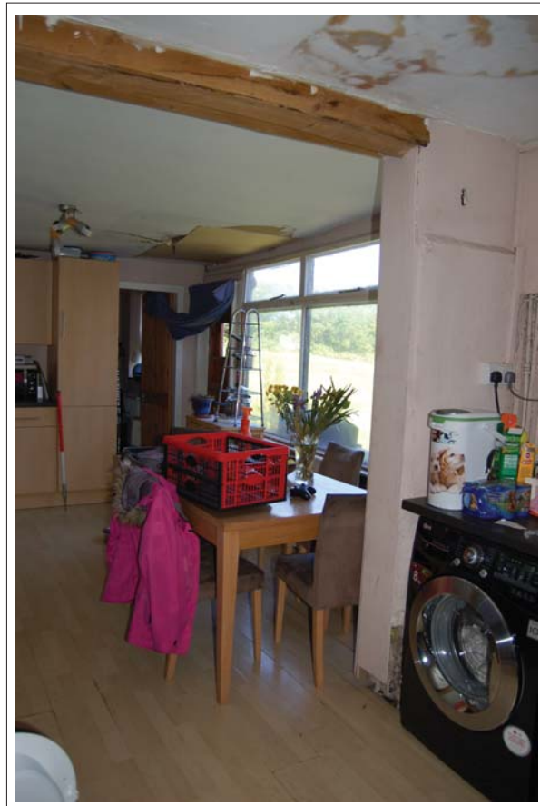
Plate 26. Northern extension, kitchen from hallway. View north. Scale 1 m
