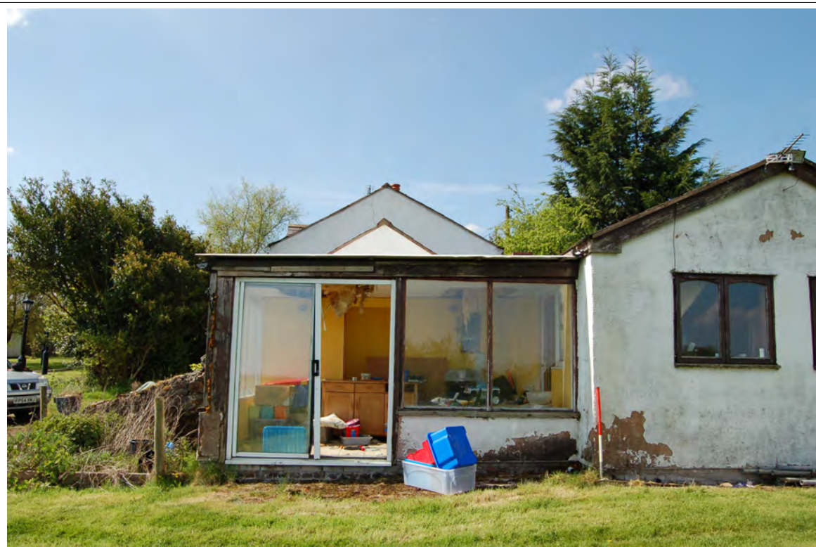
Plate 6. Modern extensions to the east of the original barn, original exterior door and window features visible, now internally. View west. Scale 1m
