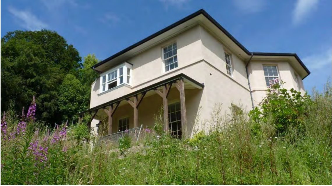
Photo 3: View northeast of the western elevation of Mount Severn, showing the projecting veranda. Photo taken from scrub-covered falling ground to the southwest of the house.
