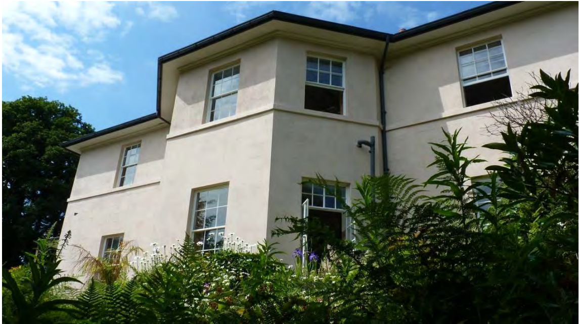
Photo 1: View northwest of the main southern elevation of Mount Severn.
