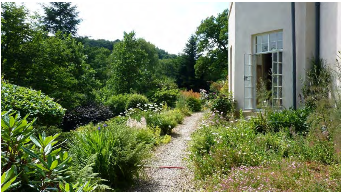
Photo 6: View west showing the path in front of the south elevation, with the garden area to the left. 1m scale.
