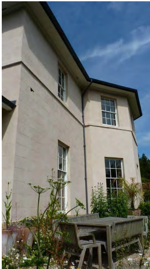
Photo 2: View ENE of the main southern elevation of Mount Severn.
