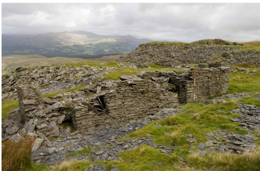
Figure 27. Barracks at Cloddfa Gwanas quarry (nprn 527068)
