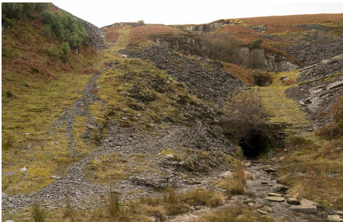
Figure 31. Minllyn slate quarry, showing an inclined plane (nprn 527475) to the left. Right of centre is the tunnel exit (nprn 527462) from a large quarry pit, which replaced the inclined plane on the right side (nprn 527474)
