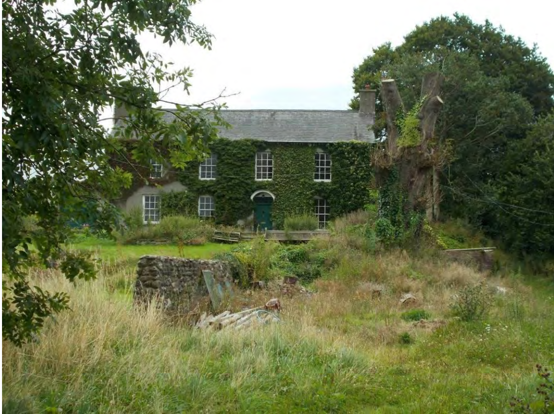
Photo 15: View southeast of The Vicarage (LB 10942), a listed building on the southern side of Llangadog.
