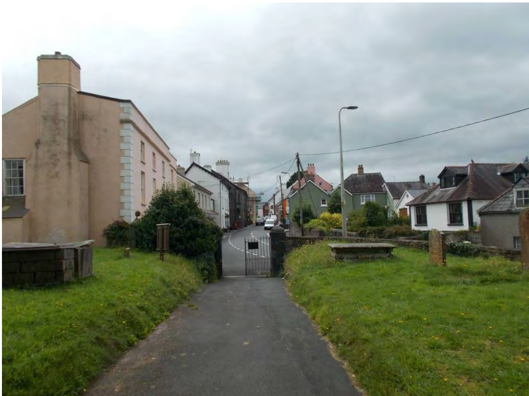
Photo 14: General view south from St Cadoc's church (LB 10936), looking into Llangadog, illustrating the limited visibility of the many listed buildings within the closely packed settlement.
