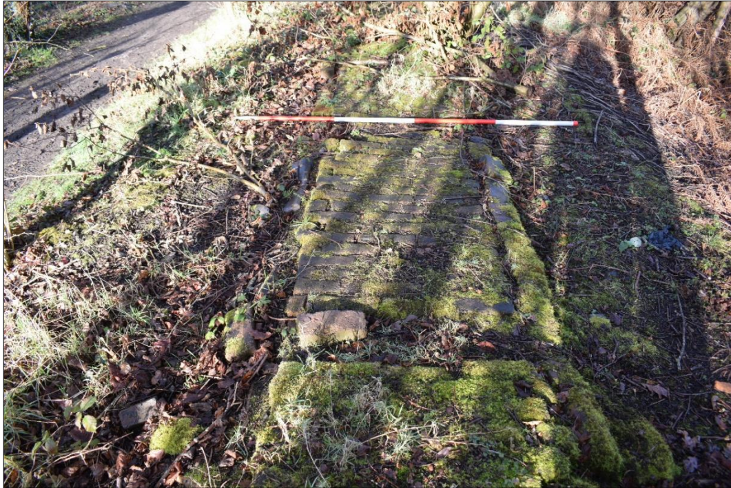
Fig. 27 A section of brick base for the tramway to the Mount Pleasant Brickworks, with the footpath to the left. Photo CPAT 4446-0034
