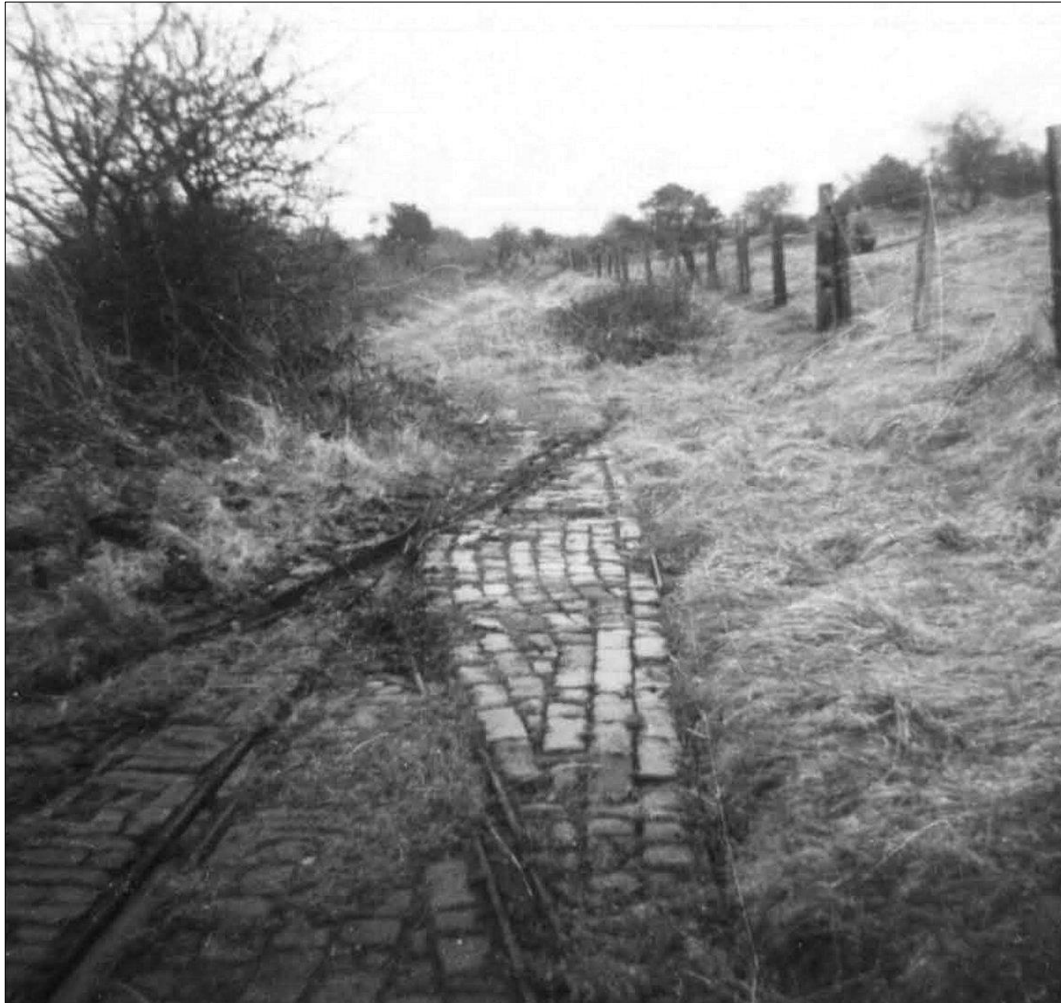
Fig.9 A section of tramway uncovered in 1967, showing the five-way junction, viewed from the north-north-west. Photo James Bentley (courtesy of the Buckley Society)
