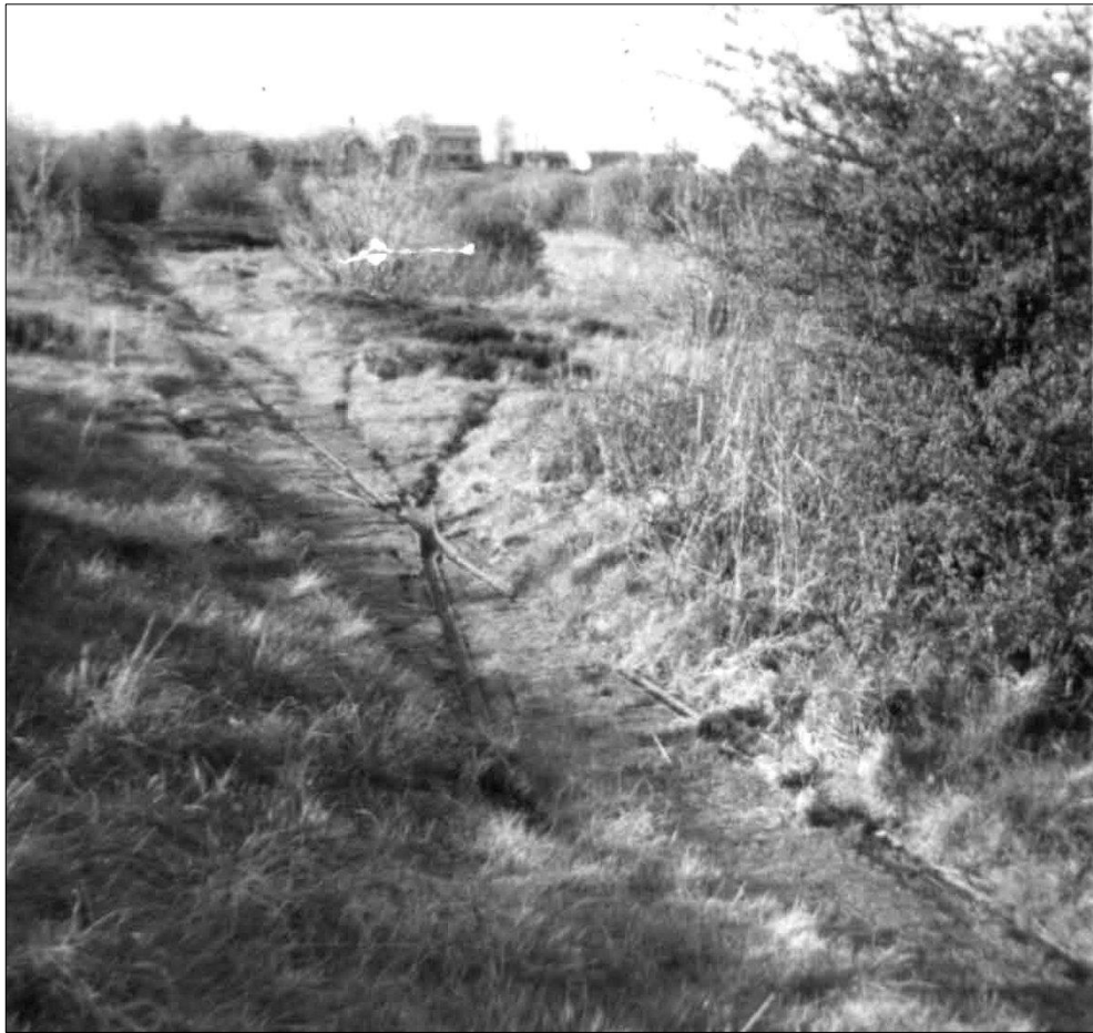
Fig. 10 A section of tramway uncovered in 1967, showing the five-way junction, viewed from the south-south-west. Photo James Bentley (courtesy of the Buckley Society)
