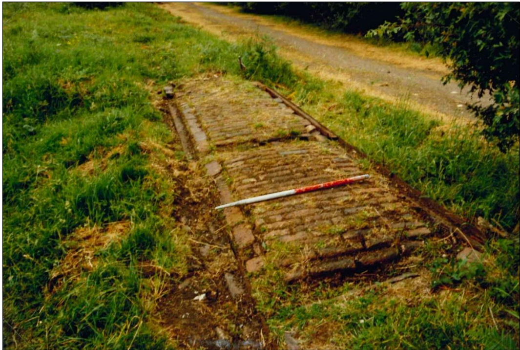
Fig. 23 One of the tramways approaching the traverser siding alongside the standard gauge siding in June 1994. Photo Cadw
