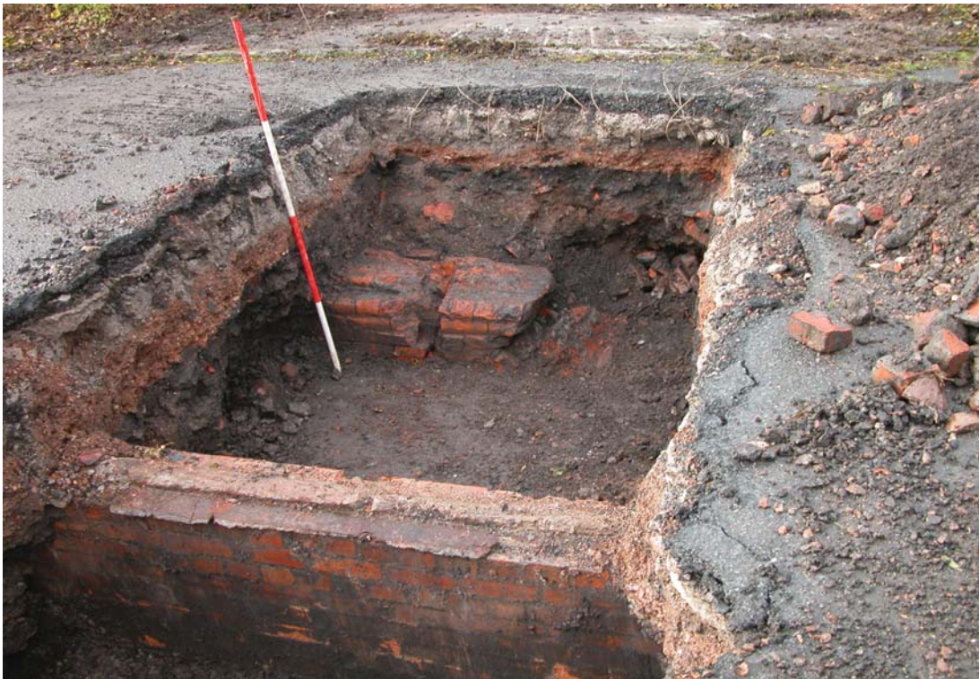
Plate 04: Tr.2, The damaged western wall of the Compressor House. CAP Report No. 542
