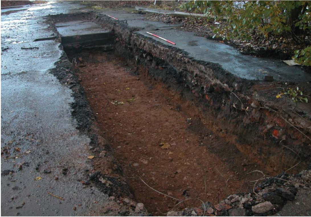
Plate 01: Tr.1, Oblique shot of West facing section showing natural (059) at base.
