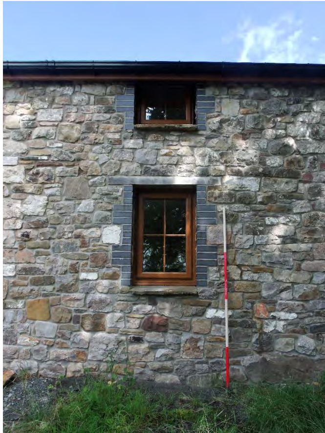
Plate 3: Front (south) elevation, windows view; shot facing N. 2m scale.
