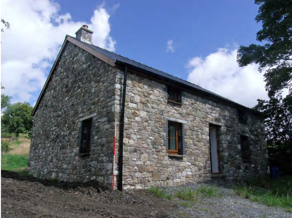
Plate 5: West side and Front (south) elevations; shot facing NE. 2m scale.
