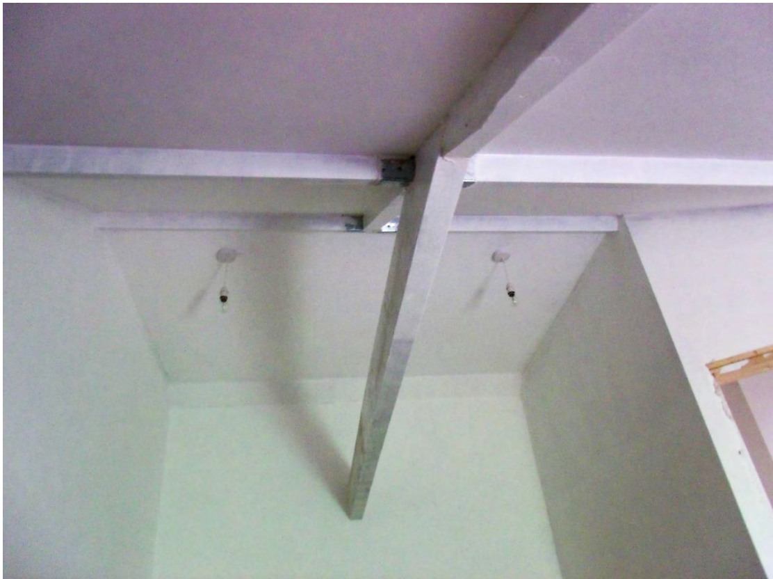
Plate 37: Interior, first floor, Room 2 detailed view of trusses; shot facing S-SW
