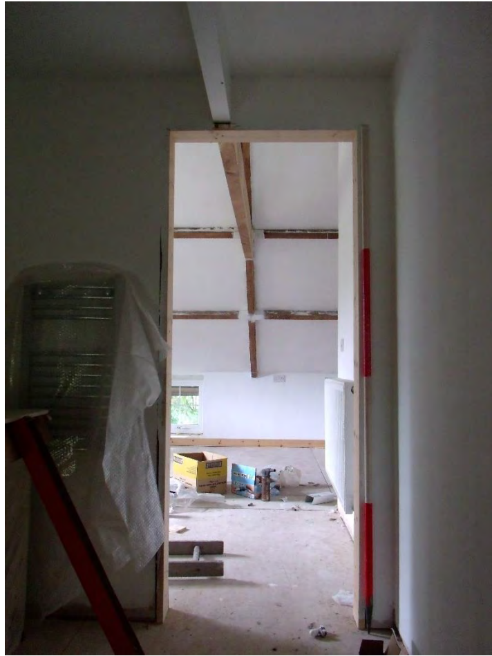
Plate 30: Interior, first floor, Room 1 entrance; view towards S. 2m scale.
