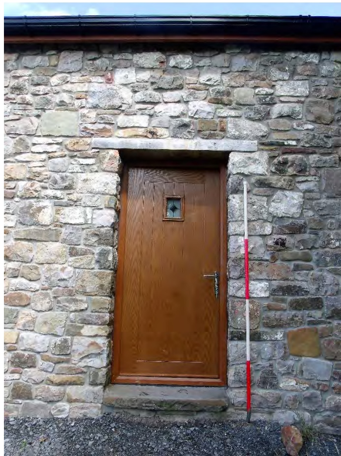
Plate 2: Front (south) elevation, door view; shot facing N. 2m scale.
