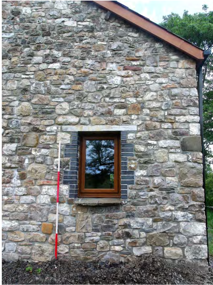
Plate 7: West side elevation, view of window; shot facing E. 2m scale.
