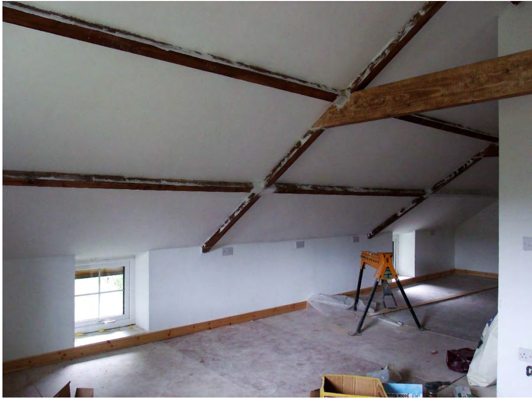
Plate 32: Interior, first floor, Room 1 general view; view towards SW
