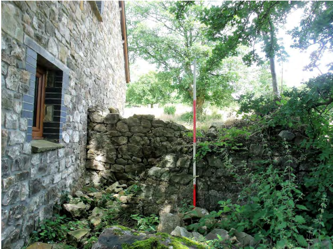
Plate 17: Lean-on structure general view from S; shot facing N. 2m scale.
