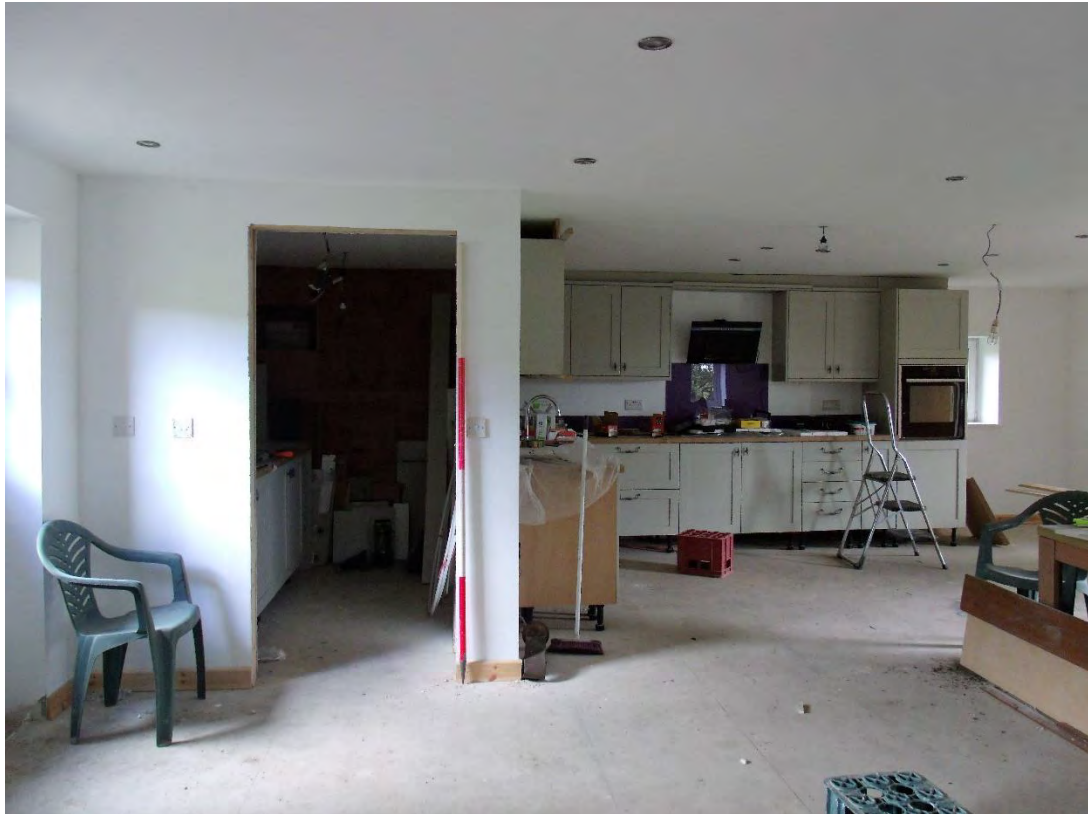
Plate 23: Interior, ground floor; view towards E. 2m scale.
