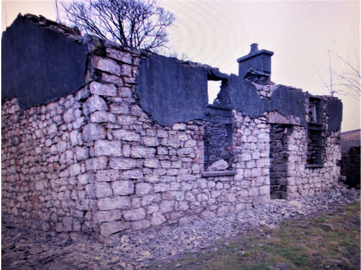
Plate 48: Photo of the house taken prior to renovation work, showing front (South) elevation and part of the west elevation. Shot facing ENE
