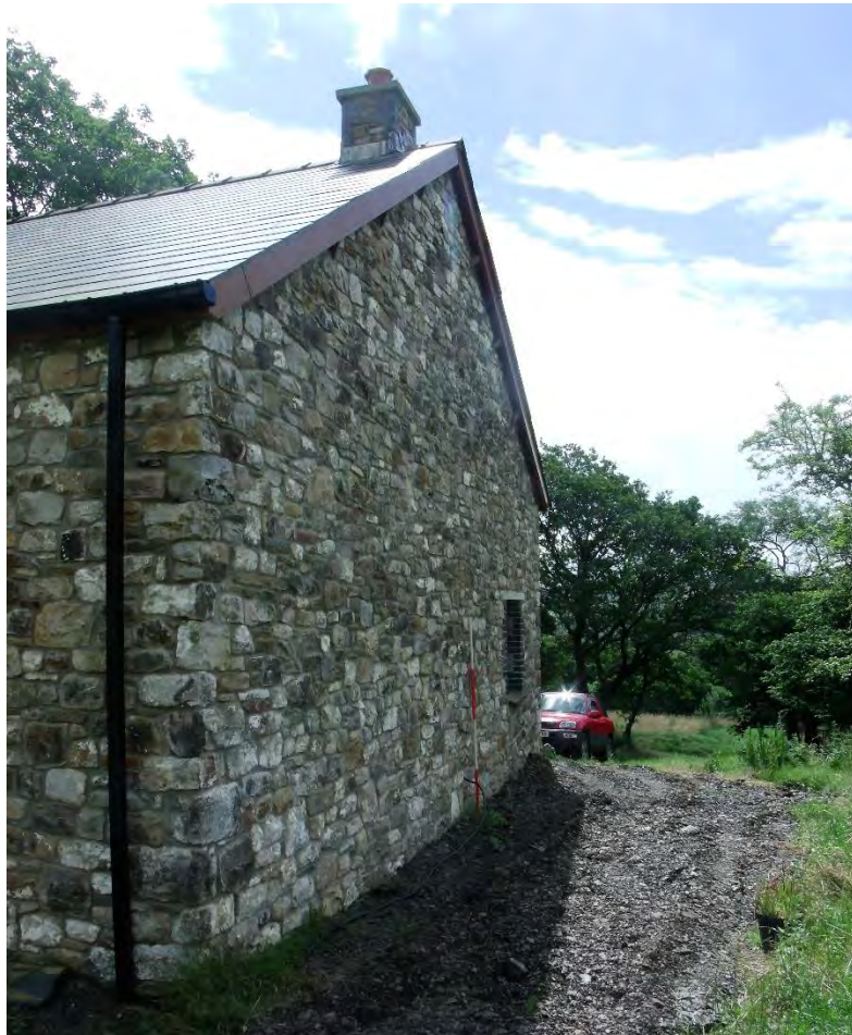
Plate 6: West side elevation; shot facing S-SE. 2m scale.
