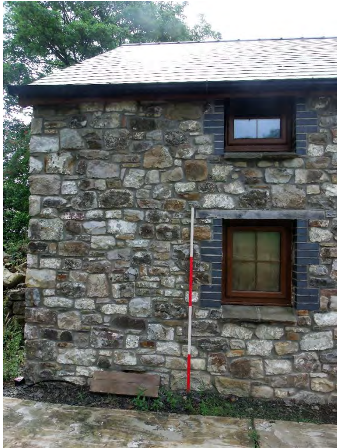
Plate 11: Rear (north) side elevation, windows view; shot facing S. 2m scale.
