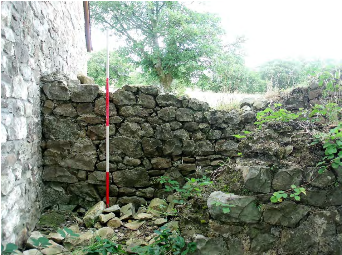
Plate 18: Lean-on structure, detailed view from S; shot facing N. 2m scale.
