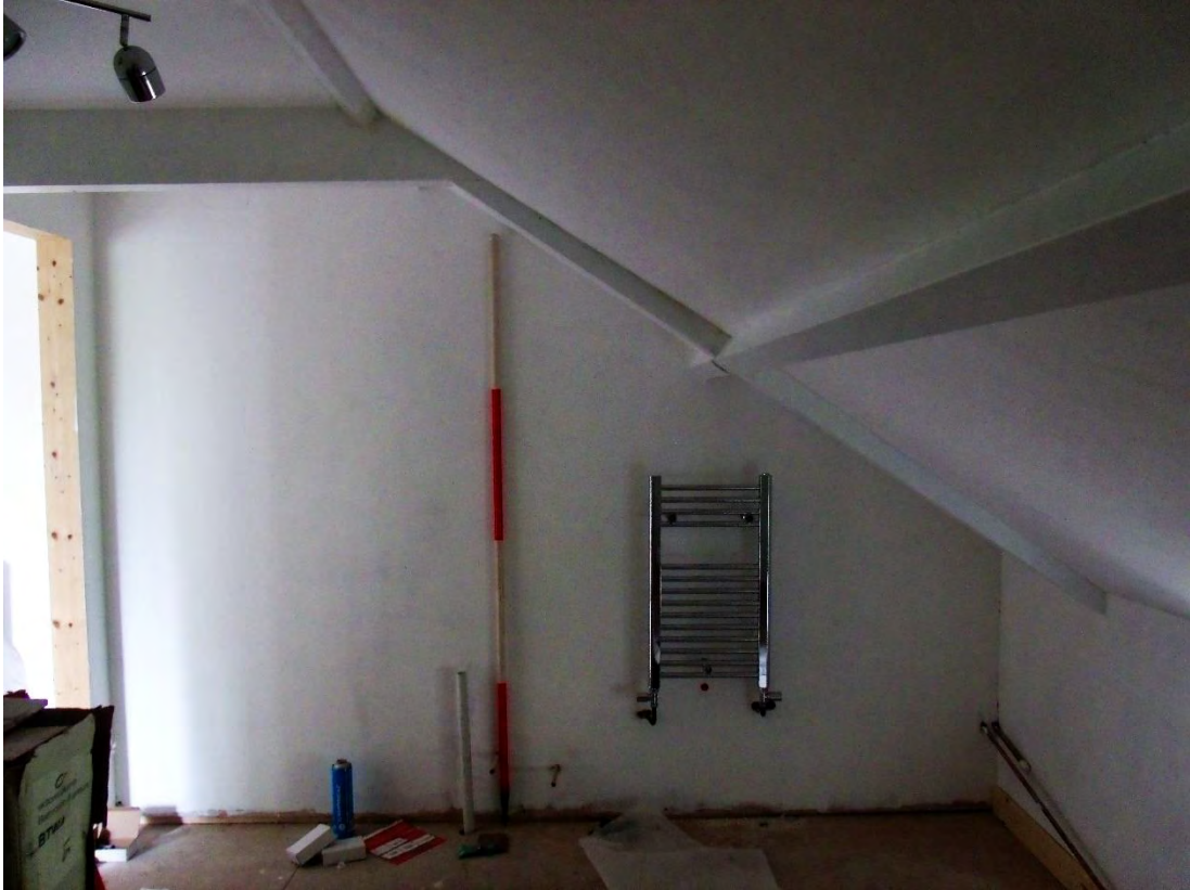
Plate 36: Interior, first floor, Room 2 general view towards W. 2m scale.
