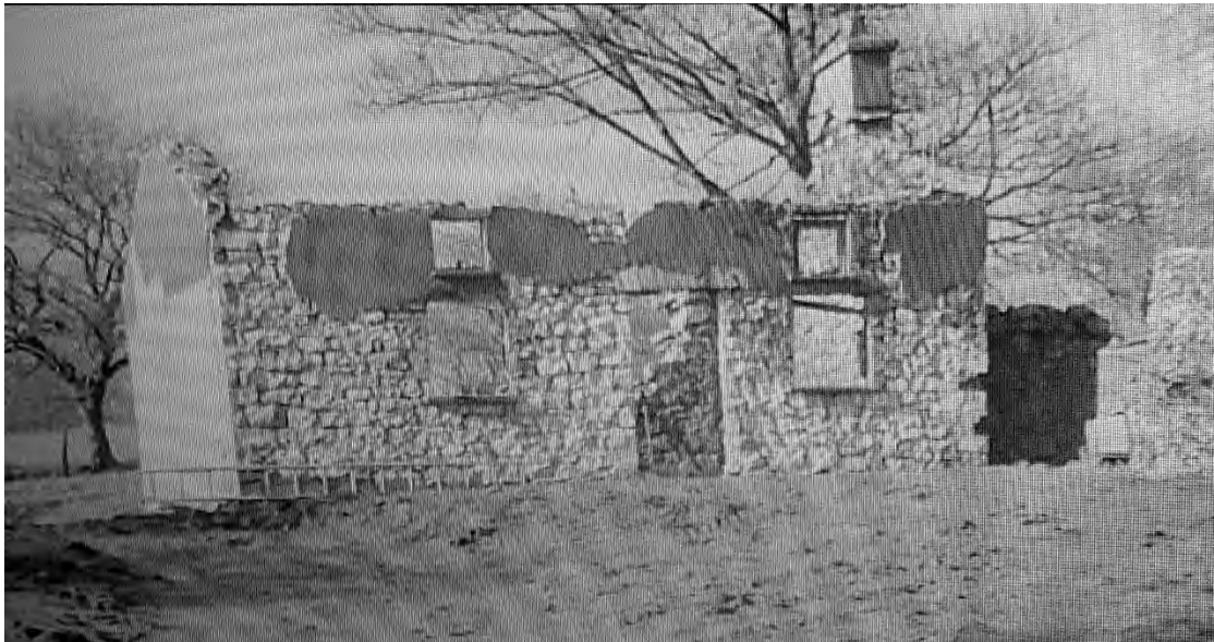
Plate 47: Photo of the house taken prior to renovation work, showing front (South) elevation. Shot facing NNE
