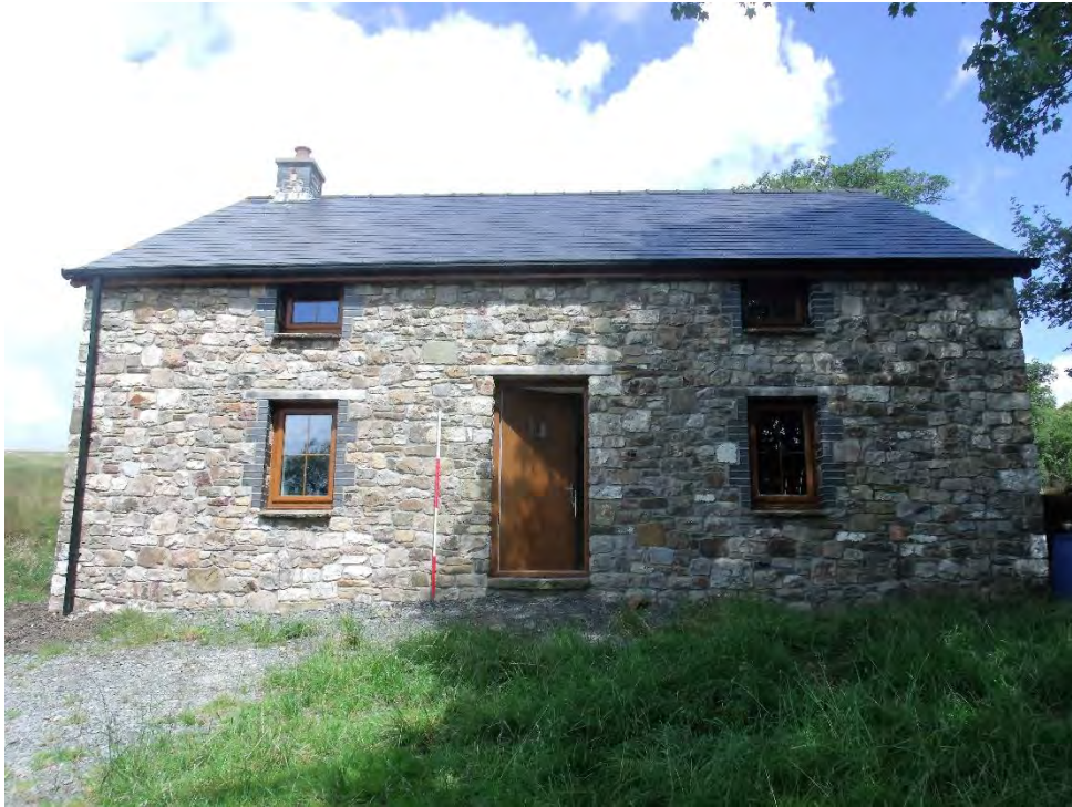
Plate 1: Front (south) elevation, general view; shot facing N. 2m scale.
