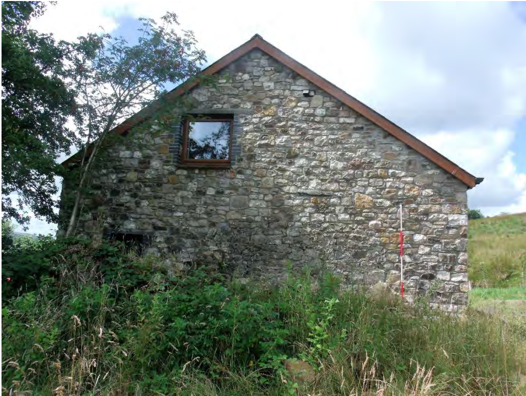
Plate 13: East side elevation, general view; shot facing W. 2m scale.
