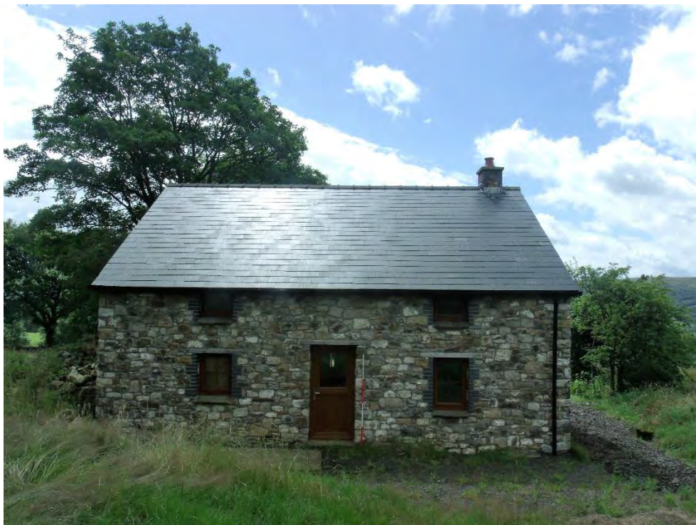
Plate 8: Rear (north) side elevation, general view; shot facing S. 2m scale.
