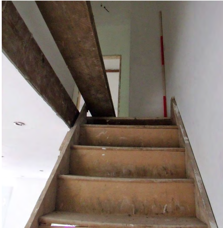
Plate 27: Interior, staircase to first floor; view towards S. 2m scale.
