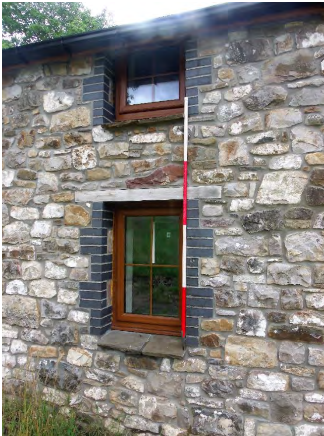
Plate 10: Rear (north) side elevation, Windows view; shot facing S-SE. 2m scale.
