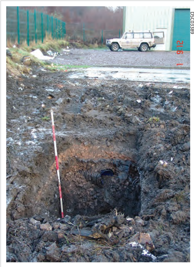
Plate 01: Soak-away 1. Various layers of land II and drain
