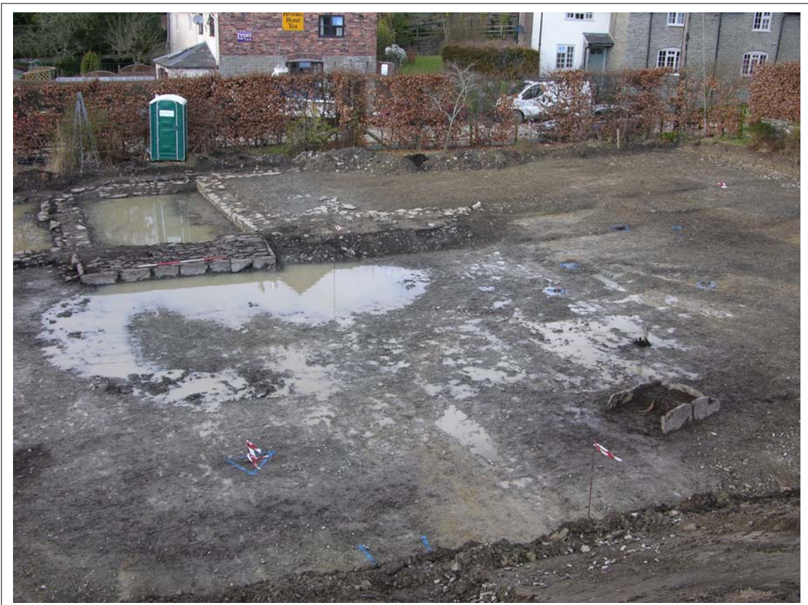
Plate 3: General overview of excavation area, Scale 1x2m
