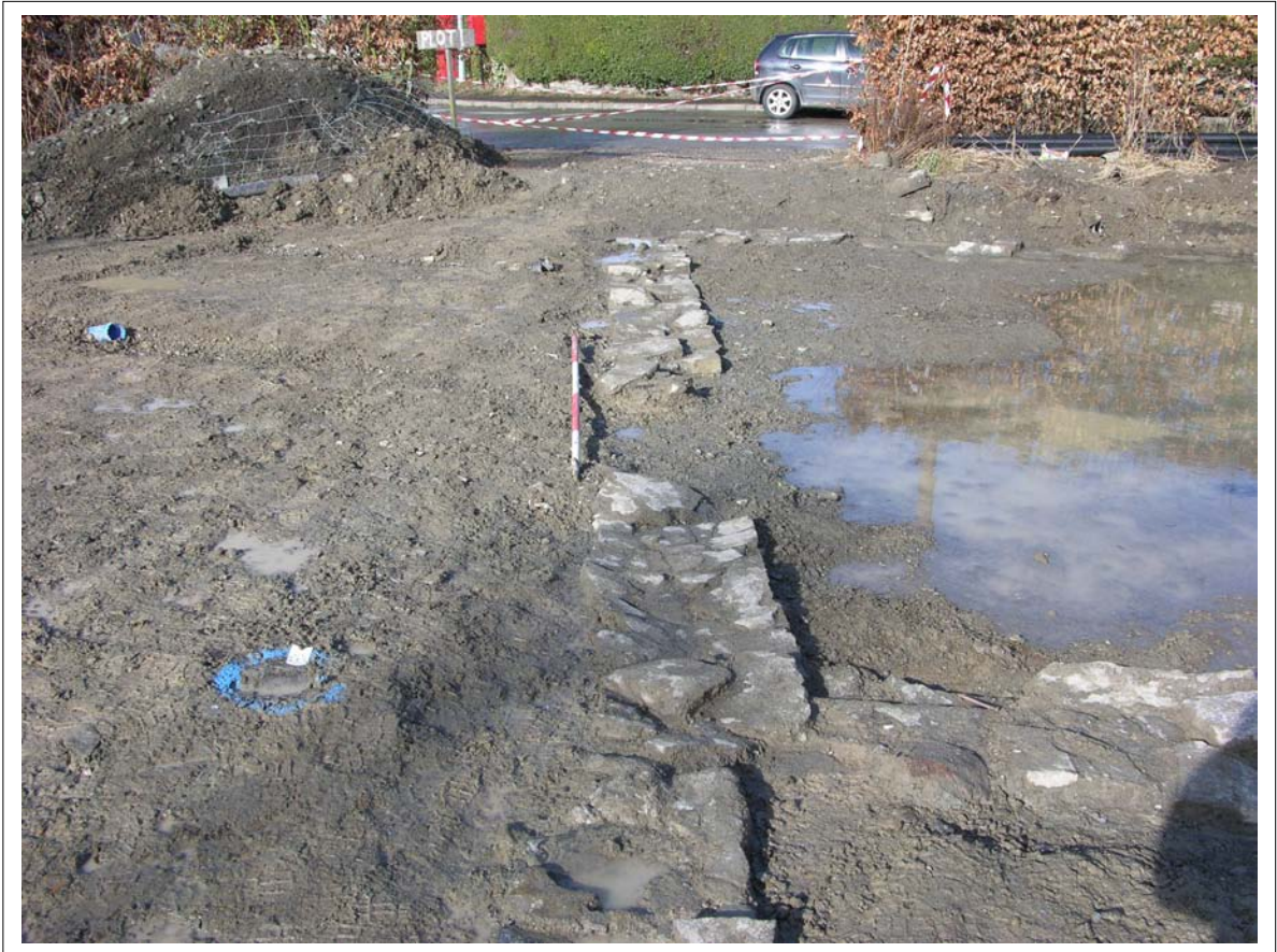
Plate 19: View of damaged doorway into southern end room of post medieval structure Scale 1x2m
