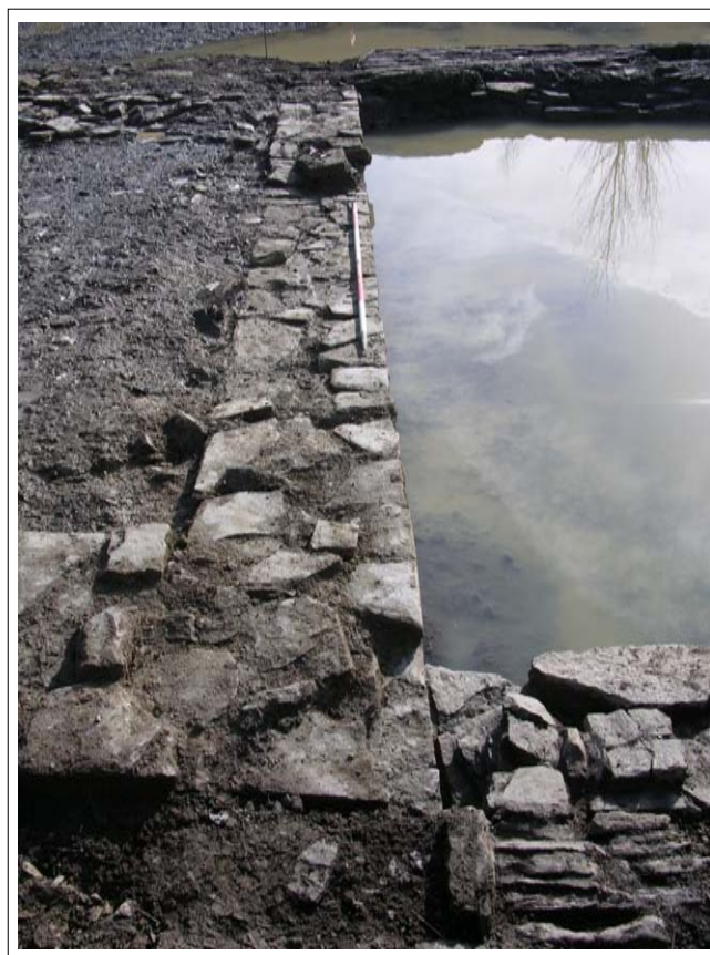
Plate 14: South wall of northern half of stone structure being clearly butted against (foreground) by later southern half of structure, Scale 1x2m
