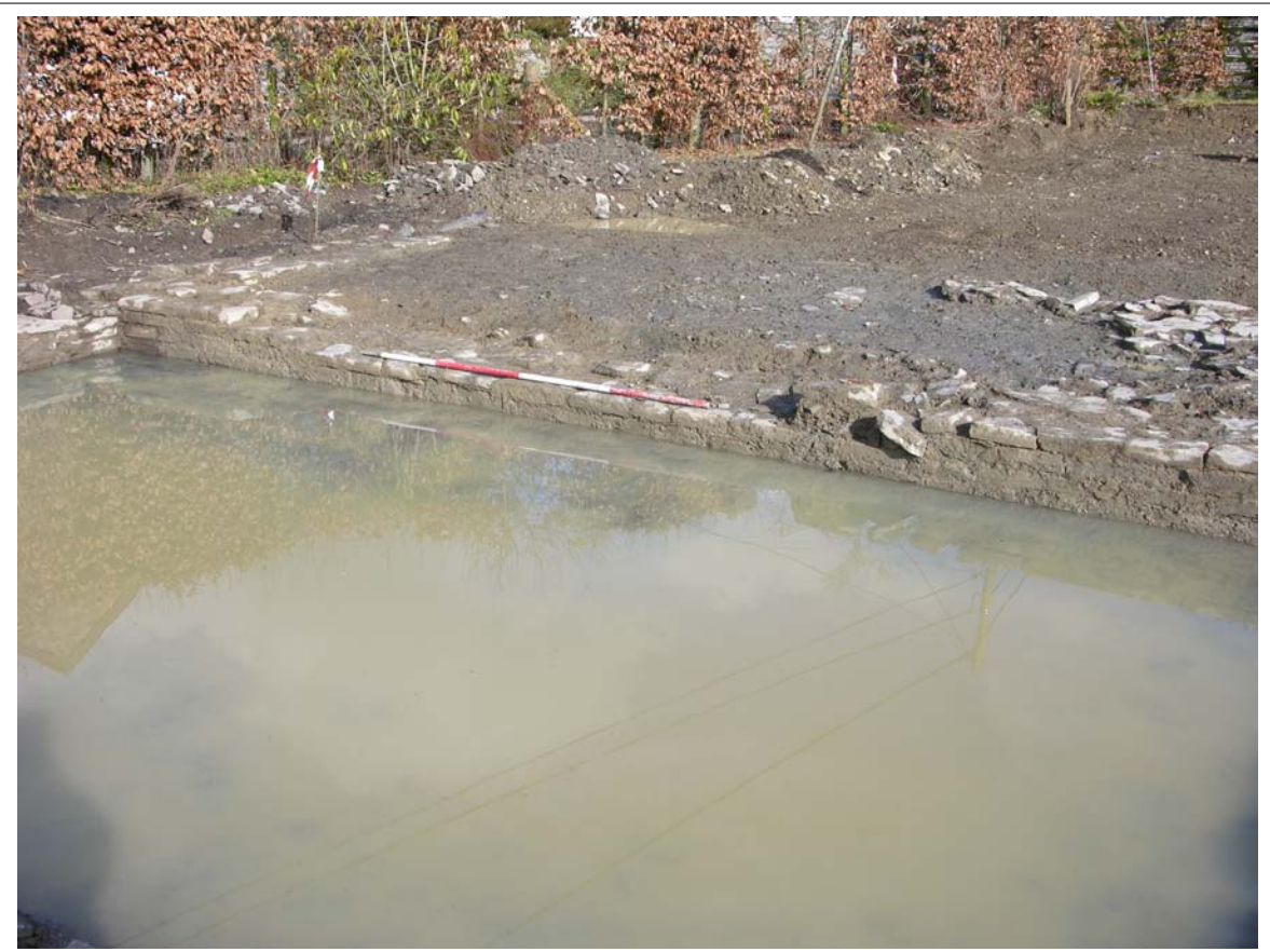
Plate 16: View of faced masonry on first phase (northern end) of post medieval structure, Scale 1x2m
