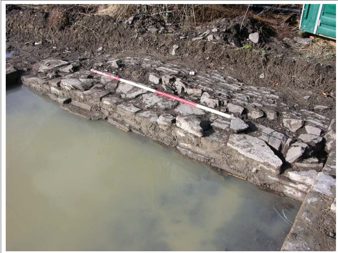
Plate 17: View of less well faced masonry on southern end of post medieval structure Scale 1x2m
