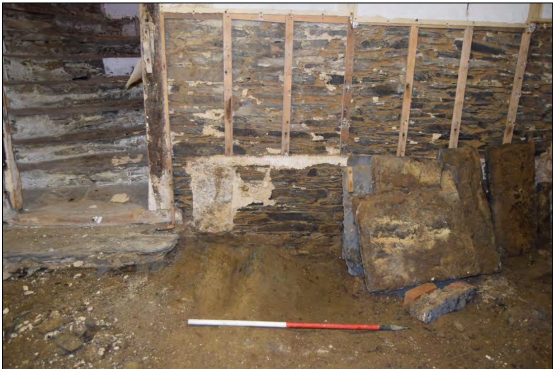
Plate 24: Basement, Test Pit 1 fully excavated, looking south-west, 1m scale.
