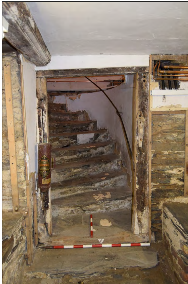
Plate 8: Basement stair, looking east south-west, 1m & 0.5m scale.
