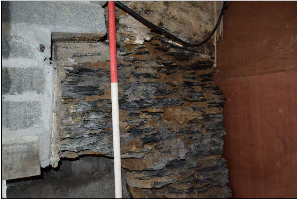
Plate 21: Basement, new doorway opening (south), looking south south-west, 2m scale.
