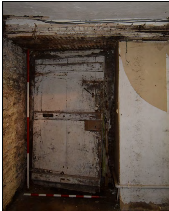
Plate 16: Basement door (external), looking south-west, 2m & 1m scale.
