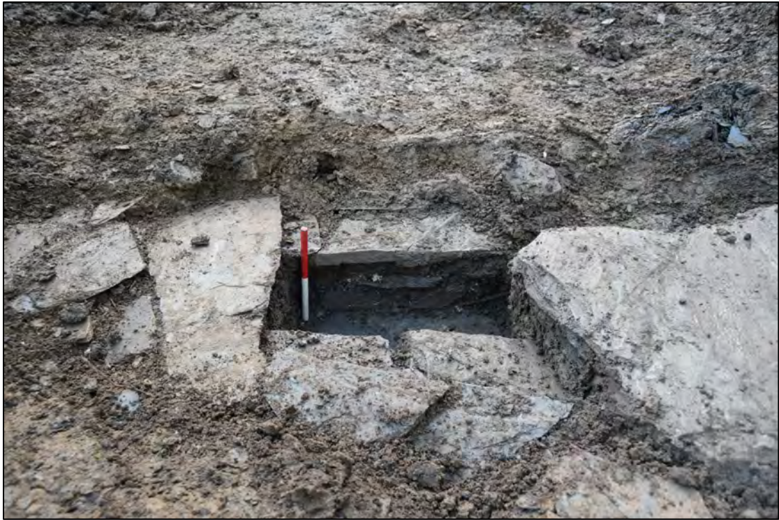
Plate 33: Watching Brief, Area 4, Box Culvert [4010]; (4006) & (4007) part removed, looking south, 0.5m scale.
