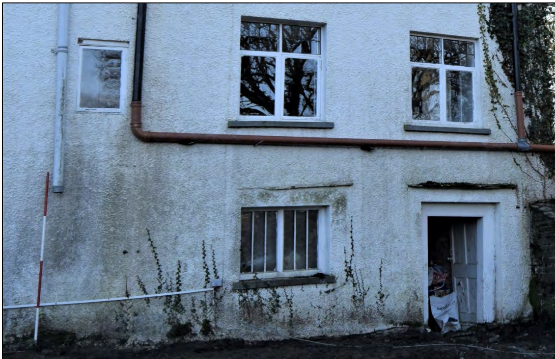
Plate 4: Basement door opening, looking east south-east, 2m scale .
