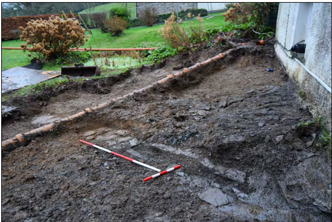
Plate 32: Watching Brief, Area 4, Box Culvert [4010] and Ceramic Pipe [4011], looking south-east, 2m & 0.5m scale.
