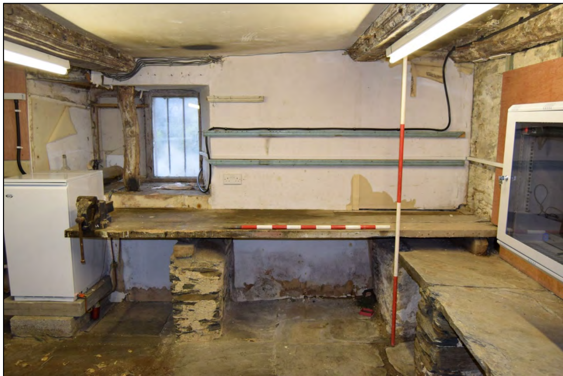
Plate 14: Basement Utility Room, looking north-east, 2m & 1m scale.
