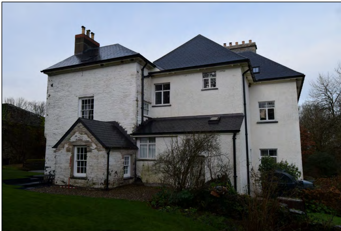
Plate 2: Glandovan Mansion, SW Facing Elevation looking north north-east, 2m scale.
