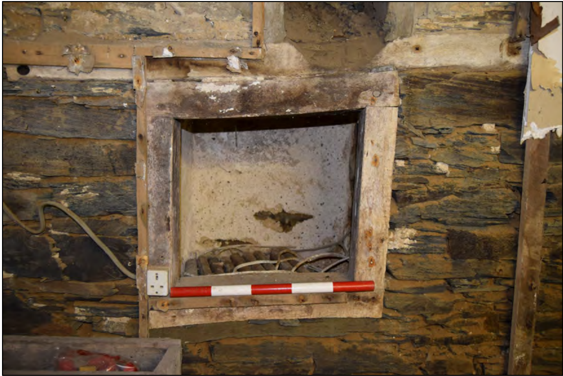
Plate 11: Basement, Utility Room niche, looking north west, 0.5m scale.
