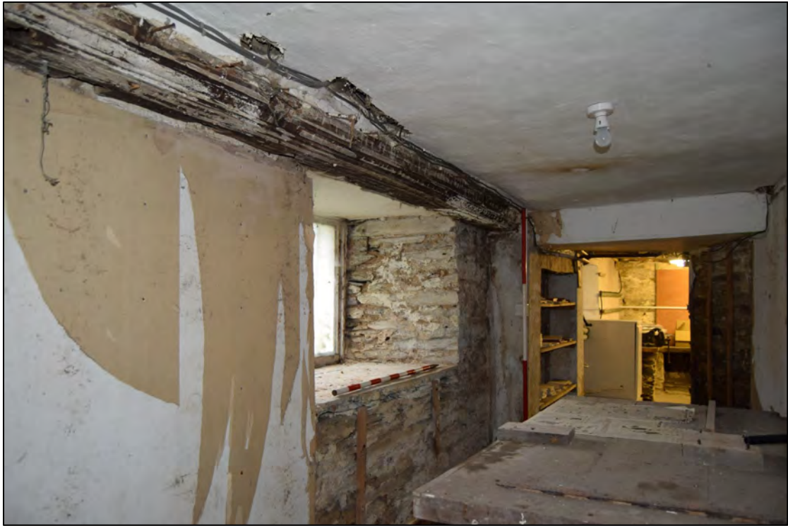
Plate 17: Basement corridor, looking south-east, 2m & 1m scale.
