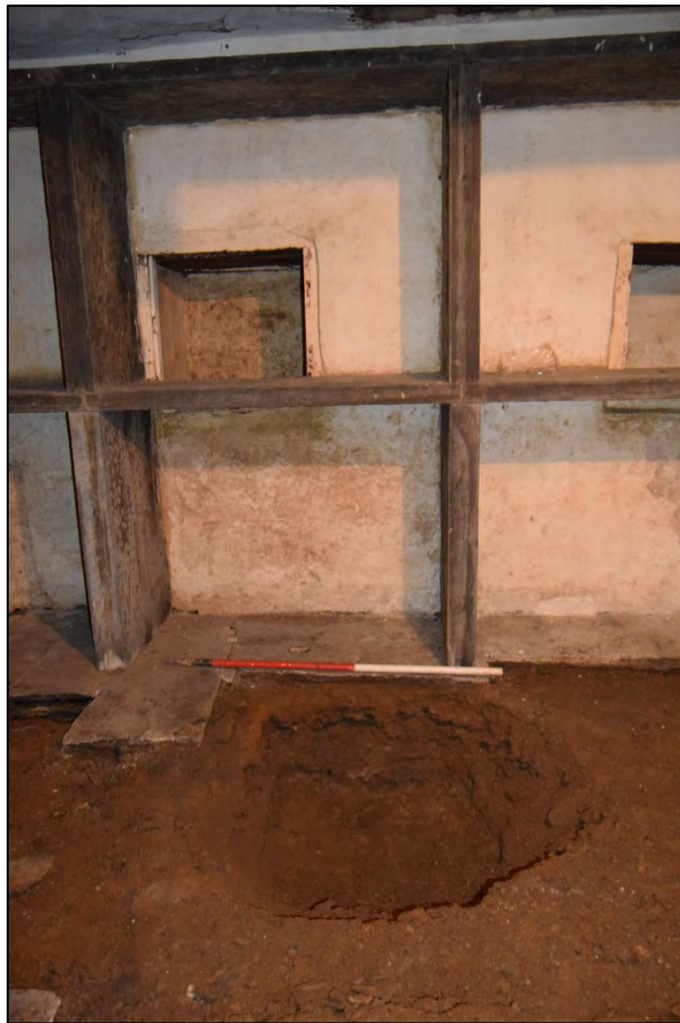
Plate 28: Basement, Test Pit 3 fully excavated, looking north-east, 1m scale.
