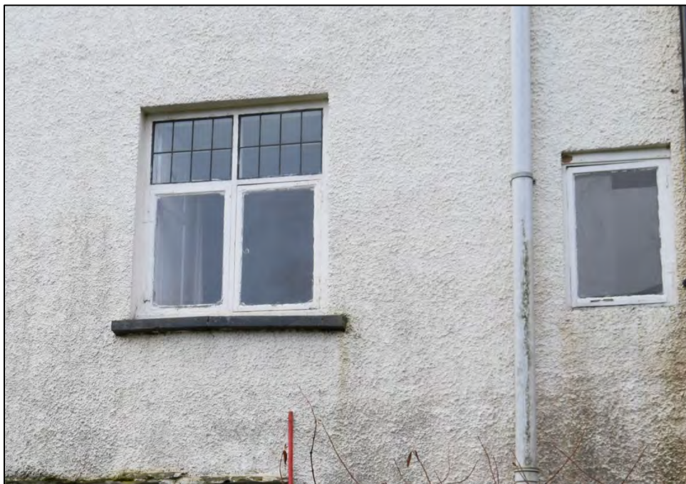
Plate 6: NE Elevation, First floor windows, looking east north-east, 2m scale.
