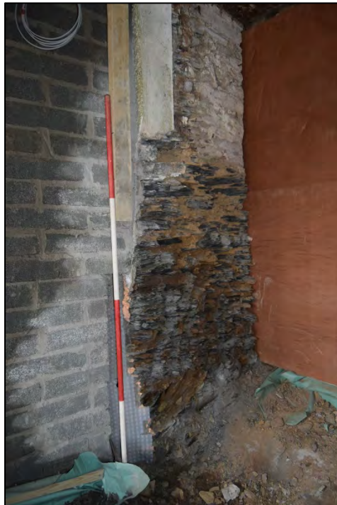
Plate 20: Basement, new doorway opening (north), looking south south-west, 2m scale.
