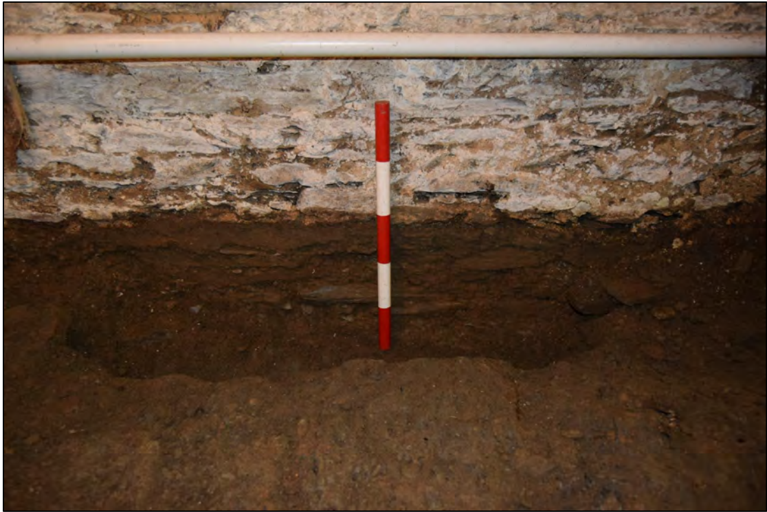
Plate 27: Basement, Test Pit 2 detail of SW facing section, looking north-east, 0.5m scale.
