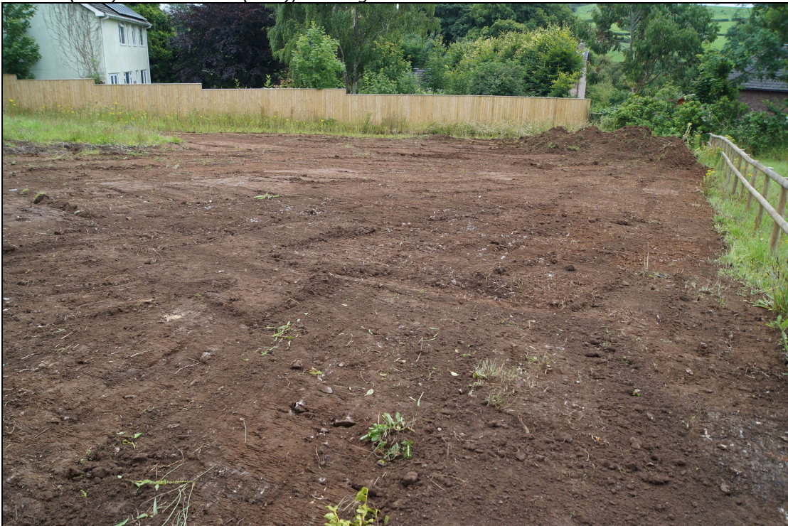
Plate 6: STF2020_106. A view of the development site after the initial scrape to remove vegetation, looking south-southwest.
