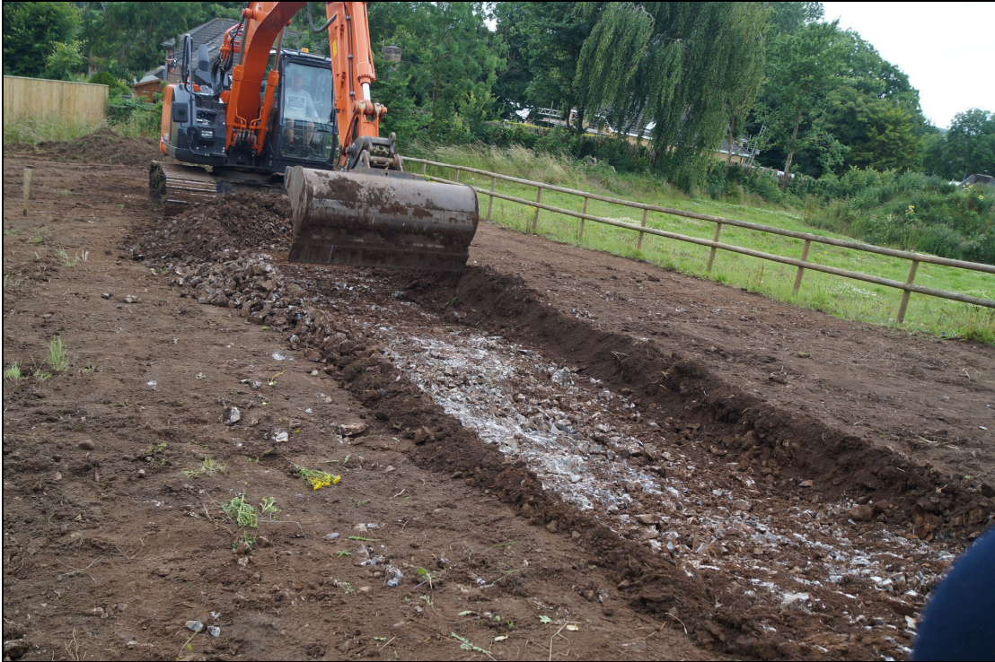
Plate 7: STF2020_107. Topsoil (001) and subsoil (002) being removed to reveal bedrock (003), looking southwest.
