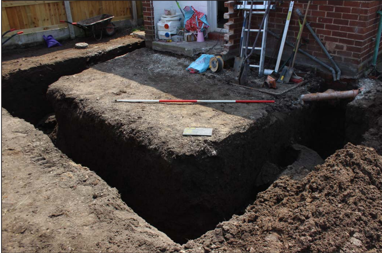
Plate 10: Completed excavation of footings - from the north - 2.00m scale
