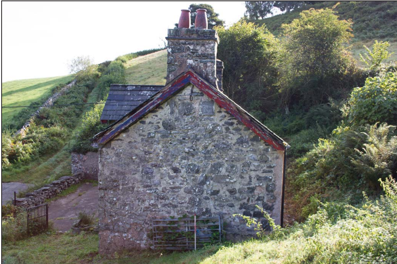
Plate 04: External shot - western elevation of the Farmhouse, Tan Y Bodran, Bodran Road, Llanfairtalhaiarn, Conwy - from the west - scale 1m
