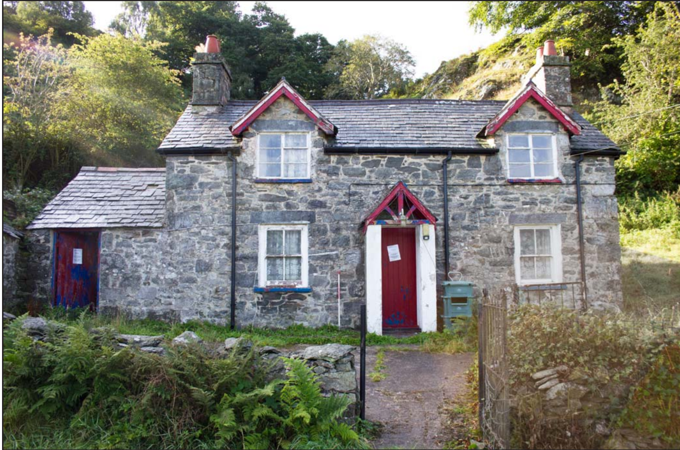
Plate 02: External shot - northern elevation of the Farmhouse, Tan Y Bodran, Bodran Road, Llanfairtalhaiarn, Conwy - from the north - scale 1m
