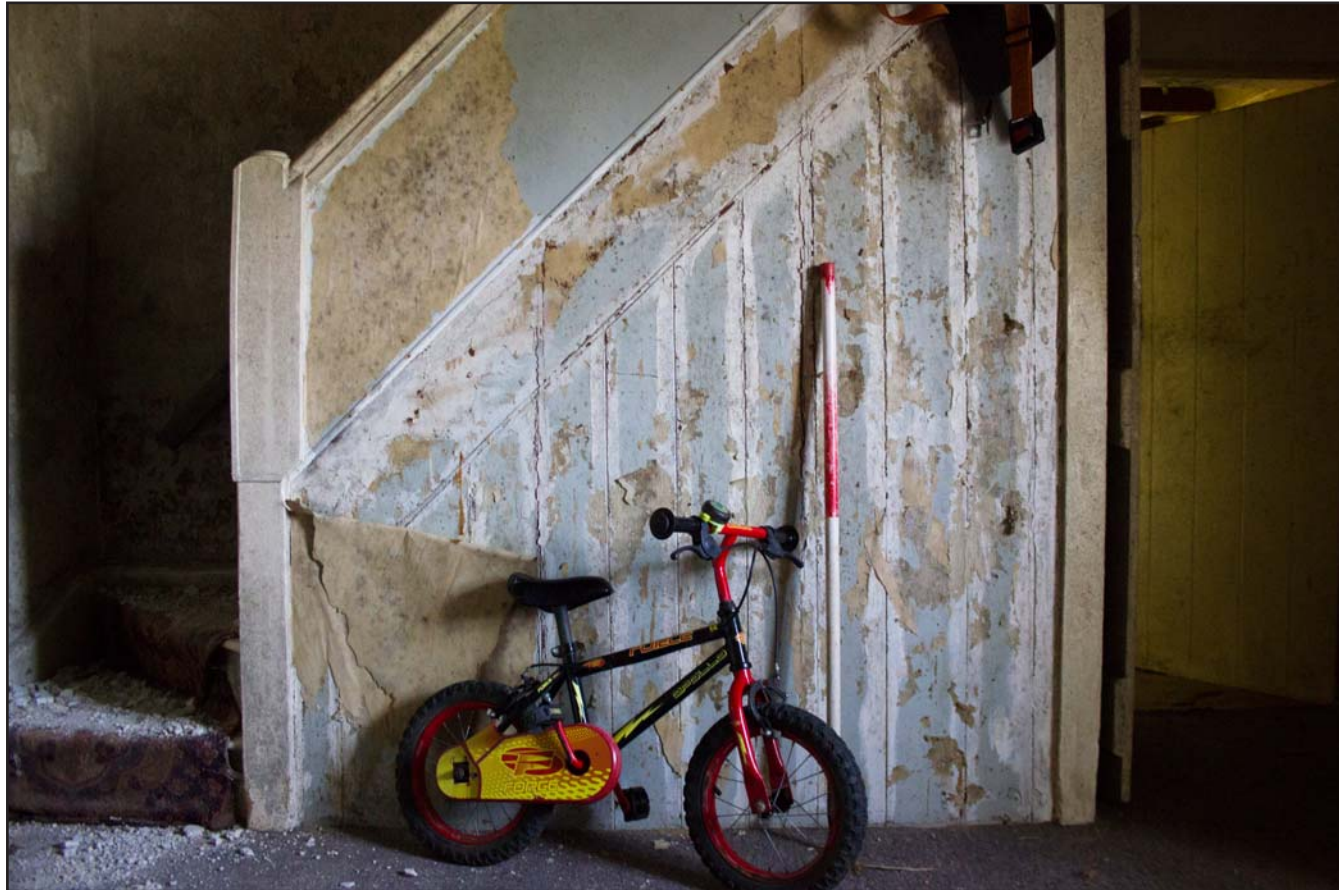
Plate 27: Internal shot - Staircase within the Lounge , Farmhouse building at Tan Y Bodran, Bodran Road, Llanfairtalhaiarn, Conwy - from the northeast - scale 1m
