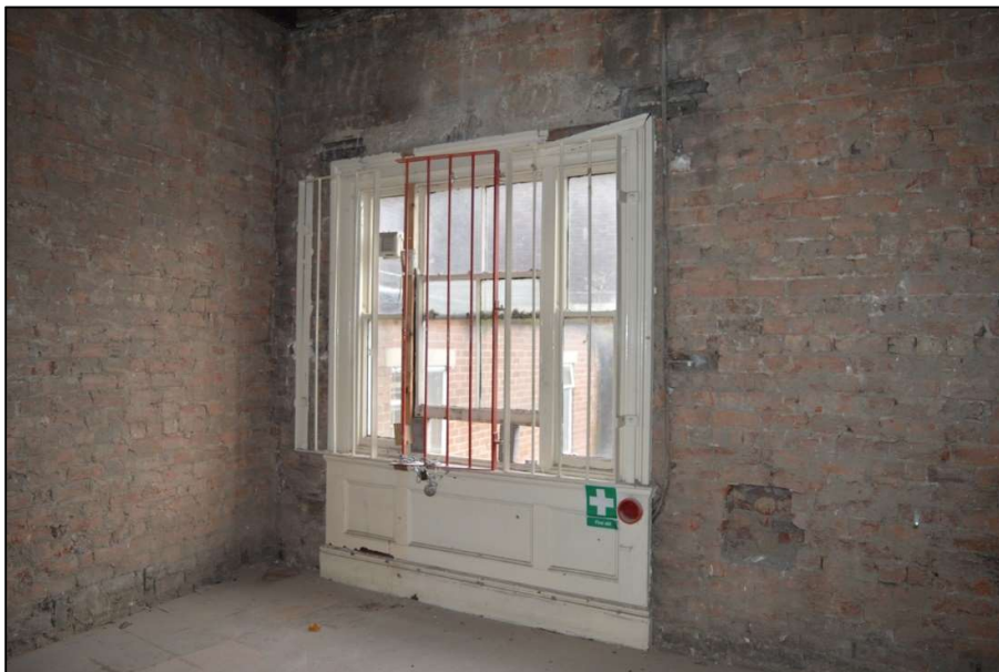
Fig 64: Window in Room 8 on the first floor (CPAT 4853-0063)
