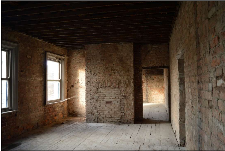
Fig 8: General view of Room 2 on second floor (CPAT 4853-0007)
