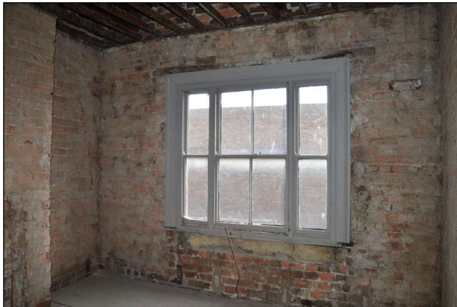
Fig 58: Window in Room 1 on the second floor (CPAT 4853-0057)
