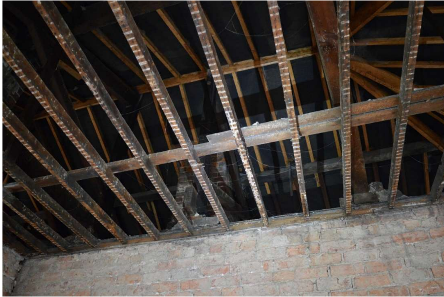
Fig 18: Ceiling timbers with Trusses 1-3 behind in roof space (CPAT 4853-0017)
