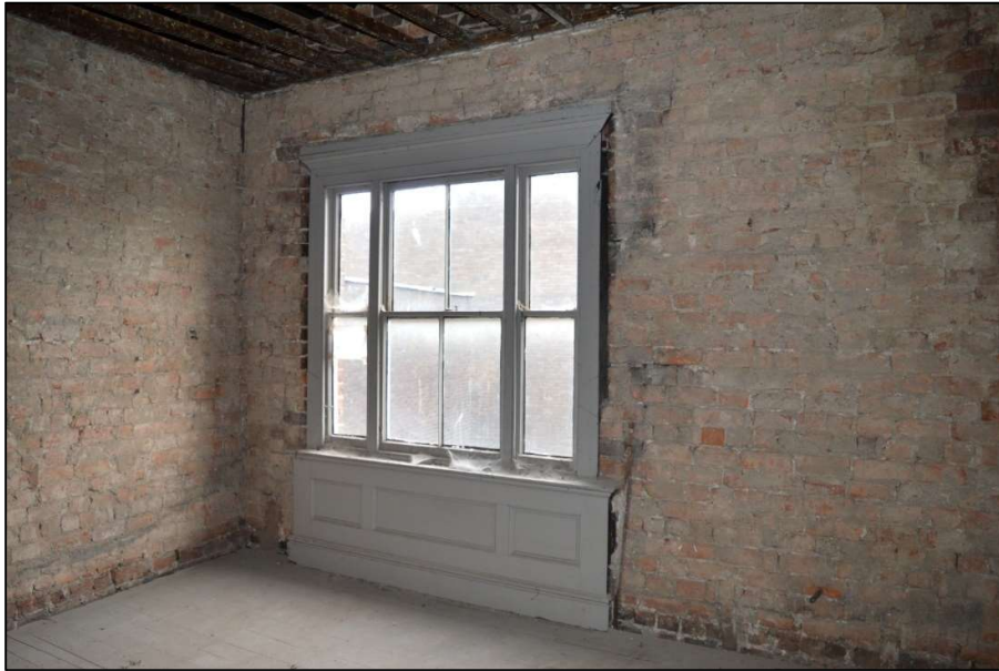
Fig 61: Window in Room 4 on the second floor (CPAT 4853-0060)
