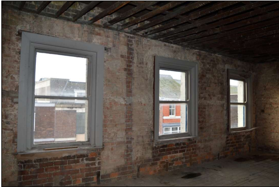
Fig 59: Windows in Room 2 on the second floor (CPAT 4853-0058)
