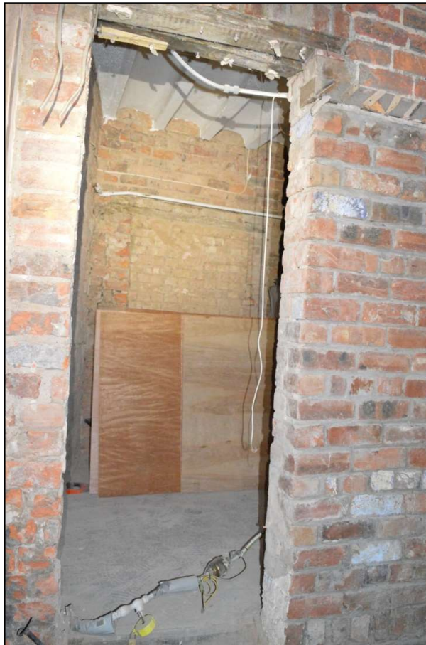
Fig 56: Doorway to rear of original building where the brick seems to be re-used. The blocked doorway in the wall behind might indicate there was an earlier yard wall to the rear of the original building (CPAT 4853-0055)
