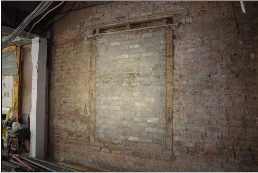
Fig 47: Blocked window in original west wall of ground floor (CPAT 4853-0046)
