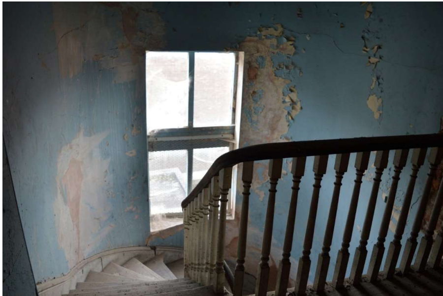
Fig 3: Top of east stair with window to rear (CPAT 4853-0020)
