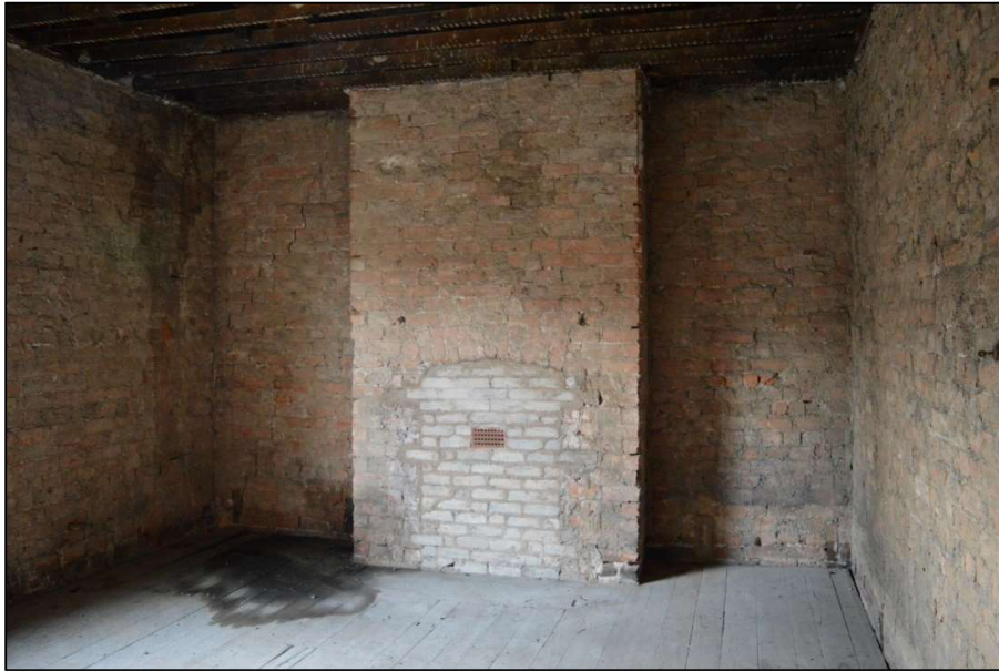
Fig 14: Blocked fireplace with hearth stone in Room 4 on second floor (CPAT 4853-0013)
