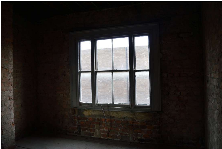
Fig 5: Window in Room 1 on second floor (CPAT 4853-0004)
