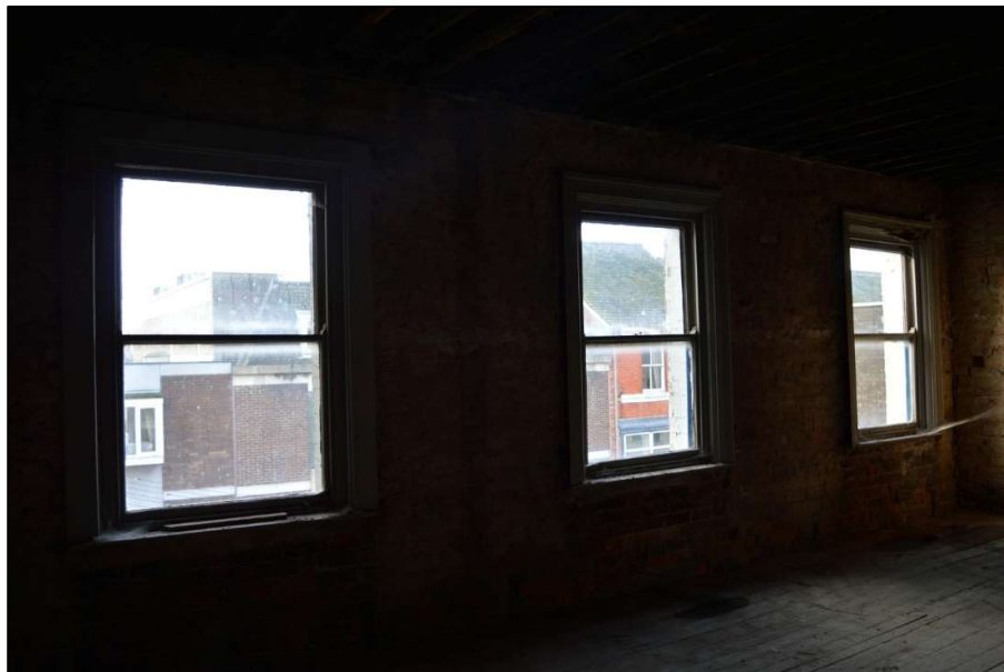
Fig 7: Windows in Room 2 on second floor (CPAT 4853-0006)
