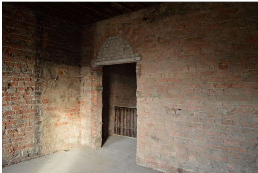
Fig 13: Partly blocked arched doorway in Room 3 on second floor (CPAT 4853-0012)
