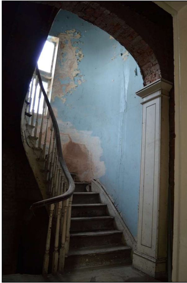
Fig 36: East stair looking up through the supporting arch from the first floor landing (CPAT 4853-0035)
