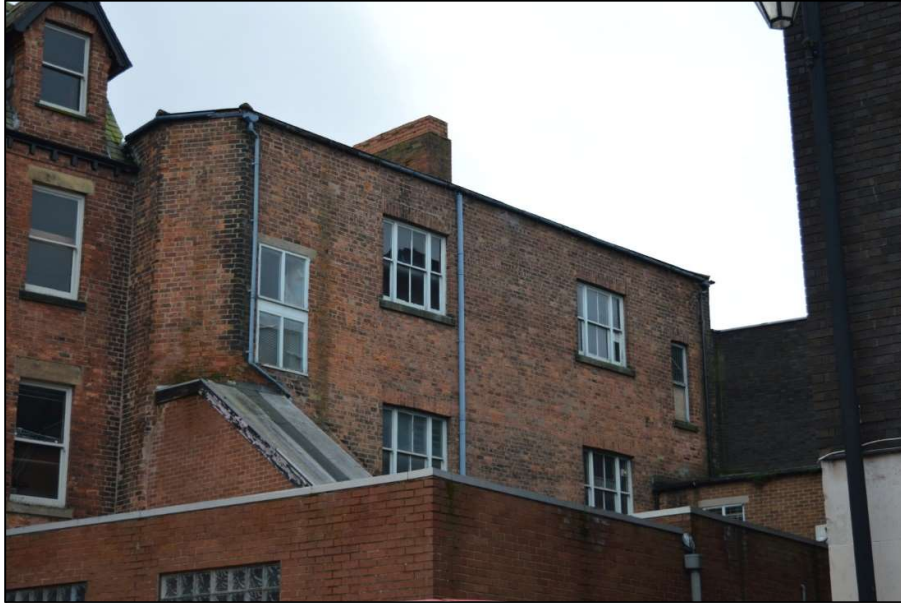
Fig 75: The rear view of the first and second floors of the original building from Argyle Street. The sloping structure to lower left is where modern steps down to the rear of the building were inserted into the east stair at first floor level (CPAT 4853-0074)
