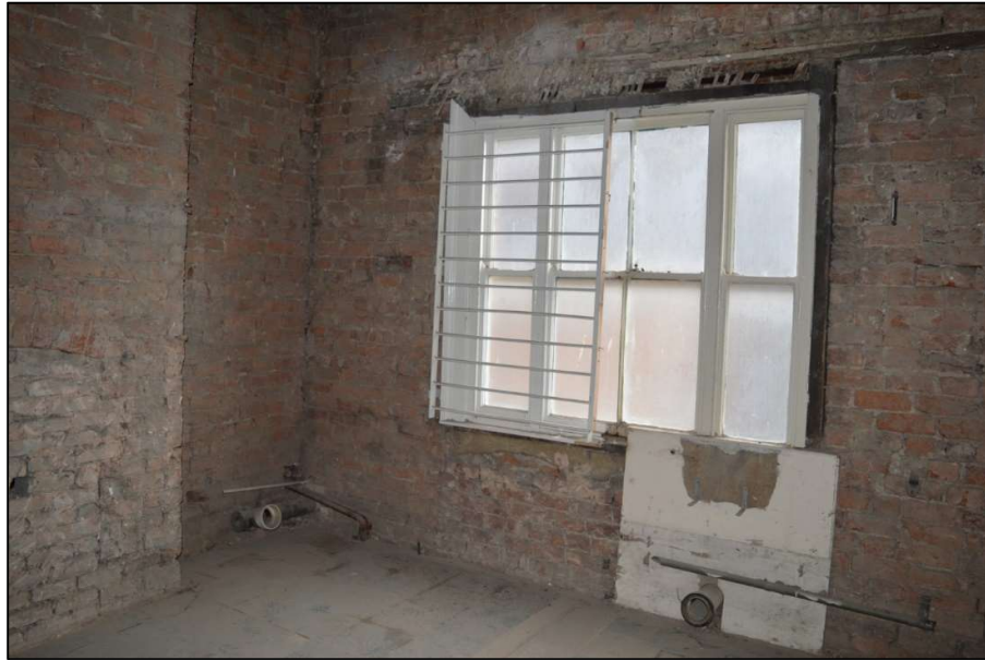
Fig 65: Window in Room 5 on the first floor (CPAT 4853-0064)
