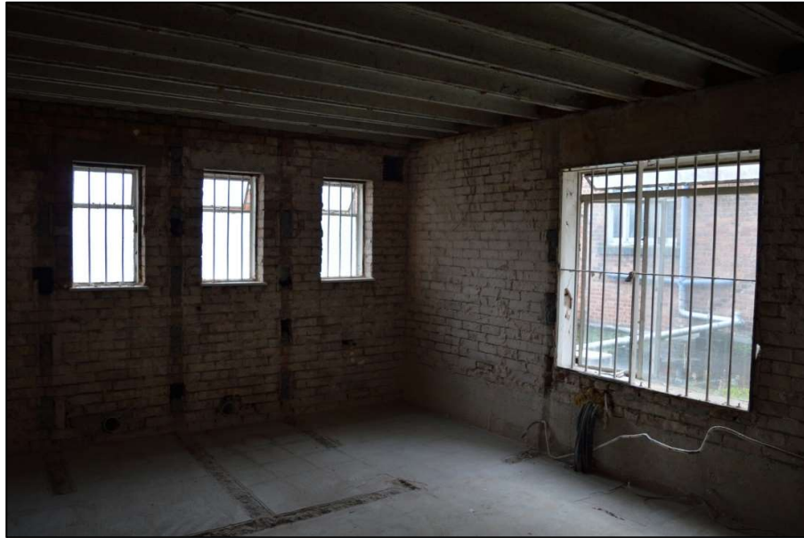
Fig 43: Rear part of modern first floor extension (CPAT 4853-0042)
