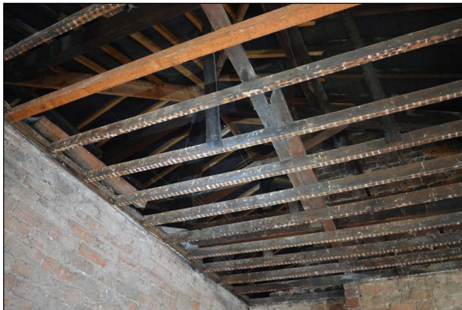
Fig 17: Ceiling timbers with Truss 4 behind in roof space (CPAT 4853-0016)
