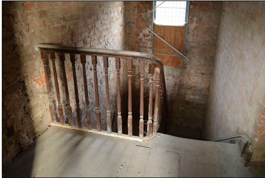
Fig 16: Top of western stair on second floor (CPAT 4853-0015)
