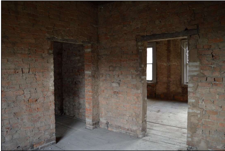
Fig 6: Doorways in Room 1 on second floor (CPAT 4853-0005)
