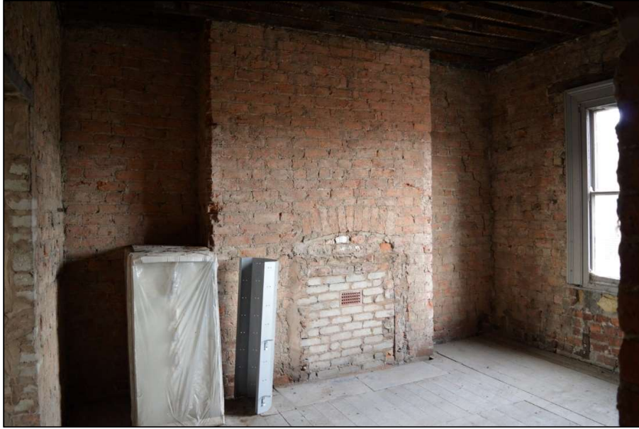
Fig 4: Blocked fireplace with hearth stones in Room 1 on second floor (CPAT 4853-0003)
