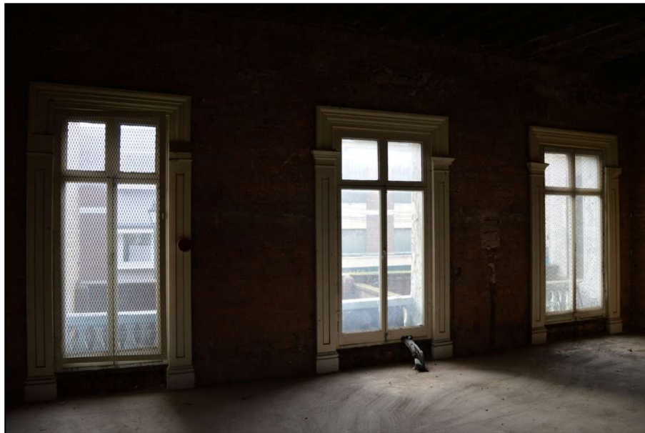
Fig 38: Windows in Room 6 on first floor. (CPAT 4853-0037)
