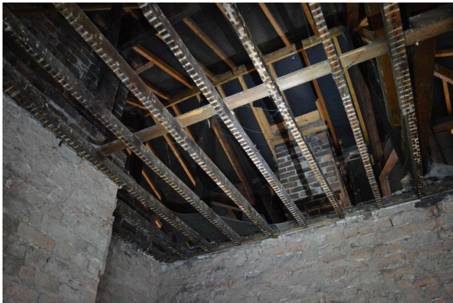
Fig 19: Ceiling timbers with Trusses 3 and 4 behind in roof space (CPAT 4853-0018)
