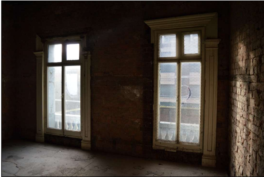
Fig 24: Windows in Room 7 on first floor (CPAT 4853-0023)
