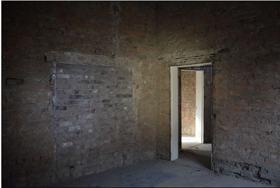
Fig 30: As 29. Blocked doorway in Room 8 on first floor. Also shows doorway to west stair (CPAT 4853-0029)
