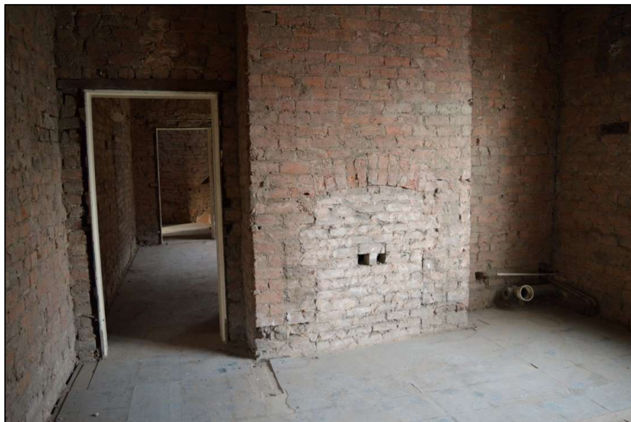
Fig 35: Blocked fireplace in Room 5 on first floor. Also shows route to west stair (CPAT 4853-0034)
