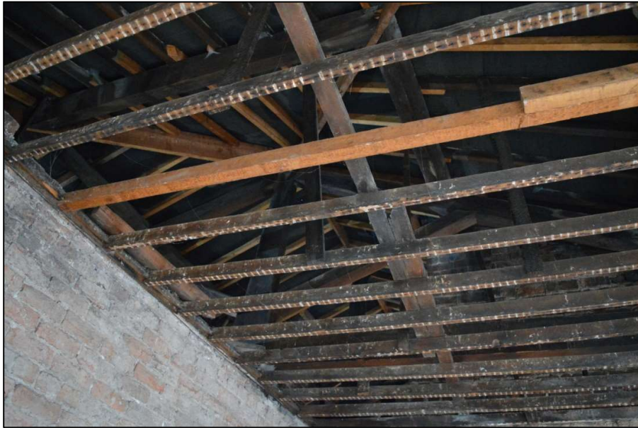
Fig 71: Ceiling timbers with Truss 4 behind in roof space (CPAT 4853-0070)
