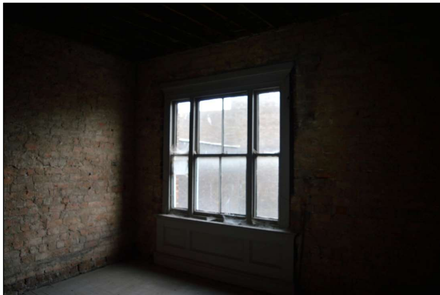
Fig 15: Window in Room 4 on second floor (CPAT 4853-0014)
