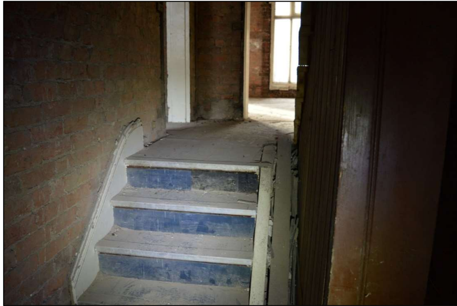
Fig 45: Stair up from modern first floor extension level to first floor of original building (CPAT 4853-0044)
