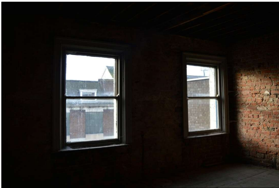
Fig 11: Windows in Room 3 on second floor (CPAT 4853-0010)
