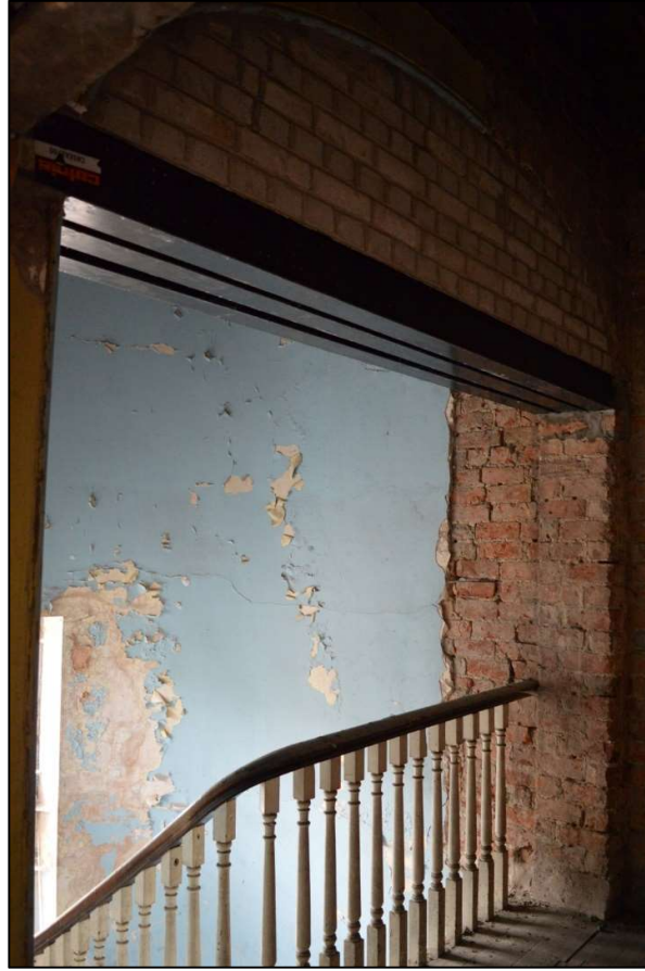
Fig 2: Arch (partly blocked) at top of east stair (CPAT 4853-0001)
