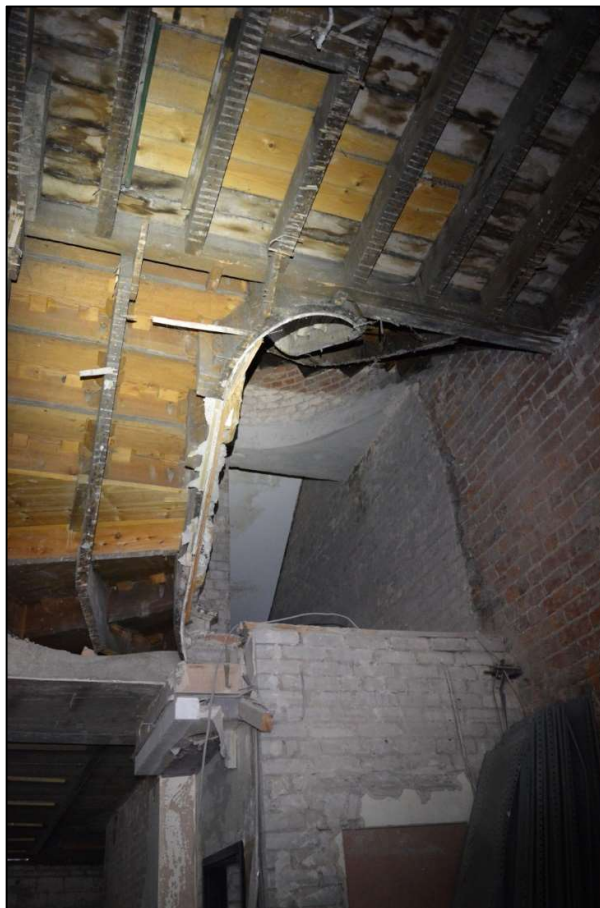
Fig 50: Bottom of the east stair, showing how it was truncated (CPAT 4853-0049)
