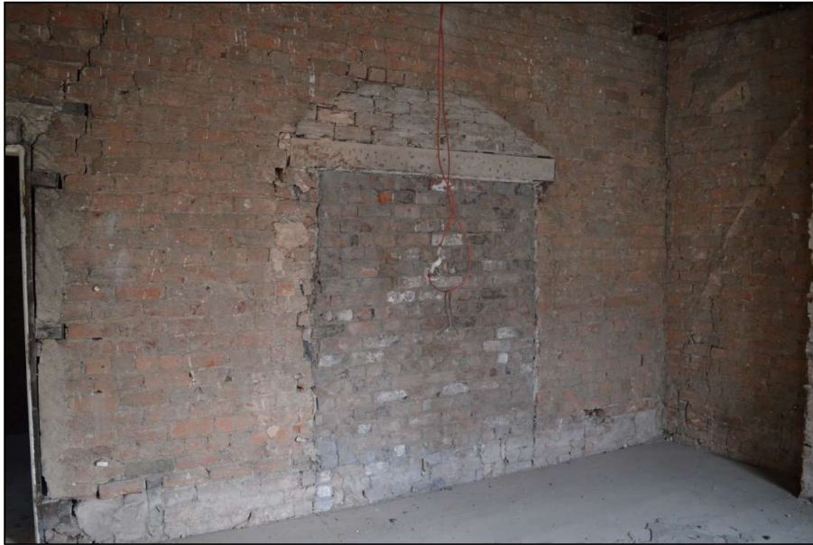
Fig 26: Blocked doorway in Room 7 on first floor. (CPAT 4853-0025)
