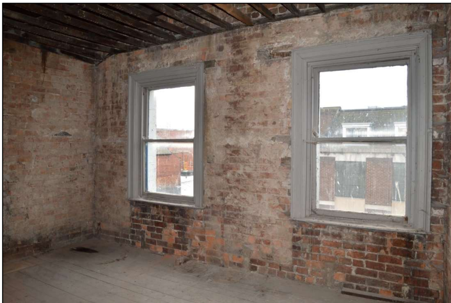
Fig 60: Windows in Room 3 on the second floor (CPAT 4853-0059)
