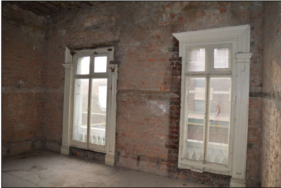
Fig 63: Windows in Room 7 on the first floor (CPAT 4853-0062)
