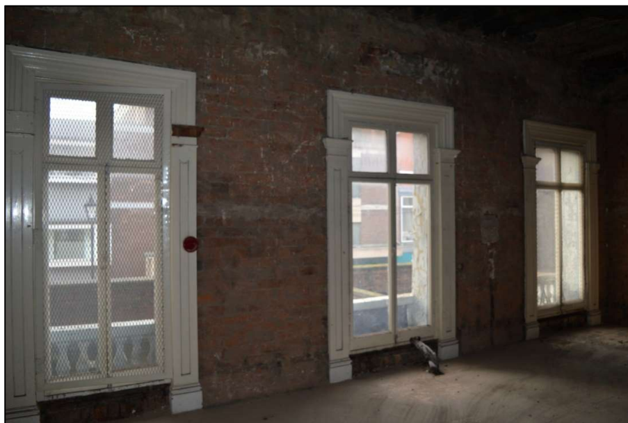
Fig 66: Windows in Room 6 on the first floor (CPAT 4853-0065)
