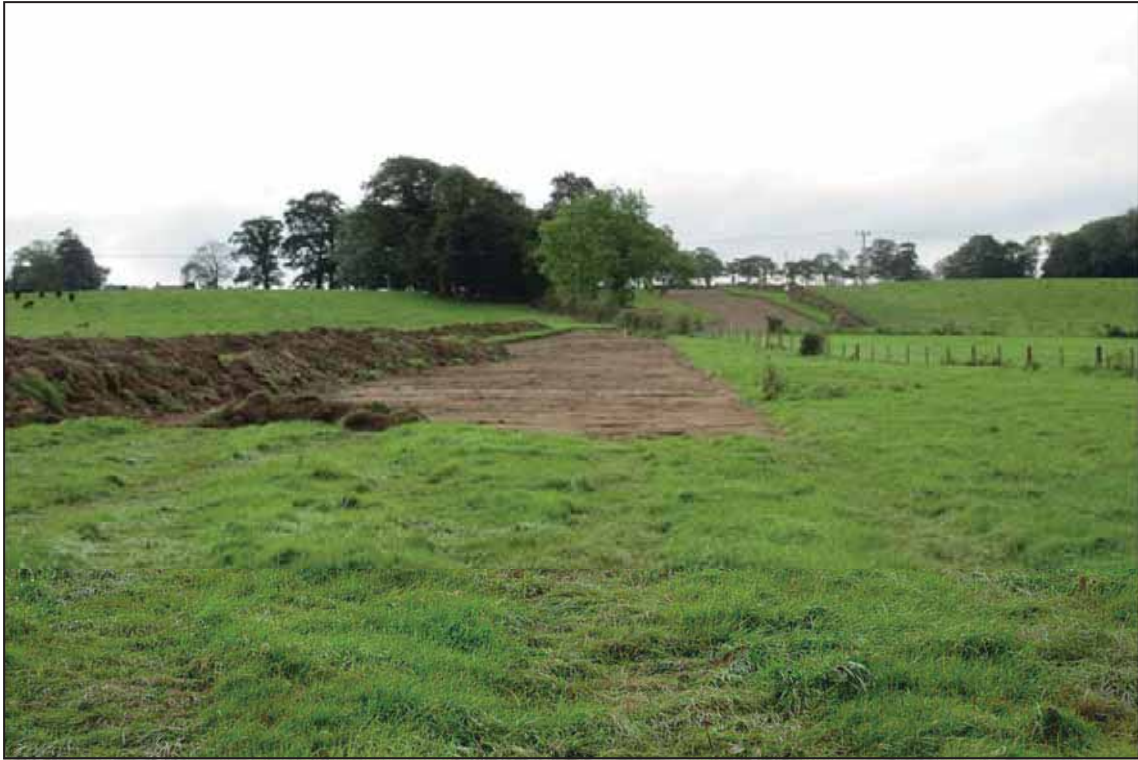
View of the pipeline easement, looking north
