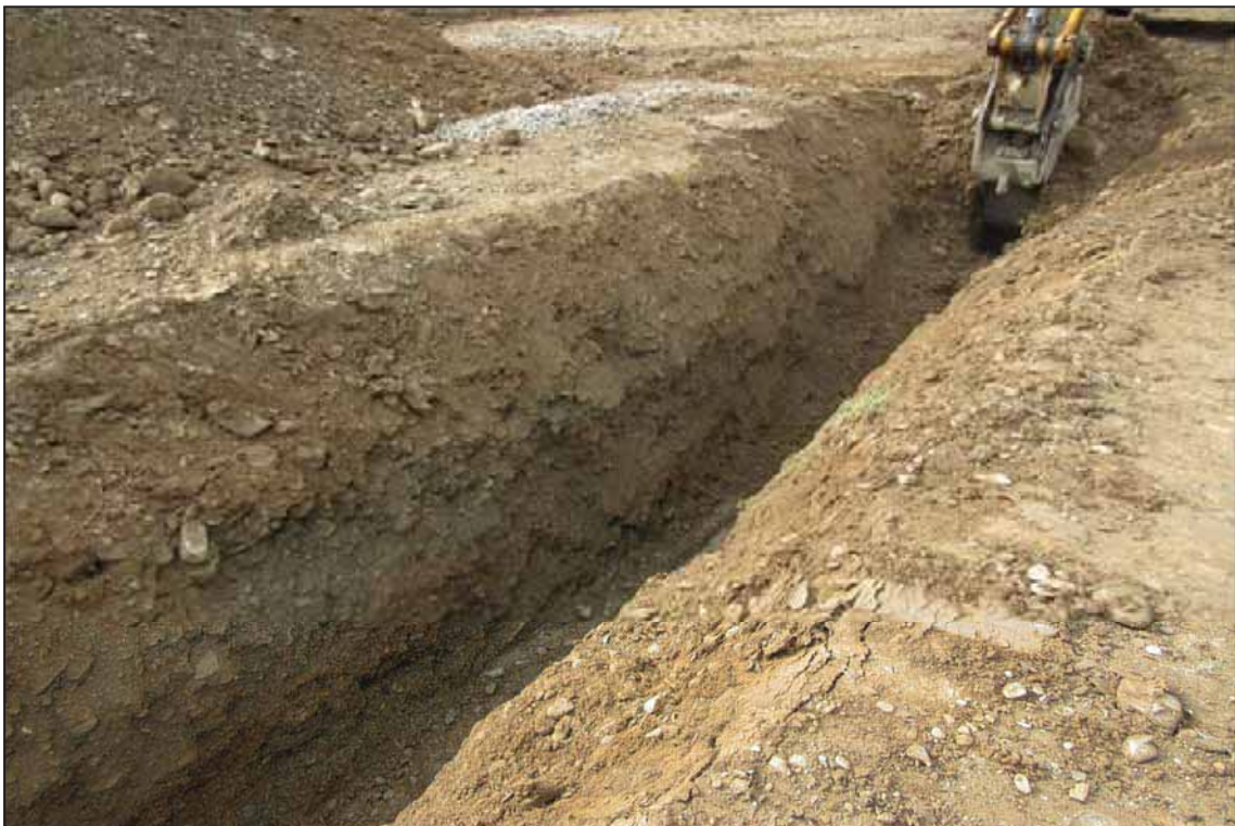
Representative section of pipe trench in northern area
