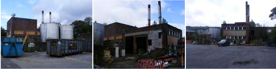
Storage tanks and associated building in the north-east corner of the site
