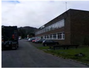
View looking west across southern elevation of the eastern factory
