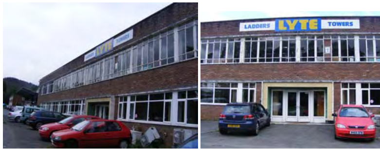
View of the 1940s southern elevation of the western factory
