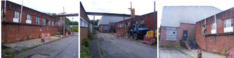
Views of the western elevation of the building in-between the two main factories – located to the rear of the late 1990s addition
