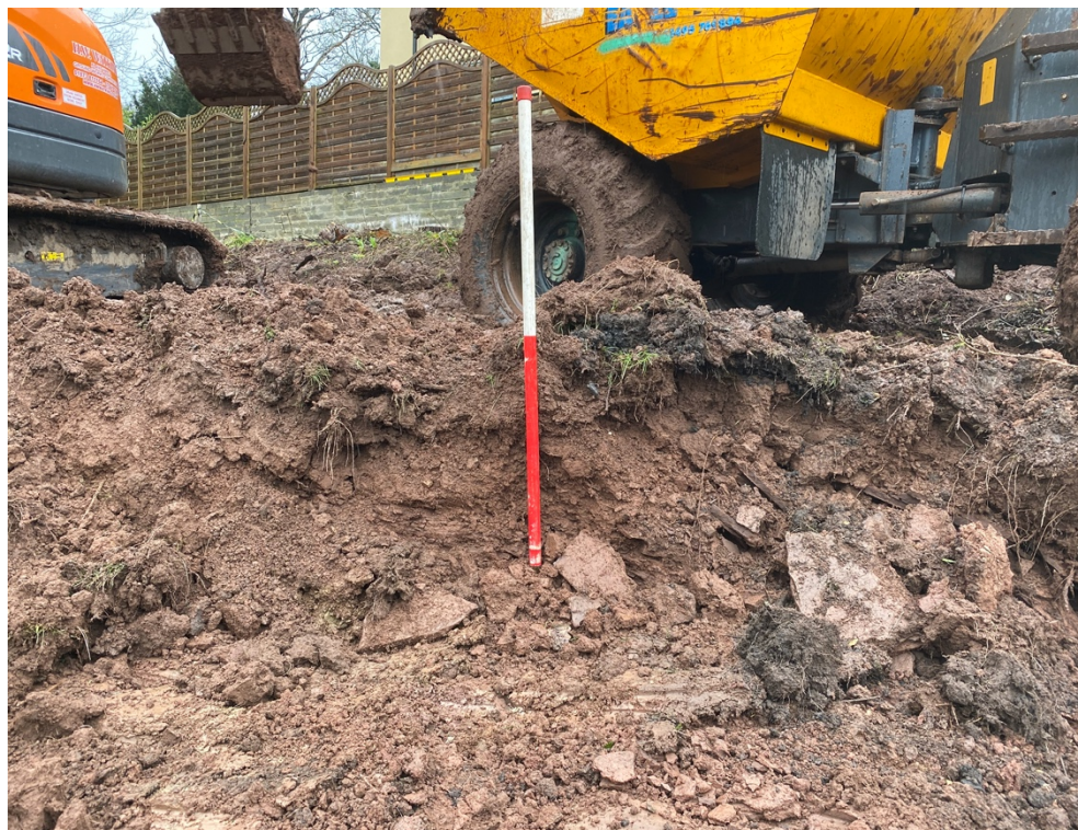
Plate 2. Southeast facing section of topsoil (001) (during topsoil stripping)
