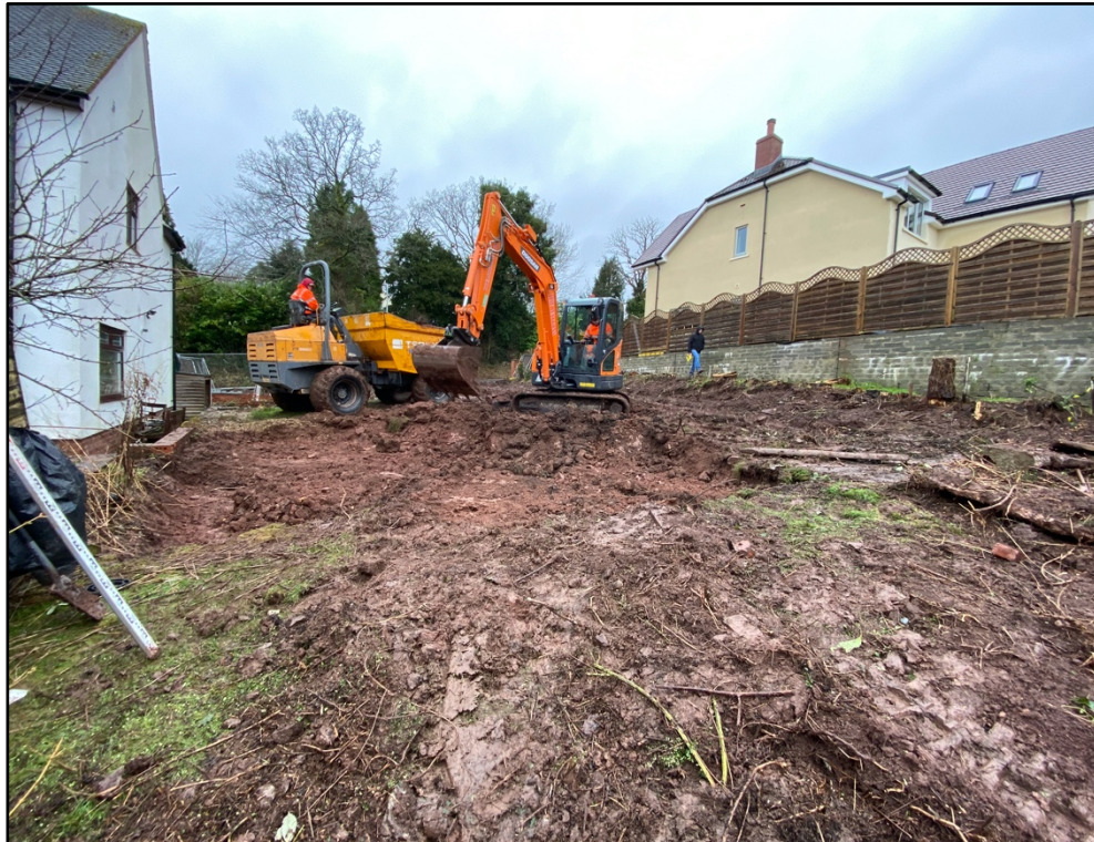
Plate 1. Topsoil stripping in progress (view northwest)
