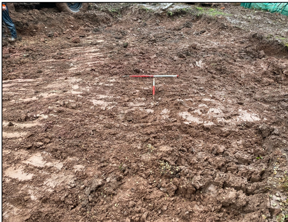
Plate 4. View of development area after topsoil stripping (view northwest)
