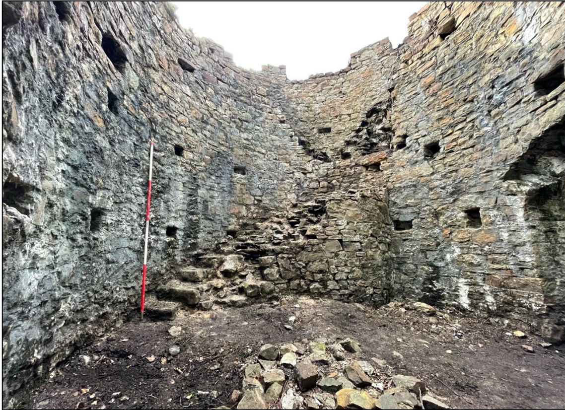
Plate 19 – E facing internal elevation of Ivy Tower showing Phase II inserted spiral staircase, internal putlog holes and two sets of joist sockets. Scale 2m.
