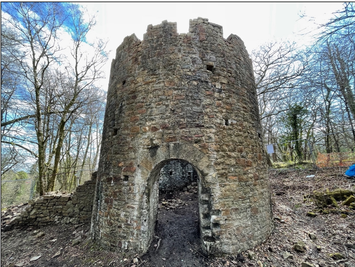
Plate 14 – N facing elevation of Ivy Tower showing inserted Phase II folly door, external putlog holes and remains of Phase I Flue.
