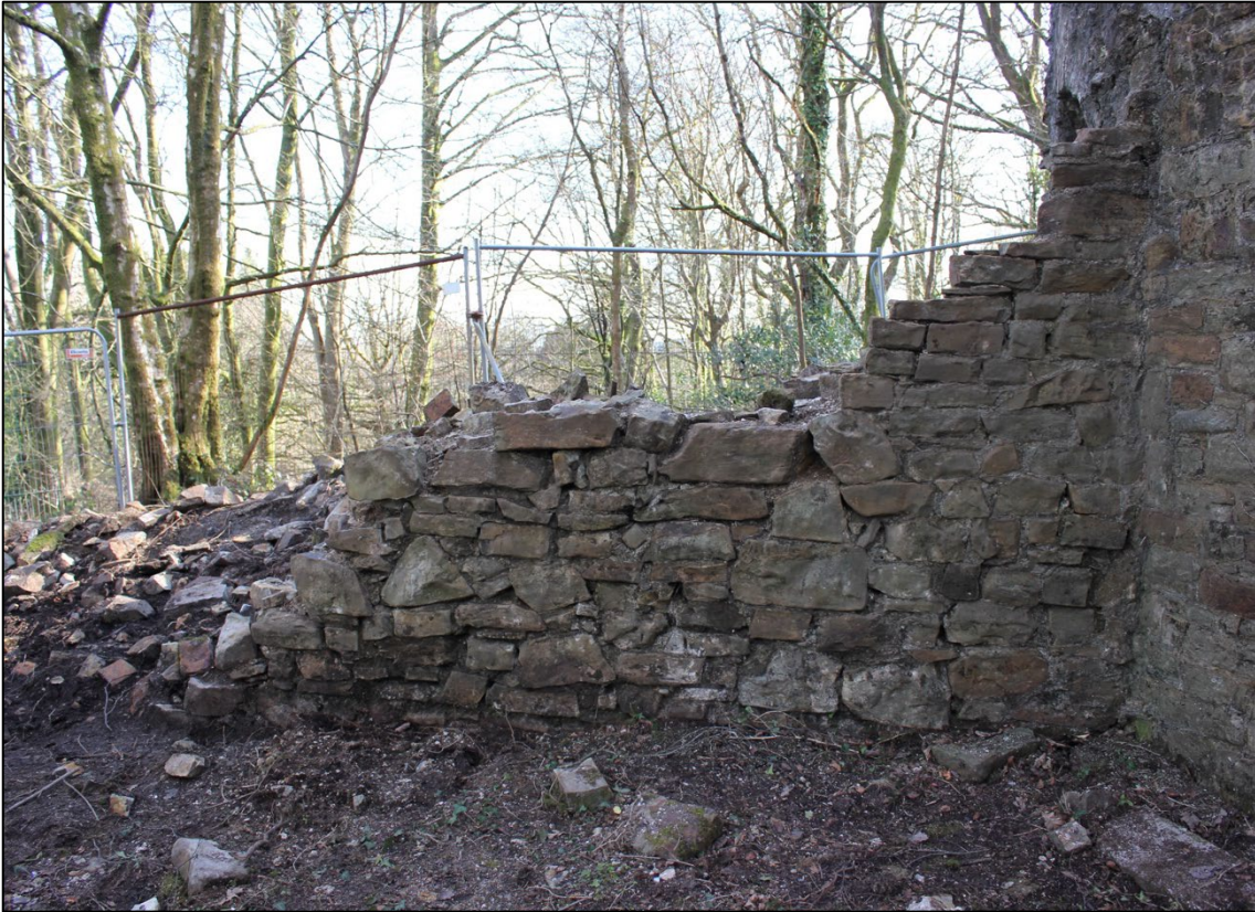
Plate 11 – NNE facing wall of the Phase I Flue.
