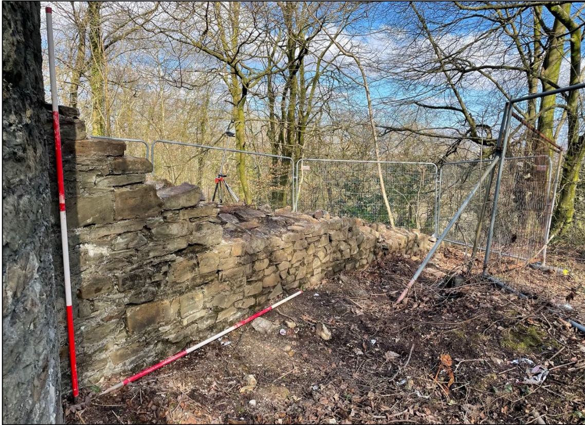
Plate 9 – SSE facing wall of the Phase I Flue. Scale 2m.
