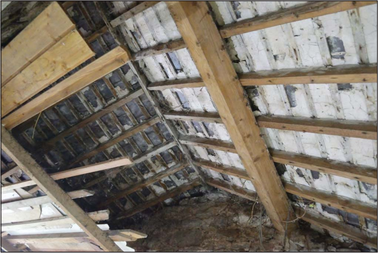
Plate 21: Inside roof of garage, from the east (archive reference: G2776_121)
