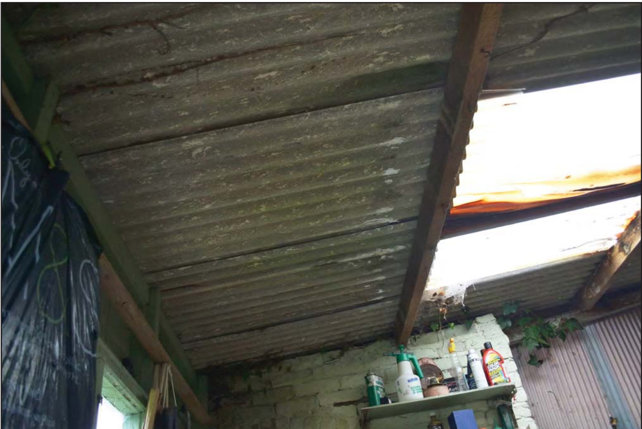
Plate 32: Inside of shed roof (archive reference: G2776_057)
