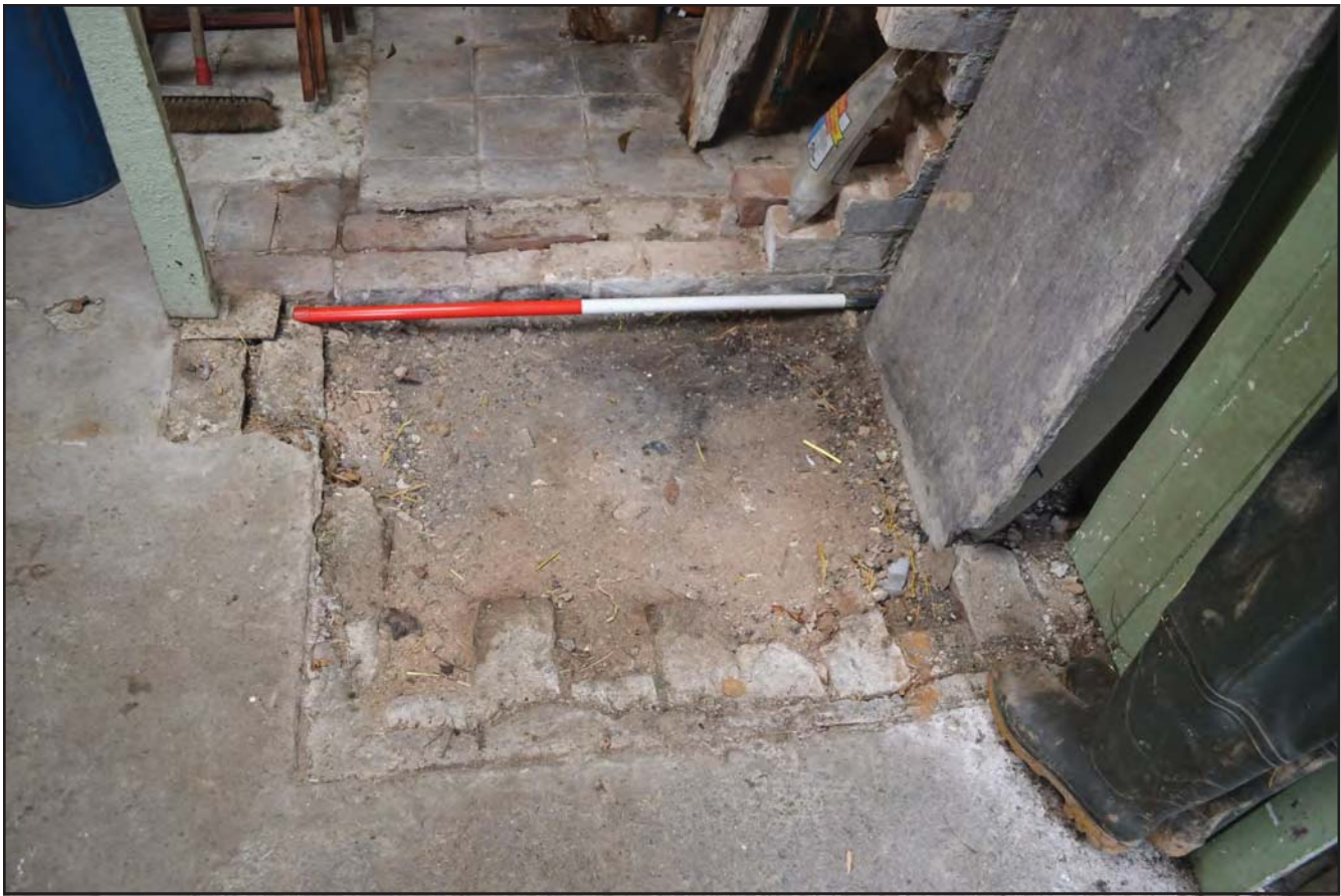
Plate 29: Remains of brick structure in the floor next to outside toilet 2, from the north-west (archive reference: G2776_052)
