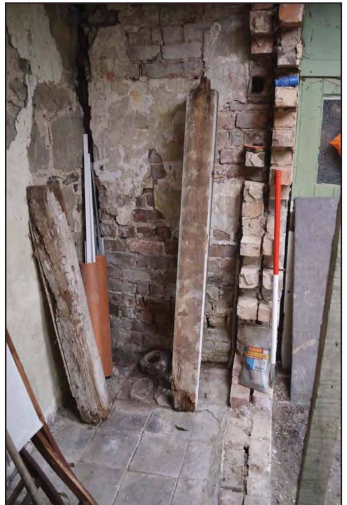
Plate 28: Partially demolished outside toilet 2, from the north-west (archive reference: G2776_048)
