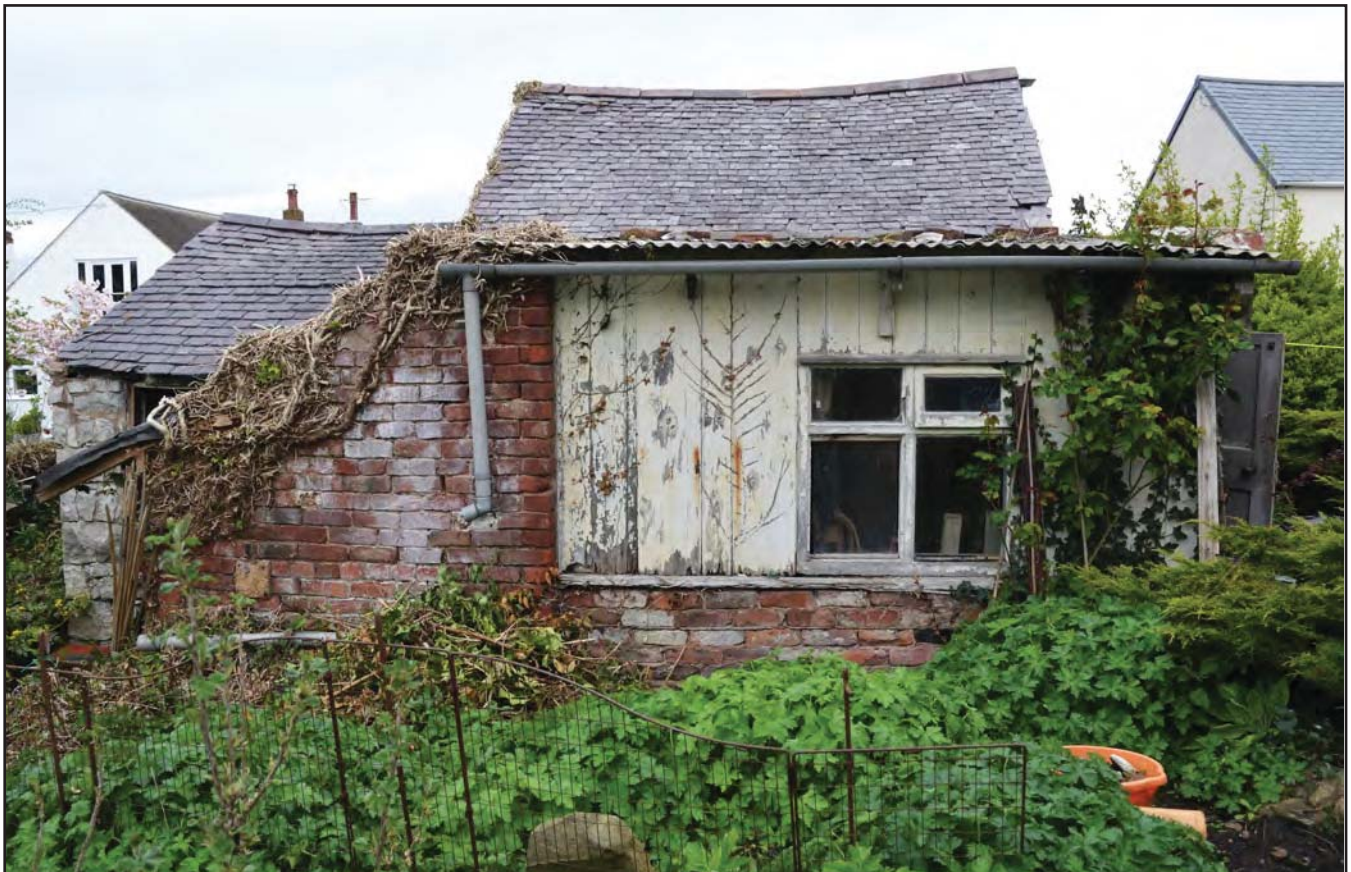
Plate 30: South-western elevation of outside toilet 1 and shed (archive reference: G2776_027)
