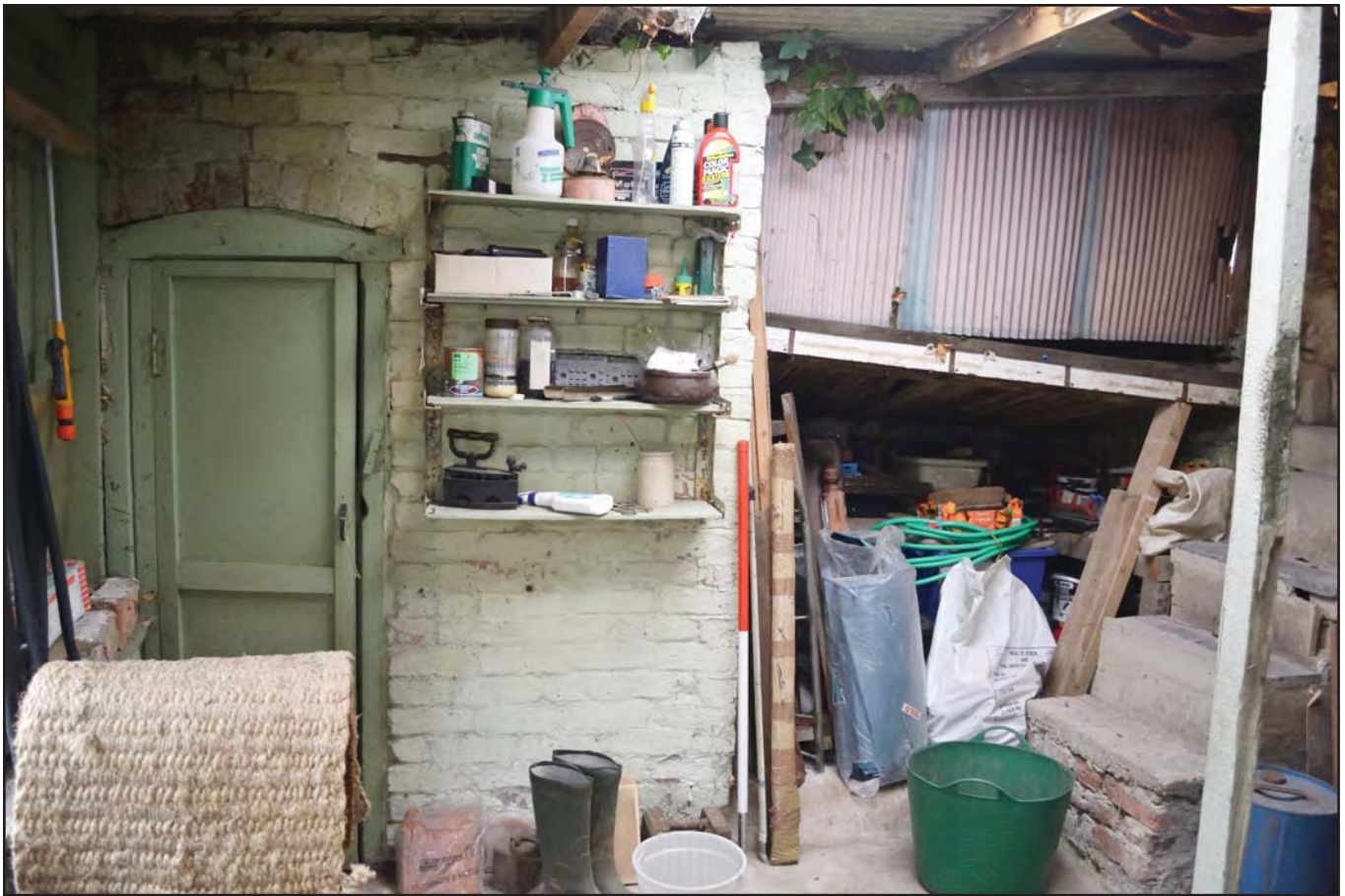
Plate 23: Outside toilet 1 incorporated into the shed, from the south-east; scale: 1x1m (archive reference: G2776_043)
