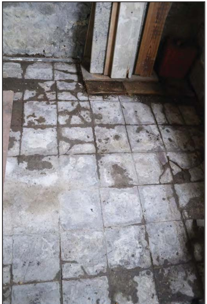
Plate 20: Tiled floor in garage (archive reference: G2776_131)
