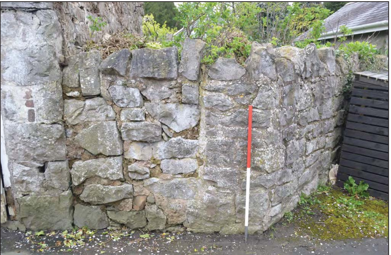
Plate 22: Blocked gateway to north-west of garage, from the north-east (archive reference: G2776_014)
