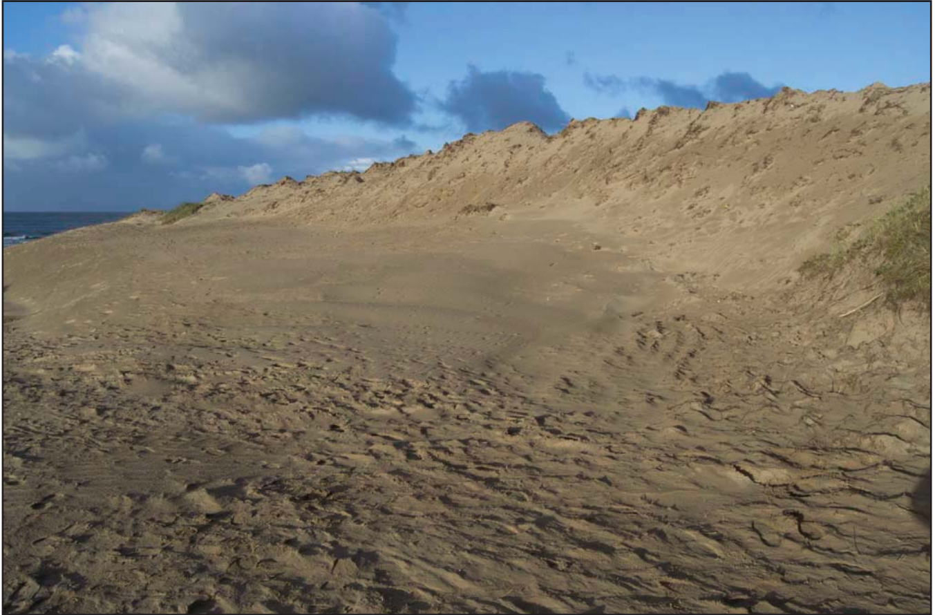
Plate 13: View of the north-west of the notch area showing sand spoil forming wall; (archive reference: G2742_70).
