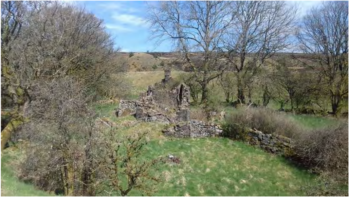
Photo 1, Row of stone-built cottages aligned east-west (NPRN 292019)
