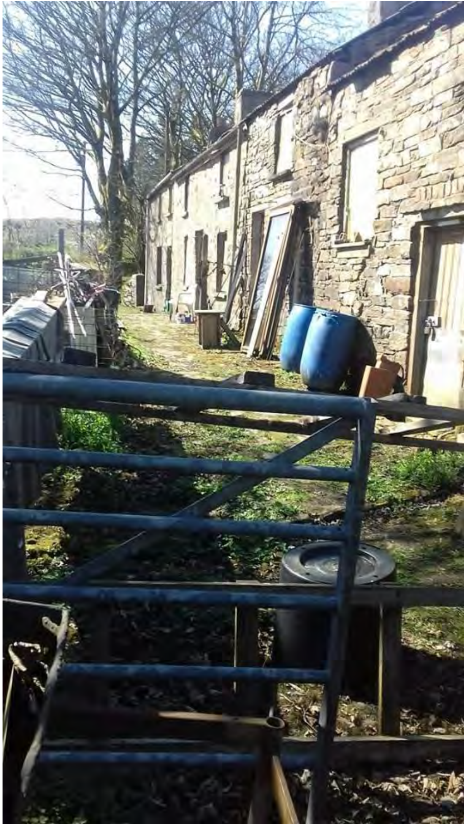
Photo 3, row of two storey cottages (NPRN 292022).
