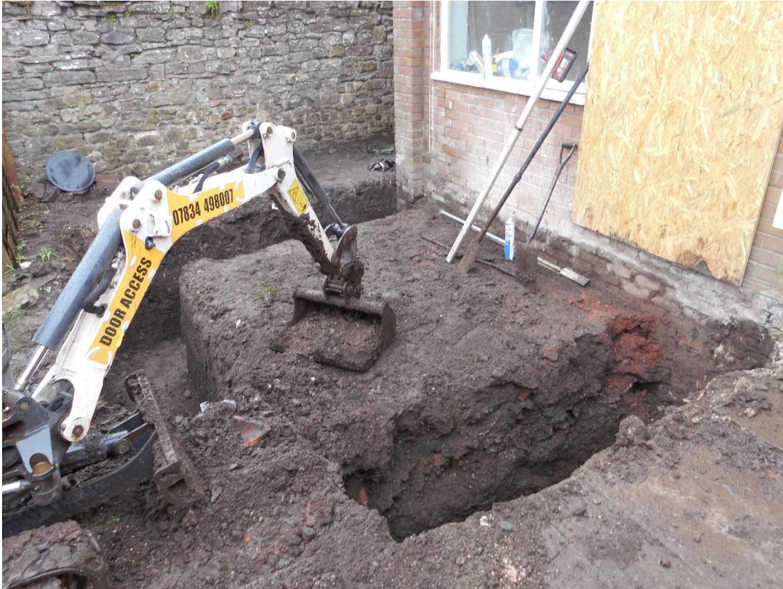
Plate 1. Overview of foundation trench, view to the south
