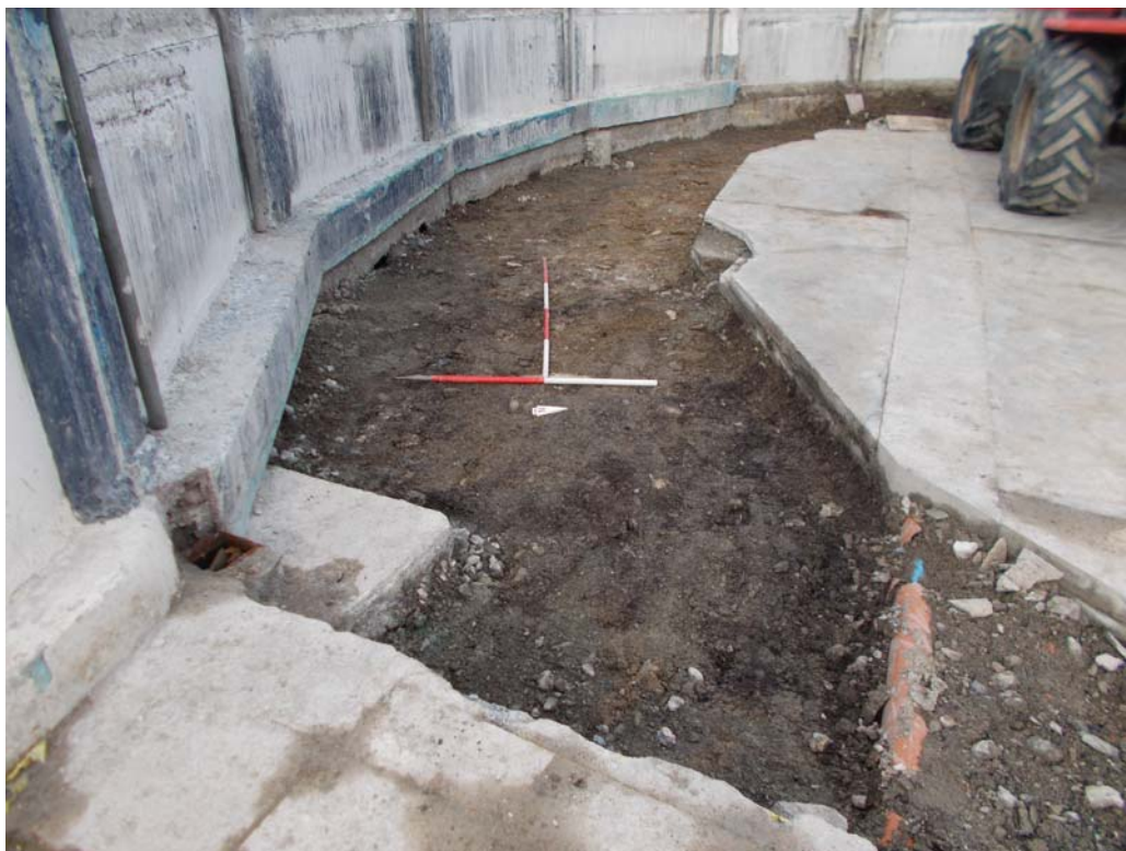
Plate 4 - Plan of groundworks below (100), looking north-west, 1m scales
