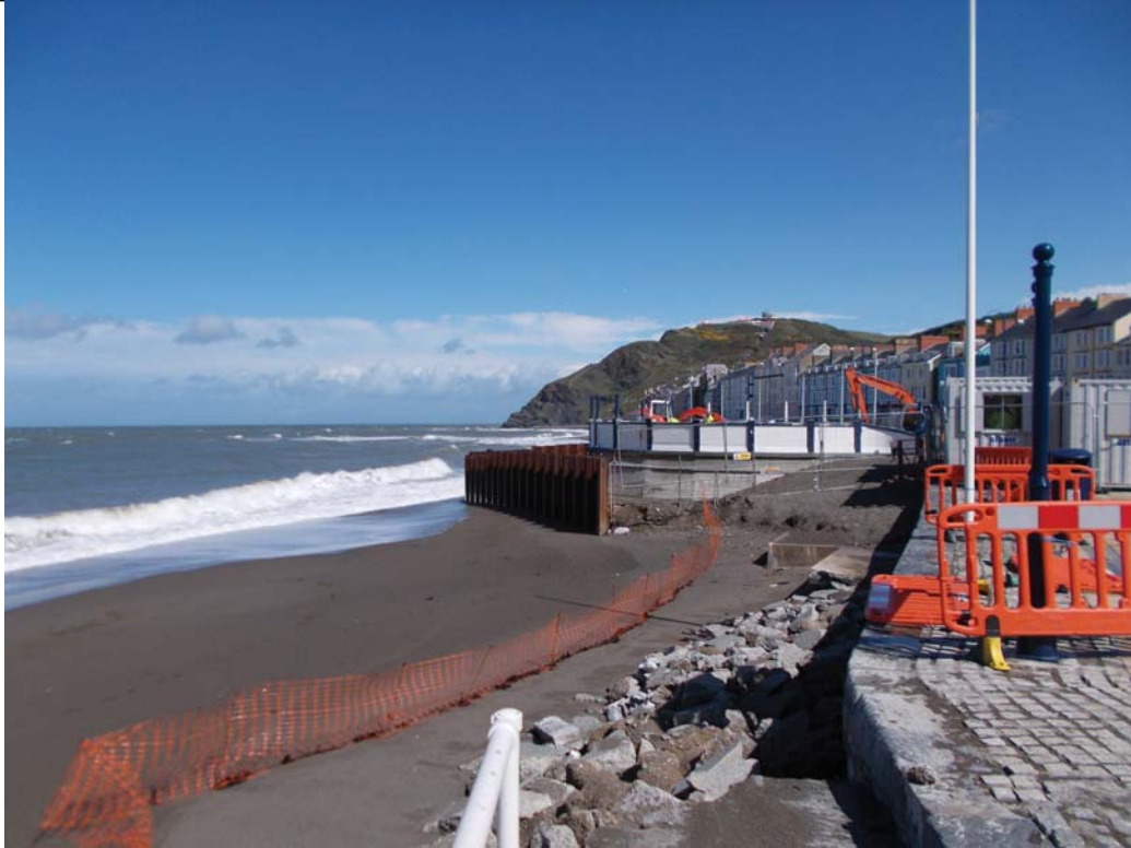
Plate 1 - Overall view of bandstand, looking north-east
