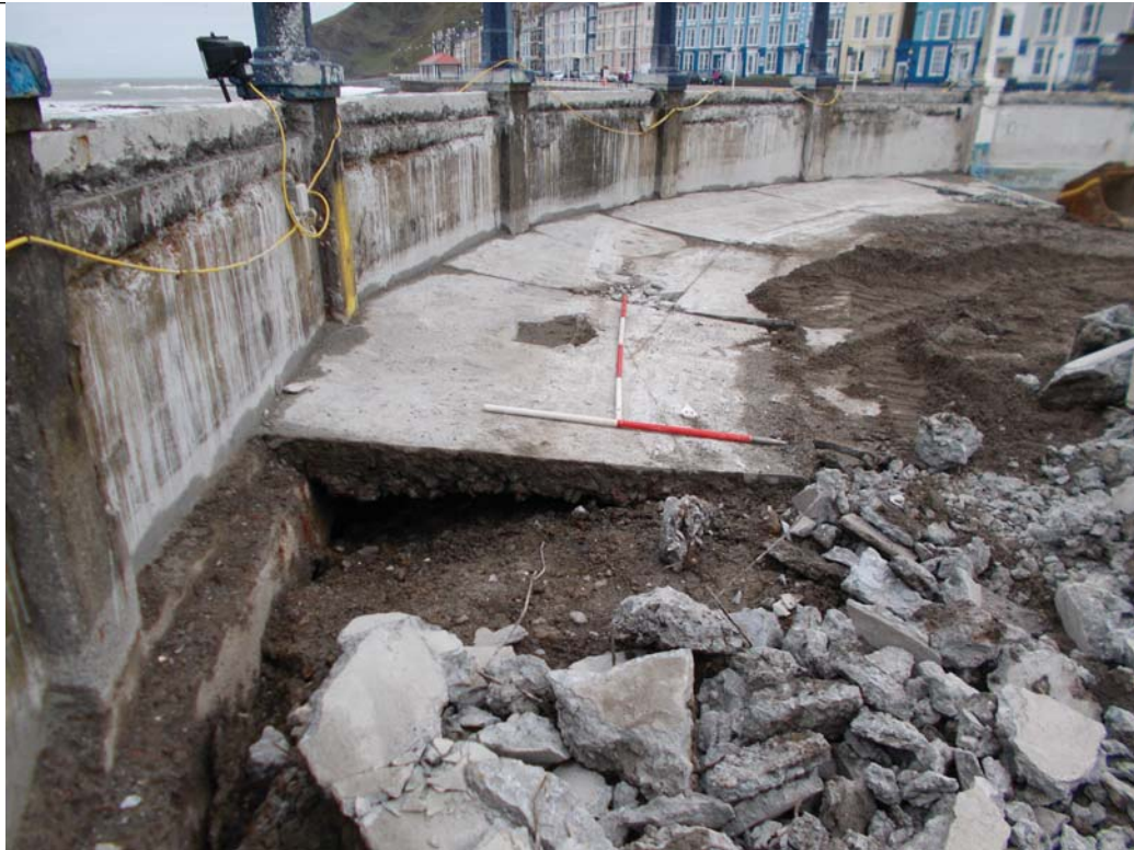
Plate 3 - Bandstand interior, breaking out of concrete slab (100), looking north-east 1m scales
