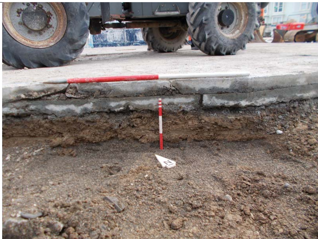
Plate 5 - Section of groundworks (100)-(102), looking north-east, 1m and 0.3m scales
