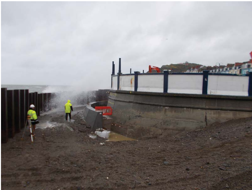
Plate 2 - Exterior view of bandstand, looking north-east
