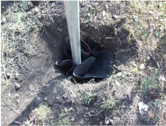
Posthole 5 with membrane covering the stone layer
