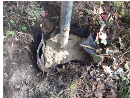
Posthole 9 with membrane covering the archaeology prior to concreting
