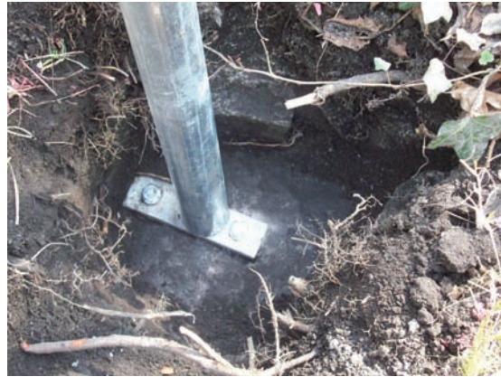
Posthole 9 with bolts drilled into the structural stone
