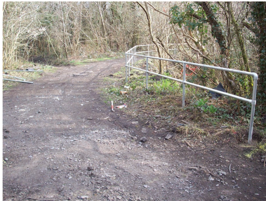
The completed rail on the eastern side of the bridge
