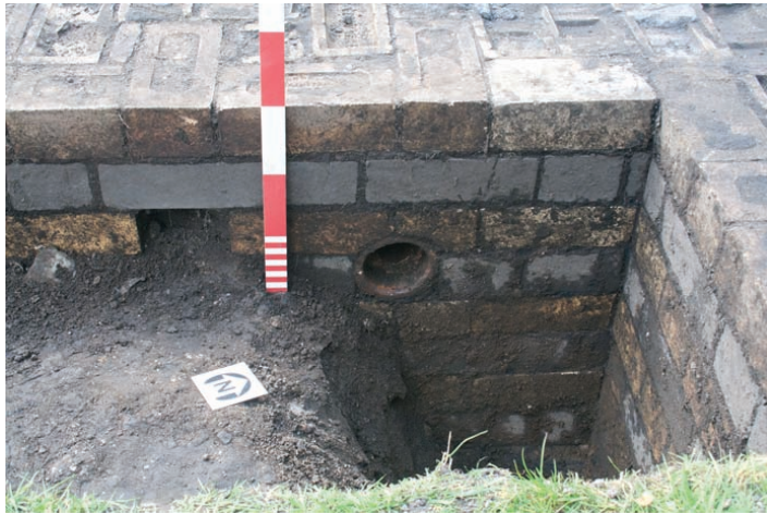
Fig. 16 a. View from the east of below ground drain outlets in north east corner of wall [703].
