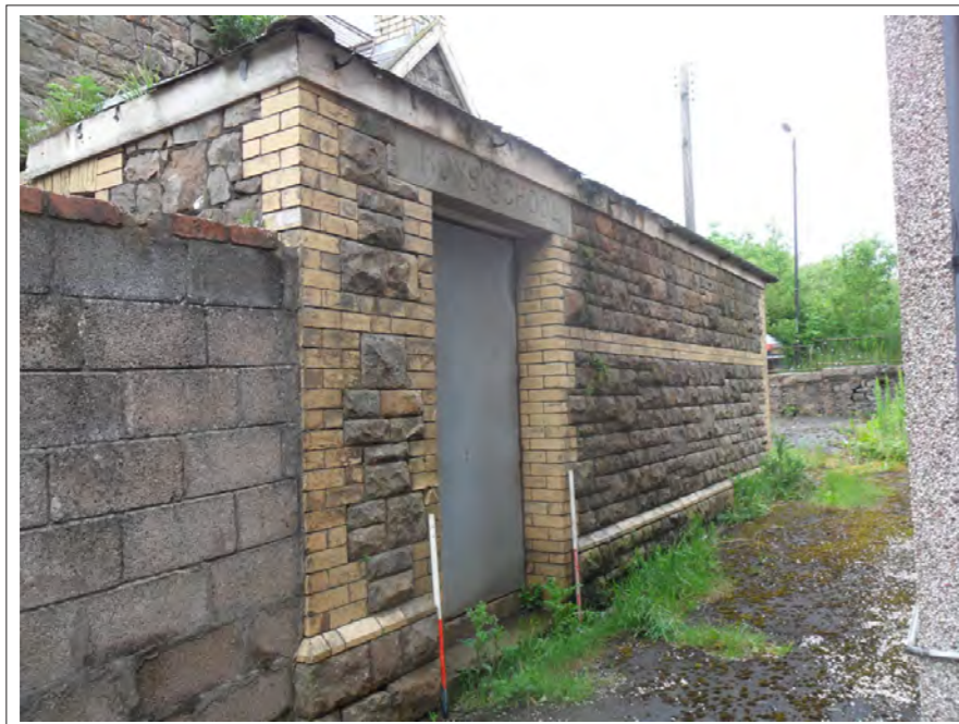
Plate 43: External view of Room 8. Looking north east Scales 2x1m
