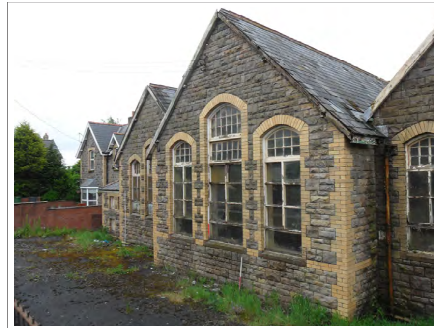
Plate 34: Oblique external view of Room 6. Looking south east Scales 2x1m
