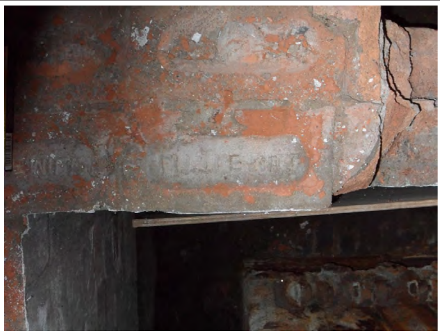
Plate 51: View of 'Little Mill' bricks within Room 9 Boiler surround
