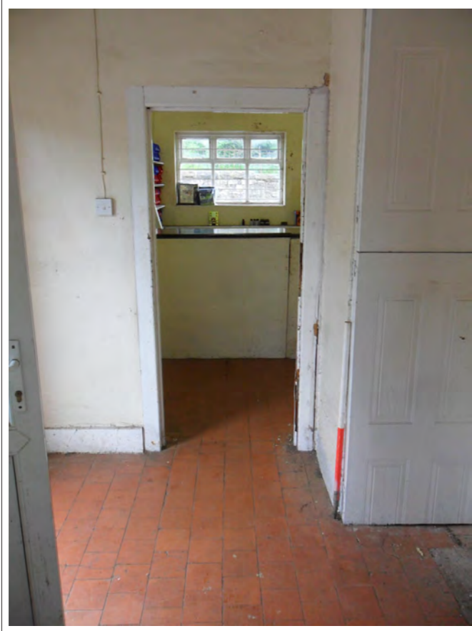
Plate 5: Internal view of Room 2. Scale 1x1m
