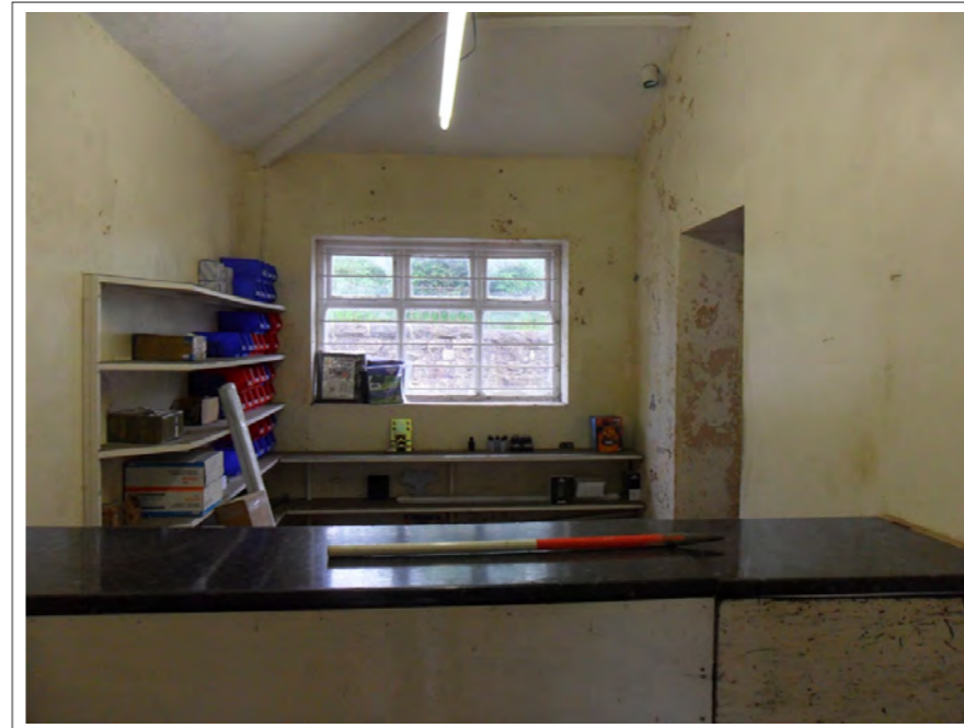
Plate 6: Internal view of Room 3. Scale 1x1m
