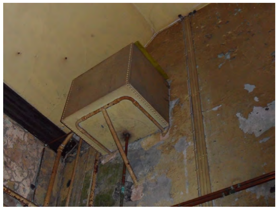
Plate 41: View of metal water tank above doorway in Room 7
