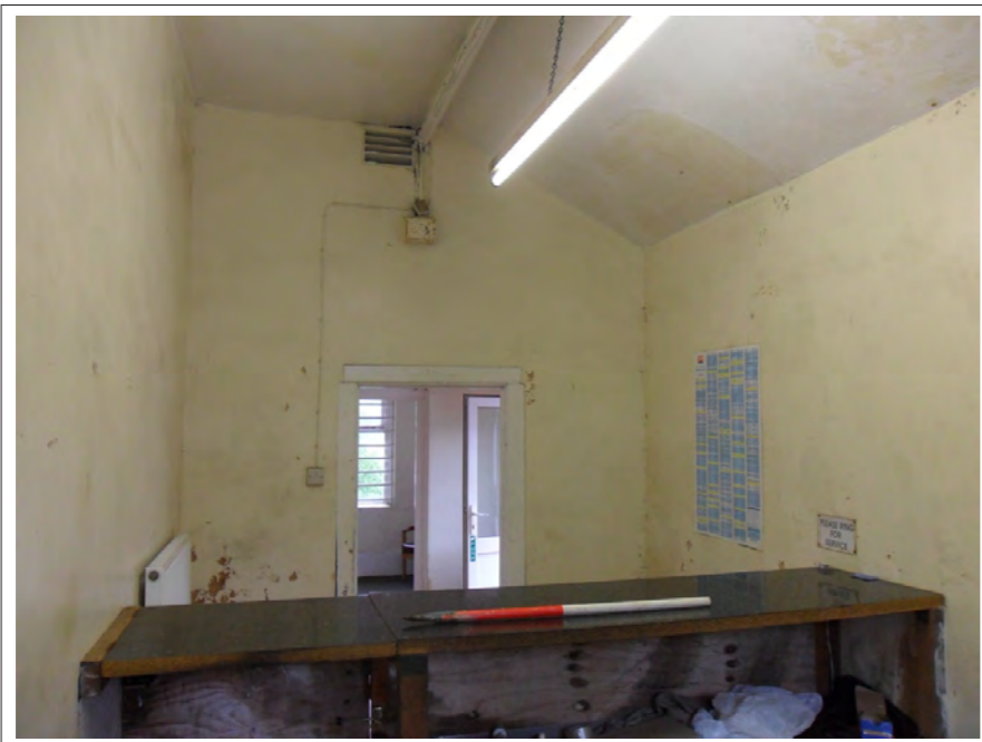
Plate 7: Internal view of Room 3. Scale 1x1m
