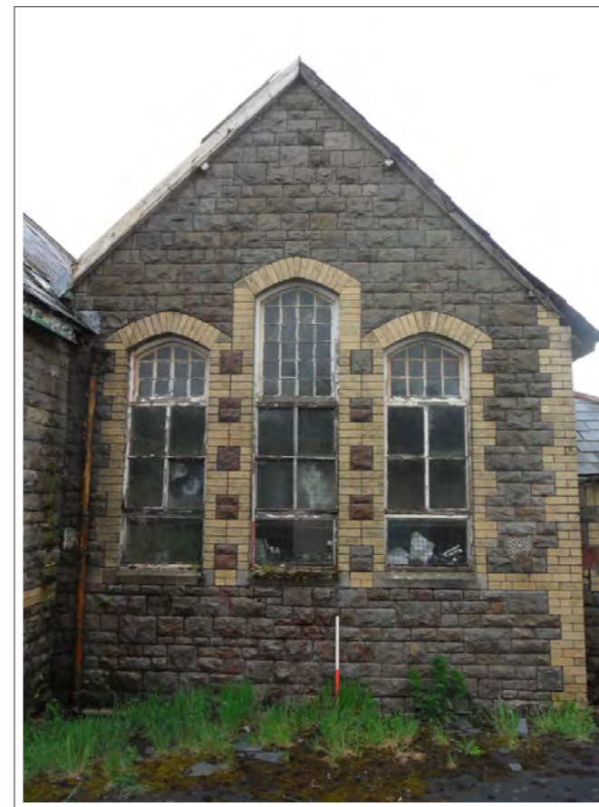
Plate 16: External view of north wall of Room 4. Scales 2x1m
