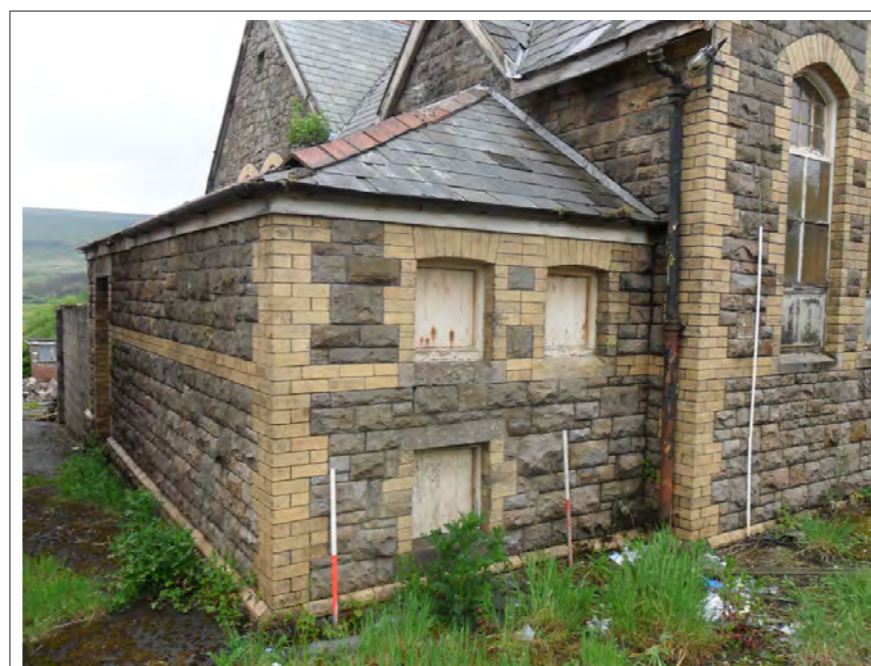
Plate 46: Oblique external view of Room 9. Looking south east Scales 2x1m
