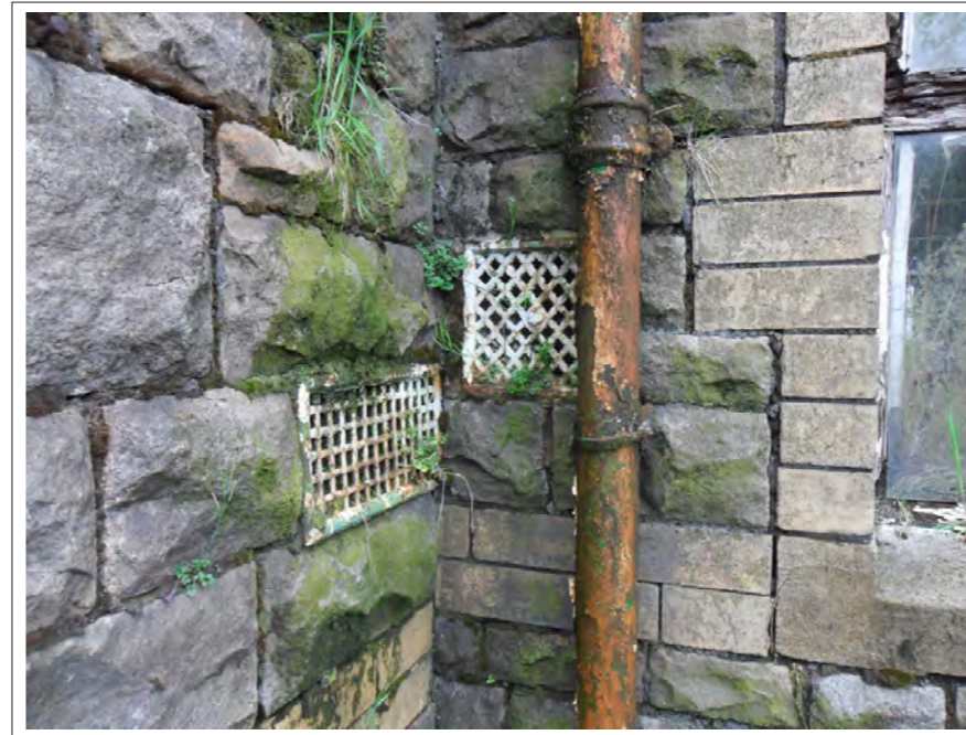
Plate 18: View of original late 19th century air vents within north wall of Room 4
