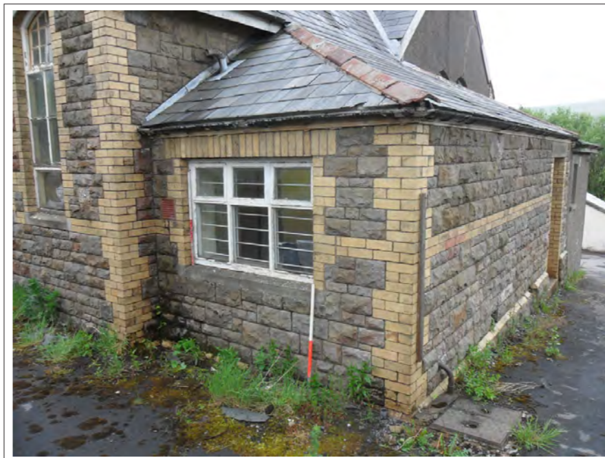
Plate 8: External view of Room 3, Looking south east. Scales 2x1m
