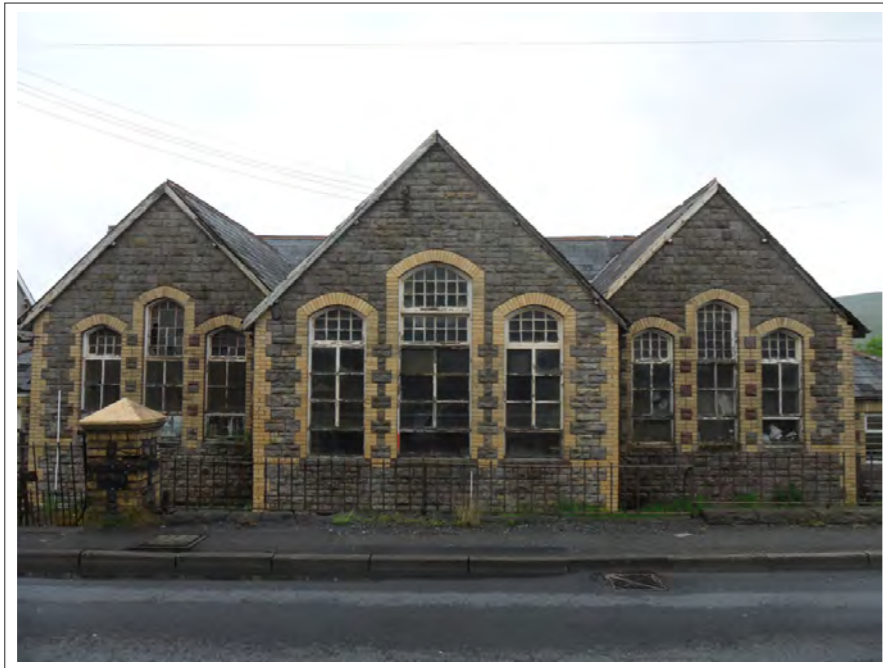
Plate 33: External view of Rooms 4, 6 and 7. Looking south Scales 2x1m
