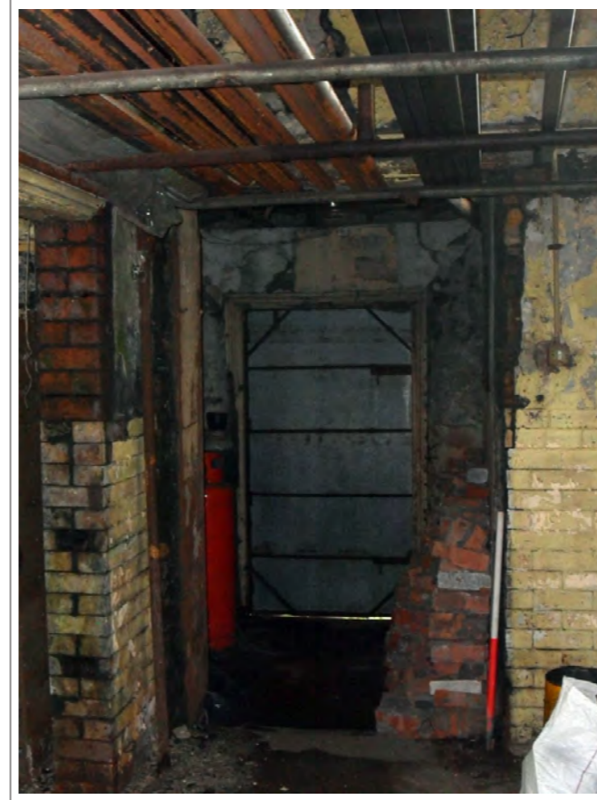
Plate 42: View into Room 8 from Room 5. Scale 1x1m
