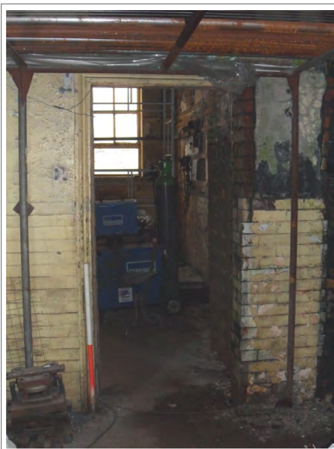
Plate 25: View of doorway into Room 7 from Room 5. Scale 1x1m
