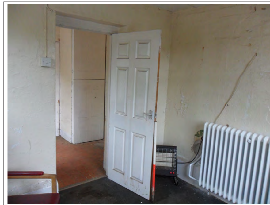
Plate 4: Internal view of Room 1. Scale 1x1m
