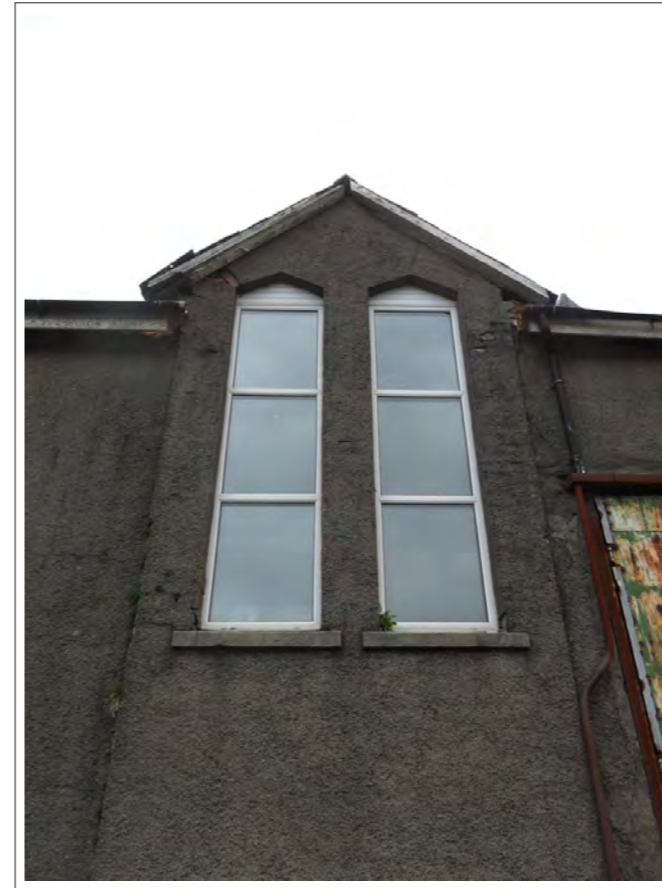
Plate 30: View of UPVC replacement windows within Room 5
