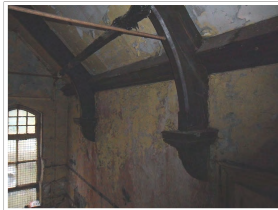
Plate 14: Example view of exposed beam work within school
