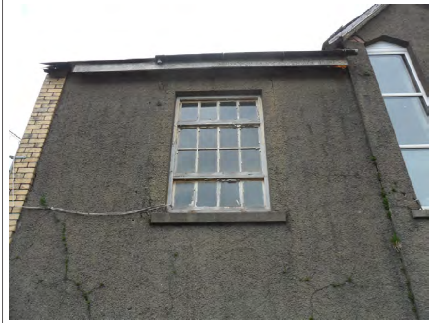
Plate 29: View of modern window inserted into west end of south wall
