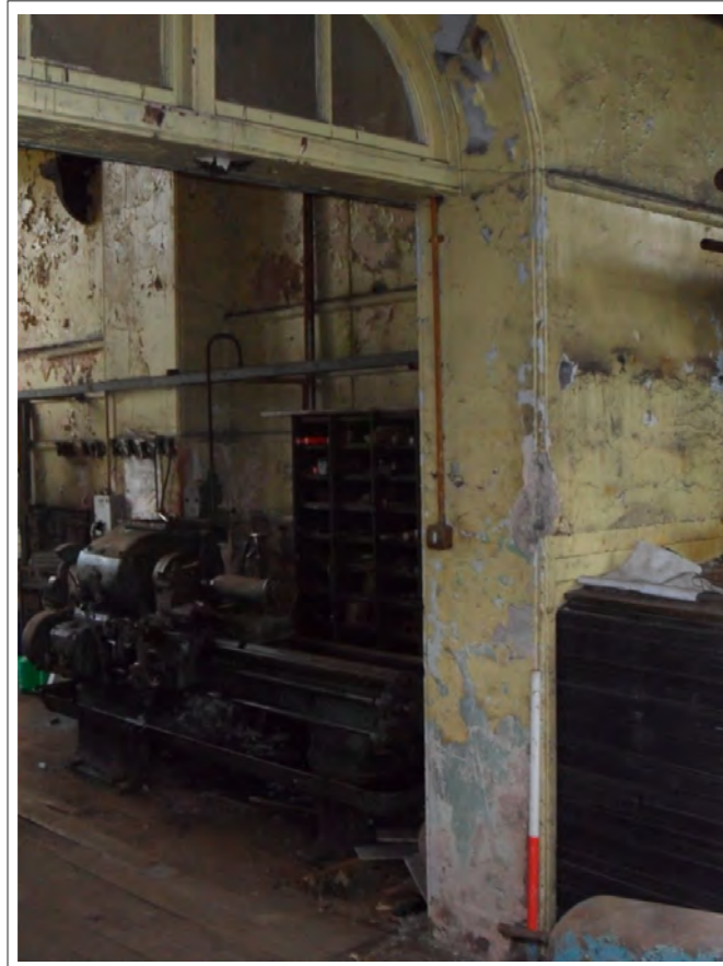
Plate 31: View into Room 6 from Room 5: Scale 1x1m
