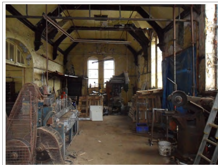
Plate 26: View along full length of Room 5. Looking east
