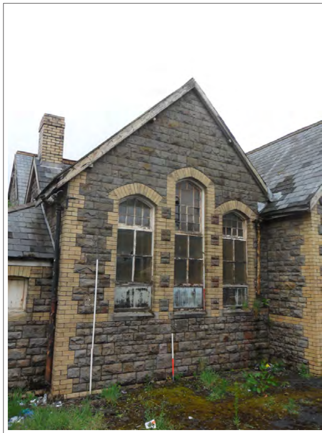
Plate 39: Oblique external view of Room 7. Looking south east. Scales 2x1m
