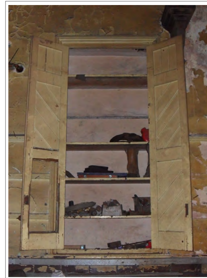
Plate 40: View of recessed cupboard within west wall of Room 7
