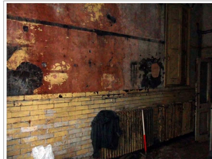
Plate 12: View of east wall of Room 4. Scale 1x1m
