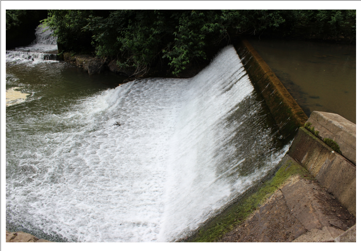
Plate 6: View looking west at weir apron
