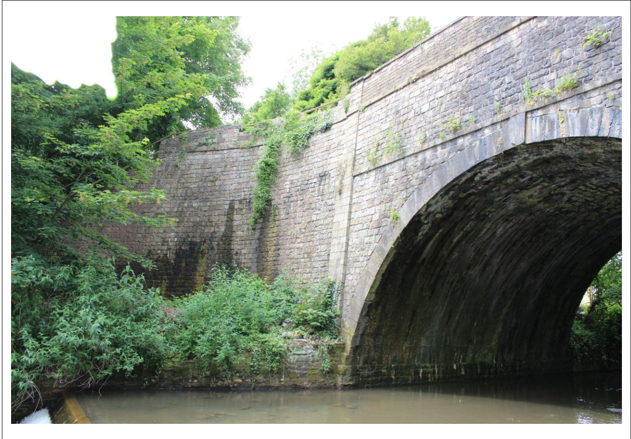
Plate 7: View of western abutment
