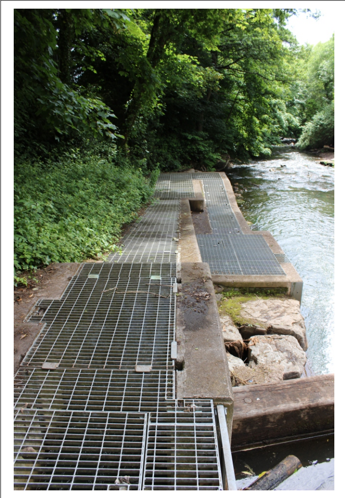
Plate 13: View of fish pass looking downstream
