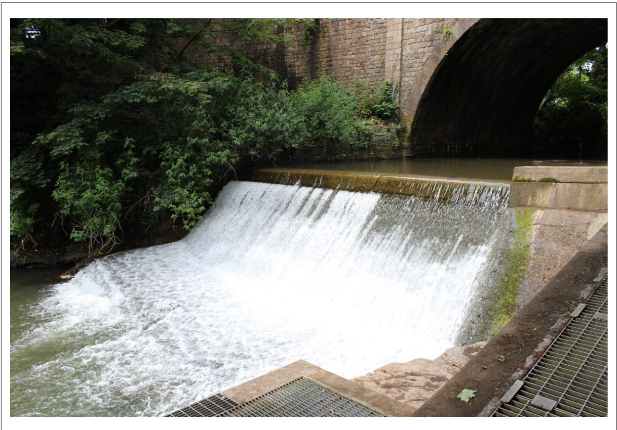
Plate 8: View of apron and scour pad
