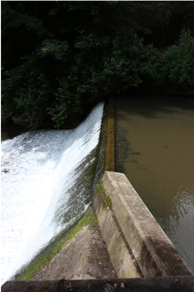
Plate 11: View of timber crest
