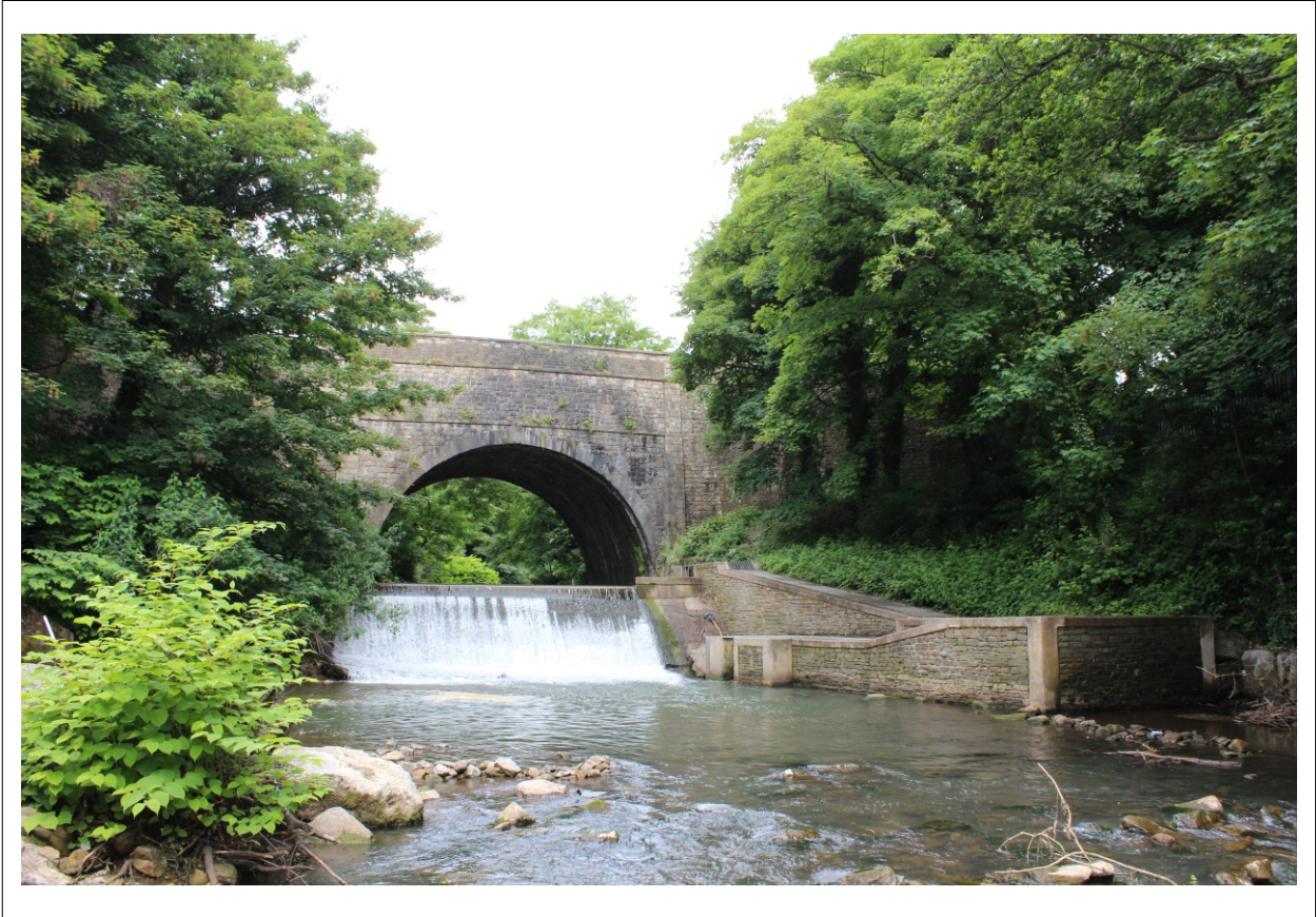
Plate 1: View looking up stream
