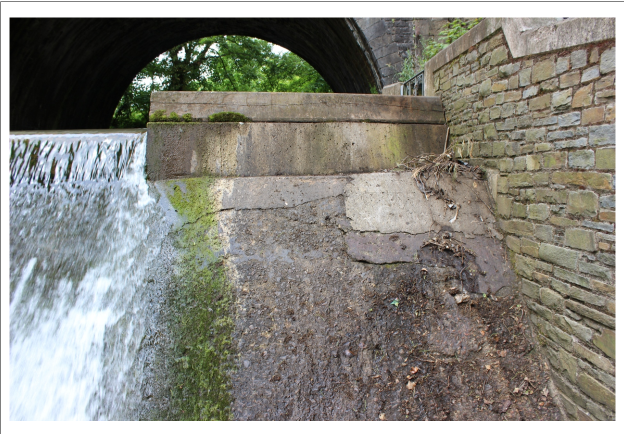
Plate 10: View of weir face and additional concrete repairs
