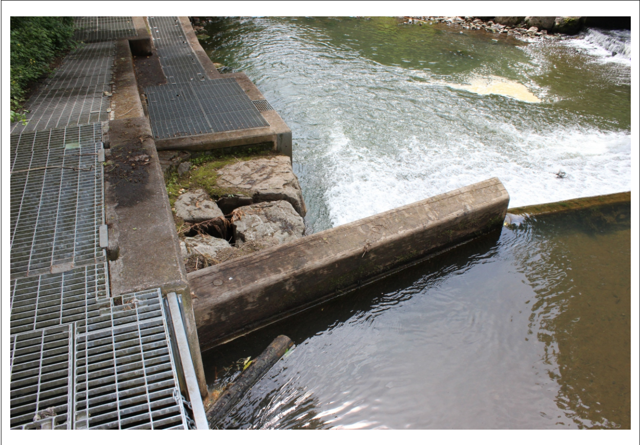
Plate 5: View looking down stream of new eastern abutment
