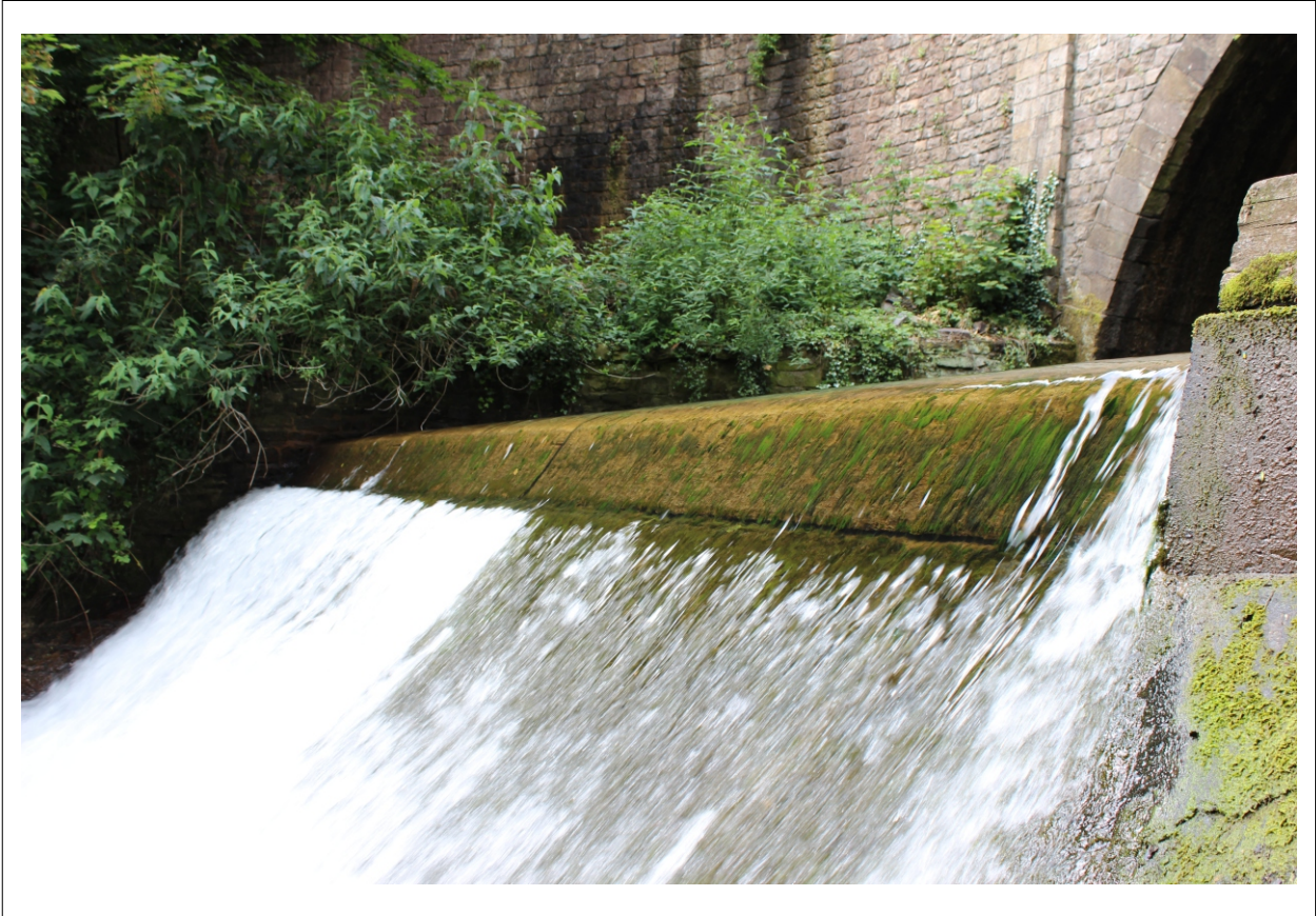
Plate 9: View of timber crest
