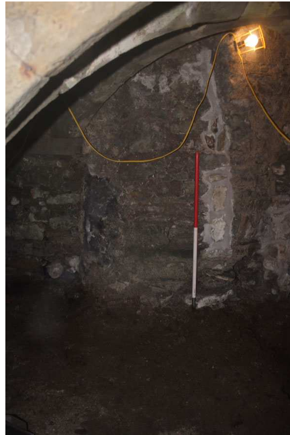
Photo. 6: Looking south at possible medieval doorway.
