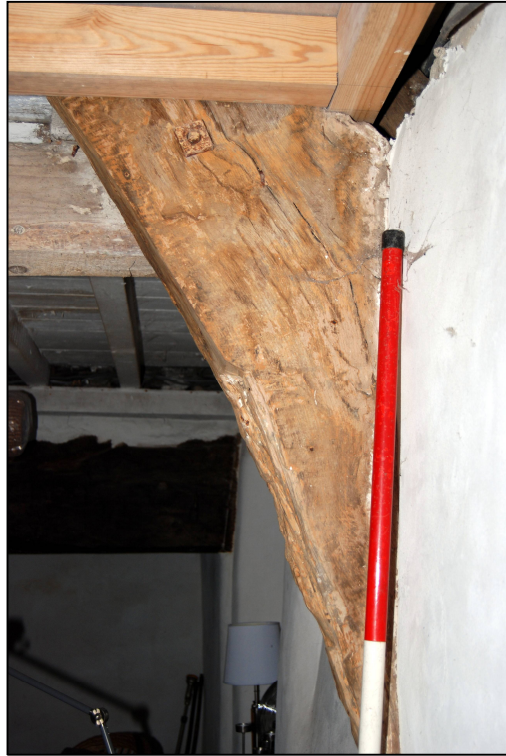
Plate 31: The southern cruck blade in the lower western room, looking west
