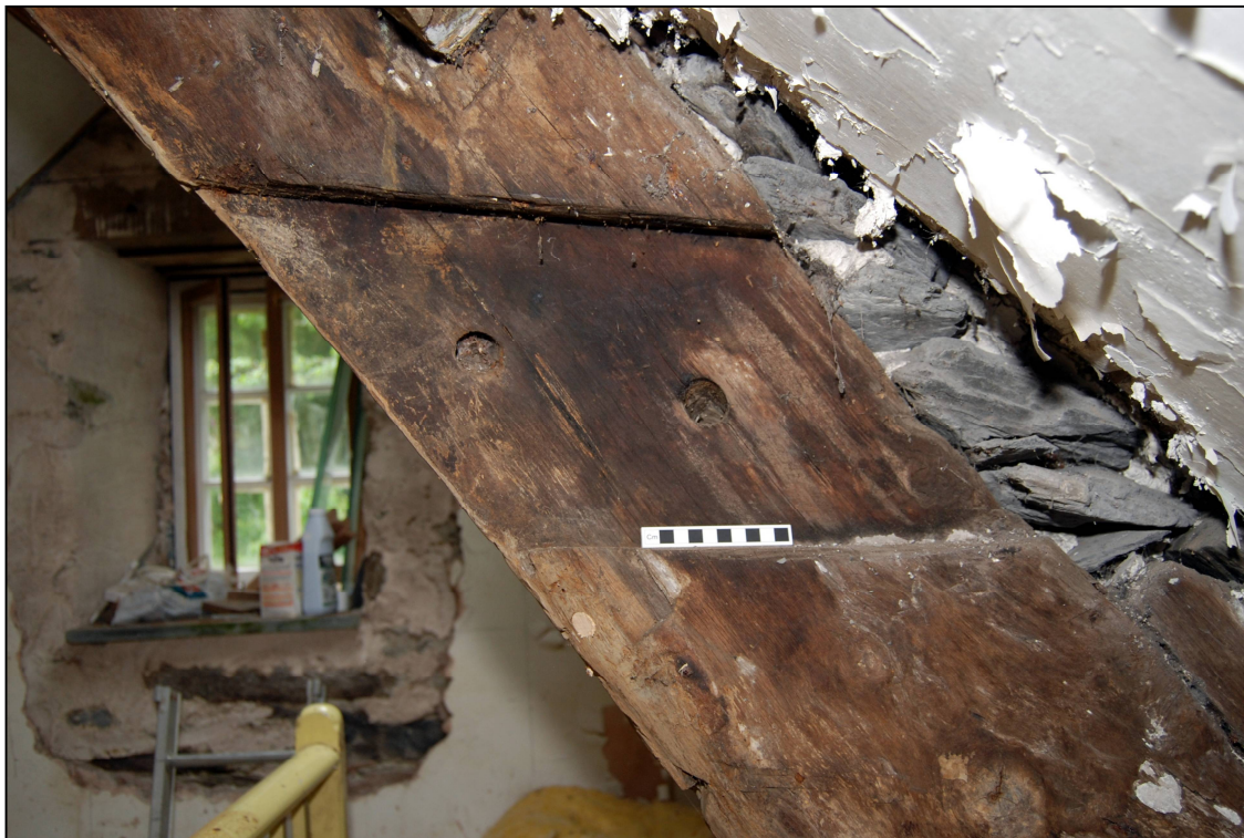
Plate 37: Socket for the collar on the northern blades of Truss 2
