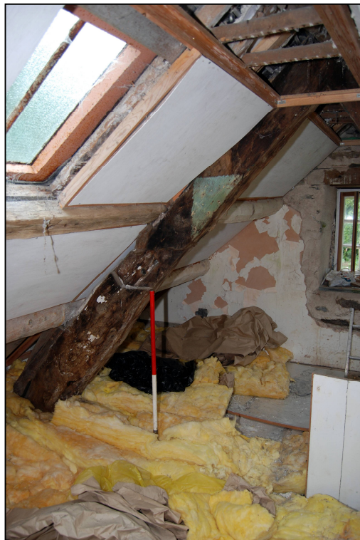
Plate 34: The southern blade of Truss 2
