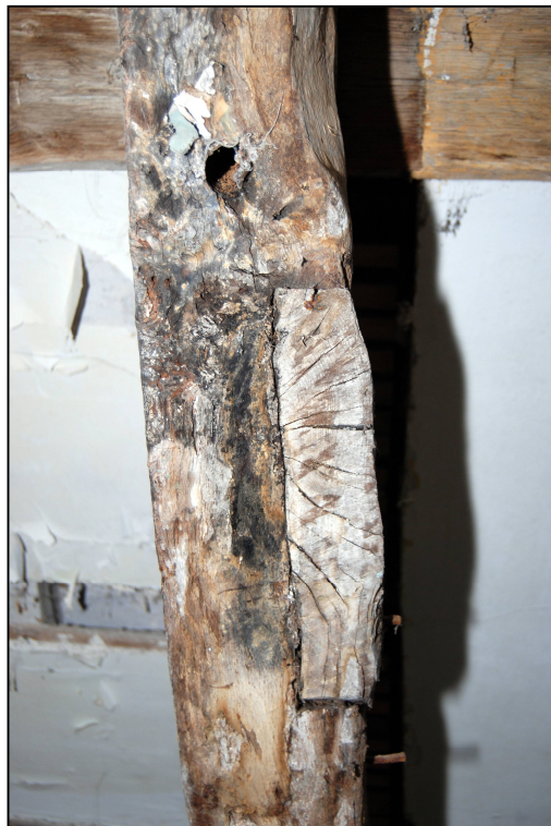
Plate 18: Joint between the collar and the northern principal rafter of Truss 1
