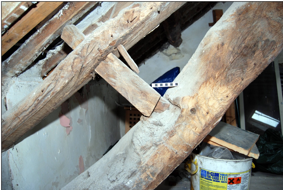
Plate 21: Support for the secondary rafter on the southern side of Truss 1
