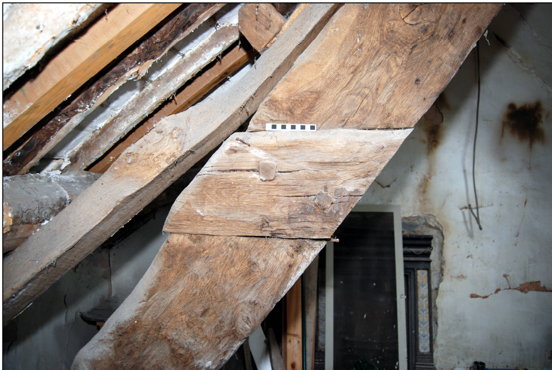
Plate 16: Remains of the collar on the southern principal rafter of Truss 1
