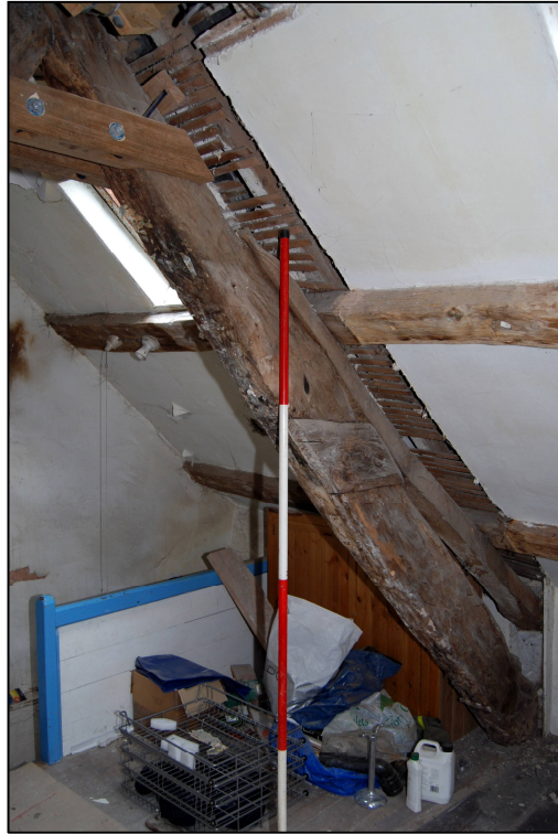
Plate 13: The northern principal rafter of Truss 1
