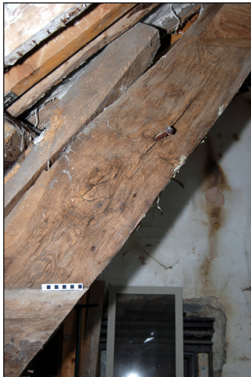
Plate 20: Iron nail on southern principal rafter of Truss 1
