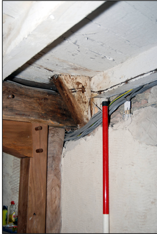
Plate 11: Base of northern principal rafter of Truss 1, looking NW
