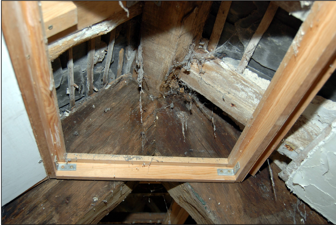
Plate 33: Peak of Truss 2
