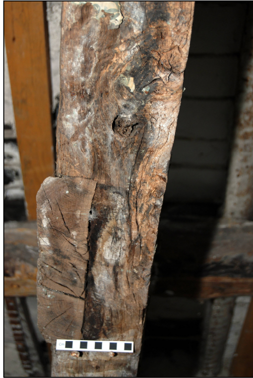
Plate 17: Joint between the collar and the southern principal rafter of Truss 1
