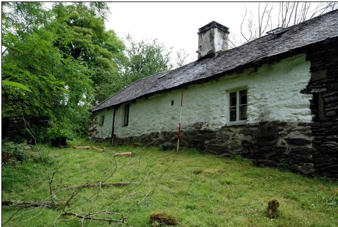
Plate 3: Rear elevation, looking NW
