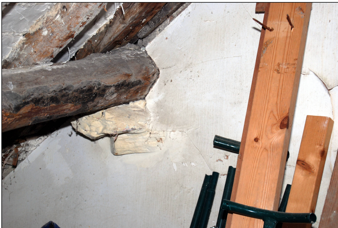
Plate 24: Rough corbel supporting the eastern end of the northern lower purlin
