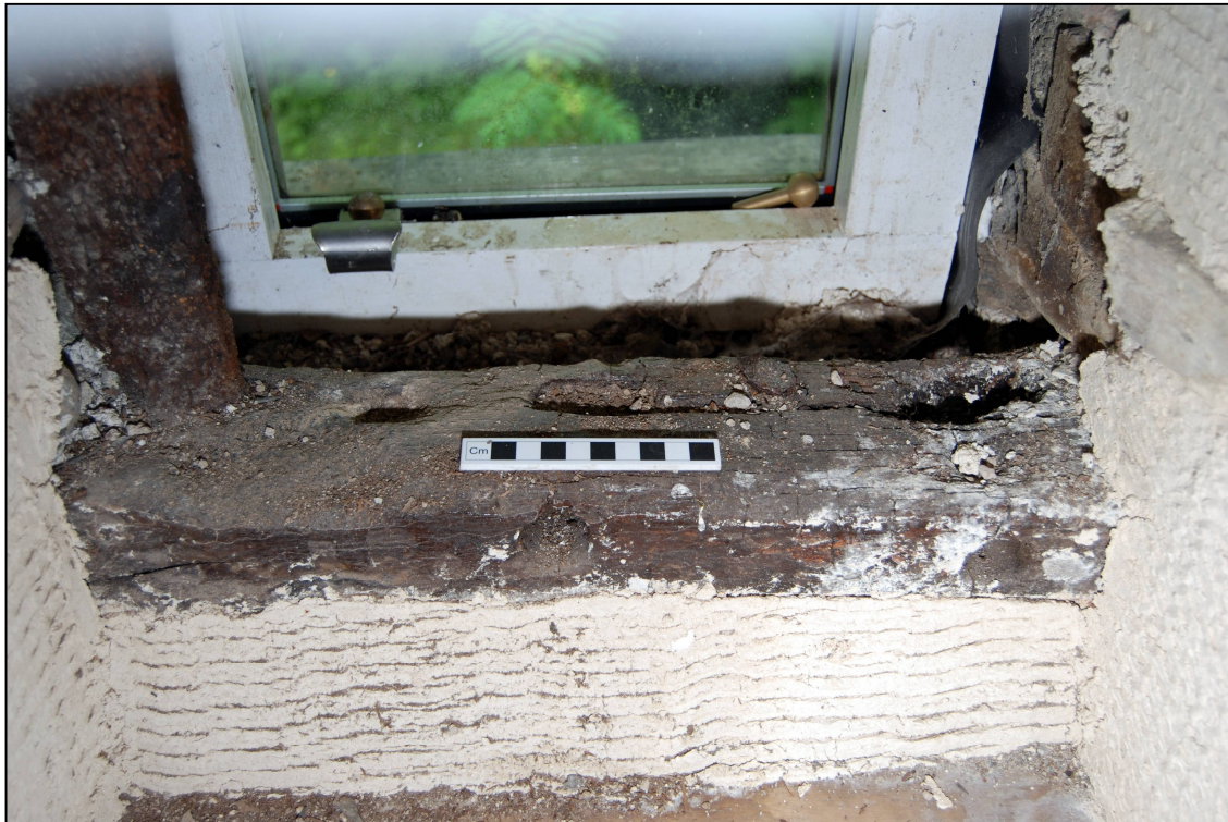
Plate 27: Sockets in the lower frame of the window in the SW corner of the lower western room
