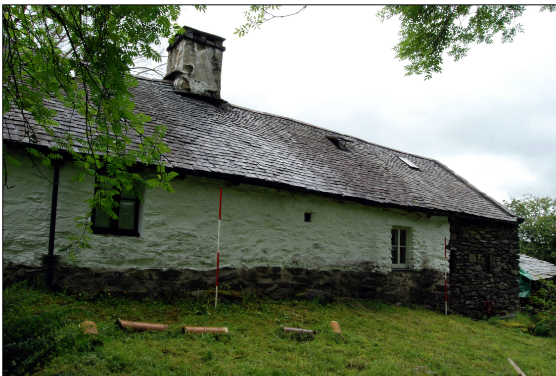
Plate 4: Rear elevation looking NE
