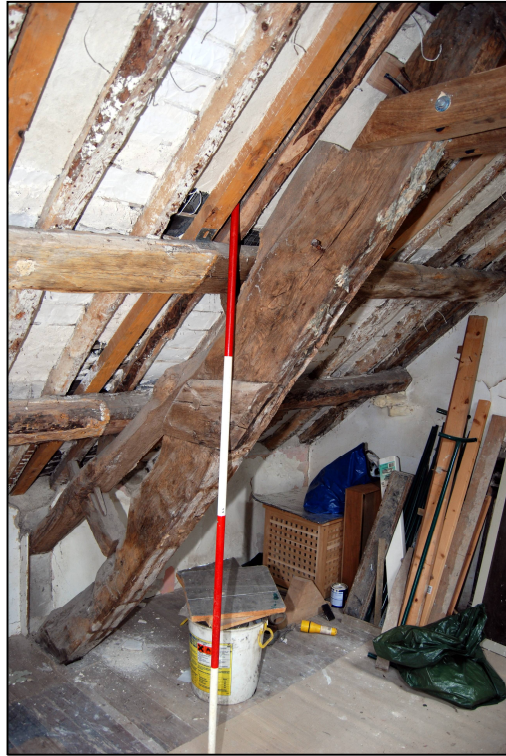
Plate 15: The southern principal rafter of Truss 1
