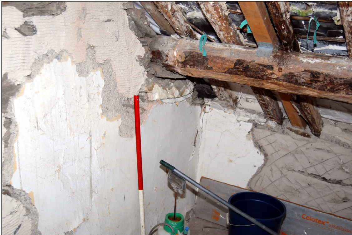
Plate 23: Rough corbel supporting the western end of the northern lower purlin
