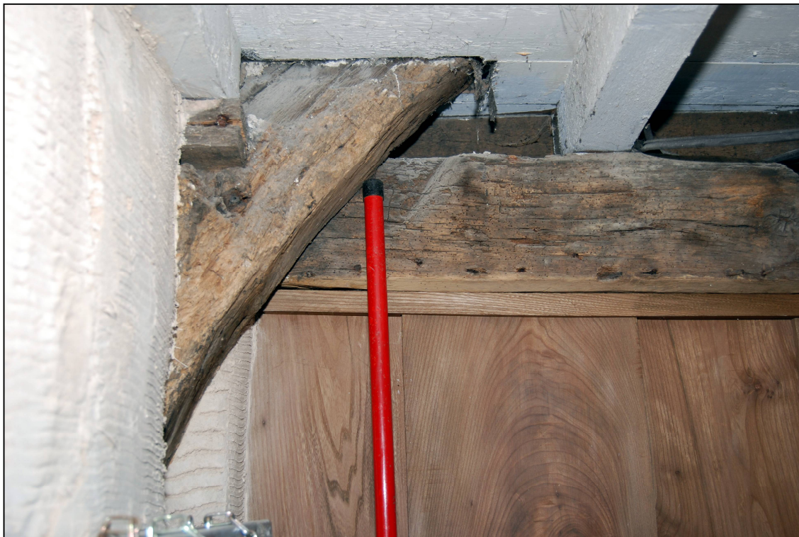
Plate 10: Base of the southern principal rafter of Truss 1, looking west
