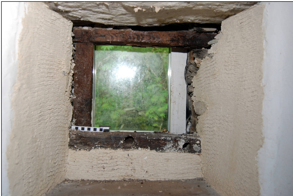
Plate 26: Window in SW corner of lower western room
