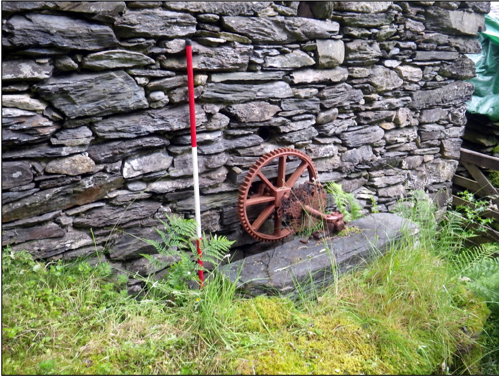
Plate 7: Iron drive wheel on rear elevation of the eastern extension
