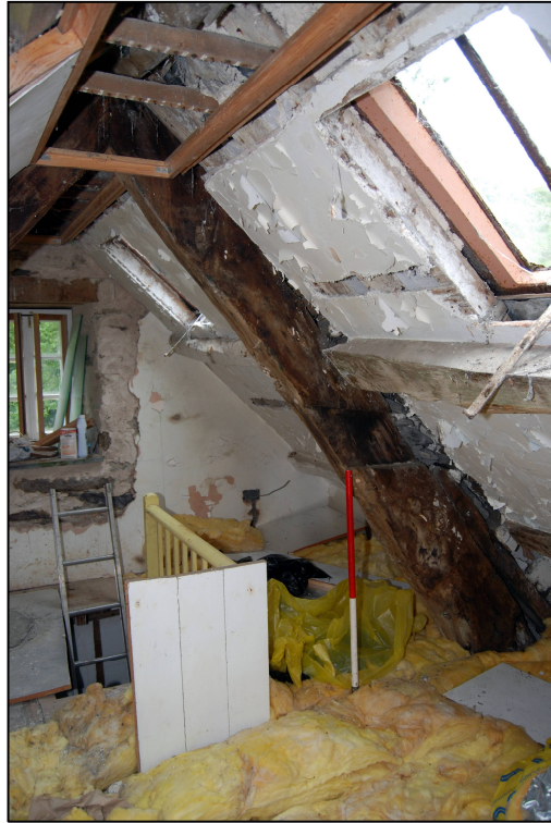
Plate 35: The northern blade of Truss 2
