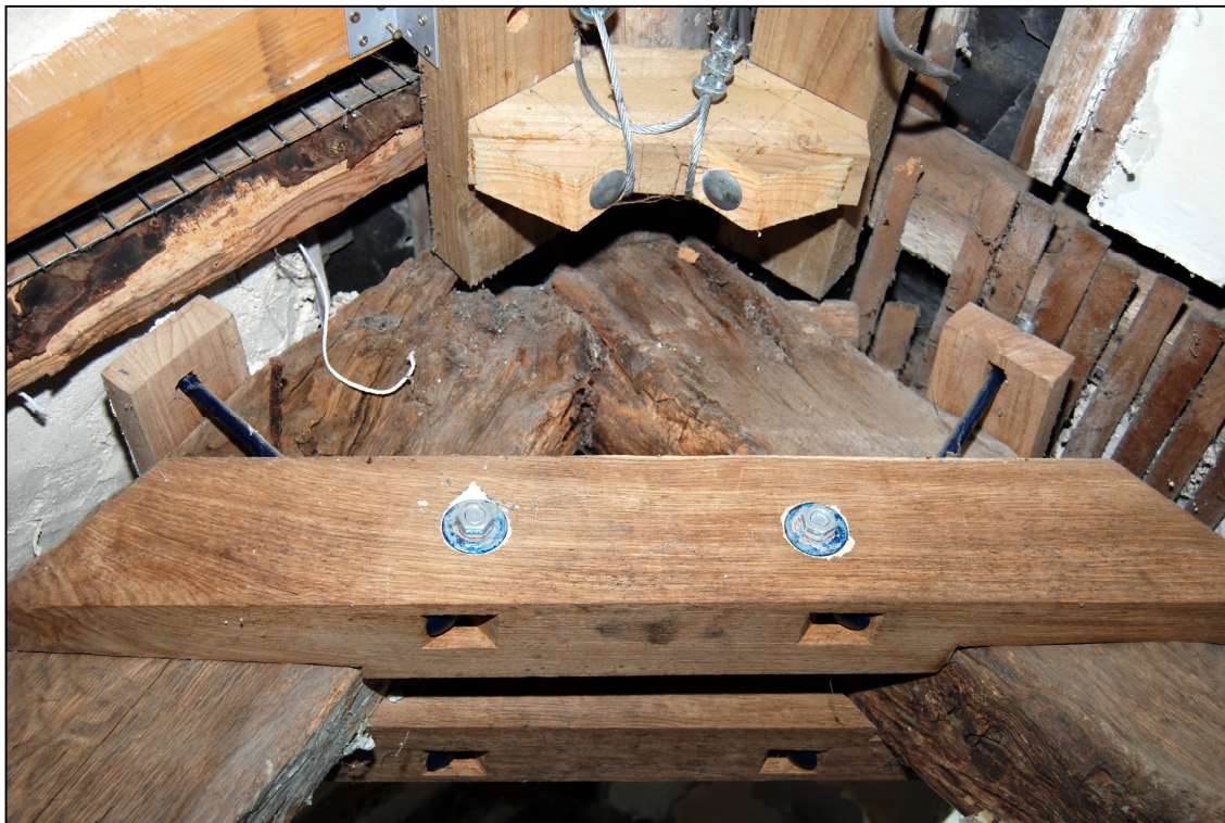
Plate 12: Peak of Truss 1
