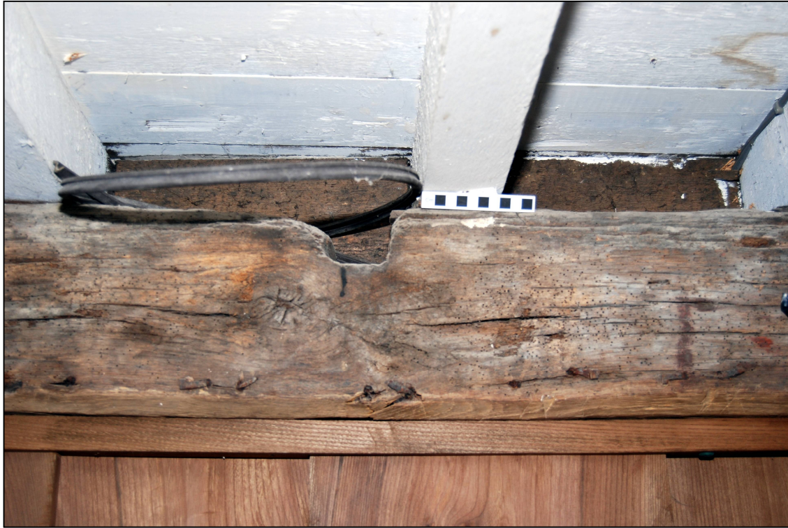
Plate 9: Mortise on top of beam in the eastern ground floor room
