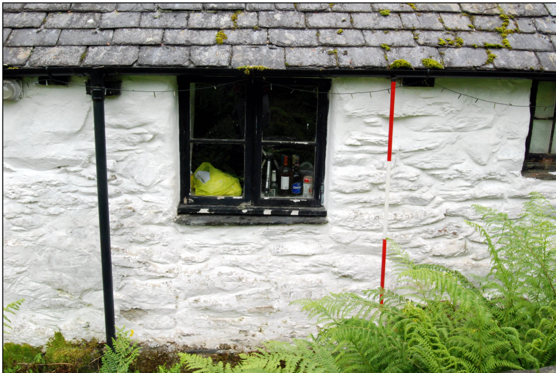
Plate 8: Partially blocked doorway in the front elevation
