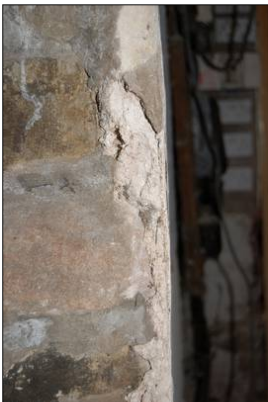
Plate 39: Detail of the section of the plaster in Room 2
