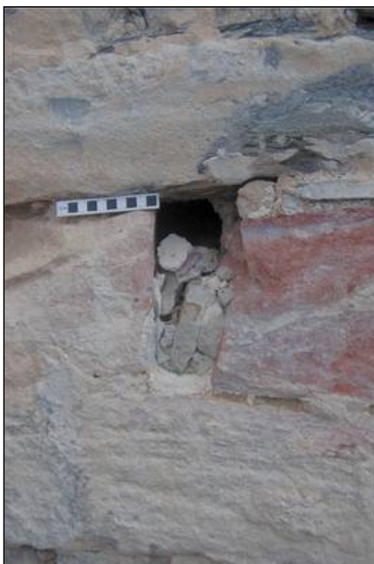
Plate 13: Detail of the “squint window” on the first floor level, northern face of the northern bay
