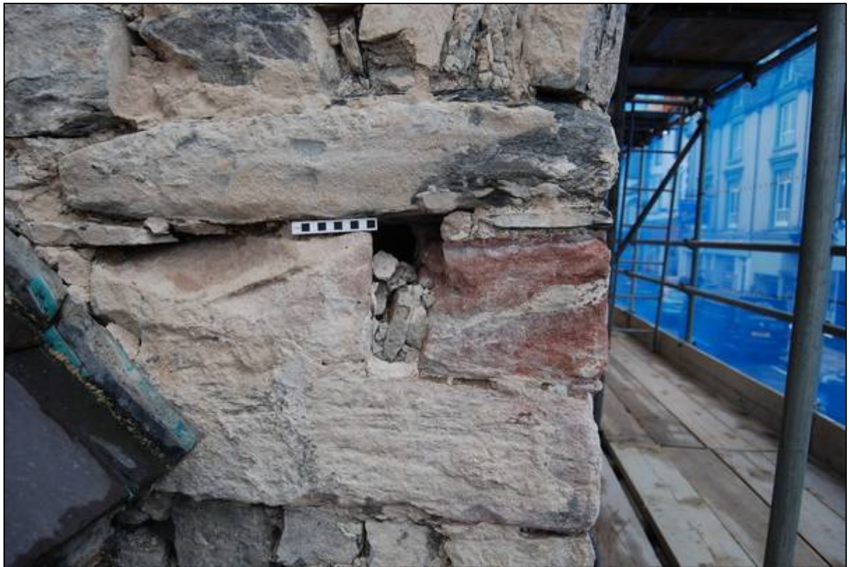
Plate 9: “Squint window” in the first floor, northern face of the northern bay
