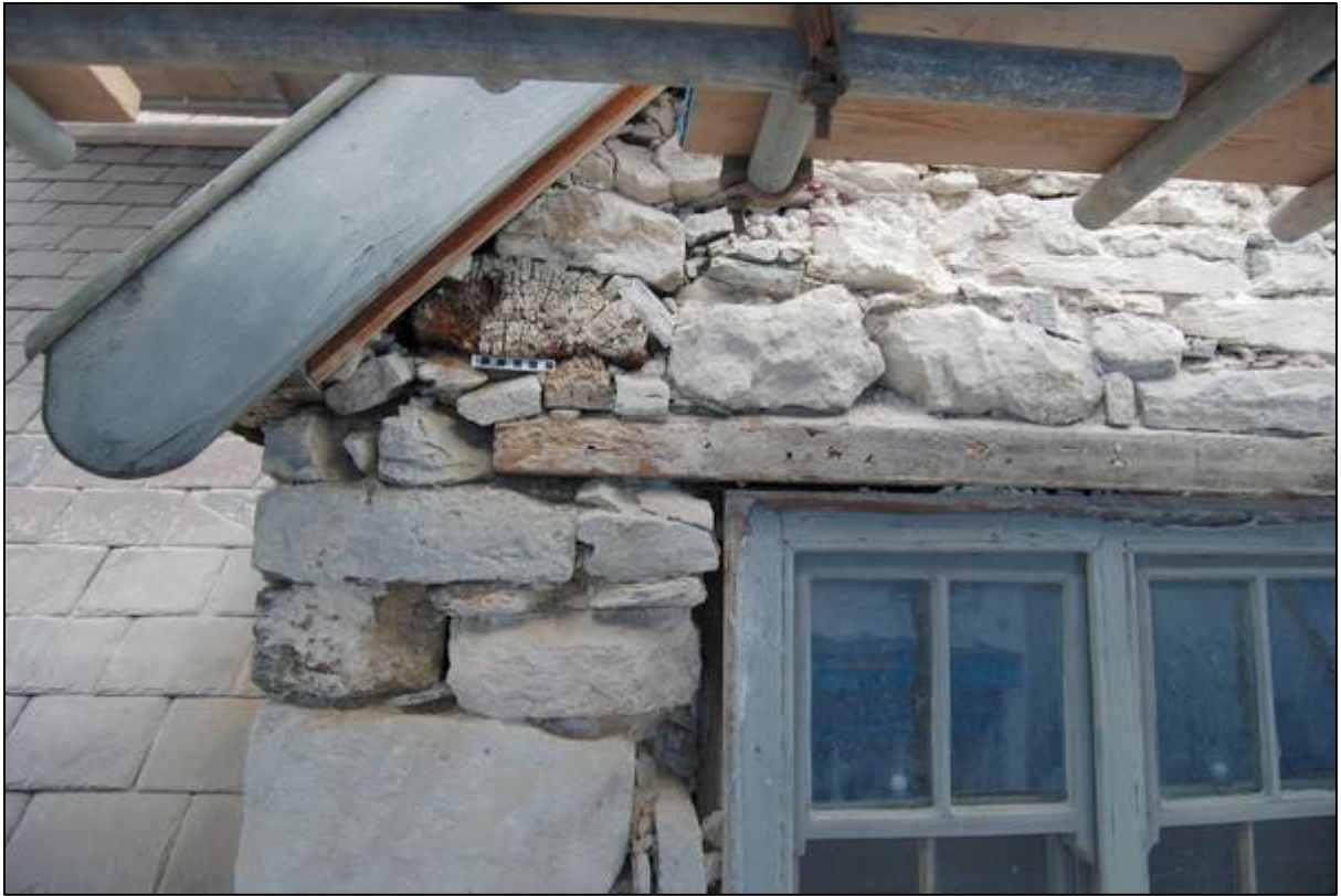
Plate 27: Exposed purlin in the gable of the southern bay
