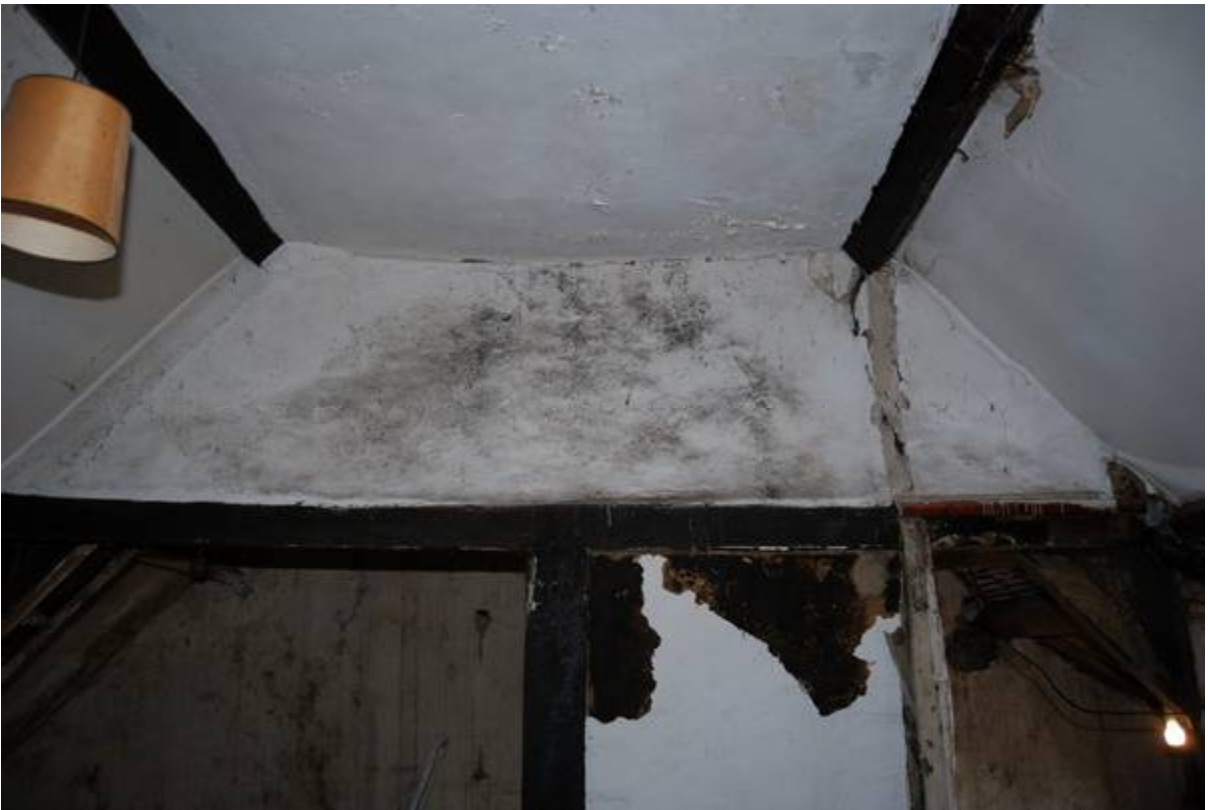
Plate 42: The wattle and daub partition below Truss 1
