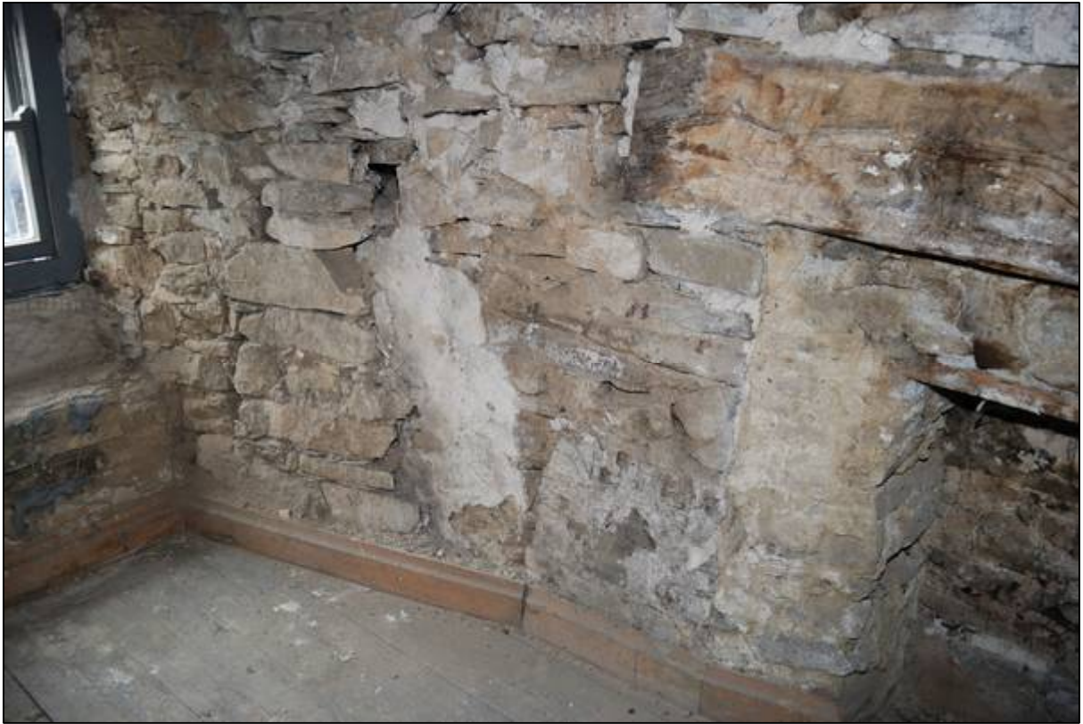
Plate 49: Plaster behind the stonework for the dormer in Room 7
