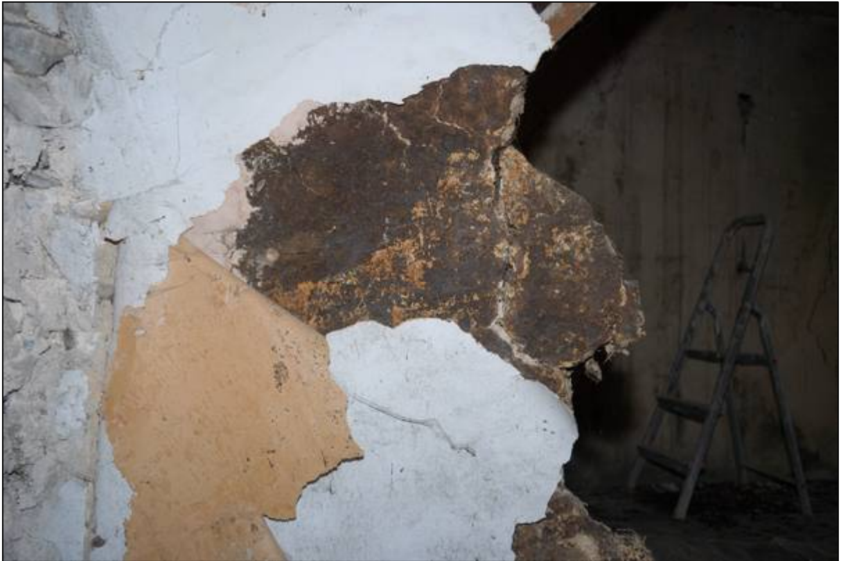
Plate 43: Detail of the surface of the wattle and daub partition below Truss 1
