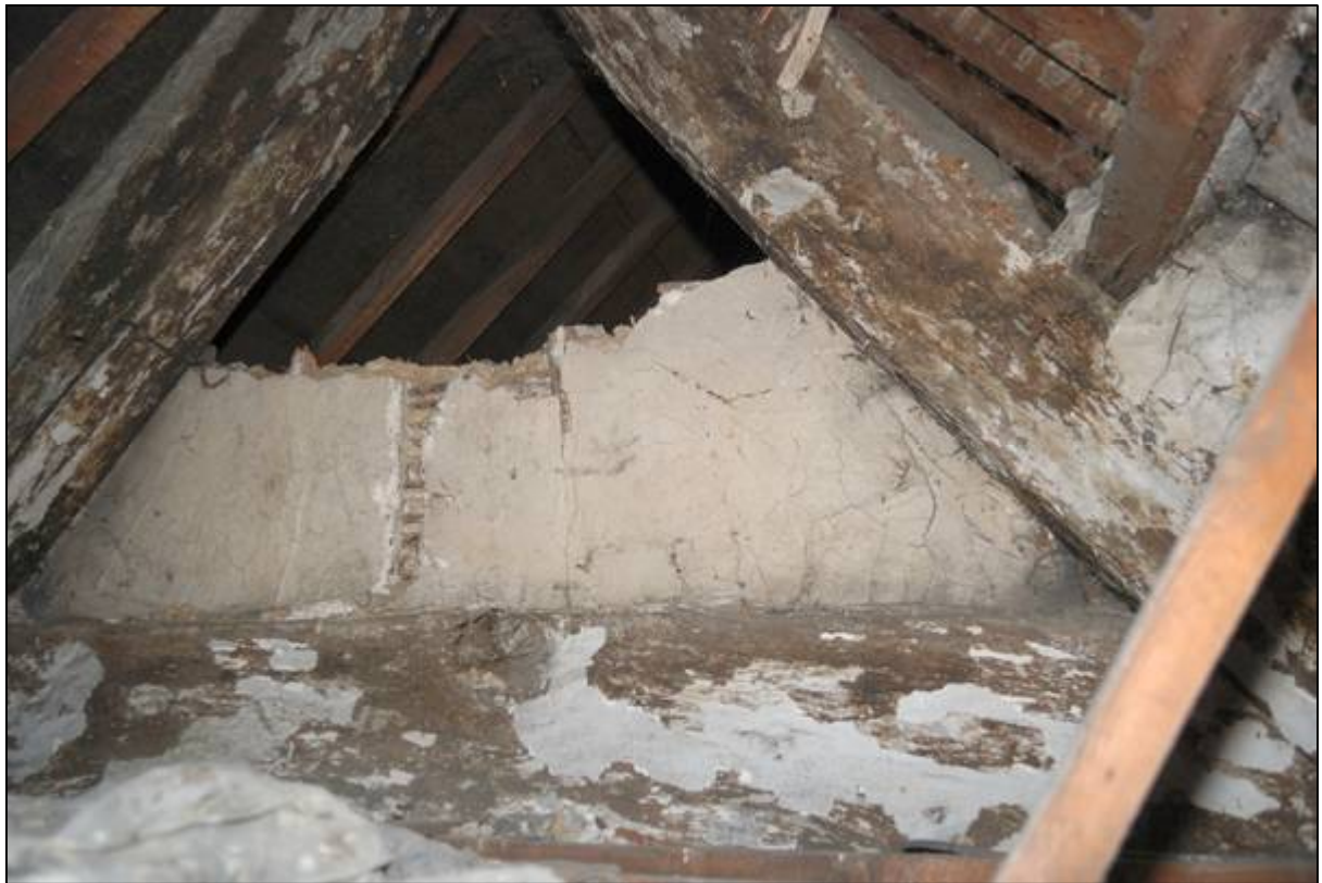
Plate 45: Partition in the roof space, below Truss 1
