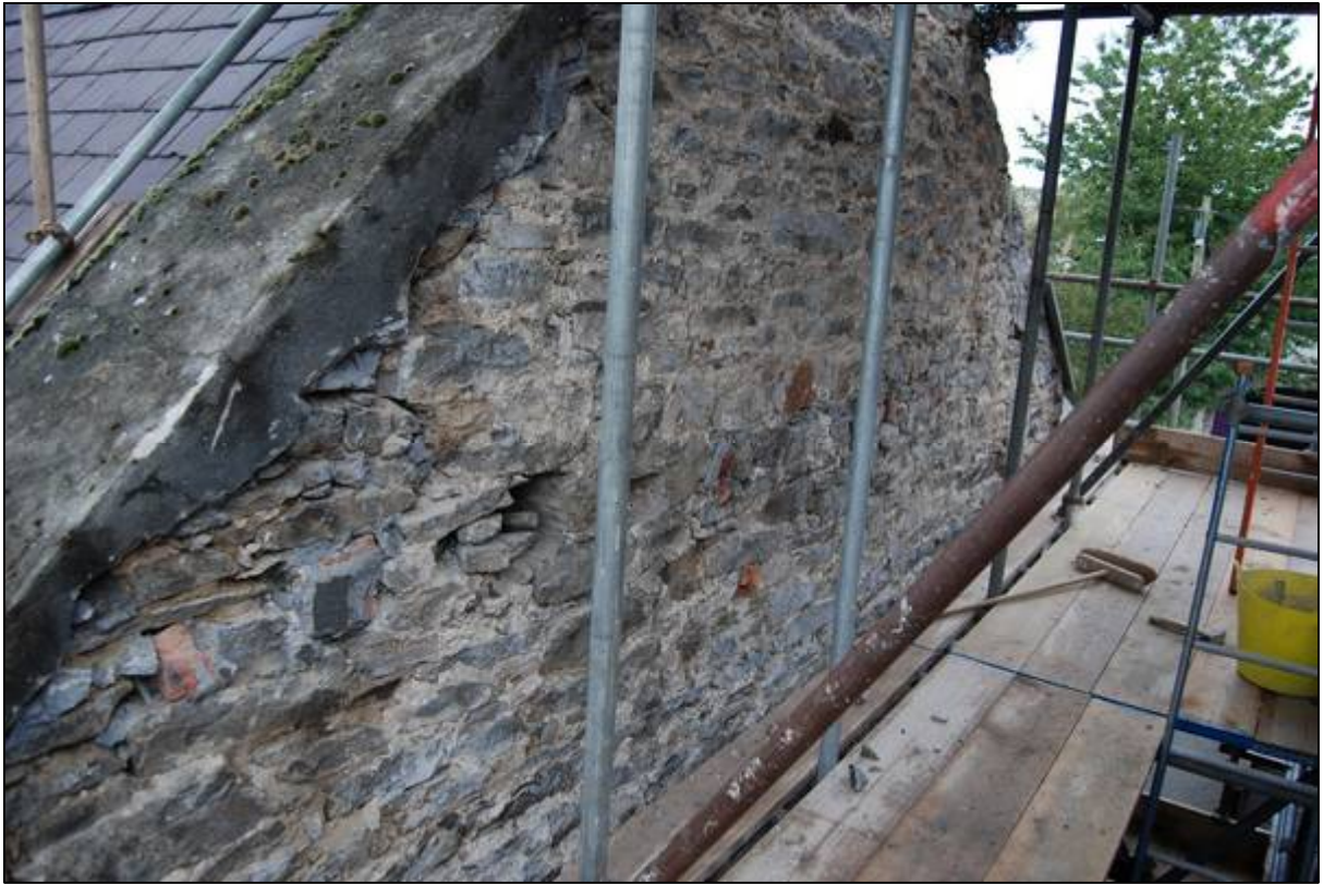
Plate 3: Sockets for joists in the SE Gable
