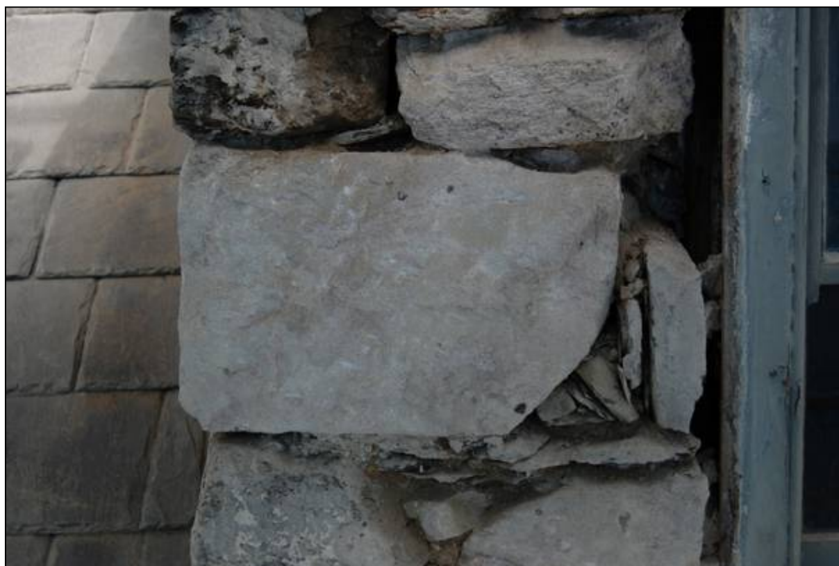
Plate 22: Shaped block in the dormer above the front door
