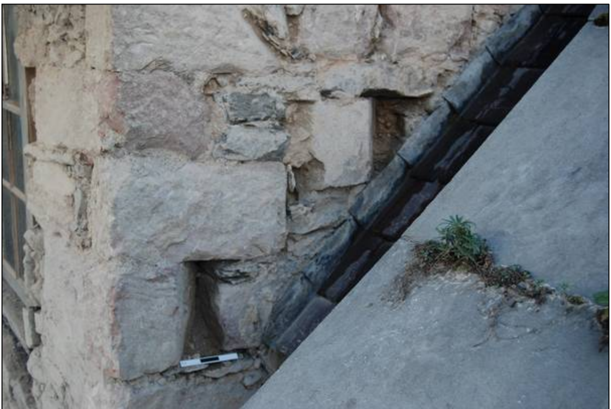
Plate 20: Shaped blocks in the southern face of the southern bay
