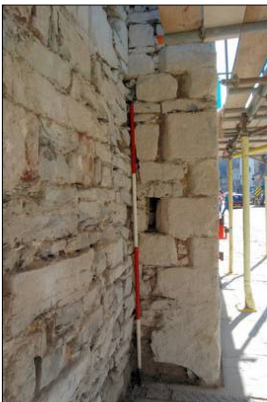
Plate 8: “Squint window” in the ground floor of the northern face of the southern bay
