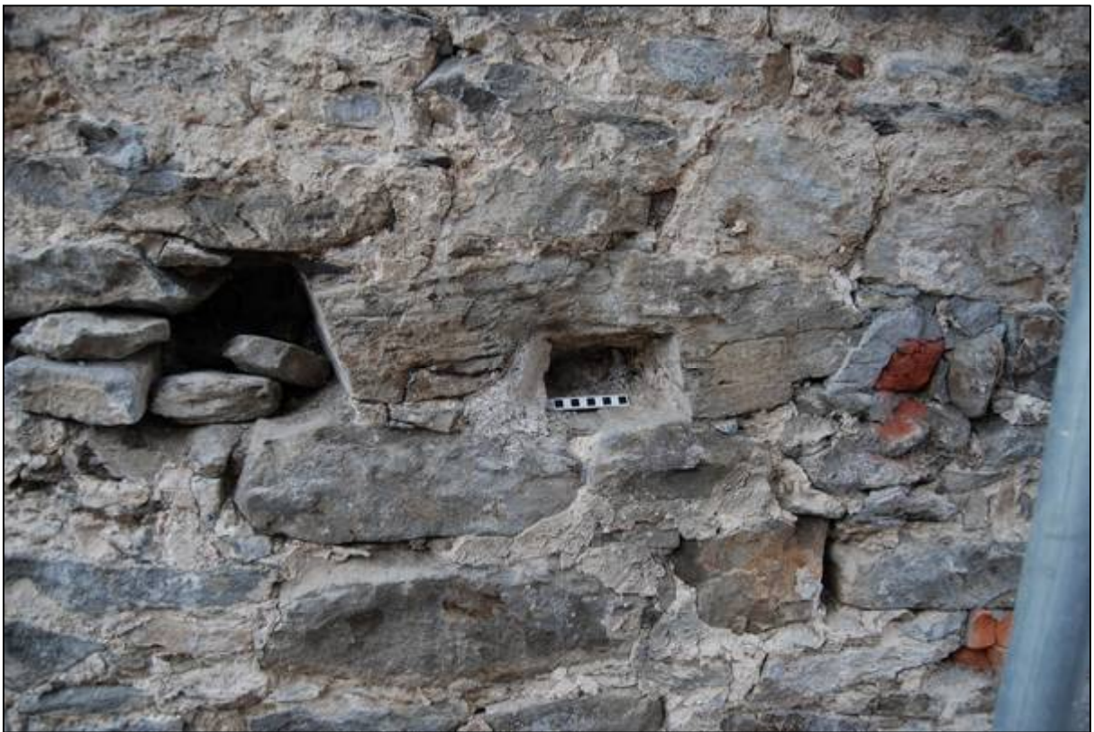
Plate 4: Detail of joist sockets
