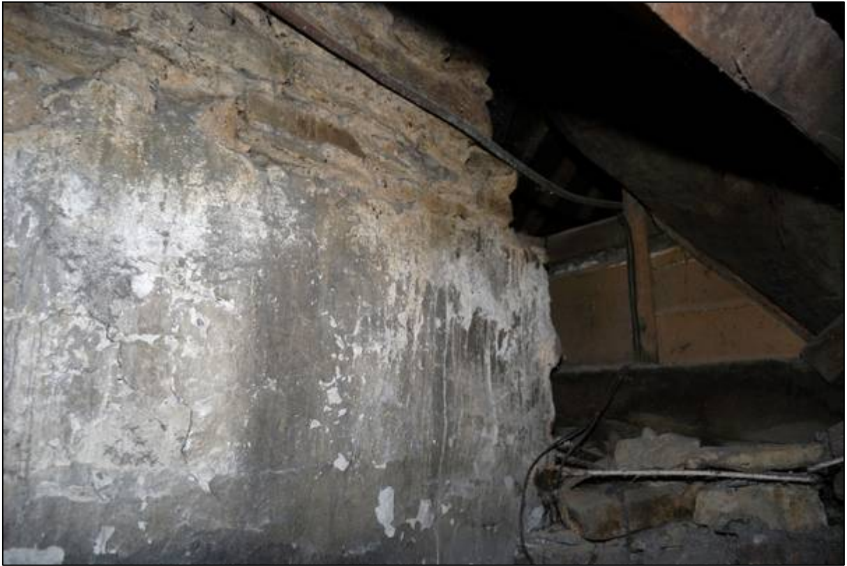
Plate 47: Plaster on the northern side of the chimney
