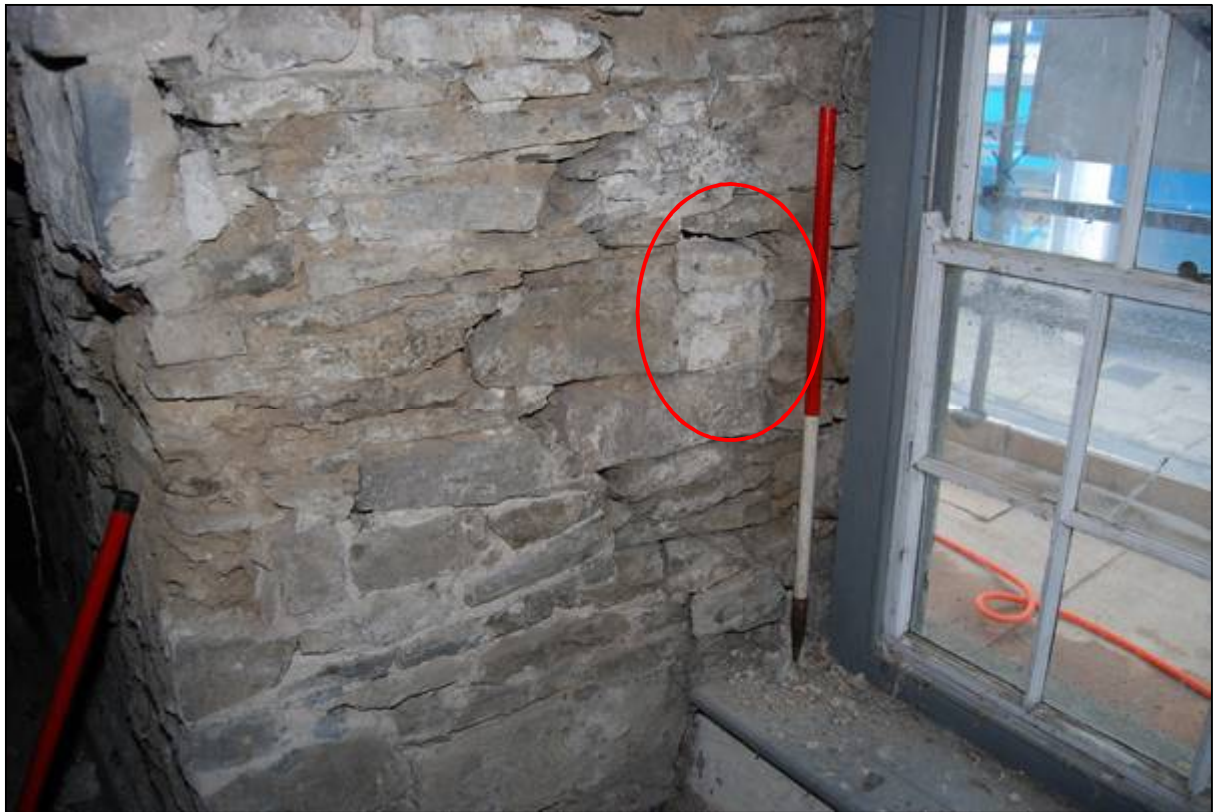
Plate 15: Internal blocking of the “squint window” on the first floor of the southern side of the northern bay
