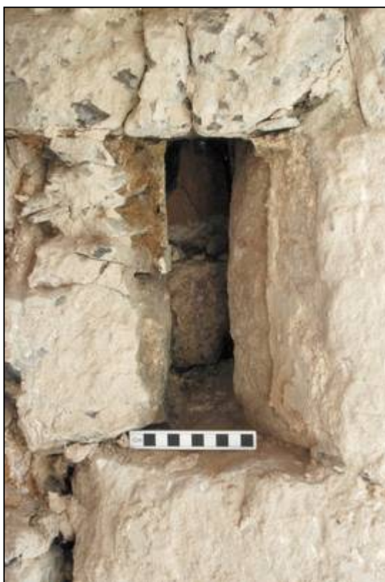
Plate 14: Detail of the “squint window” on the first floor, southern face of the southern bay
