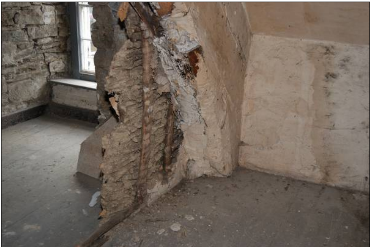
Plate 44: Rear of wattle and daub partition below Truss 1
