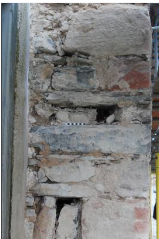
Plate 17: Socket in the northern face of the northern bay
