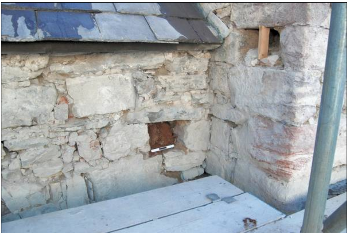
Plate 30: Exposed timber to the south of the front door
