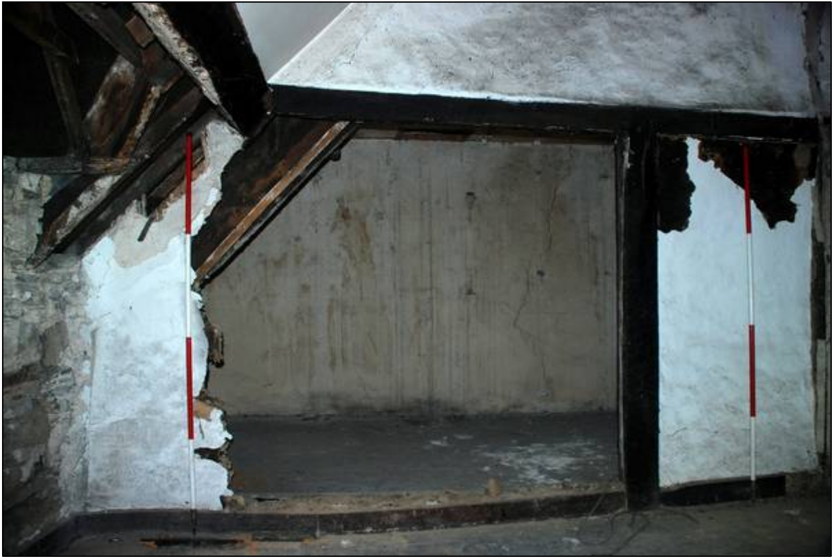
Plate 41: The wattle and daub partition below Truss 1
