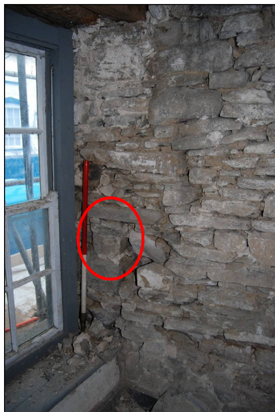
Plate 16: Internal blocking of the “squint window” on the first floor of the northern side of the northern bay
