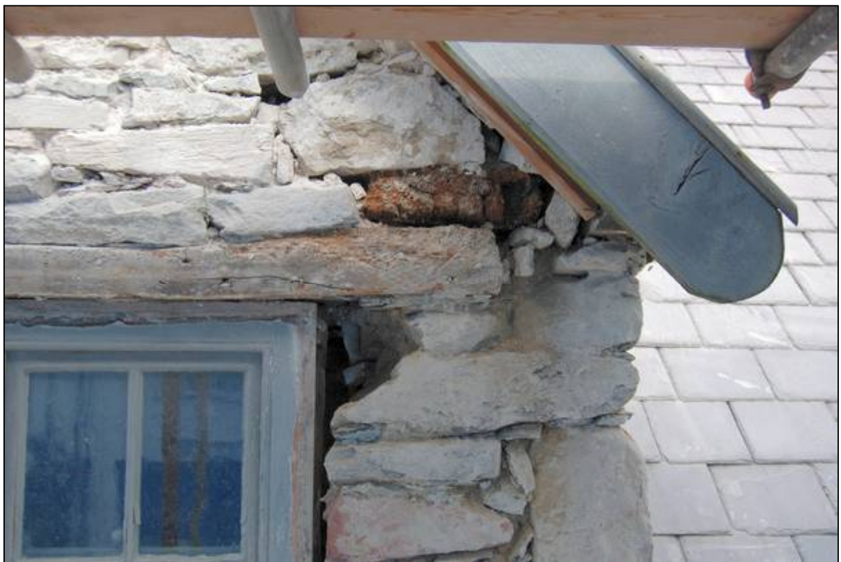
Plate 26: Exposed purlin in the gable of the southern bay
