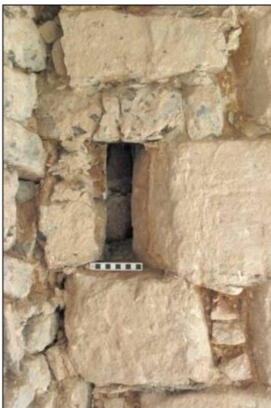
Plate 21: Shaped blocks forming the lower “squint window”, northern face of the southern bay
