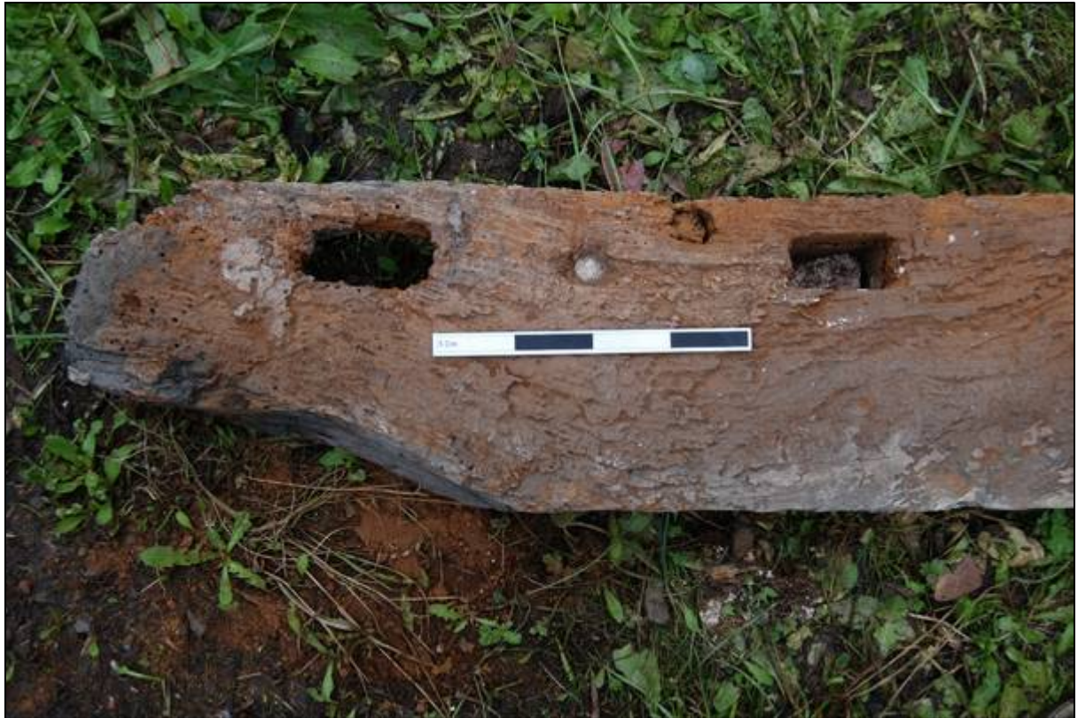
Plate 25: Detail of mortise holes and dowel hole in the re-used rail.
