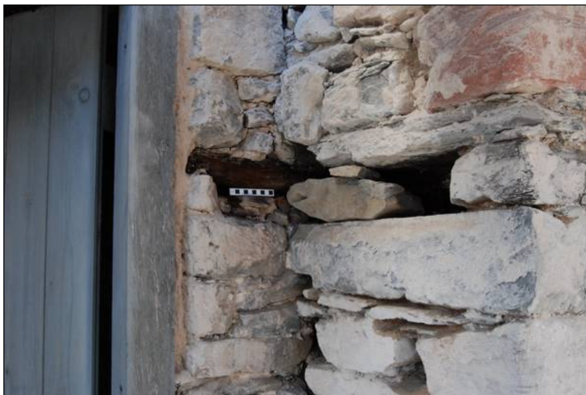
Plate 18: Timber sockets in and near the northern face of the northern bay
