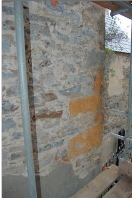
Plate 1: Re-used blocks incorporated within the SE Gable
