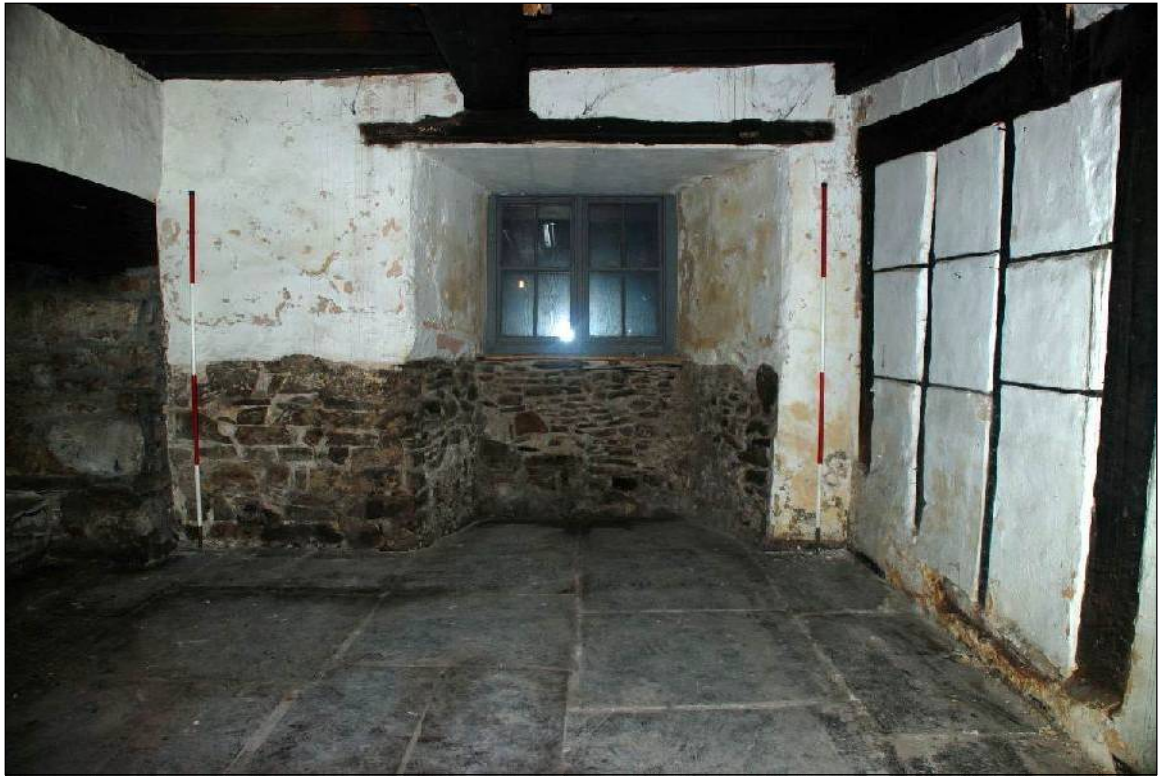
Plate 21: Room 1 bay window
