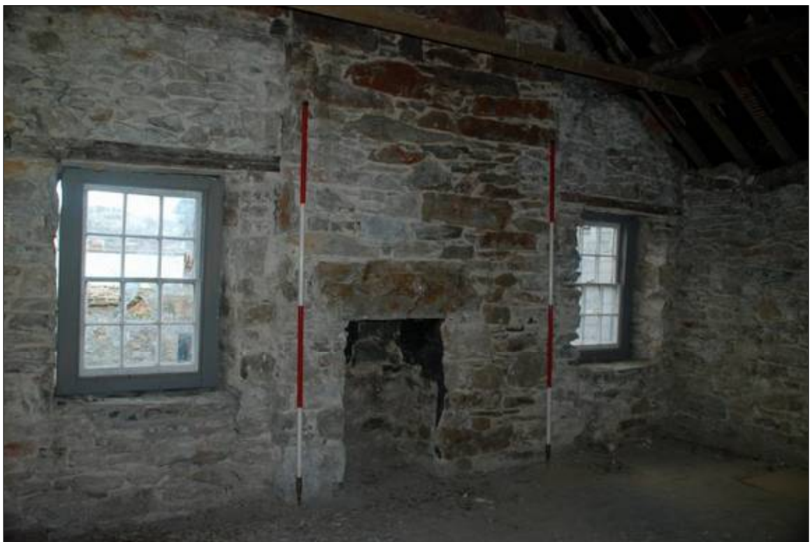
Plate 76: Room 6, chimney and fireplace
