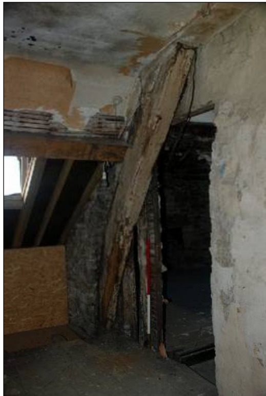
Plate 48: Truss 1, rear principal rafter
