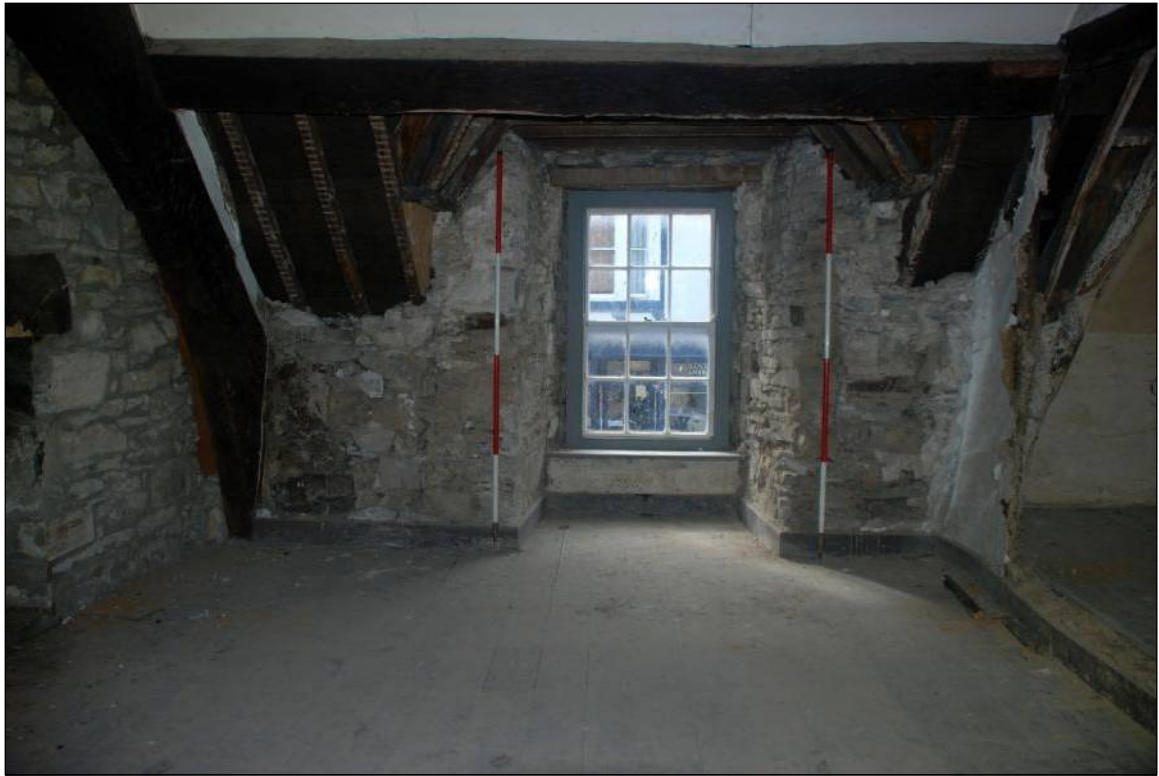
Plate 63: Bay window in the front of Room 4
