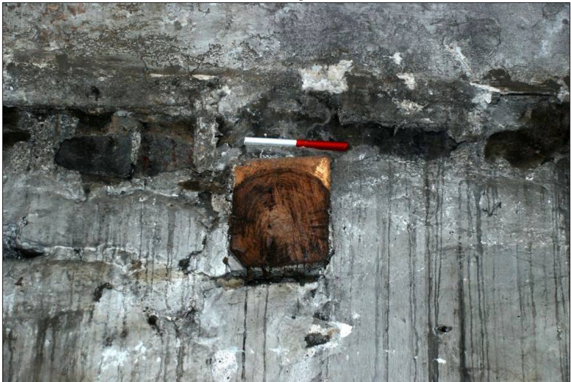
Plate 108: Sawn off beam in the Service Range
