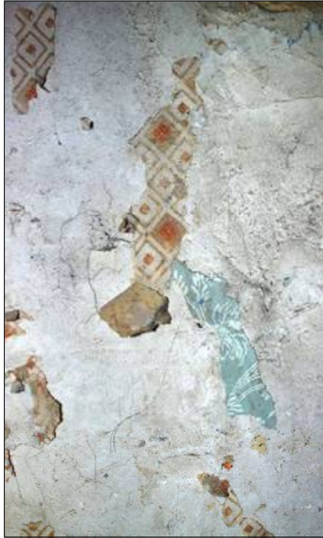
Plate 53: Wall paper on the partition below Truss 1
