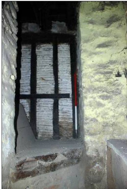
Plate 26: Cupboard behind the chimney in Room 2
