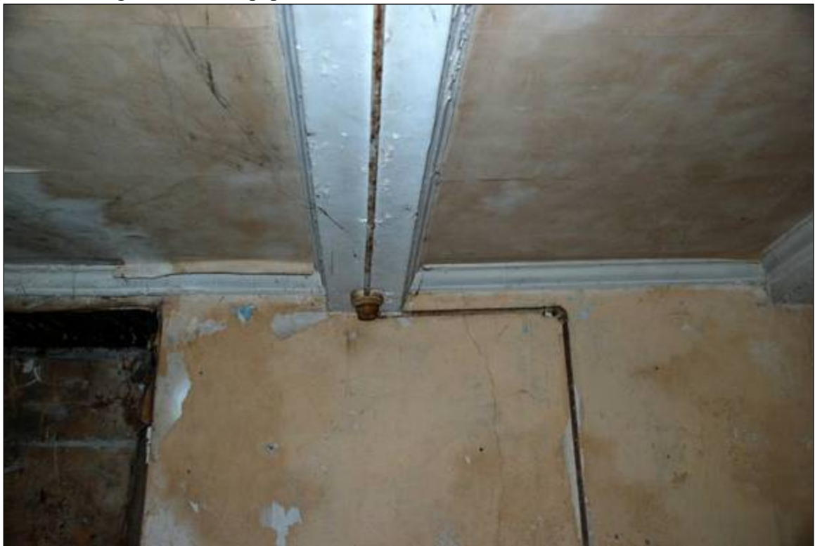
Plate 92: Ceiling beam in Room 8
