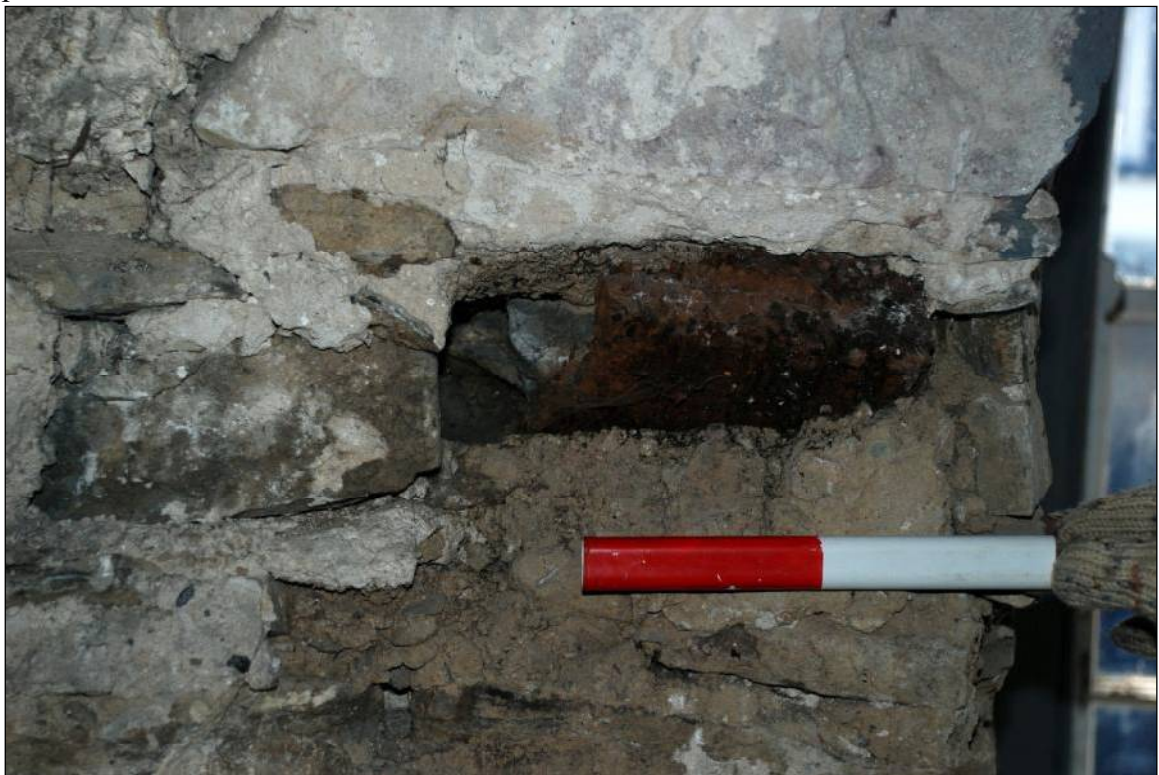
Plate 58: Sawn off common rafter embedded in the front wall
