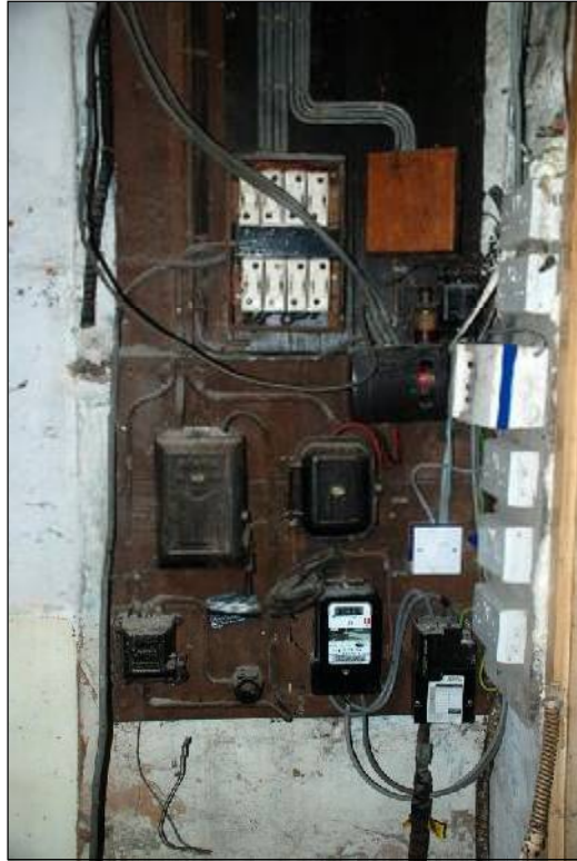
Plate 27: Electricity panel in Room 2
