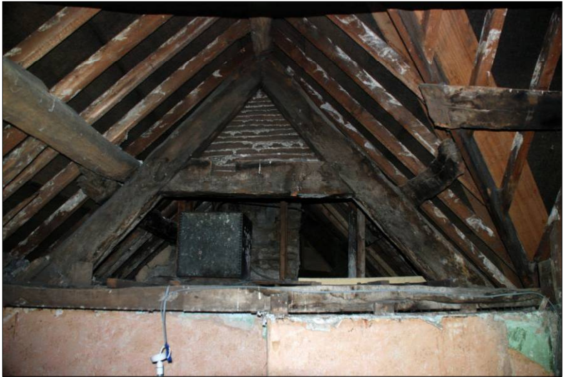
Plate 67: Staggered overlap on upper front purlin in Room 5
