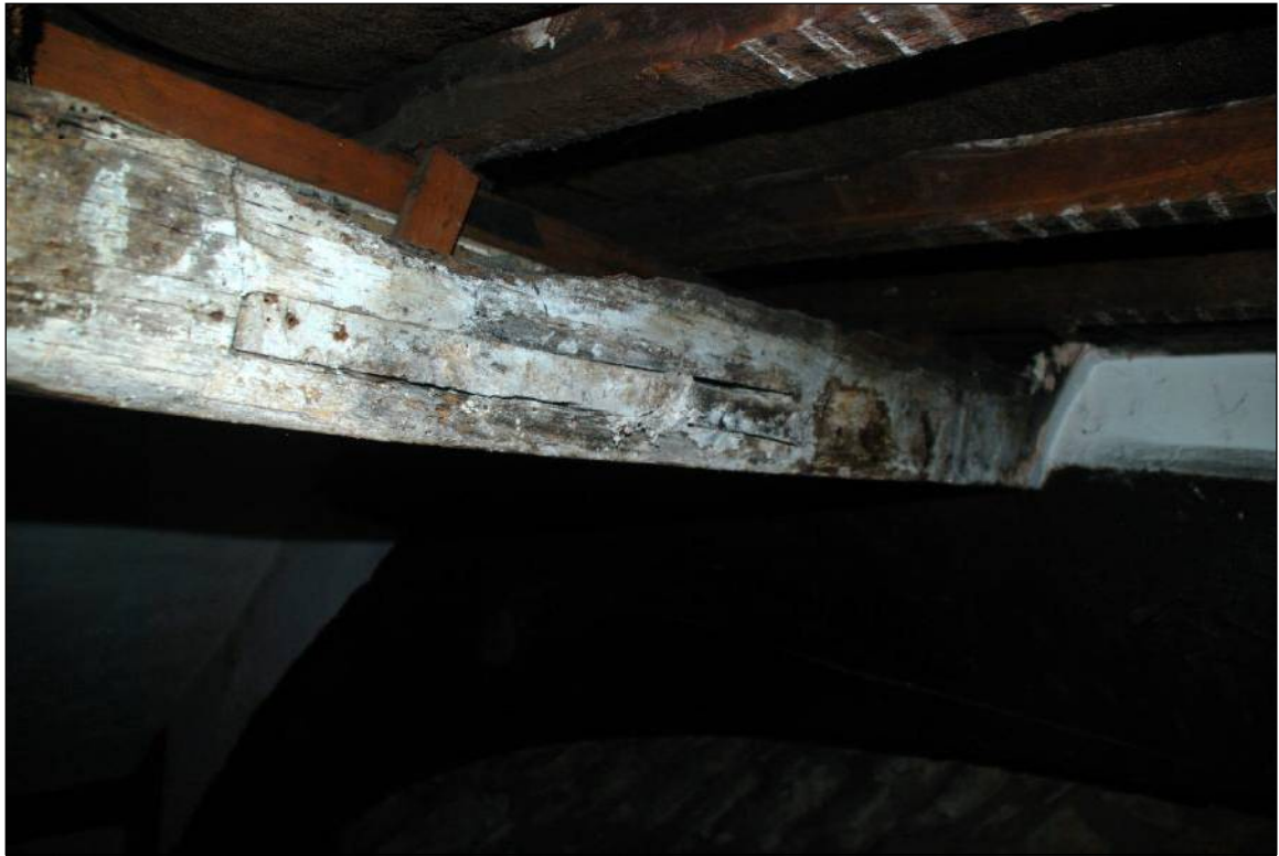
Plate 57: Tenon showing position of windbrace between Truss 2 and the lower front purlin
