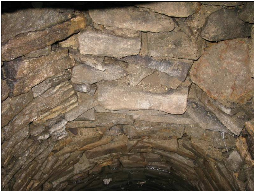
Plate 40: Patch in the top of the well
