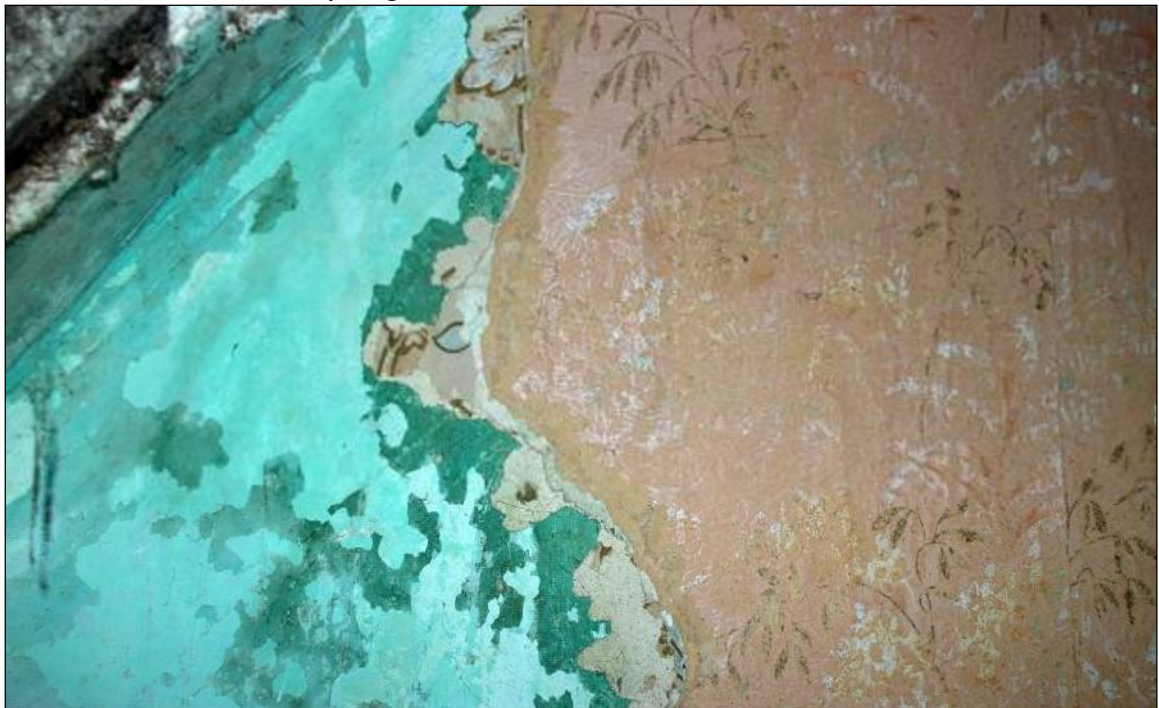
Plate 74: Wallpaper surviving on partition wall between Rooms 5 and 7
