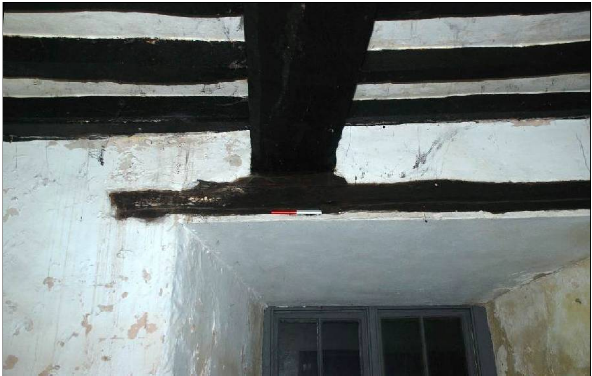
Plate 18: End of main beam in Room 1 over the bay window
