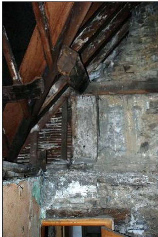
Plate 72: Relationship between the stud and purlin above the chimney in Room 5
