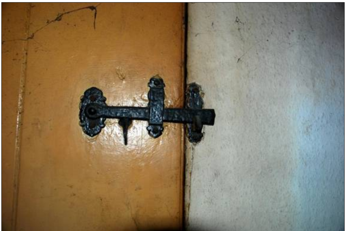
Plate 100: Drop catch on the Attic door
