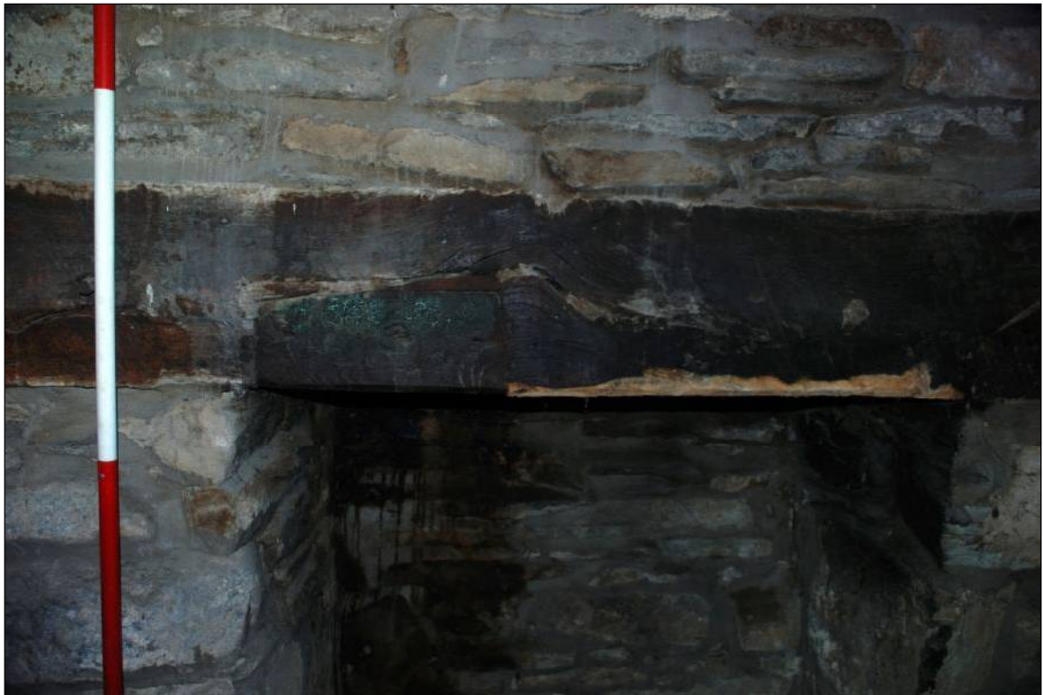
Plate 60: Repair to the lintel above the fireplace in Room 4
