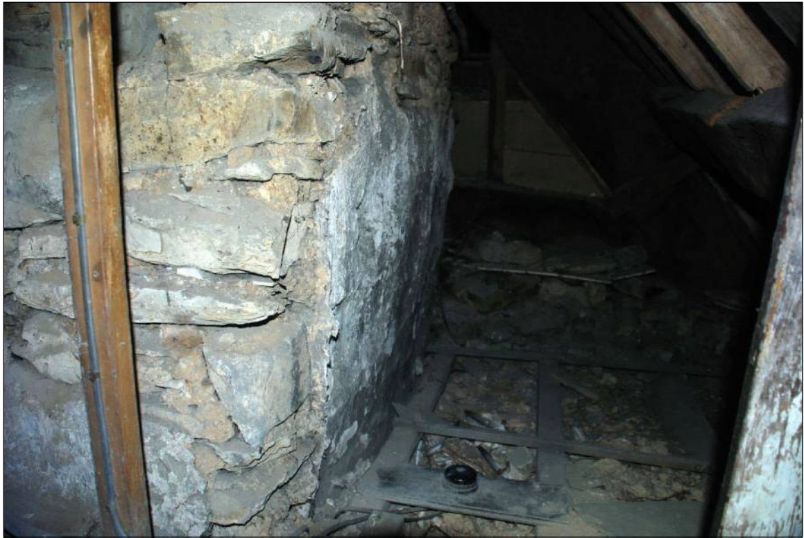
Plate 81: Plastered face of the chimney stack above Room 7 showing lip
