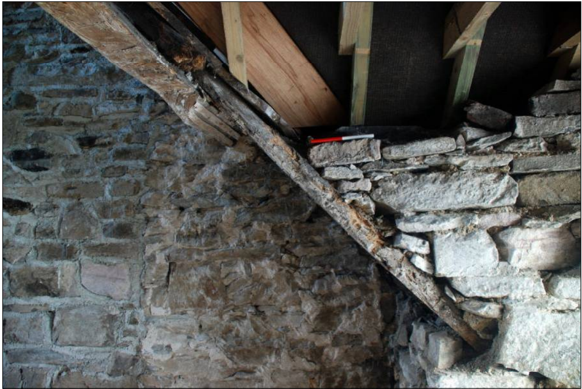
Plate 69: Common rafter adjacent to the bay window in Room 5
