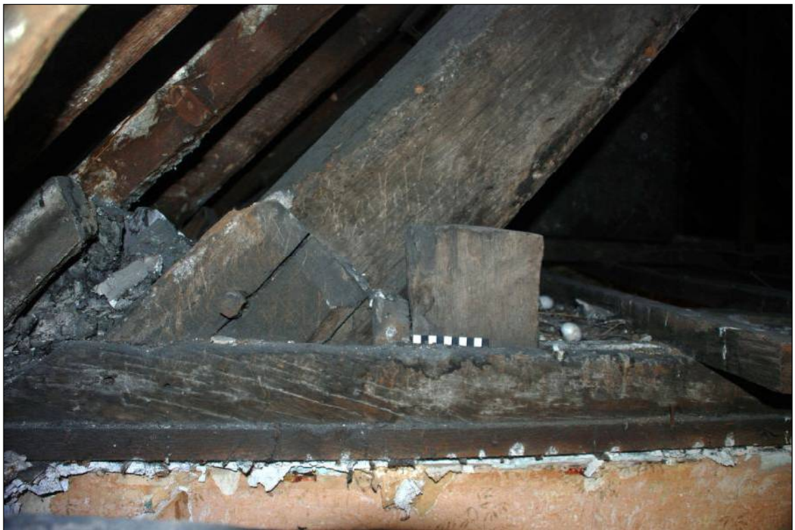
Plate 66: Repair to Truss 3
