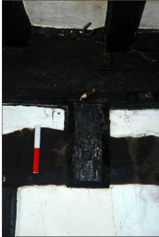
Plate 17: Filler between the partition and the ceiling beam in Room 1
