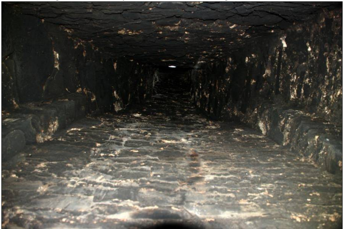
Plate 110: View up the chimney flue in the Service Range
