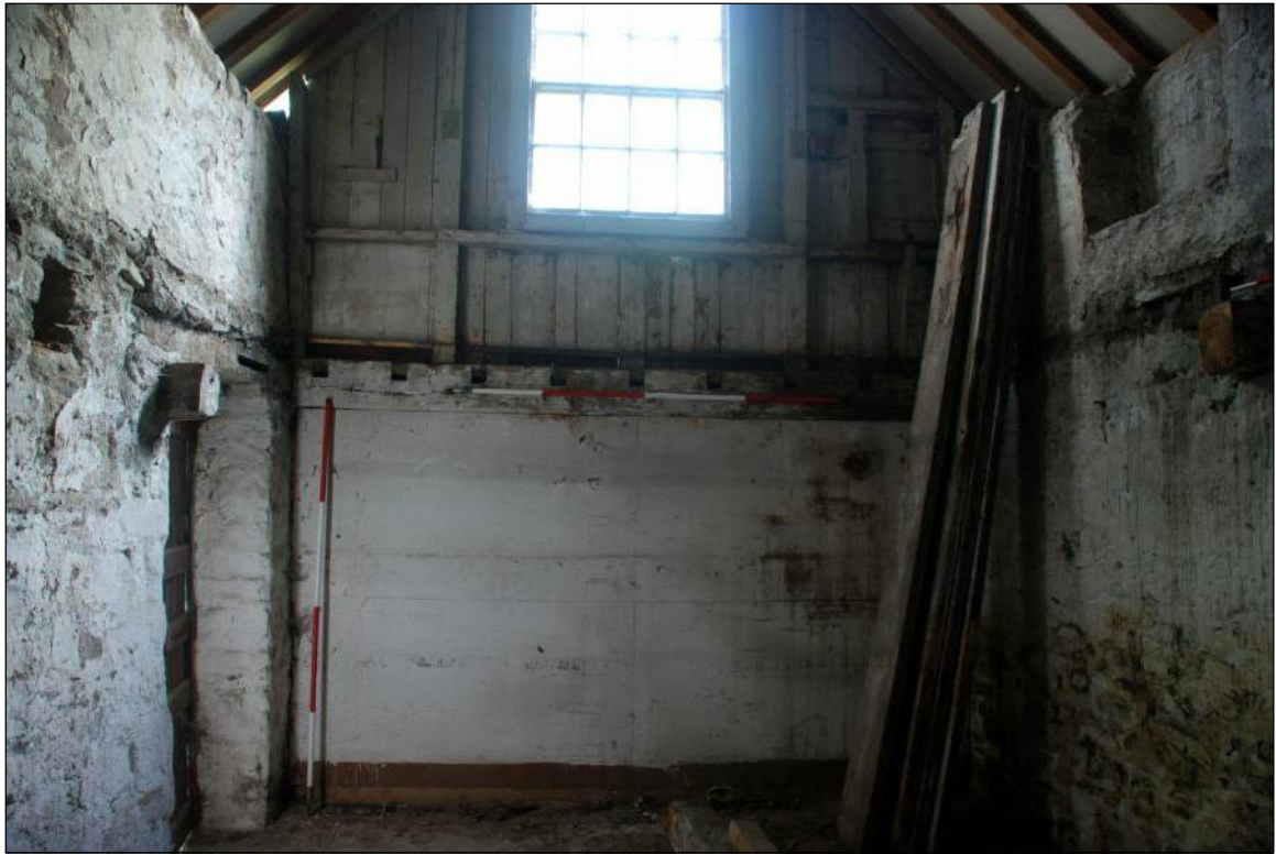
Plate 107: The northern end of the Service Range
