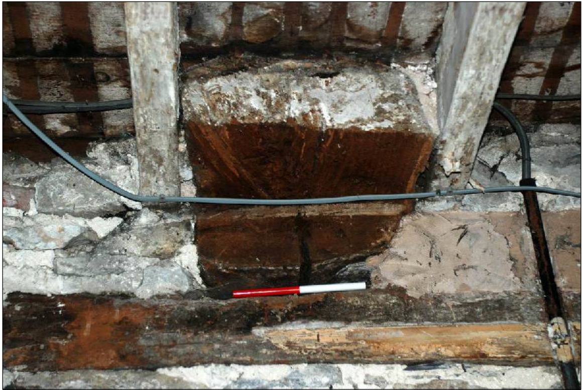
Plate 19: End of Room 1 main beam in New Kitchen
