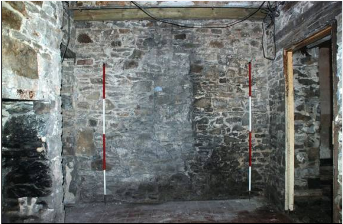
Plate 37: Blocked window in eastern wall of the New Kitchen
