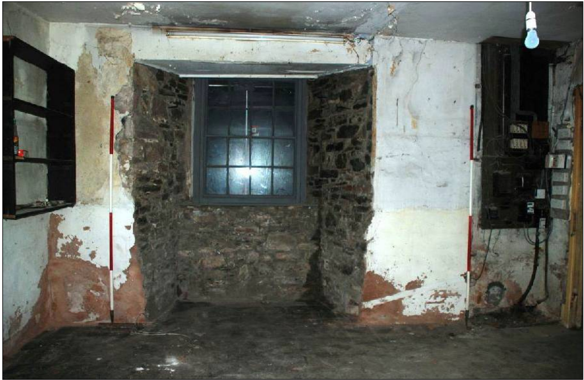
Plate 23: Room 2, bay window
