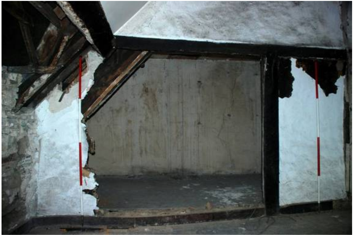
Plate 51: The partition below Truss 1
