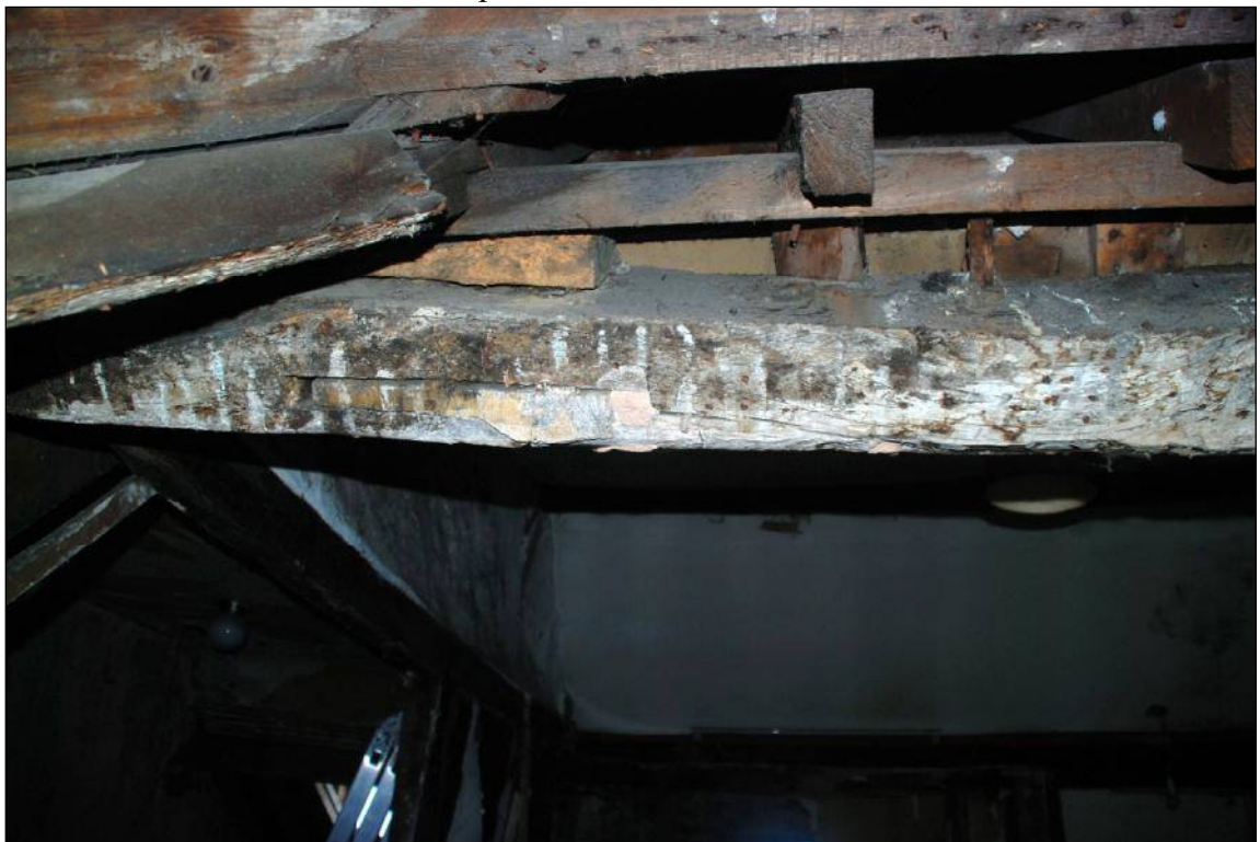
Plate 49: Peak of Truss 1 in roof space over Room 4
