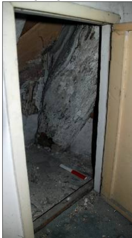
Plate 106: Eastern principal rafter in the Attic
