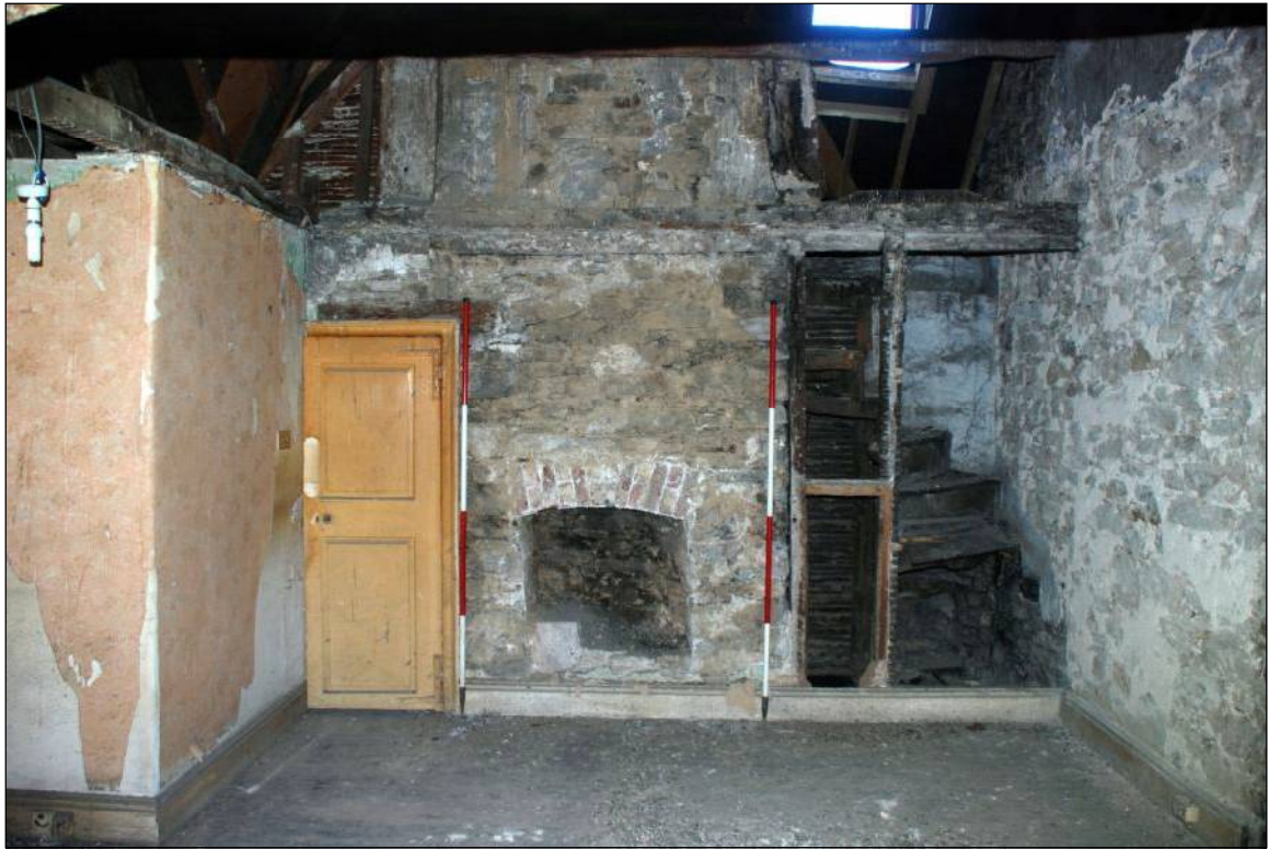
Plate 71: Chimney on north side of Room 5
