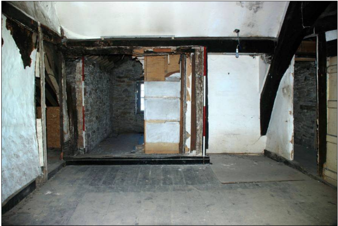
Plate 61: Room 4 looking north
