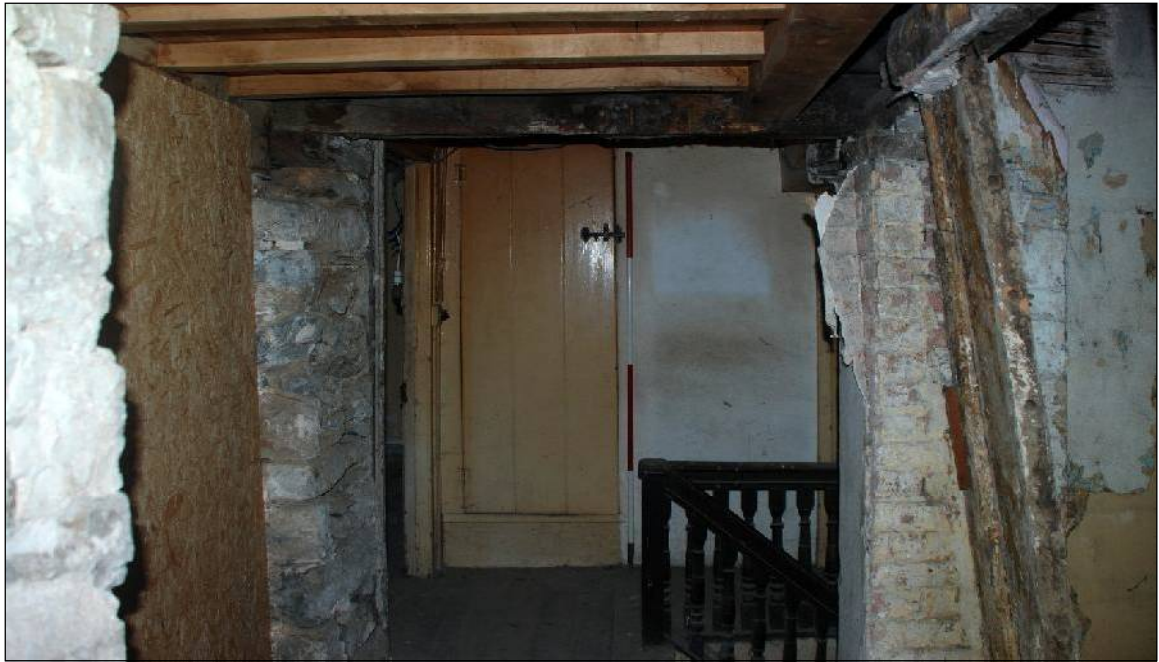
Plate 99: The door to the Attic stairs
