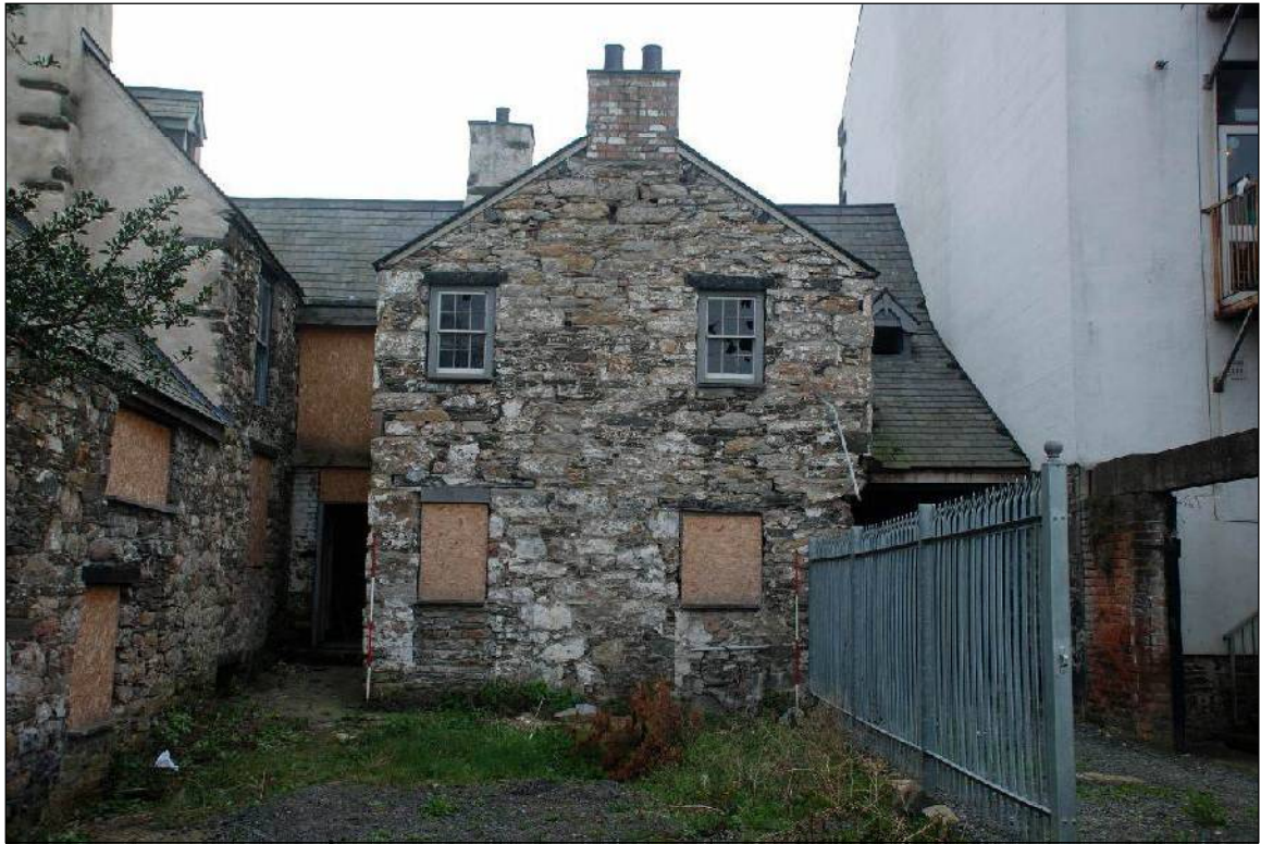
Plate 13: New Kitchen range.
