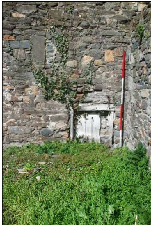
Plate 114: Blocked opening in the western wall of the garden
