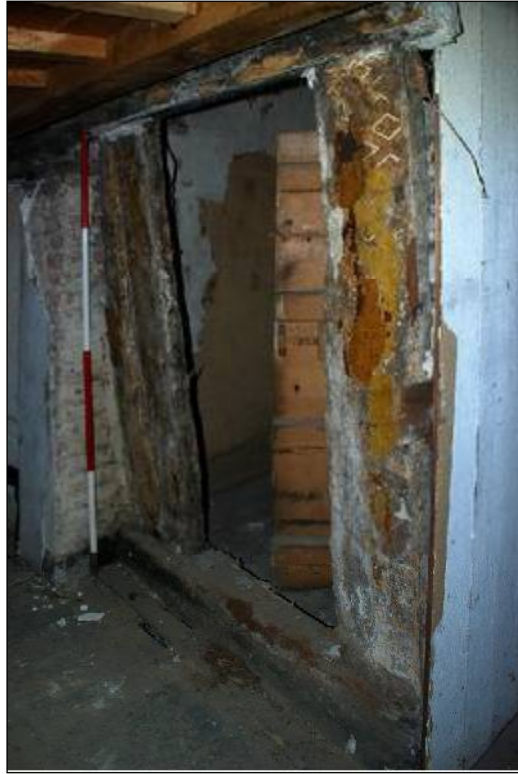
Plate 83: Planking partition wall for Room 7, viewed from the Landing corridor
