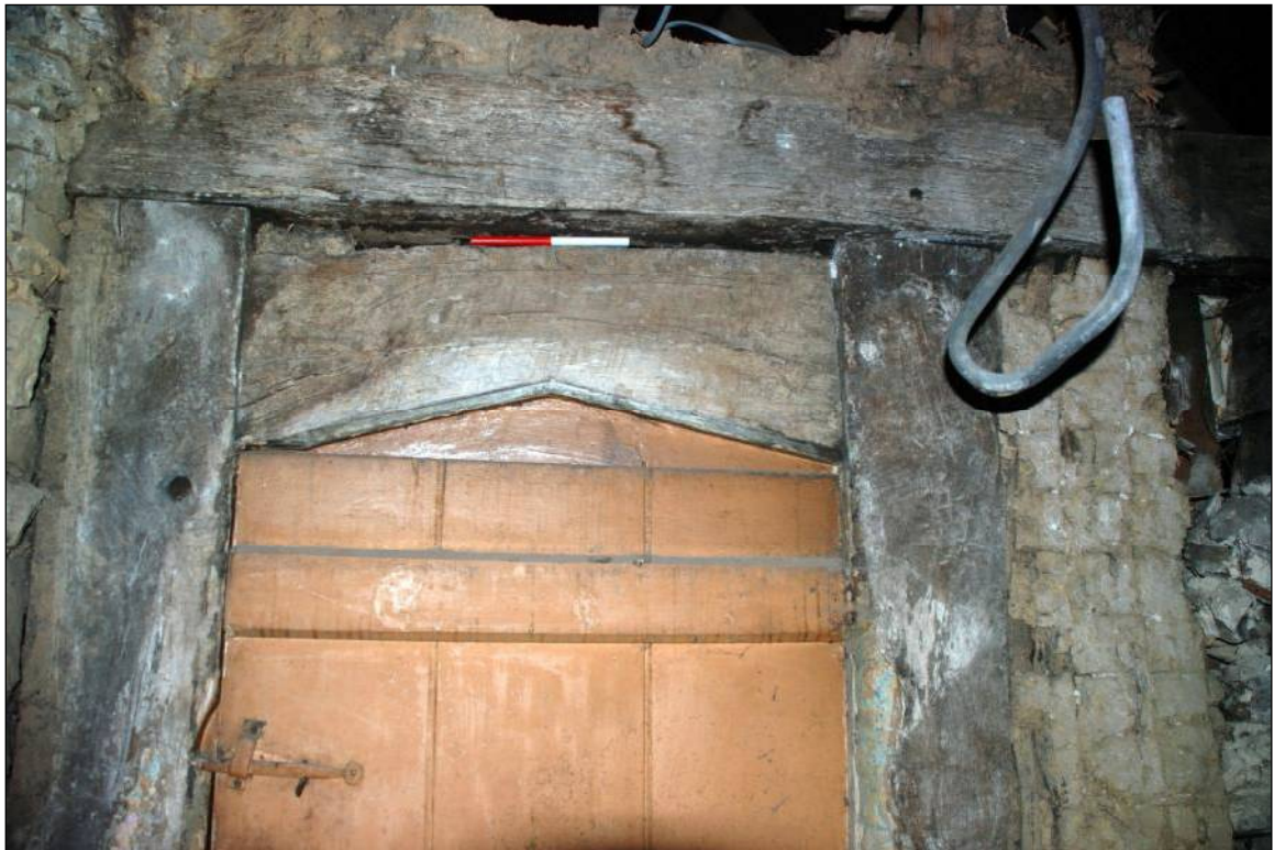
Plate 78: Door head over door to Room 7
