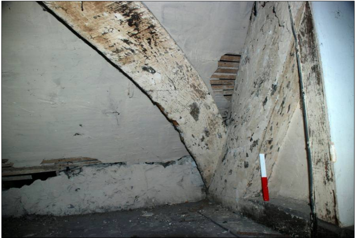
Plate 105: Windbrace and western principal rafter in the Attic
