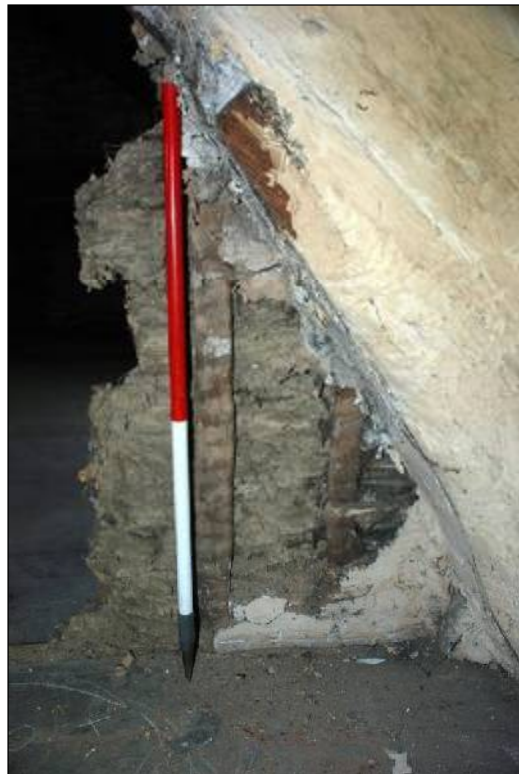
Plate 52: Detail of wattle and daub partition below Truss 1
