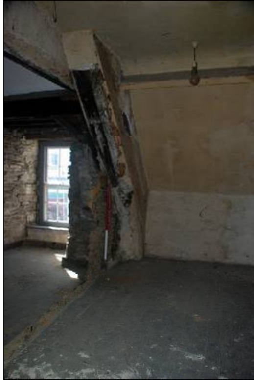
Plate 47: Truss 1, front principal rafter
