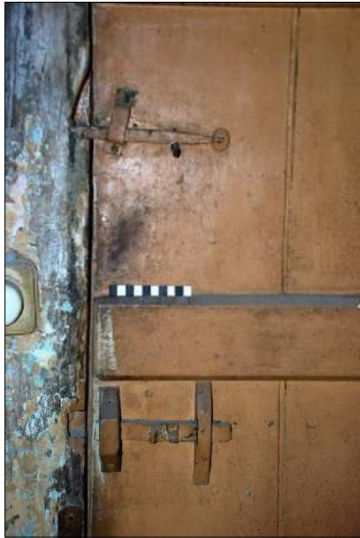
Plate 79: Latches on door to Room 7
