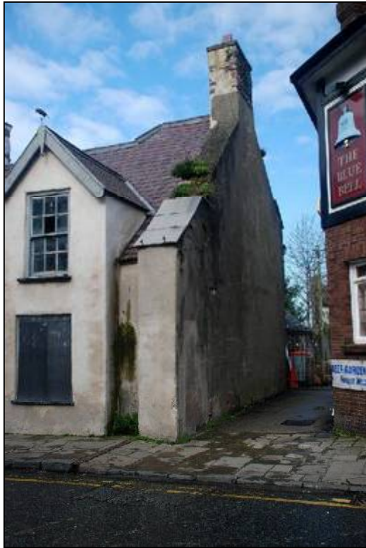
Plate 9: Projecting wall on the eastern gable wall
