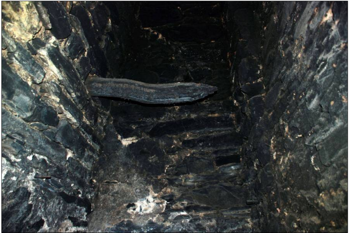
Plate 111: Timber in the flue of the Service Range
