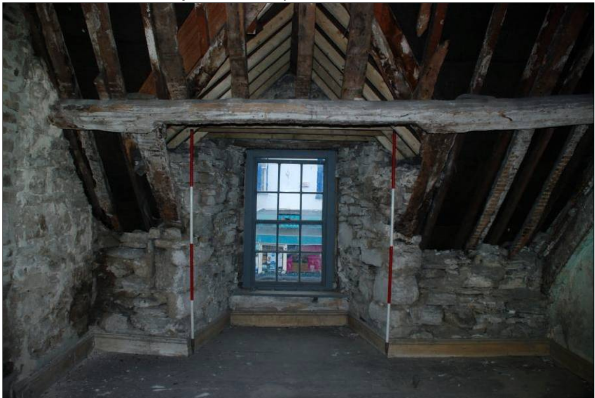
Plate 70: Bay window in Room 5
