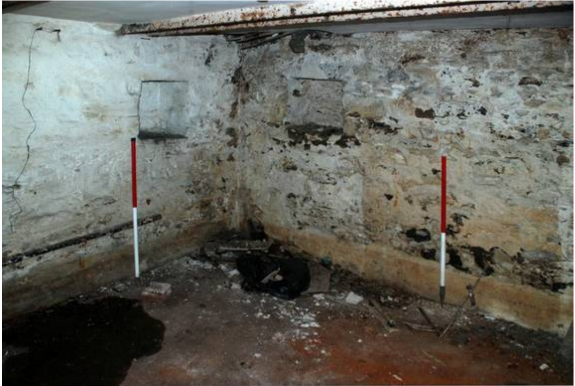
Plate 45: North east corner of the Cellar showing two of the recesses
