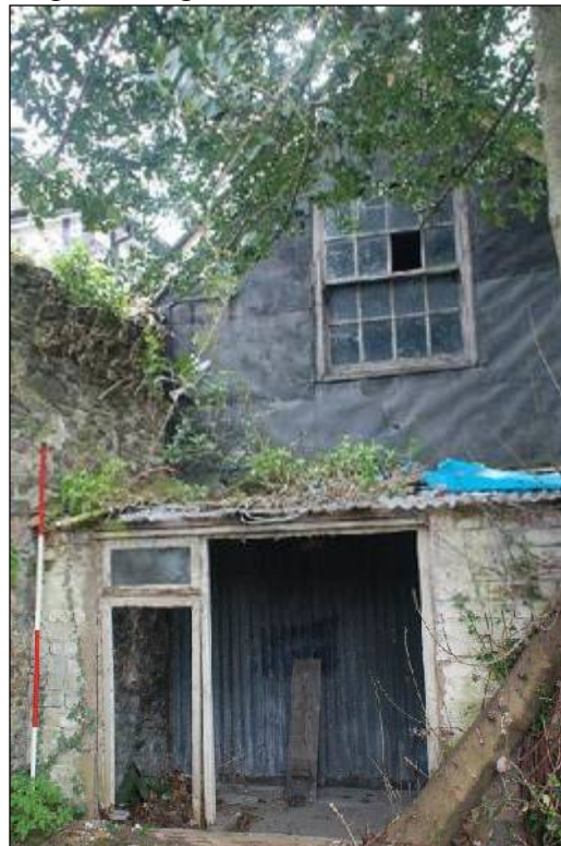
Plate 12: Lean-to at the northern end of the Service Range
