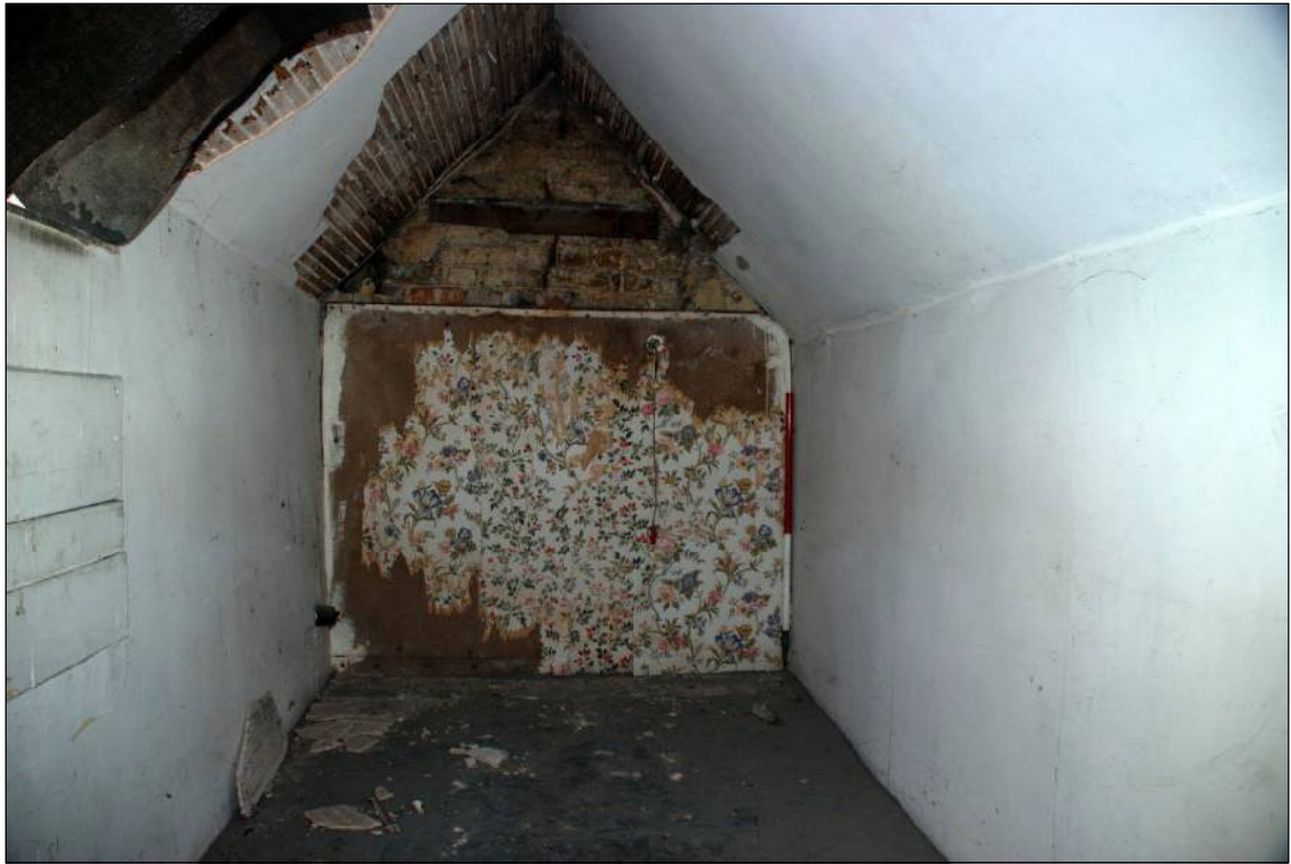
Plate 101: The Attic looking north
