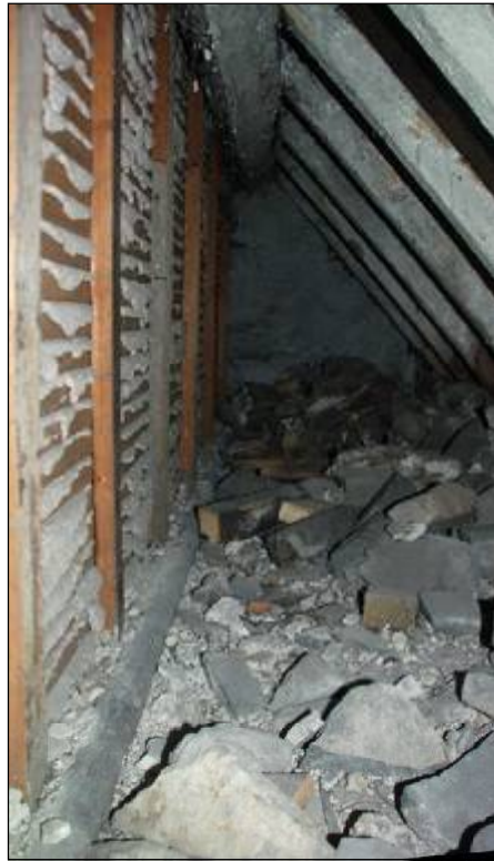
Plate 103: Eastern space between the partition and the roof in the Attic
