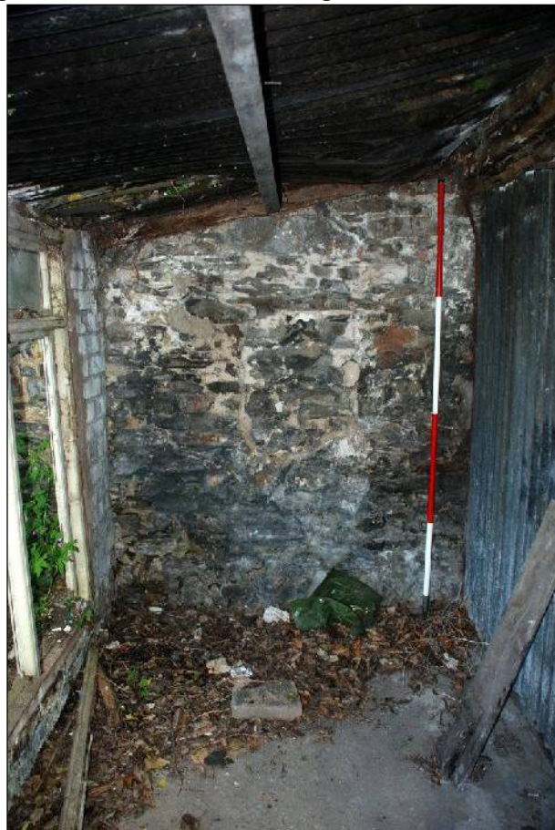
Plate 116: Blocking in the eastern wall, within the Lean-to
