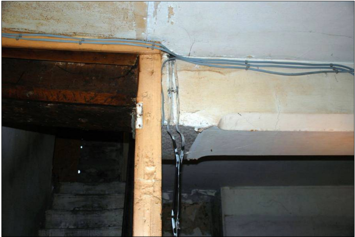
Plate 25: Ceiling beam in Room 2
