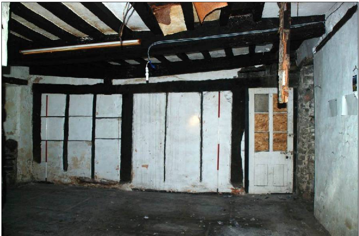
Plate 16: Room 1, wood and brick partition
