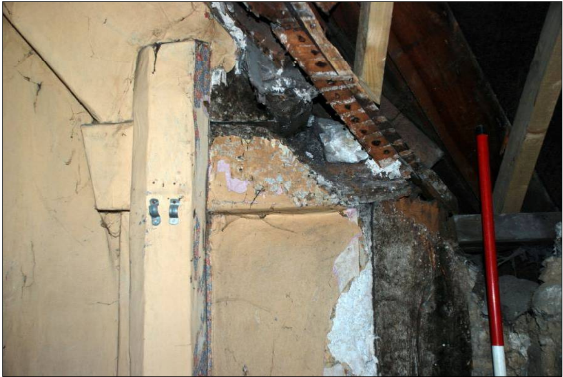
Plate 85: Base of Truss 3, Room 7
