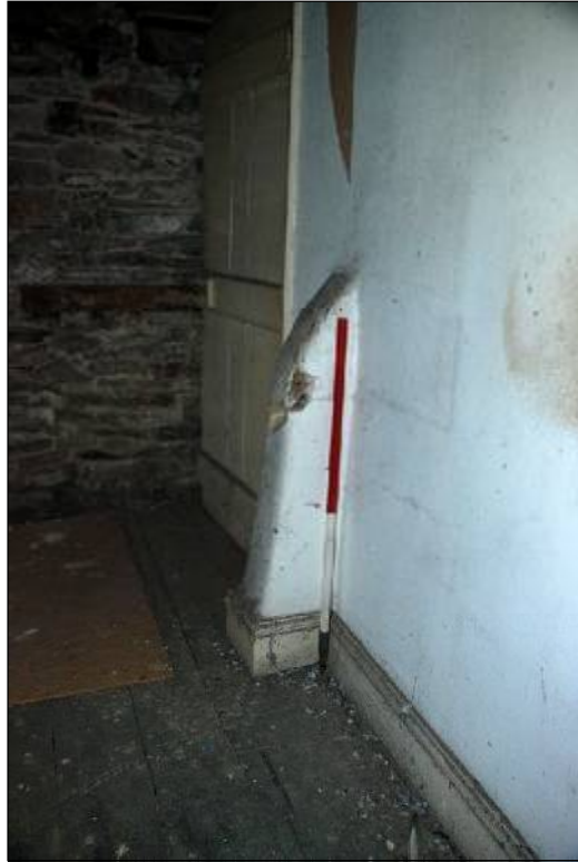
Plate 77: The northern end of Truss 2 protruding through the wall between Rooms 4 and 6
