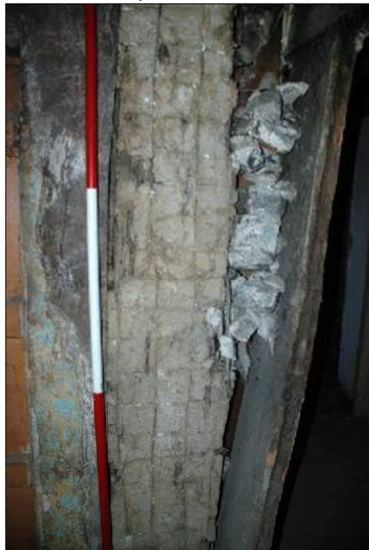
Plate 81: Plastered face of the chimney stack above Room 7 showing lip
