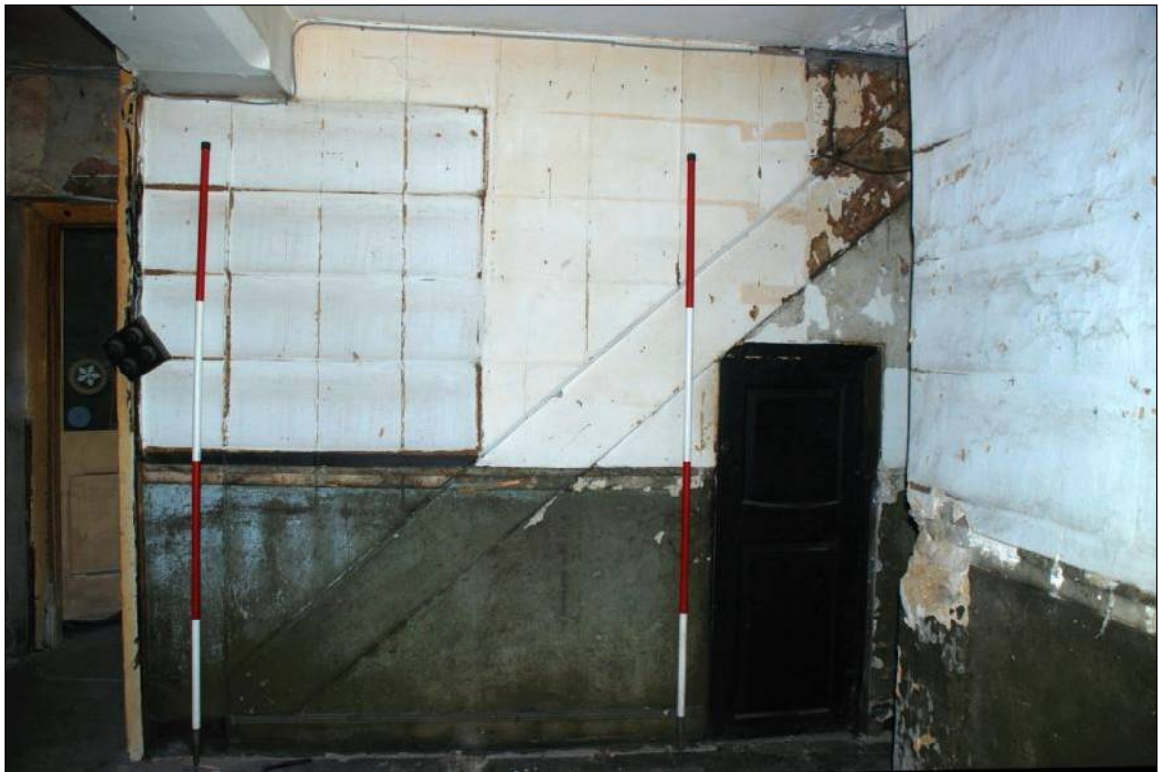
Plate 24: Paneling for staircase in Room 2
