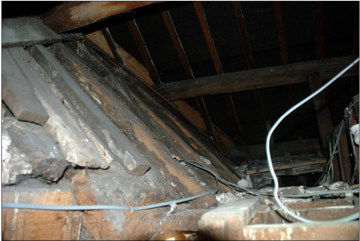
Plate 59: Old roofline above the rear of Room 4
