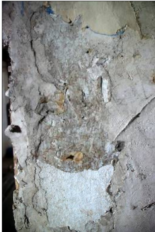
Plate 54: Wall paper on partition below Truss 1
