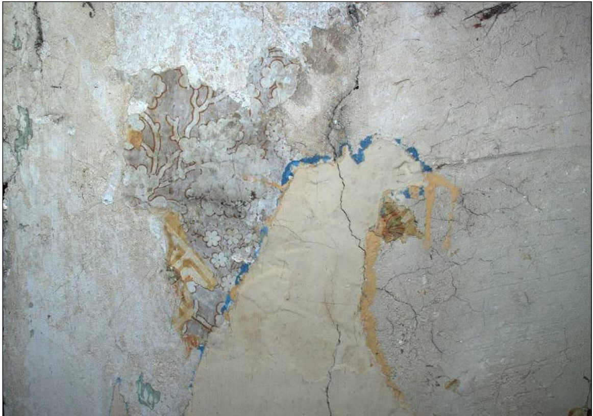
Plate 55: Wall paper on partition below Truss 1
