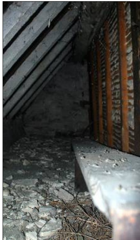
Plate 102: Western space between the partition and the roof in the Attic
