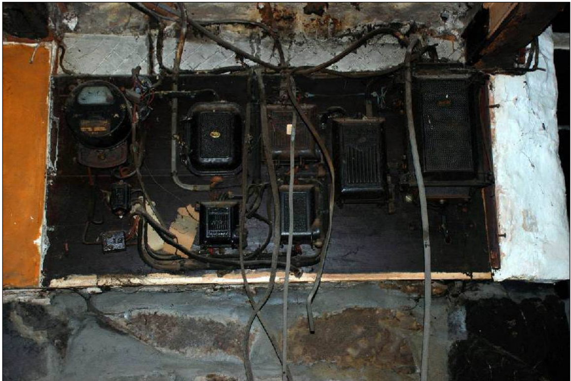
Plate 22: Room1 electrical panel
