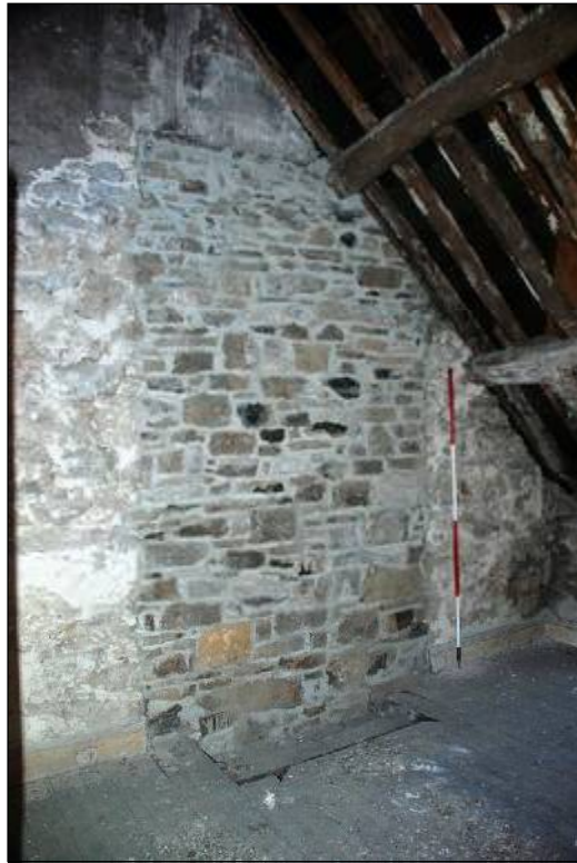
Plate 73: Inserted chimney in gable end of Room 5
