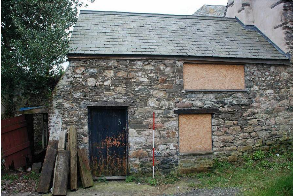
Plate 11: The Service Range looking east
