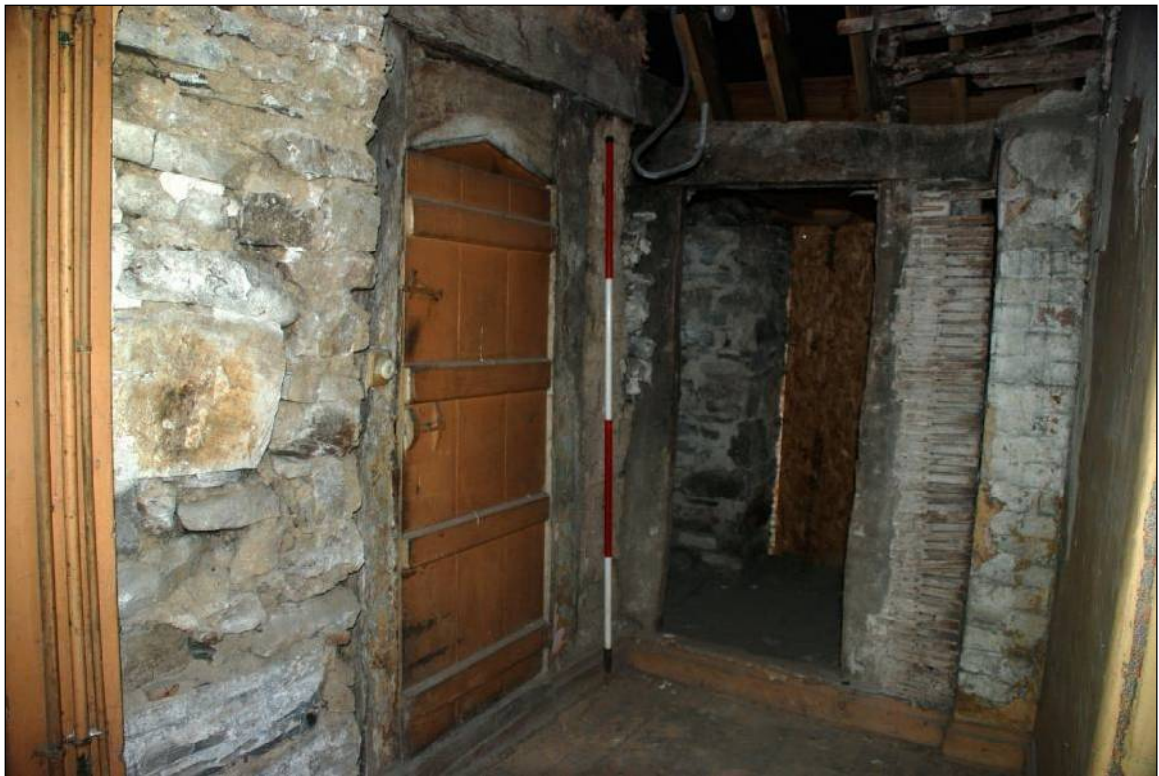
Plate 80: Door, partitions and chimney stack in Room 7
