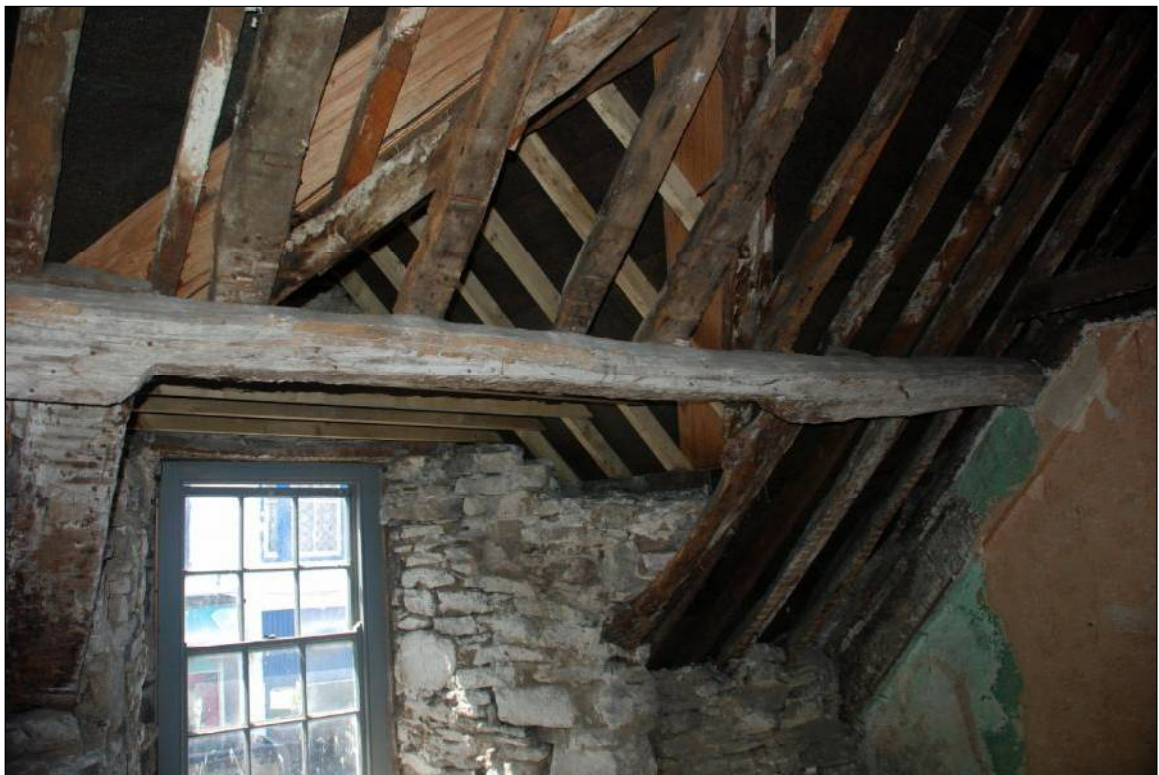
Plate 68: Modification of the lower, front, purlin in Room 5
