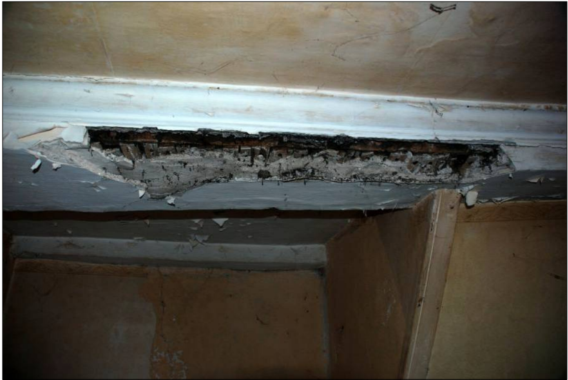
Plate 93: Structure of ceiling beam in Room 8
