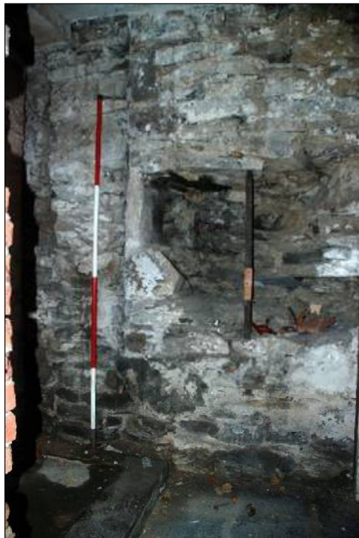
Plate 32: Possible salt box in the Hallway
