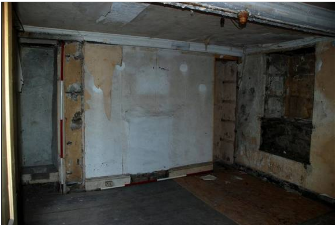
Plate 94: Blocked fireplace in Room 8
