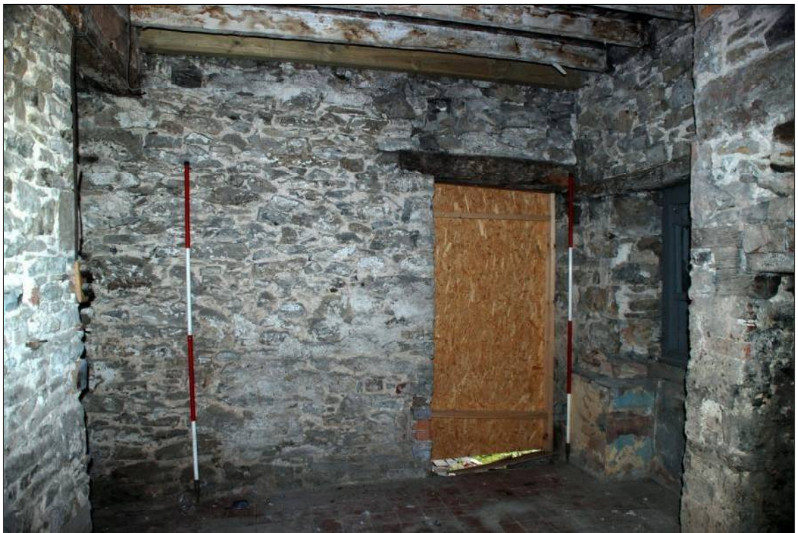
Plate 38: Doorway in western wall of the New Kitchen
