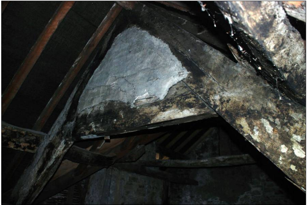
Plate 65: Plastered finish to western side of Truss 3
