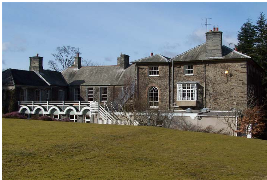
Figure 10: Castell Malgwyn from the south showing the east block and staircase bay to the right, and kitchen block to the left. In the centre is the mid-19 th century 'infill' range, with the 20 th century, single storey, ballroom at the front
