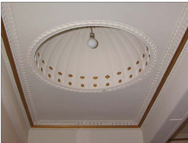
Figure 7: The domed ceiling decoration and cornicing of the c. 1795 dining room
