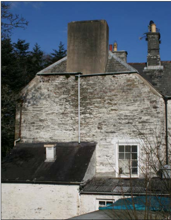
Figure 5: West gable end of the Phase I building showing the steep pitch of the original roof line
