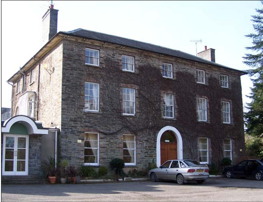
Figure 6: The east elevation of Sir Benjamin Hammet's house, constructed c. 1795 and later refenestrated
