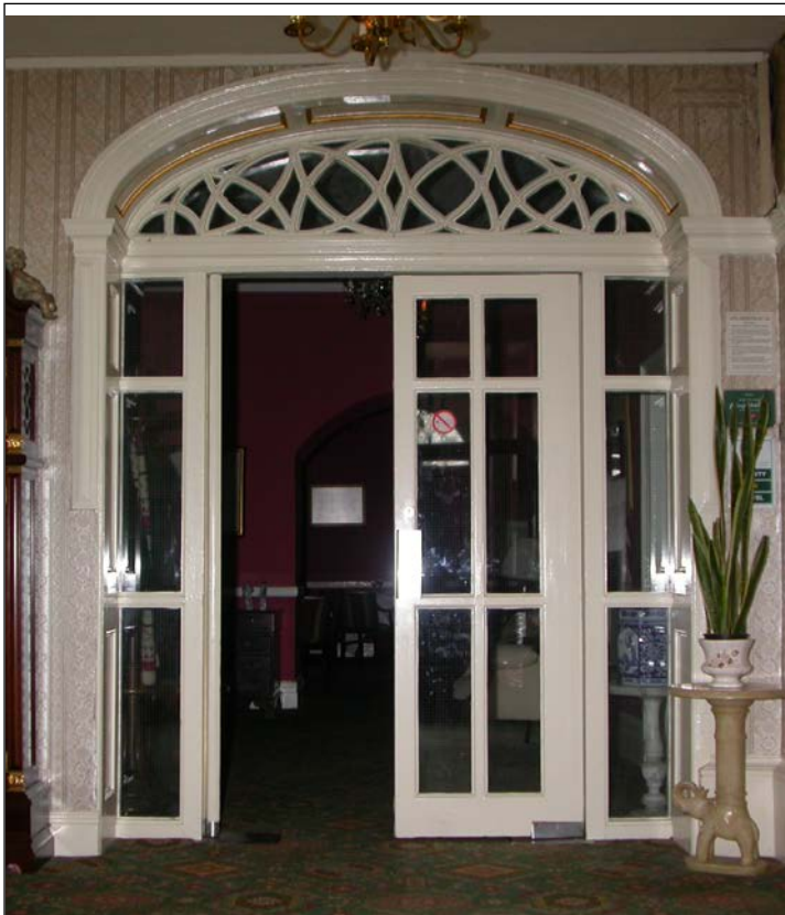
Figure 8: Arched doorway with traceried fanlight at the north end of the hall, probably originally leading out into a courtyard area
