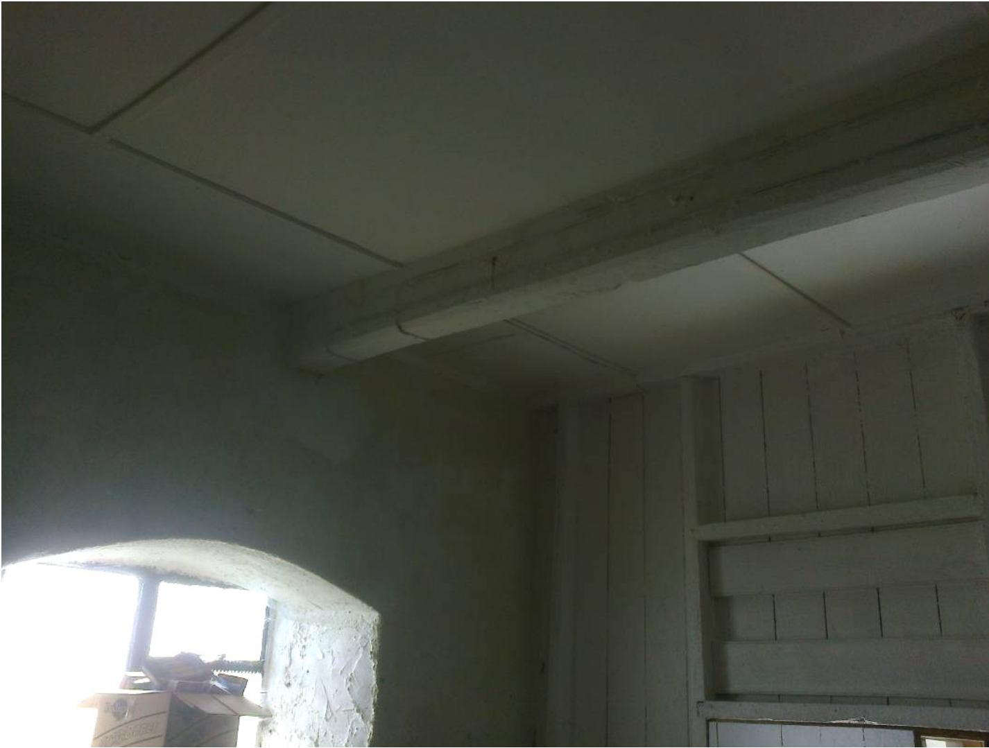
View of curved window head and beam supporting floor over in kitchen store.
