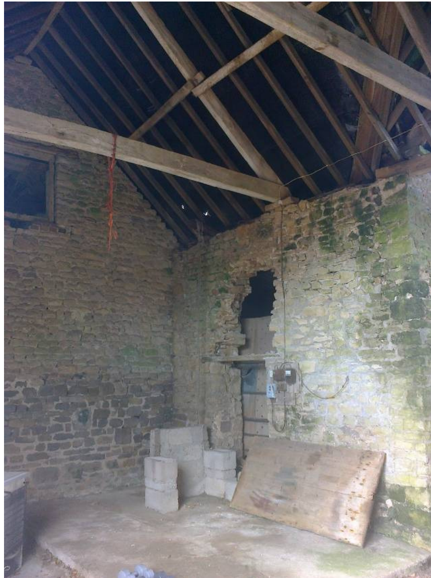
View of roughly formed internal opening between threshing floor and the 1980's extension containing the grain silo.
