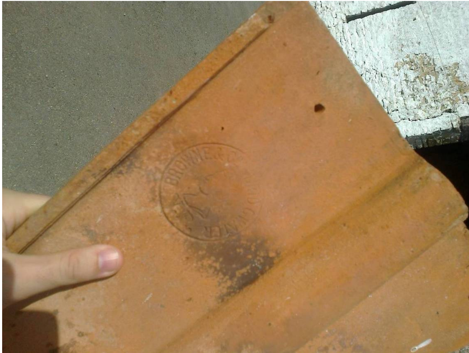
Detail of rear of roof tile showing manufacturers stamp.
