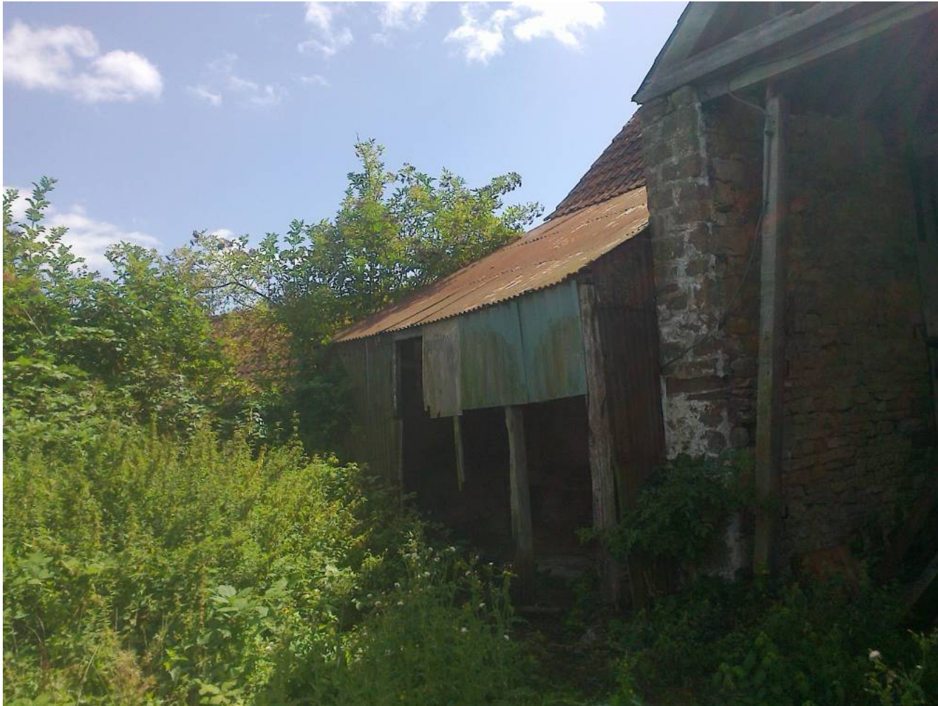
North elevation of the barn showing the timber framed, metal sheeted lean-to which is to be demolished.
