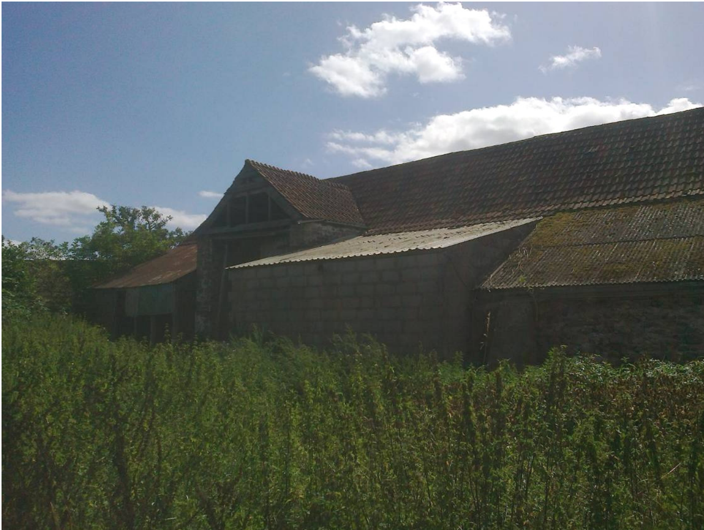
North elevation of the barn showing concrete block extension built to enclose a silo.
