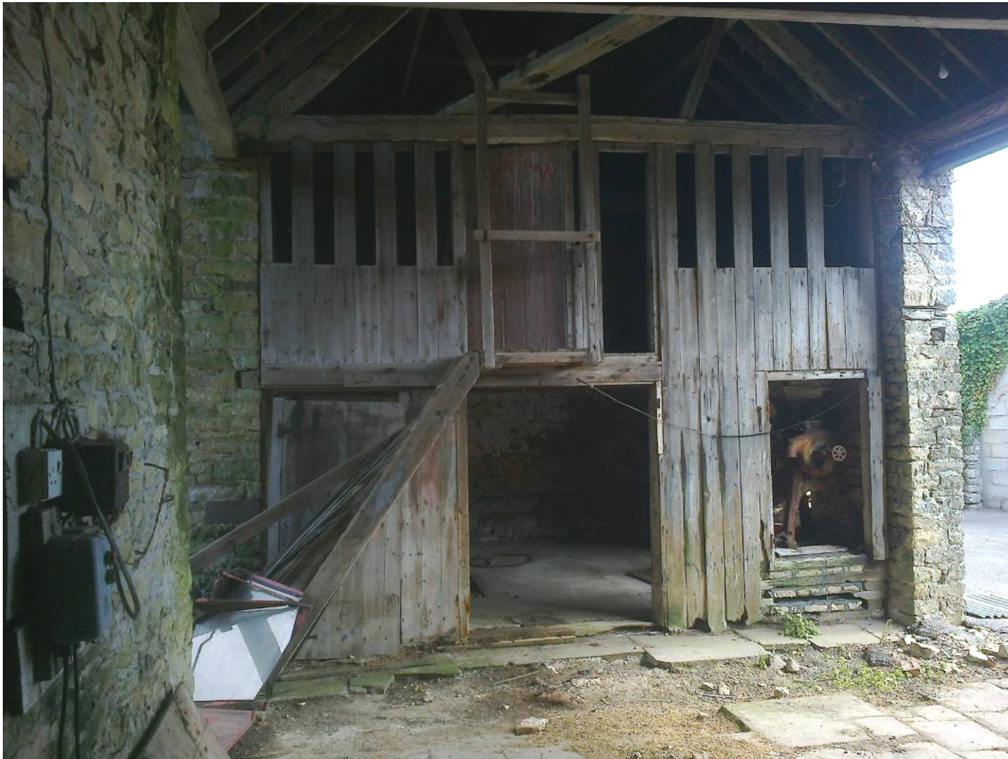
View east showing the partition and stairs between the threshing floor, first floor granary and ground floor process and store room
