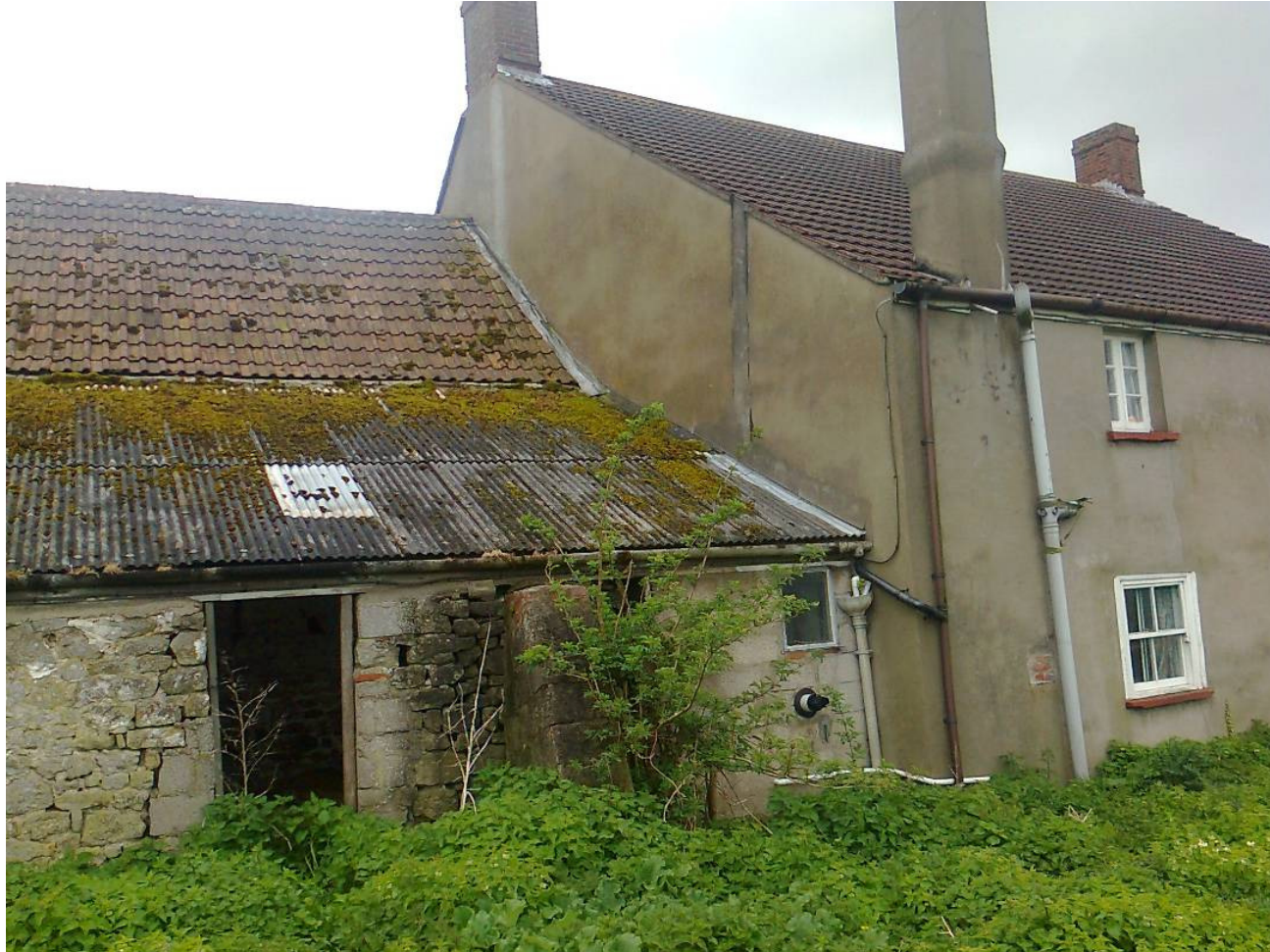
West end of the north elevation of the barn where it joins the existing farmhouse showing the existing lean to part converted into a WC and containing the central heating boiler serving the farmhouse.
