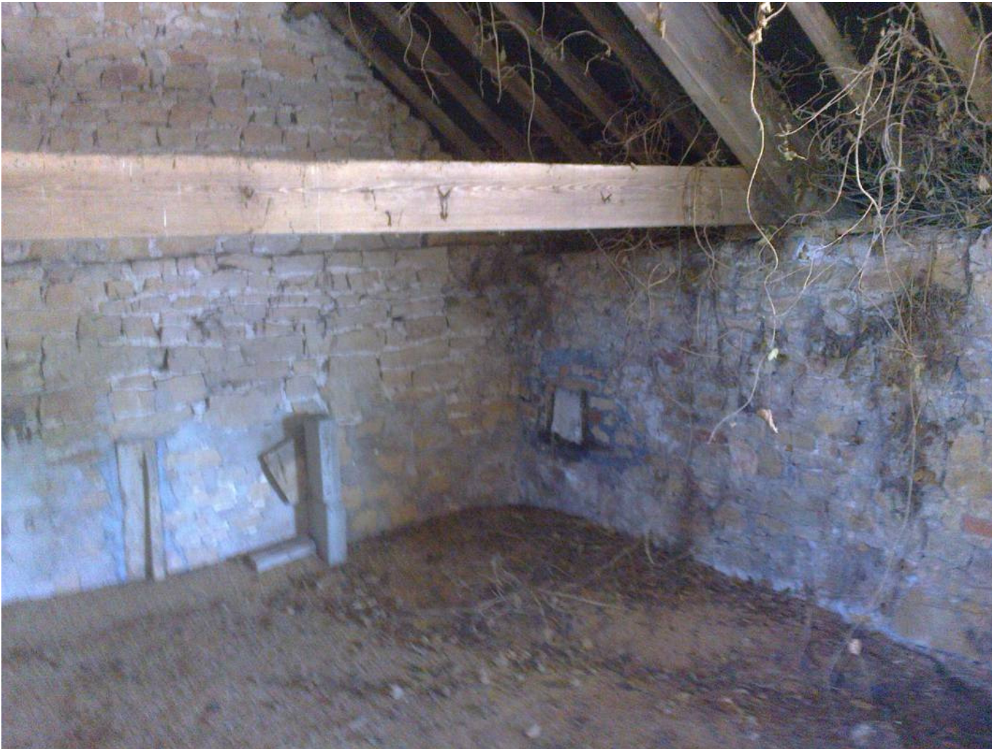
View of south east corner of first floor grain store showing blocked up window opening.
