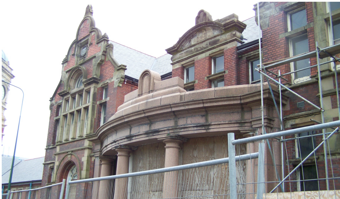
Principal entrance from Steelworks Road June 2008
