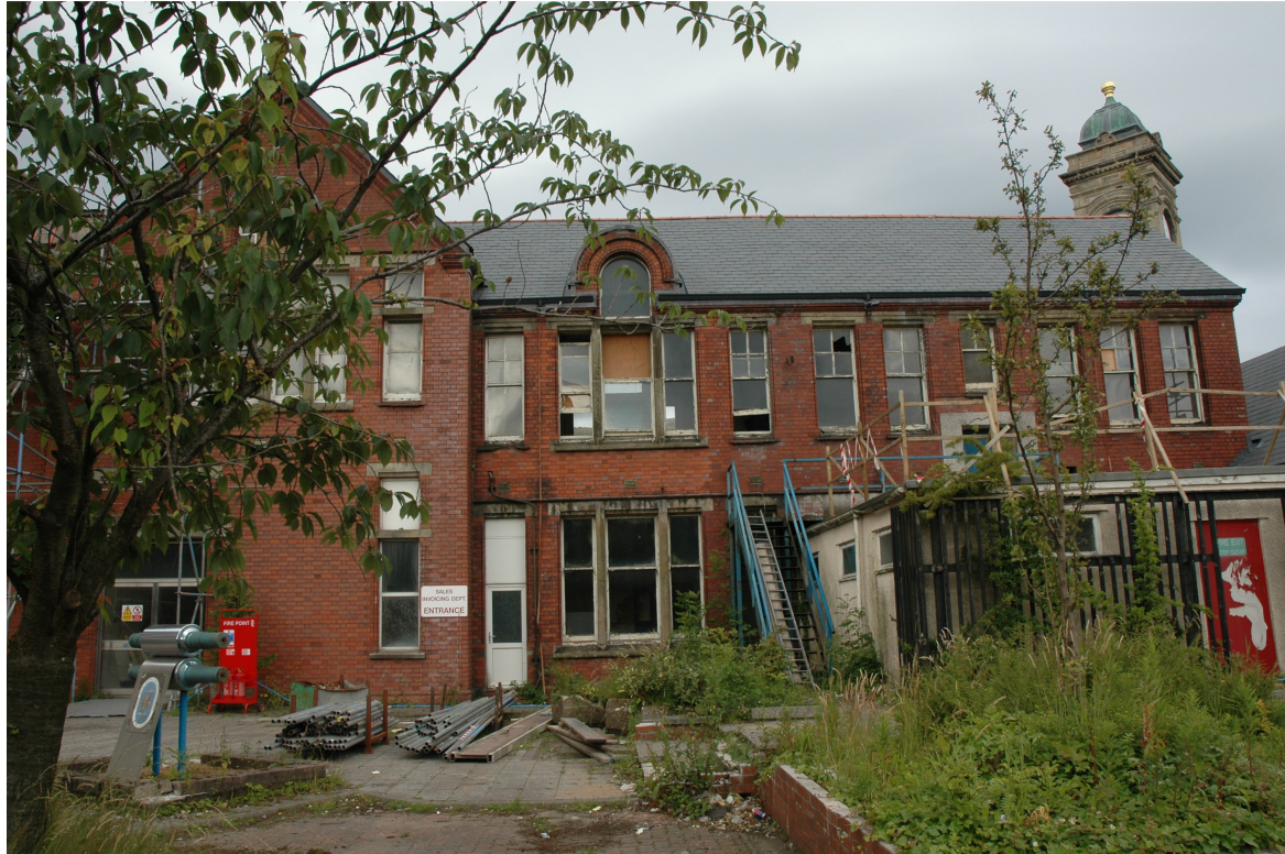
Existing West façade, July 2008
