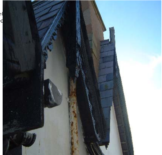
Details of eaves/barge boards and rusting rainwater goods.
