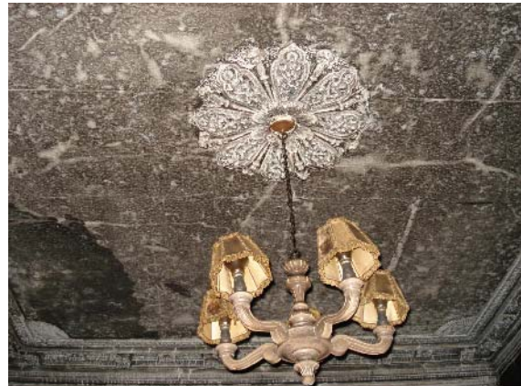
Example of fire smoke damage to ground floor staircase and hall way
