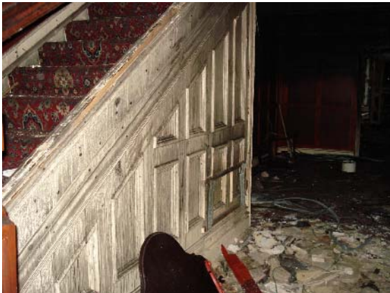
Example of fire smoke damage to ground floor staircase and hall way
