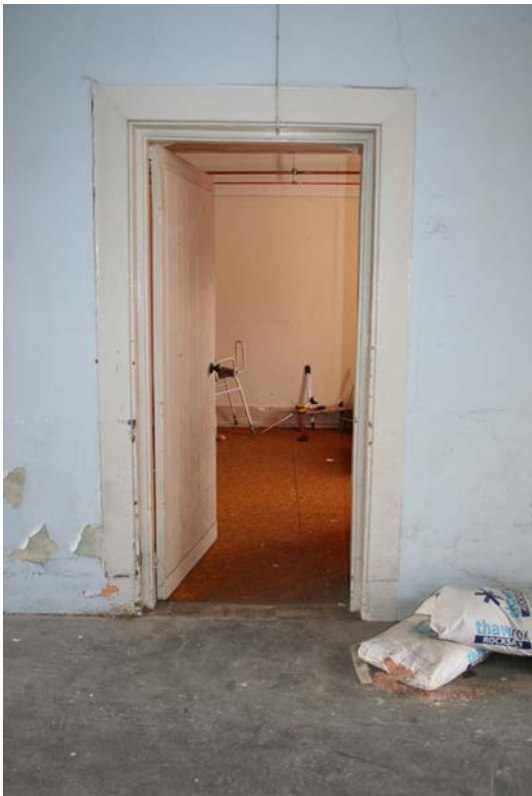
Plate 63: Workhouse north wing
