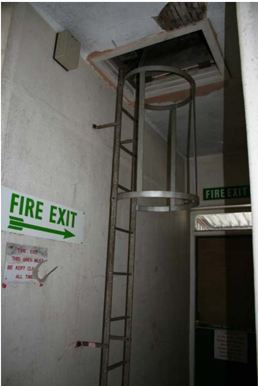
Plate 90: Second floor roof access
