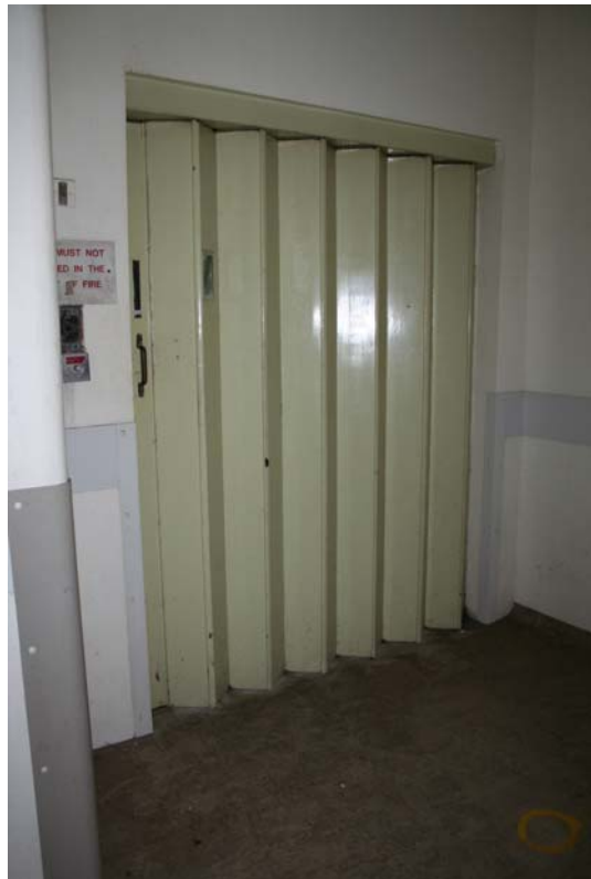
Plate 91: First floor lift access
