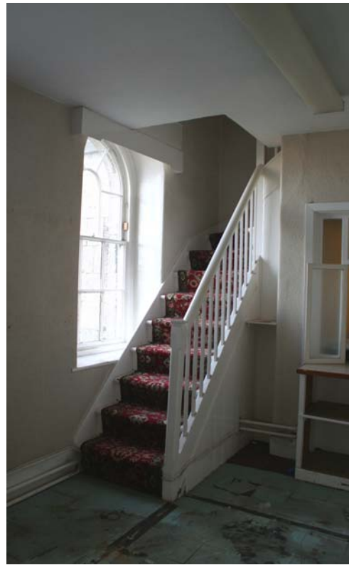
Plate 64: Workhouse flat staircase
