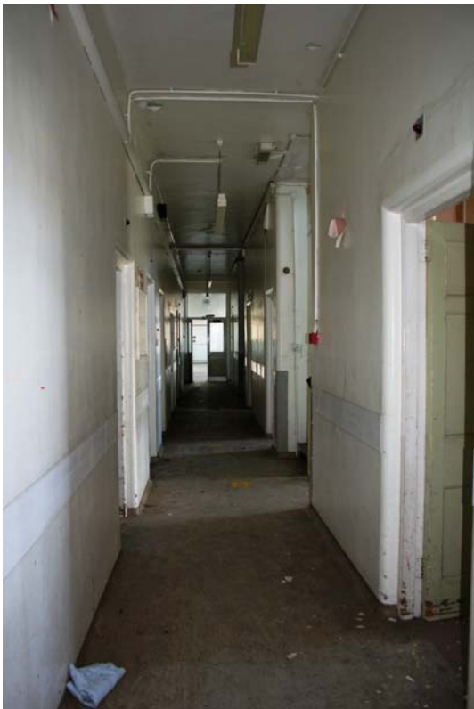
Plate 86: First floor corridor
