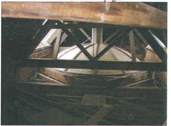
Photo 14: Smaller Attic Space
