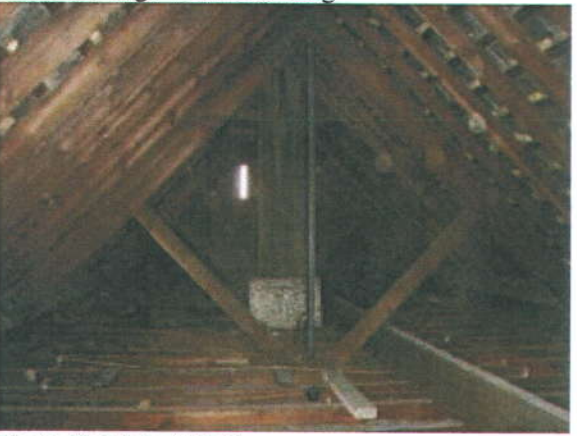
Photo 13: Main Attic Space
