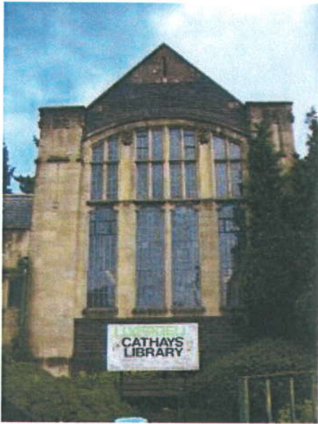
Photo 1: Front Elevation – Eastern Wing
