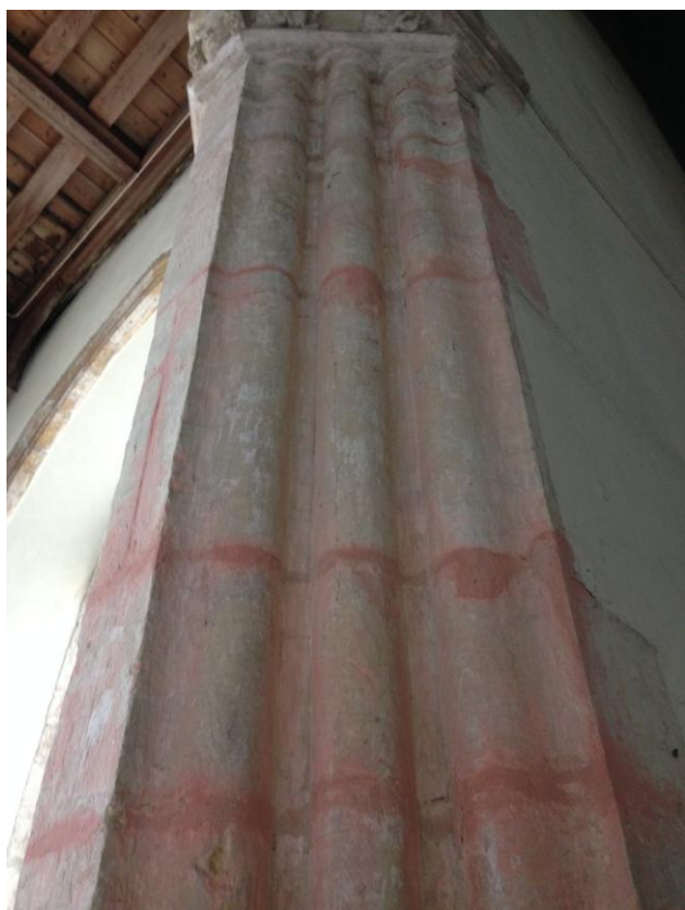
Plate 13 - View looking WSW
