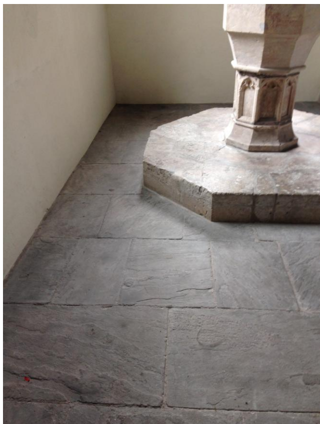
Plate 15 - View looking WSW
