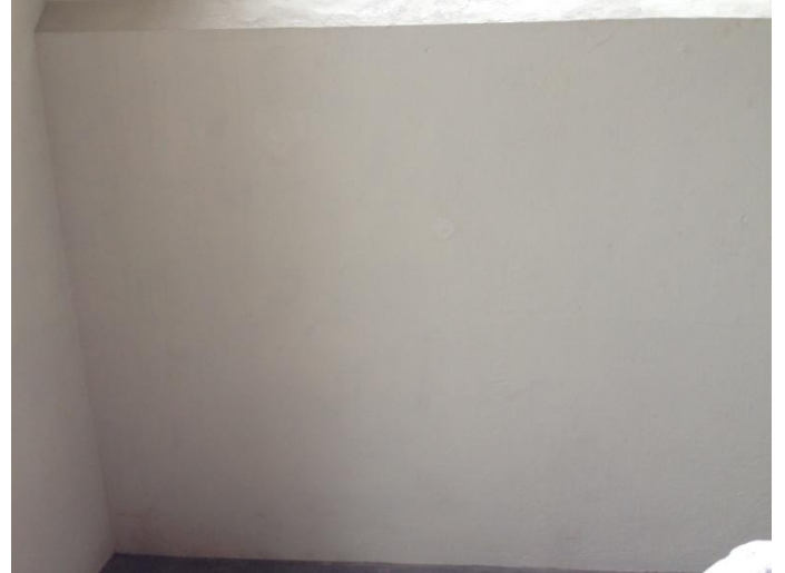
Plate 8 - View looking WSW
