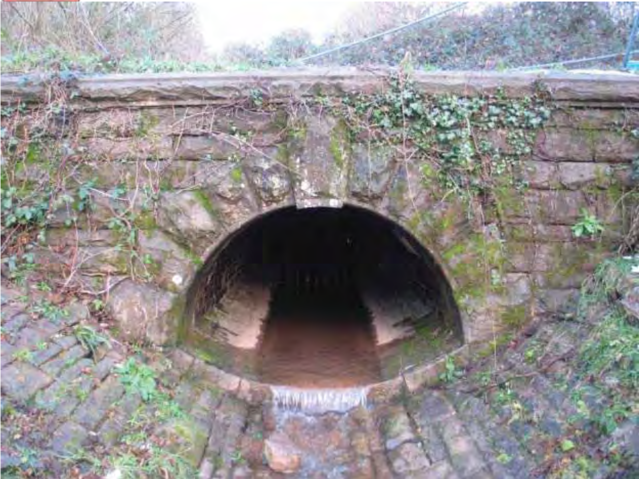
Appendix 4.7: Southern opening of the Nant Mawr discharge culvert
