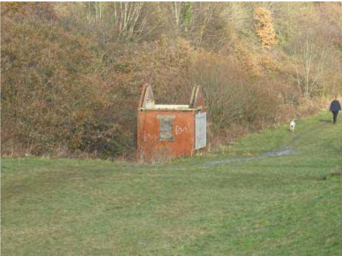
Appendix 5.14: Former Venturi meter well house, view to the northwest
