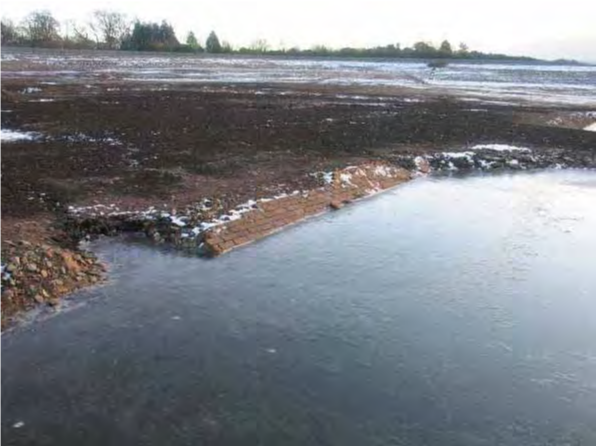
Appendix 5.24: Brick lined former filtering bed, view to the southeast
