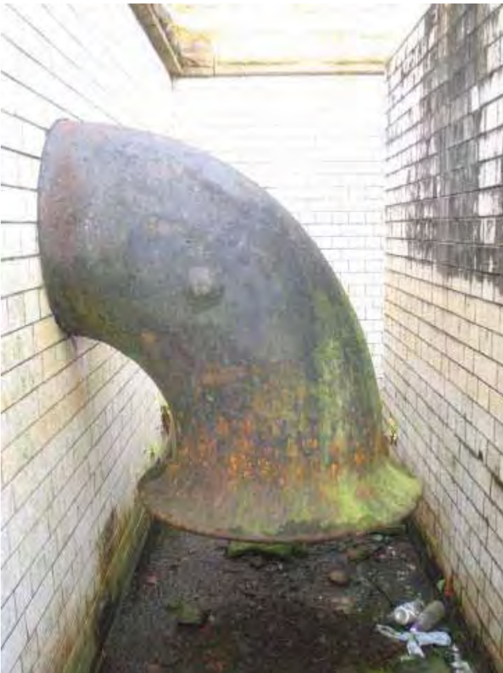
Appendix 4.10: 29" inlet pipe, view to the north
