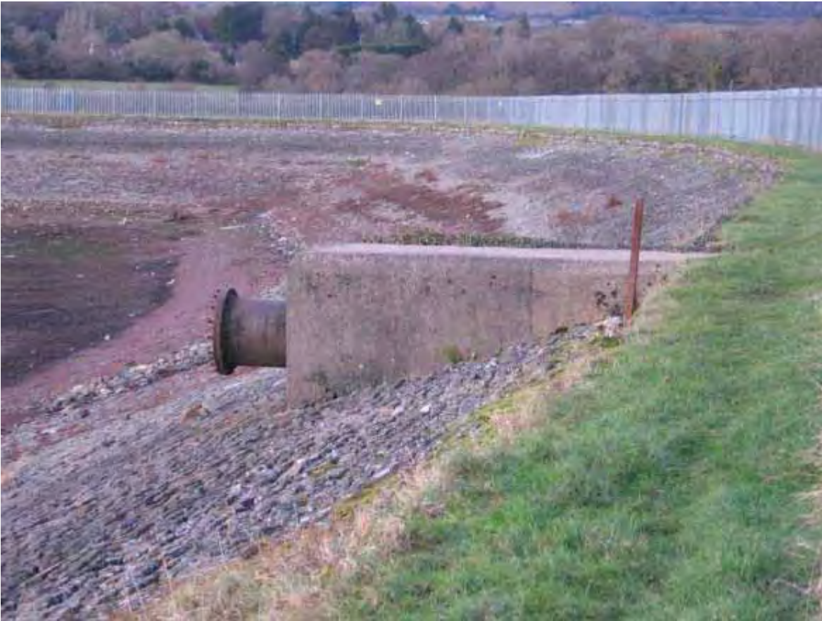
Appendix 5.19: Inserted concrete cased inflow pipe, view to the north
