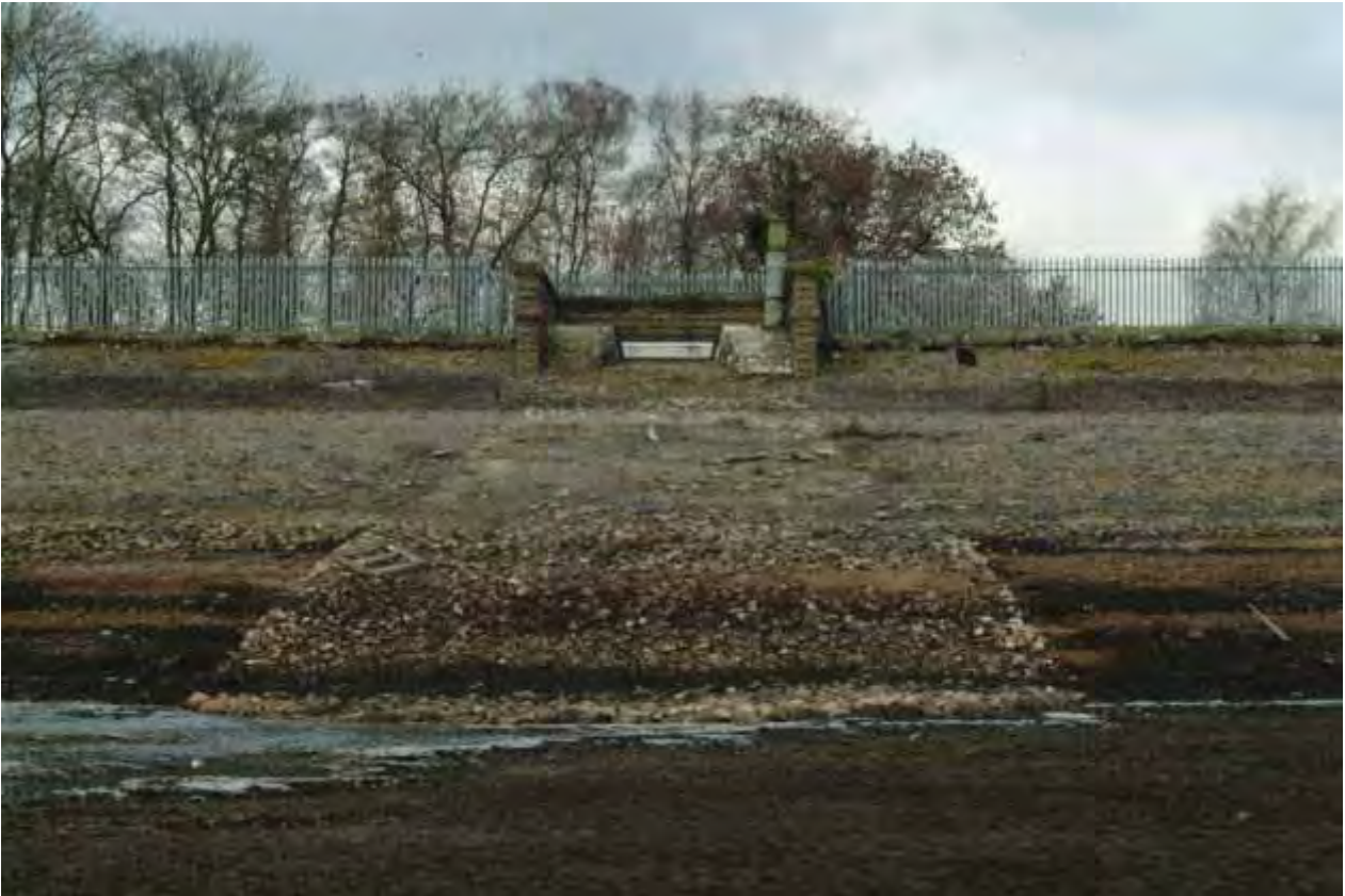
Appendix 5.11: 1930s inlet showing Cipoletti Weir and rudimentary spillway protection
