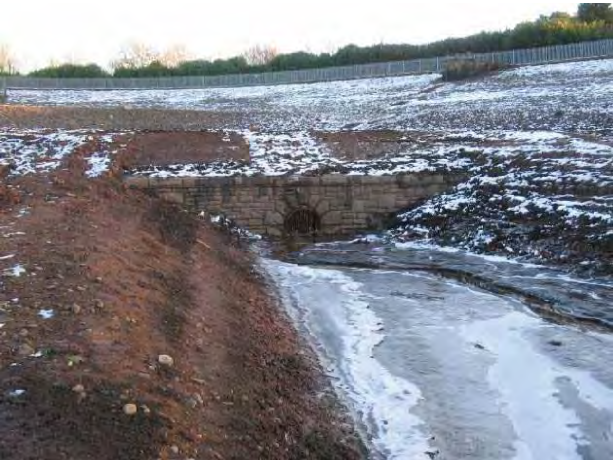
Appendix 5.12: Entrance to scouring culvert, view to the east
