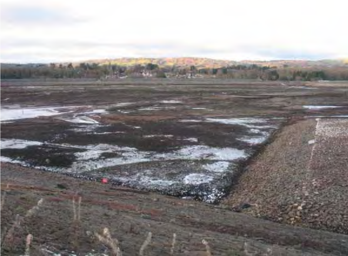
Appendix 5.13: Western edge of raised platform in the southeast corner, view to the north
