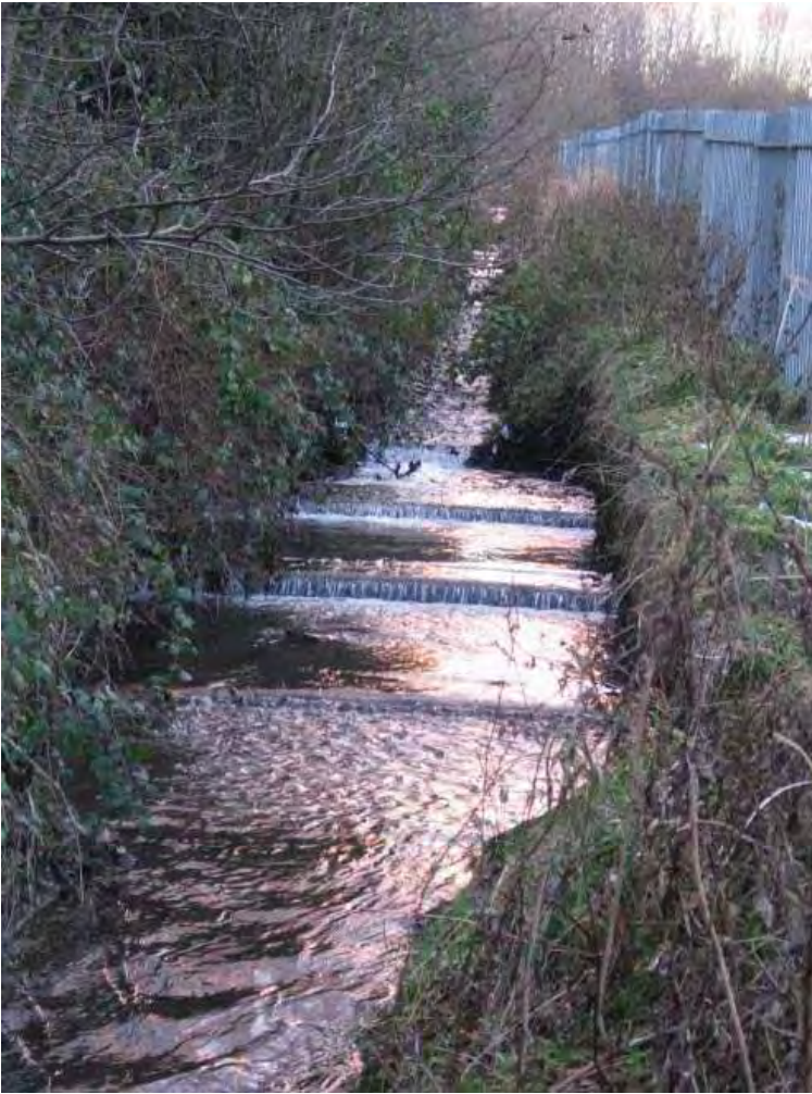
Appendix 5.21: Bye Channel showing stone weirs, view to the west
