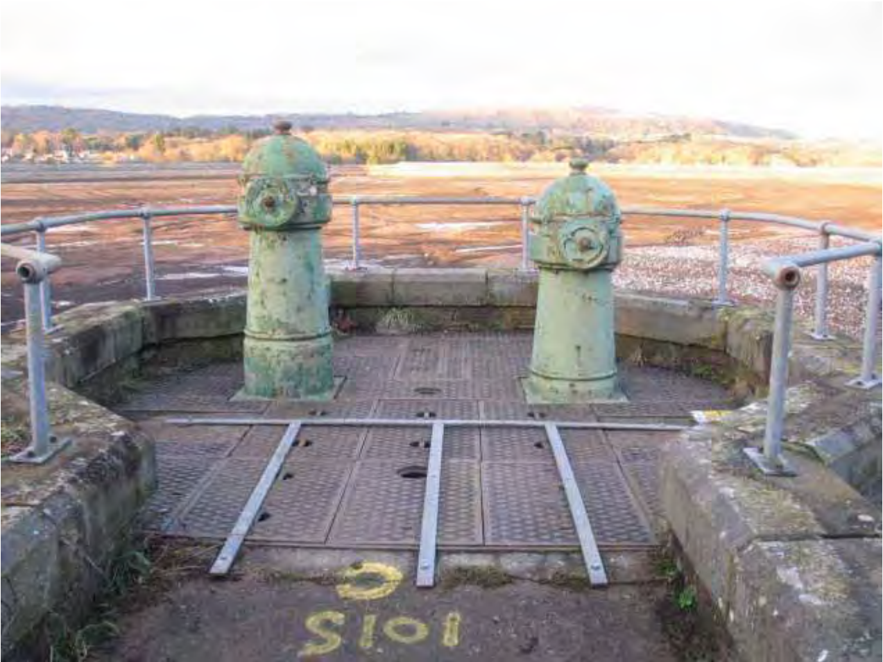
Appendix 4.5: Detail of valve gauges over original valve shaft, view to the north
