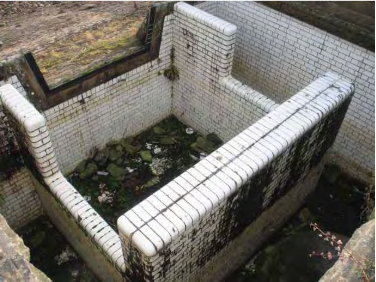
Appendix 4.9: c.1920s inflow tank, view to the southeast
