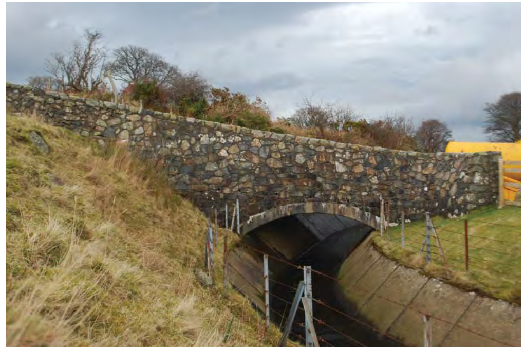
Plate 06: PRN 31897 - Modern Bridge, View From SW
