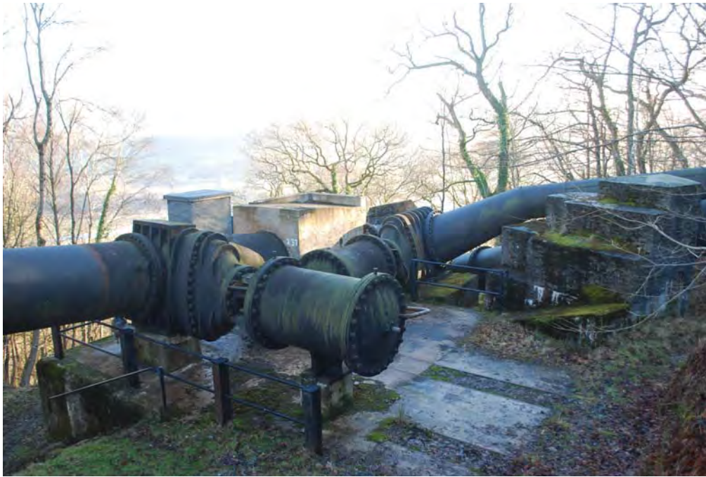
Plate 01: PRN 16321 - Marble Arch Pipe Junction, View From SW
