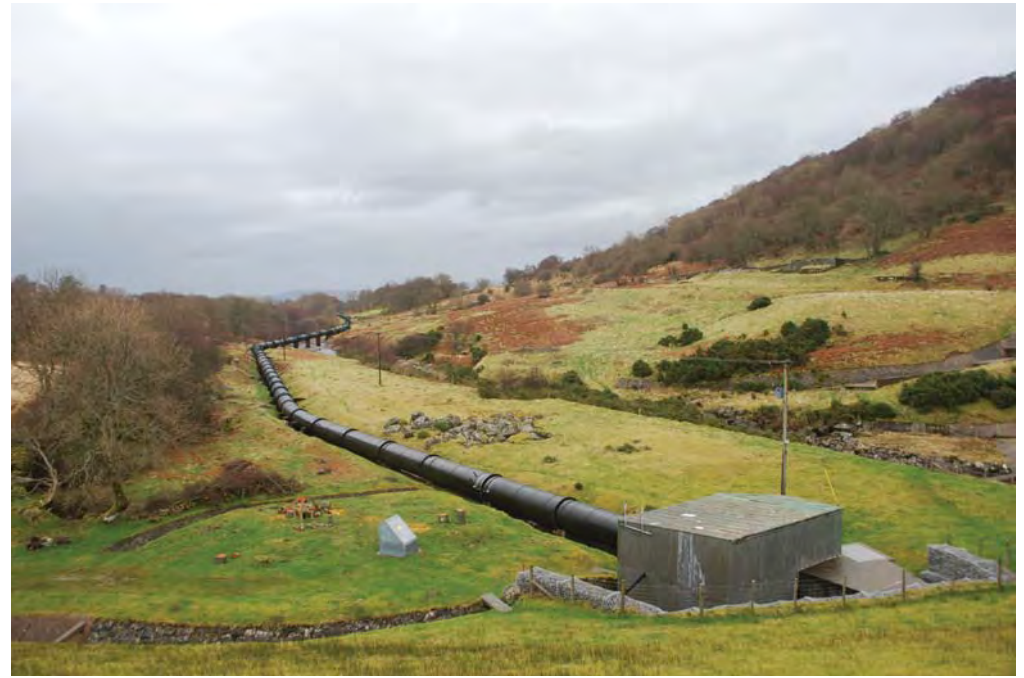
Plate 03: PRN 31890 and 31907 - Llyn Coedty Valve House and Pipe, View From SW
