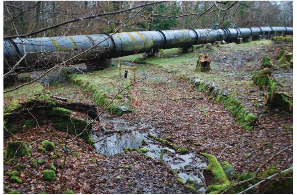
Plate 38: PRN 31965 - Drainage Channels, View From South
