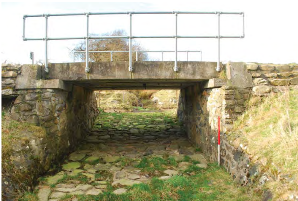
Plate 44: PRN 31974 - Channel for Stream Passing Under Leat, View From SE
