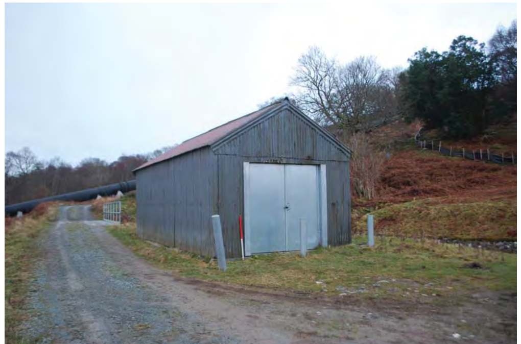
Plate 31: PRN 31952 - Former Locomotive Shed, View From NNW
