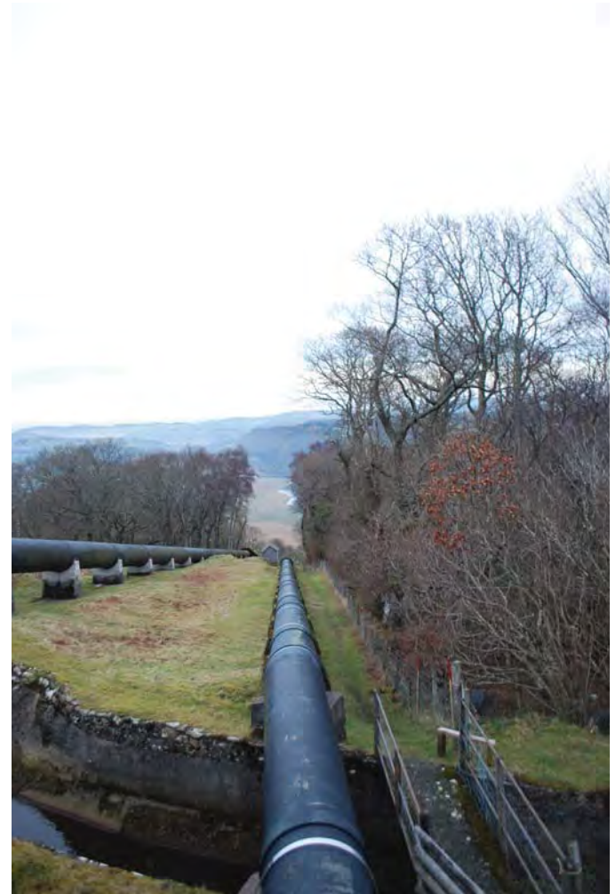
Plate 24: PRN 31934 - Incline and Water Pipe, View From SW
