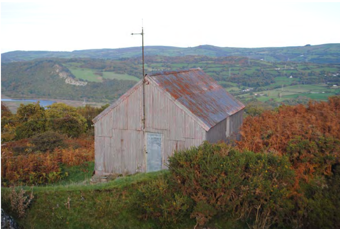
Plate 6 Former engine shed of the Llyn Colwyd Tramway at the former Coed Sadwrn Yard
