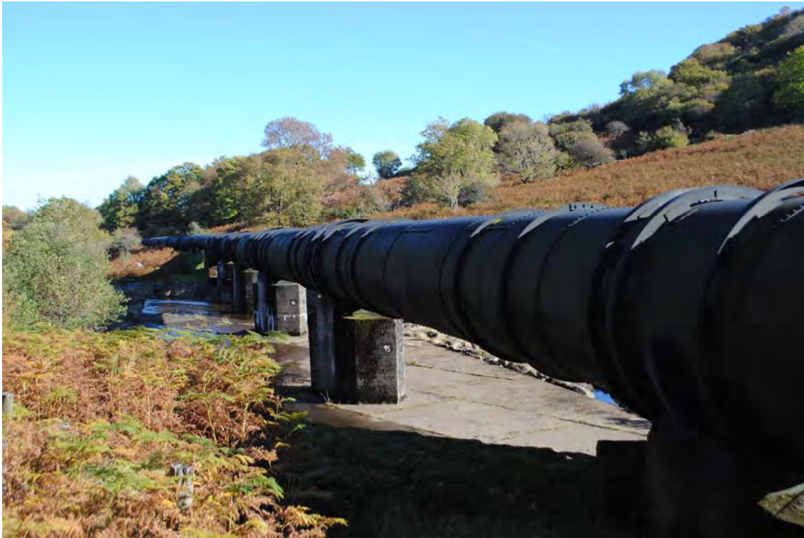
Plate 1 The pipeline (Feature 25) as it crosses the Afon Porth Llwyd
