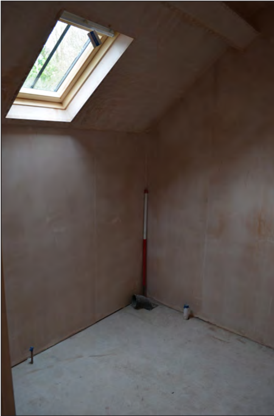
Plate 17: Internal view of bathroom adjacent to front bedroom (Scale 1 x 1m).
