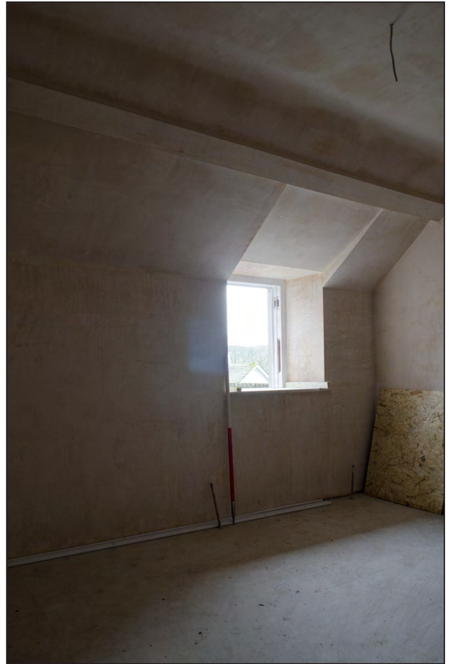
Plate 16: Internal view from northwest of first floor room (Scale 1 x 1m).
