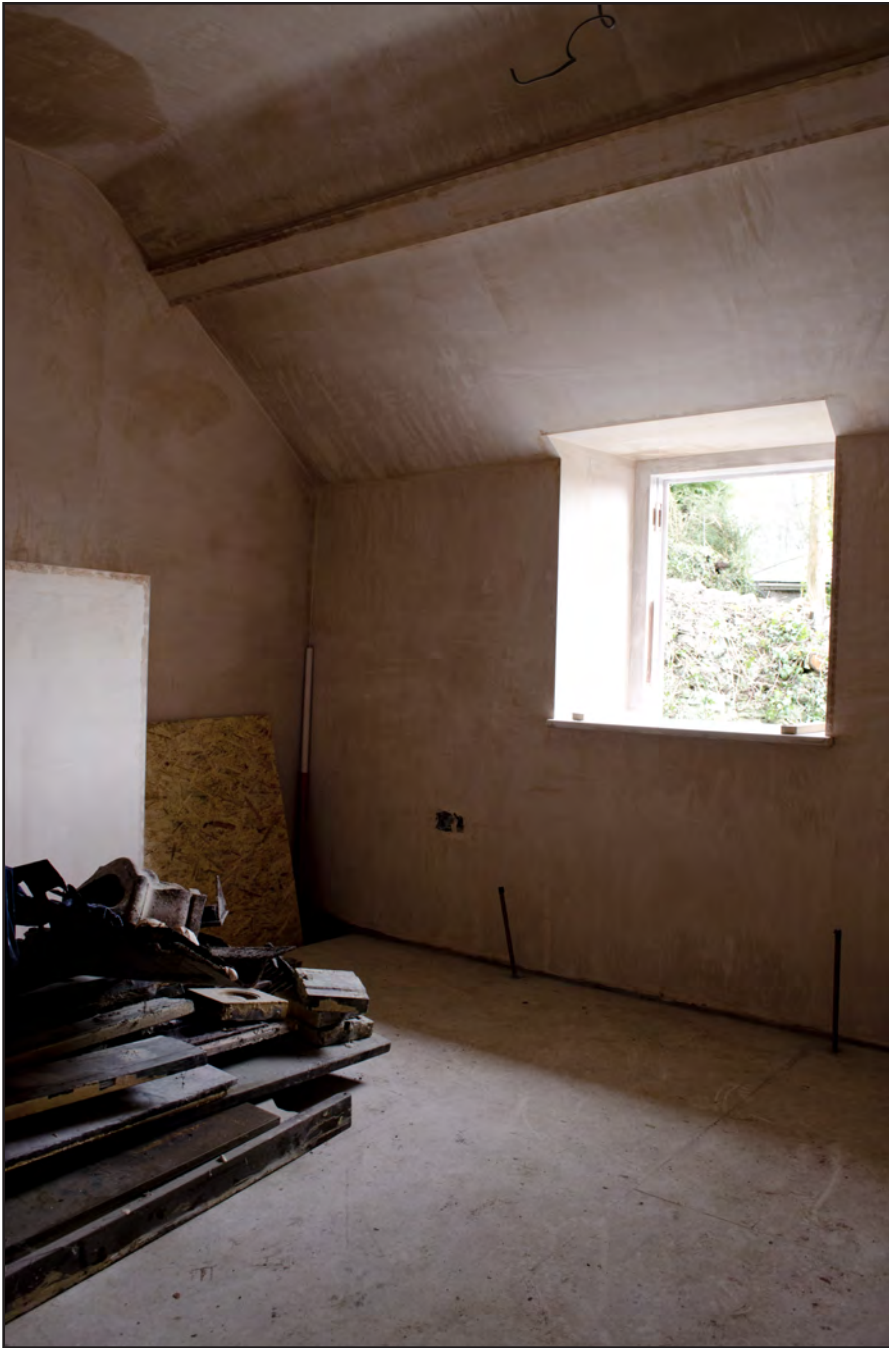
Plate 15: Internal view from southwest of first floor room (Scale 1 x 1m).
