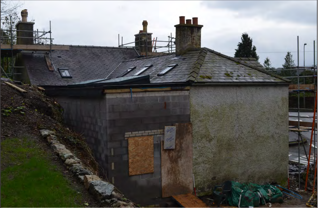
Plate 08: Detail of western end of Nant Cottage.
