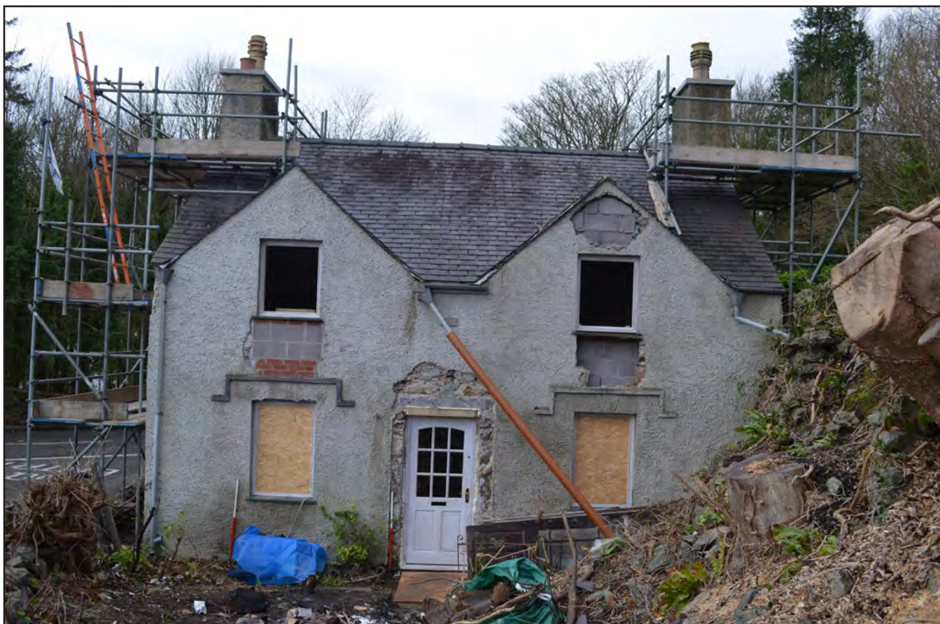
Plate 02: View from the east of eastern elevation (Scale: 1 x 1.0m)
