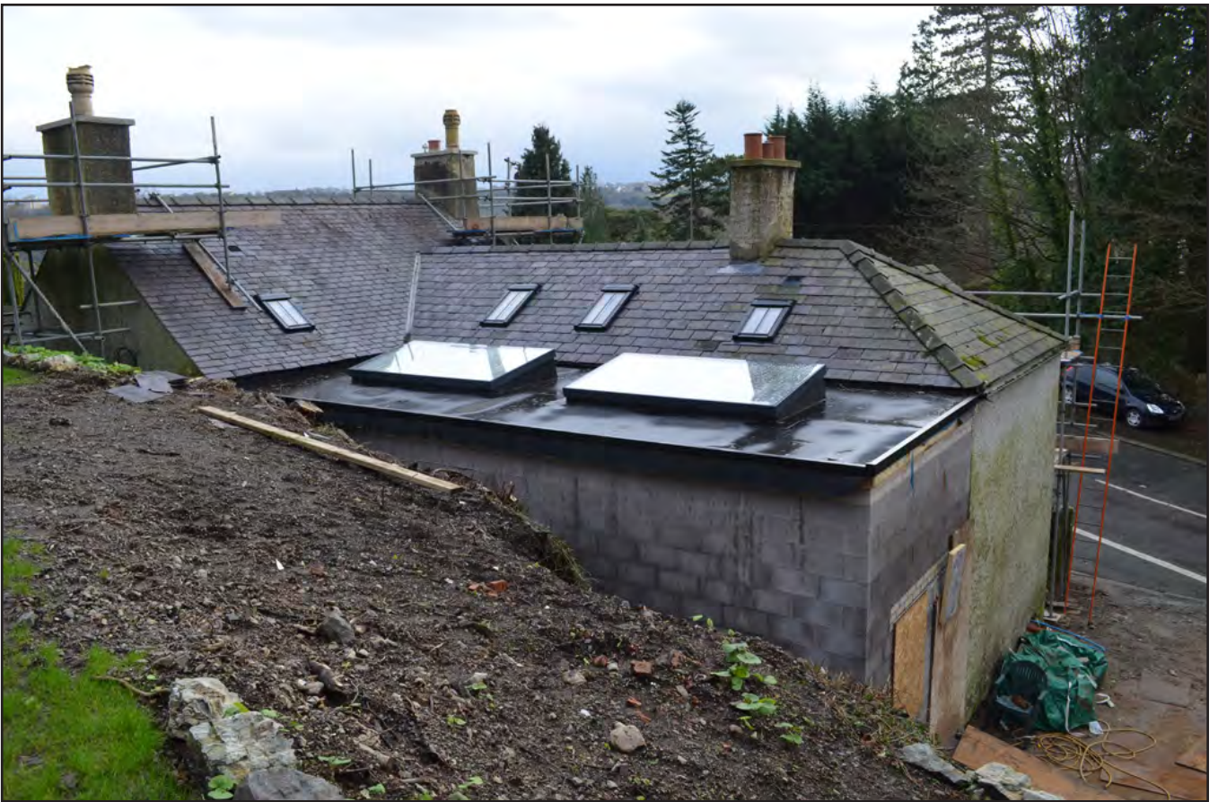
Plate 07: Northern elevation of the cottage with view of pitched roof.
